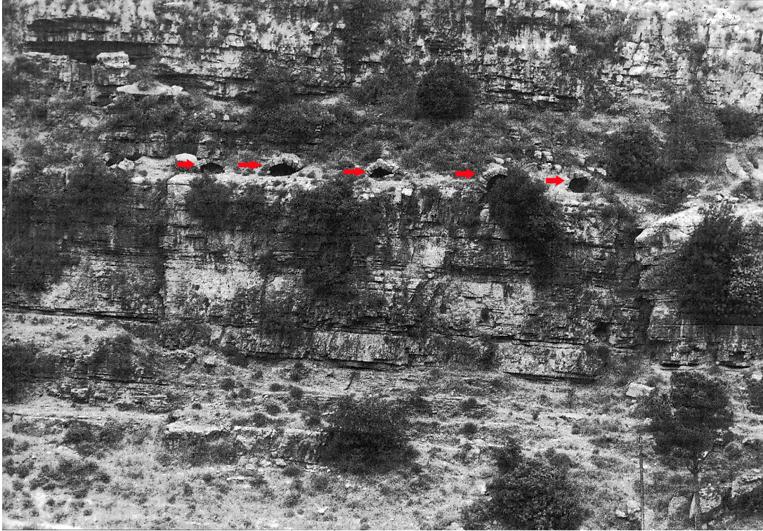
Fig. 6.13: Vaulted covers over the tunnel shafts (indicated by red arrows), Beirut, Lebanon [Davie et al. 1997, pl.11.2].
