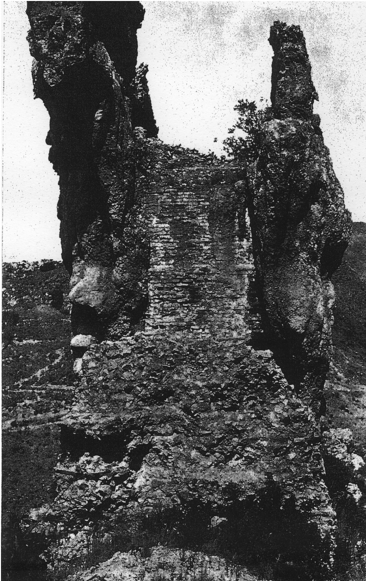
Fig. 6.16: Brick pier on Antioch- south bridge, south-eastern Turkey [Wilber 1938, fig. 5].
