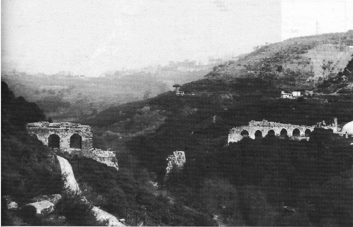
Fig. 6.17: View of the Beirut bridge, Lebanon [Davie et al. 1997, fig. 1].
