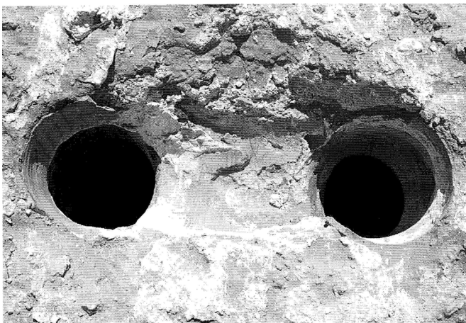
Fig. 6.22: Hydraulic device on the Caesarea southern pipeline, view from above [Porath 2002b, fig. 17].
