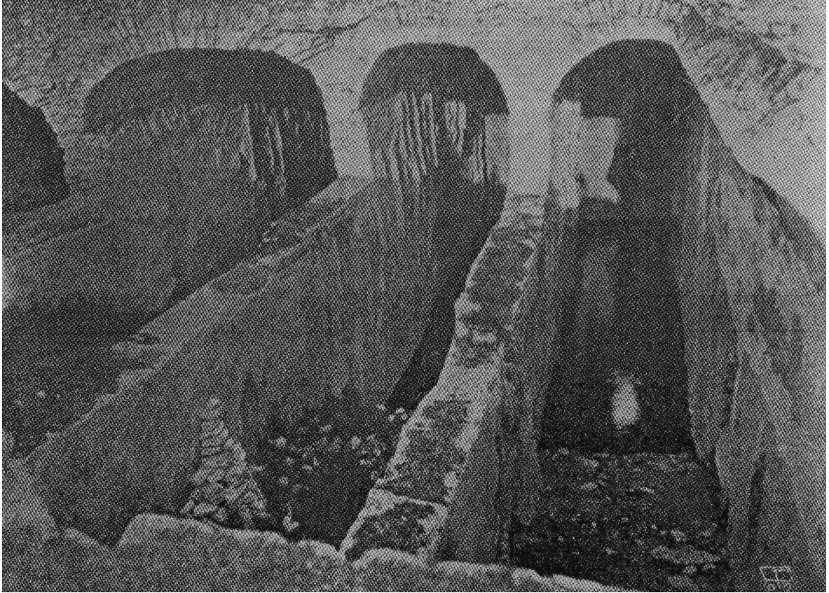
Fig. 7.27: The reservoir-cistern at Dara [Preusser 1911, fig. 57].
