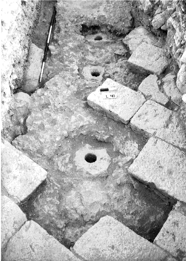
Fig. 7.40: Holes in the stone pipeline at Hippos/Susita [Tsuk et al. 2002, fig. 1].
