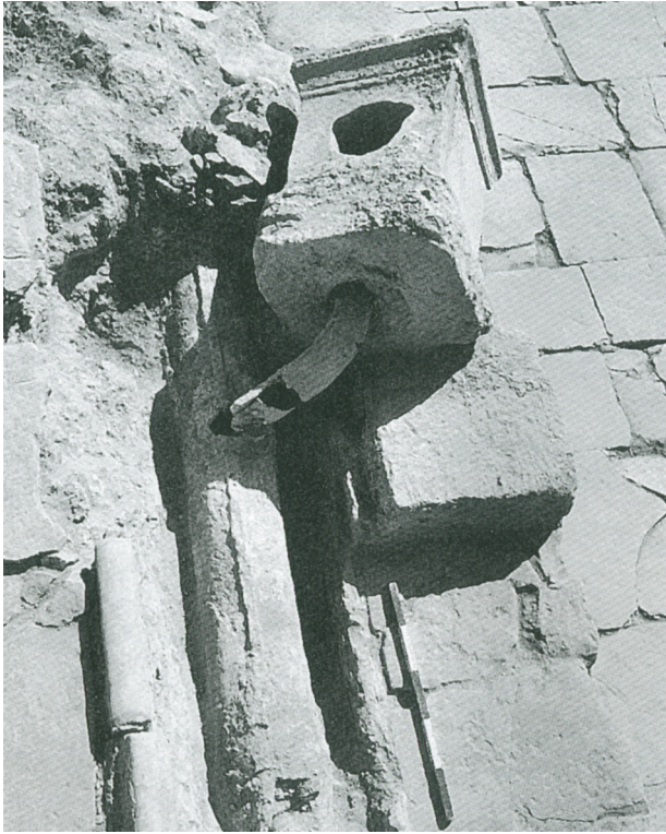
Fig. 8.21: Lead pipe network feeding fountain at the edge of the pool in Area D [Hirschfeld 1997, fig. 45].
