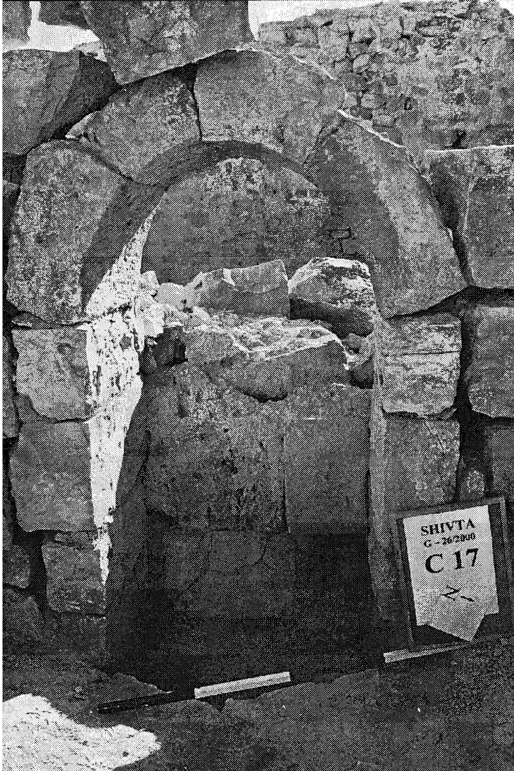
Fig. 9.12: Cistern no.17, Sbeitih/Shivta. A hole, 15 mm large, was found in the arch structure that may have been used for a pulley system over the recessed draw-shaft [Tsuk 2002c, fig. 3].
