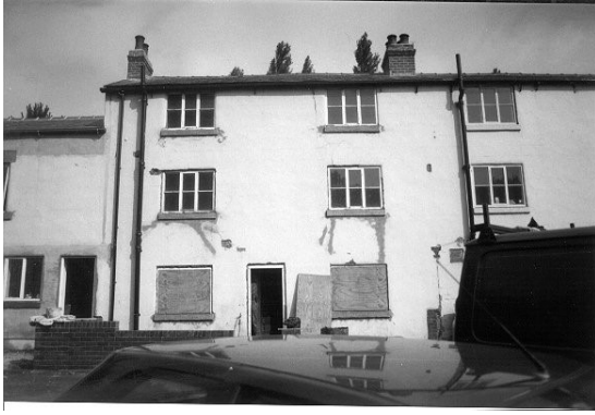
01/29 Cottages, west of centre, exterior facing N
