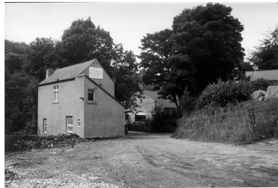
02/13 Counting House exterior facing SW
