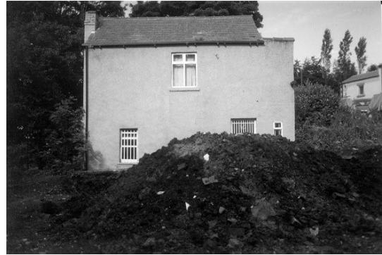
01/24 Counting House exterior, facing W
