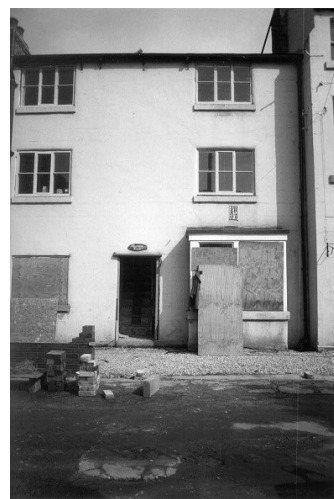
01/28 Cottages, east of centre, exterior facing N
