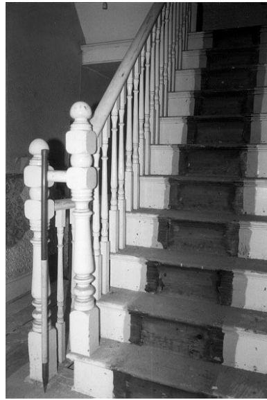
02/11 Cottages interior, easternmost, 1 st floor detail of banister facing N
