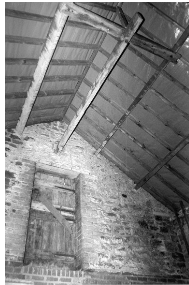
01/34 Dam House interior, detail of taking-in door and hoist facing NE
