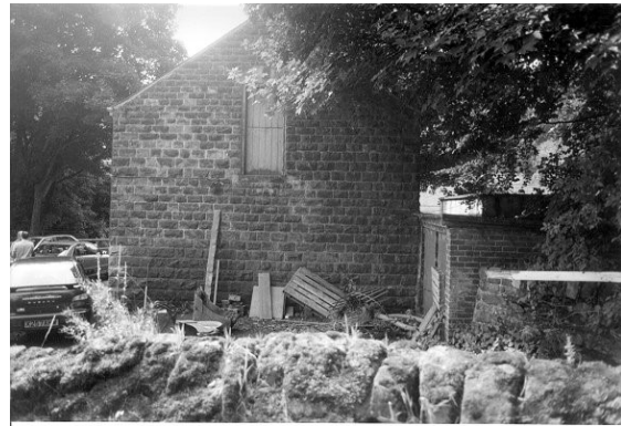
01/32 Dam House exterior facing S
