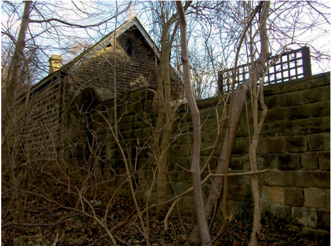
Plate 17 – E view along terrace wall to Annex
