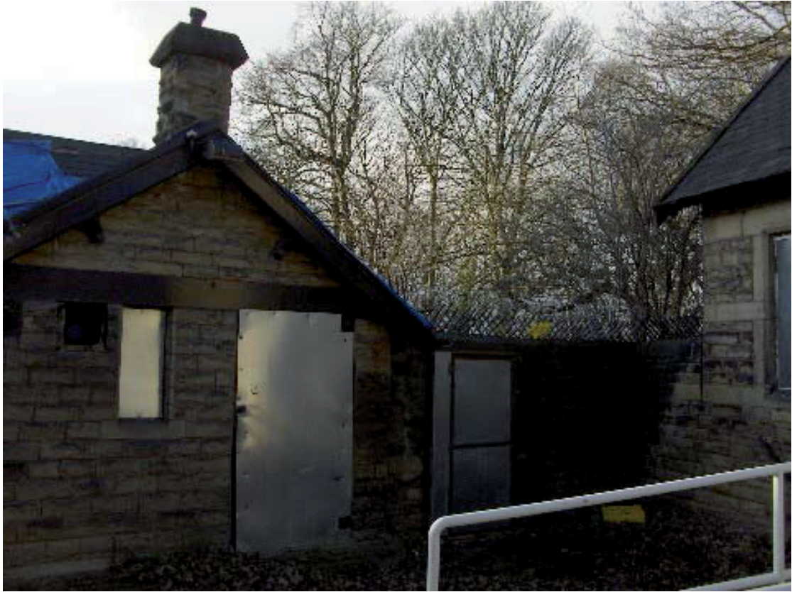
Plate 28 – W view of connecting wall between house (left) and Annex (right)
