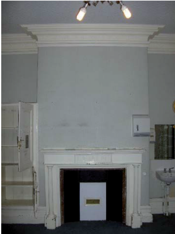
Plate 39 – Fireplace and ceiling cornice in intermediate room
