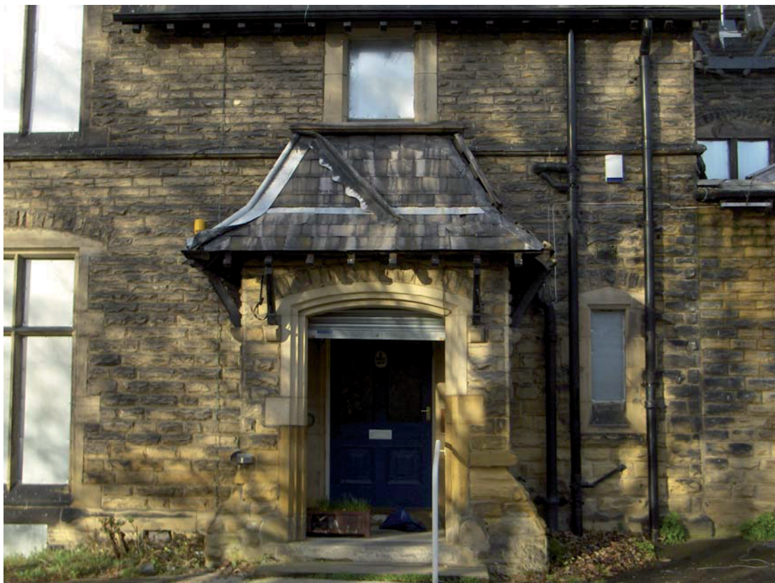
Plate 19 – Detail view of main entrance
