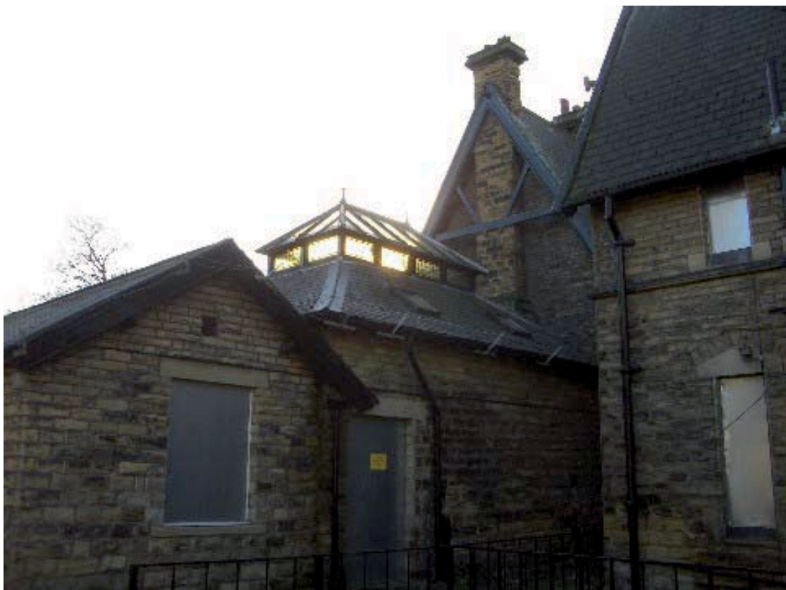
Plate 27 – South wing of house, looking S
