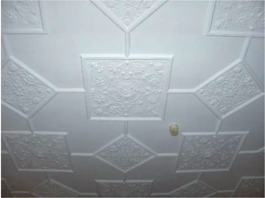
Plate 42 – Ceiling moulding in north-west room
