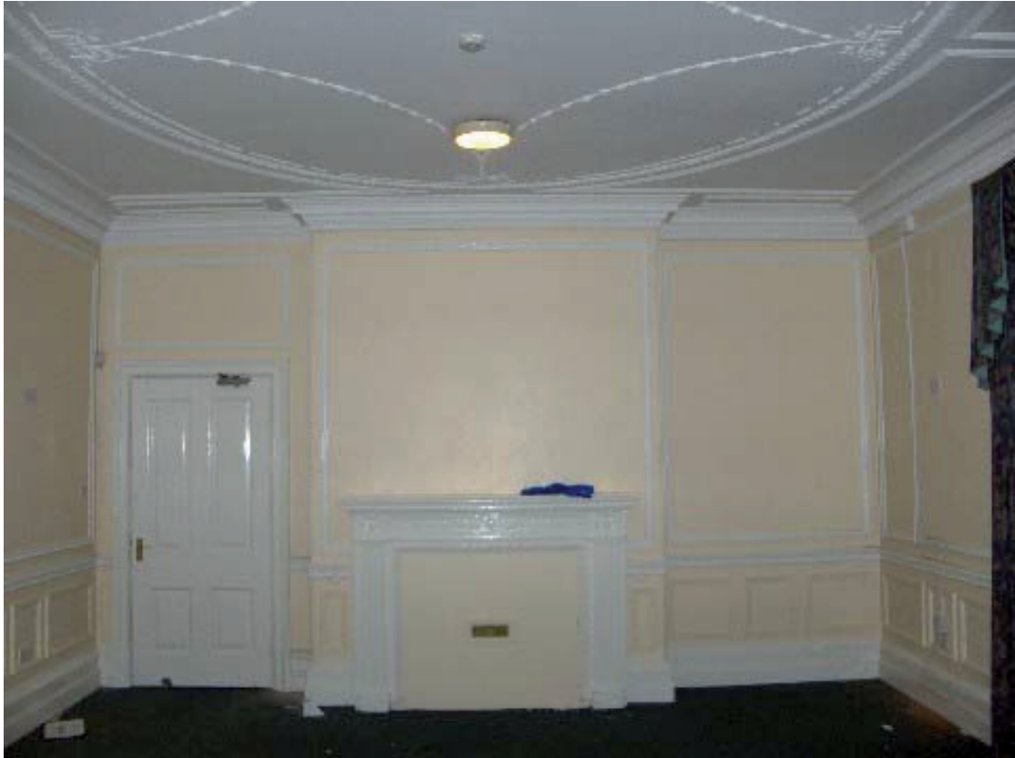
Plate 38 – Principal room showing fireplace, skirting board, dado rail and mouldings and ceiling with cornice and mouldings
