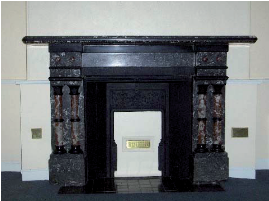
Plate 41 – Detail of fireplace in north-west room
