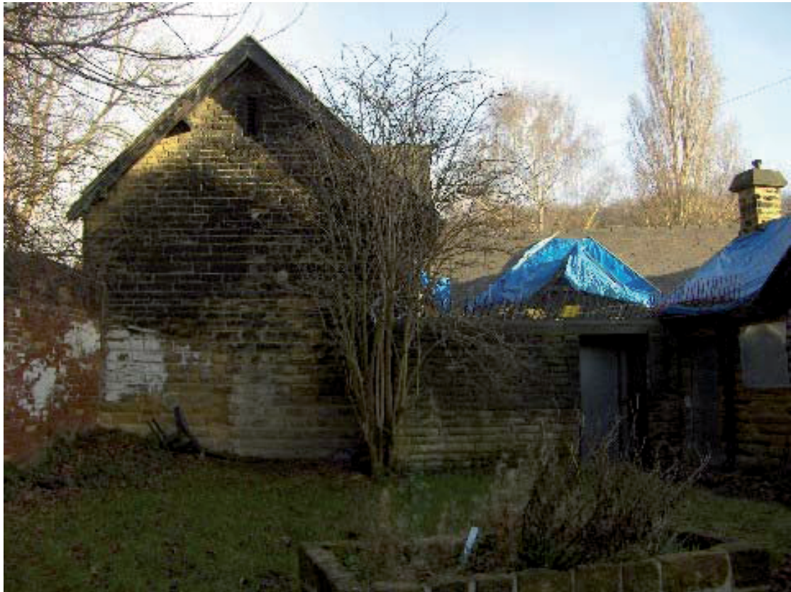
Plate 24 – E view of Annex
