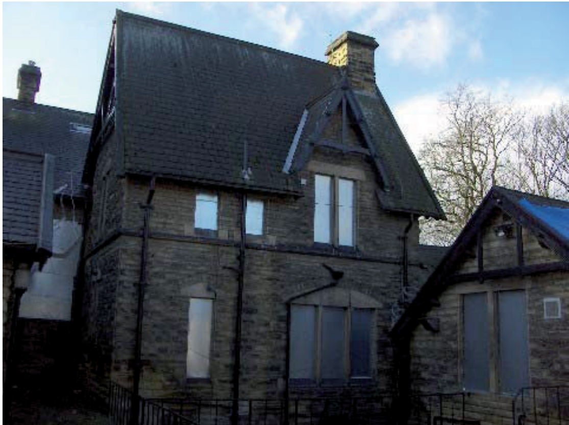
Plate 26 – NE elevation of house
