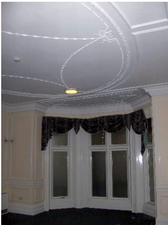
Plate 37 – Principal room showing bay window and ceiling mouldings
