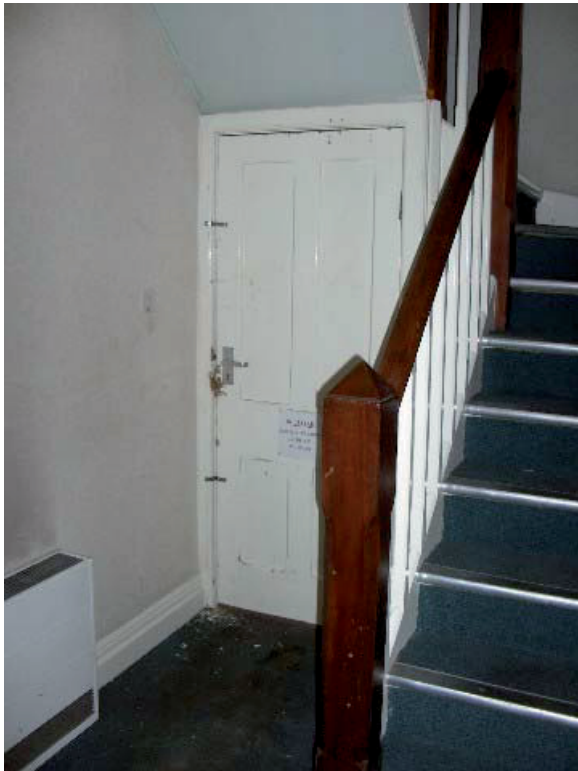
Plate 43 – Existing access to basement
