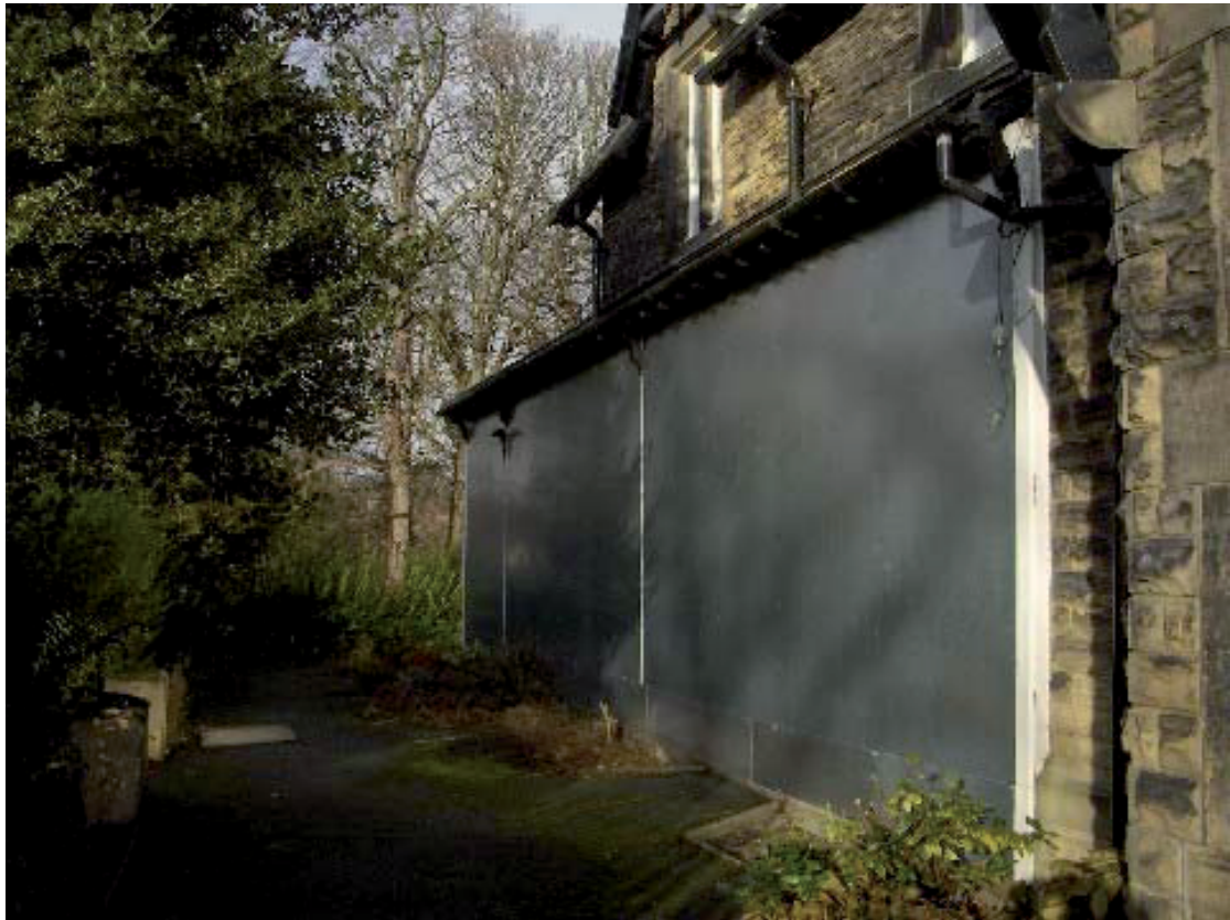
Plate 20 – NW view along terrace of SW elevation of house
