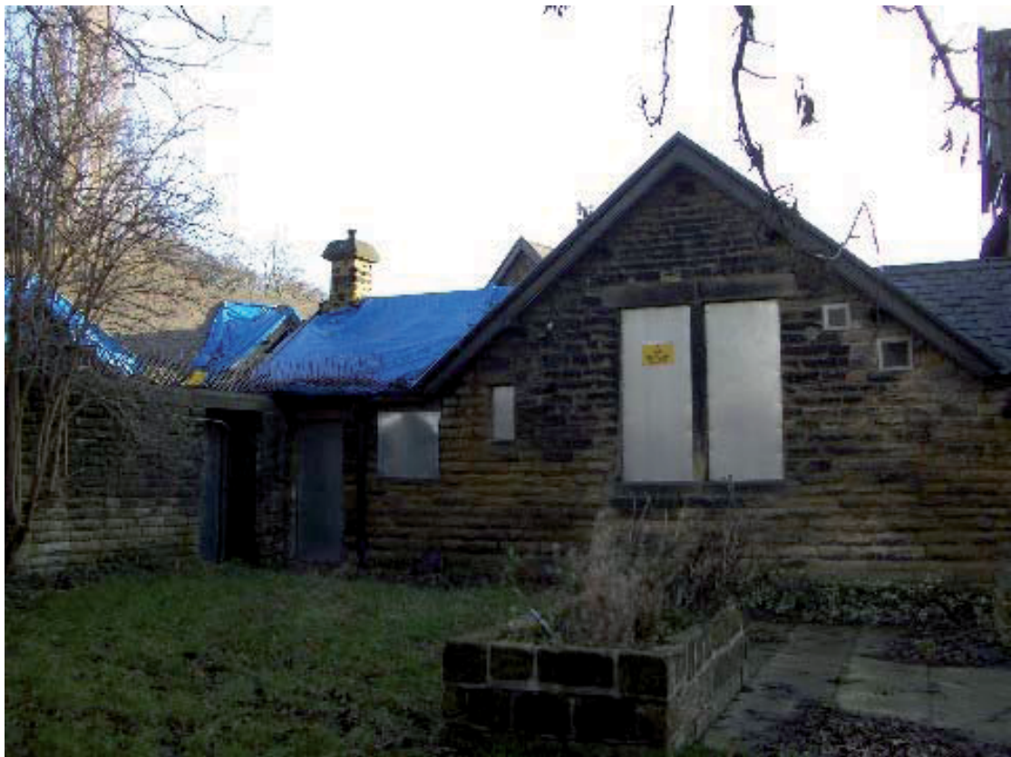
Plate 23 –E view of NW elevation of house towards Lodge
