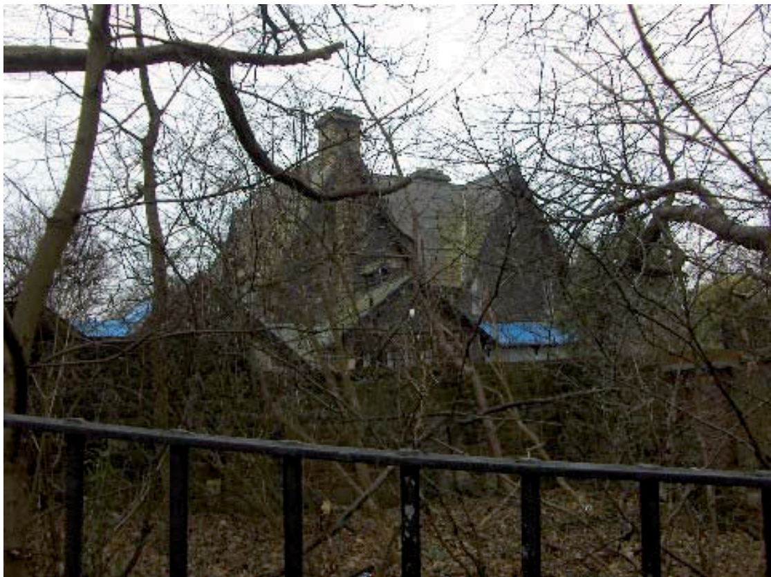
Plate 33 - SE view of house from boundary fence
