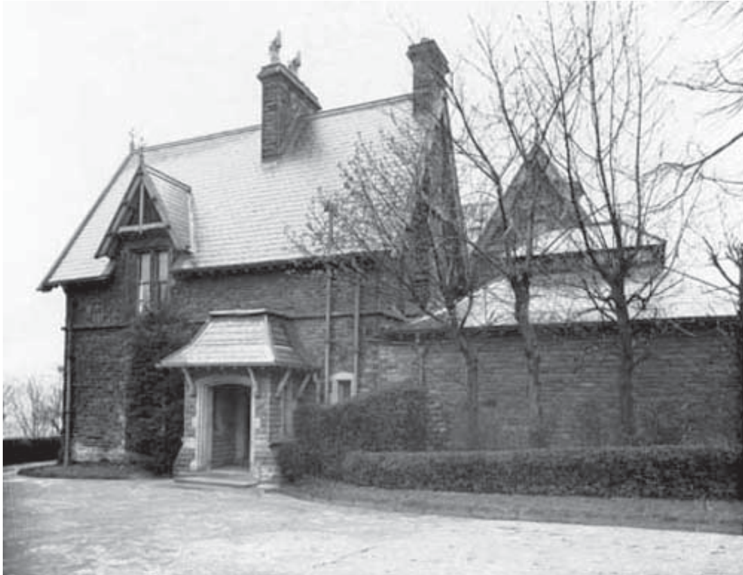
Plate 5 – Main entrance. Crooked Acres, 1937 © Leeds Library & Information Services
