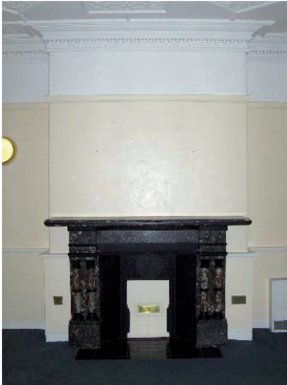
Plate 40 – North-west room showing fireplace and ceiling detail
