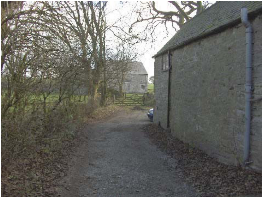
Plate 12. View looking east further along lane towards field barns in background.
