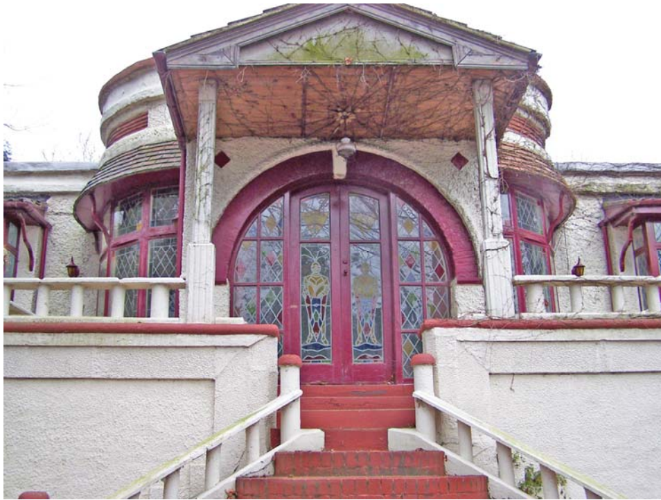
Plate 5: Detail of the entrance hall, Station Road frontage of number 7 showing brick-built staircase, timber-built porch, decorated glass panes and art-deco elements.
