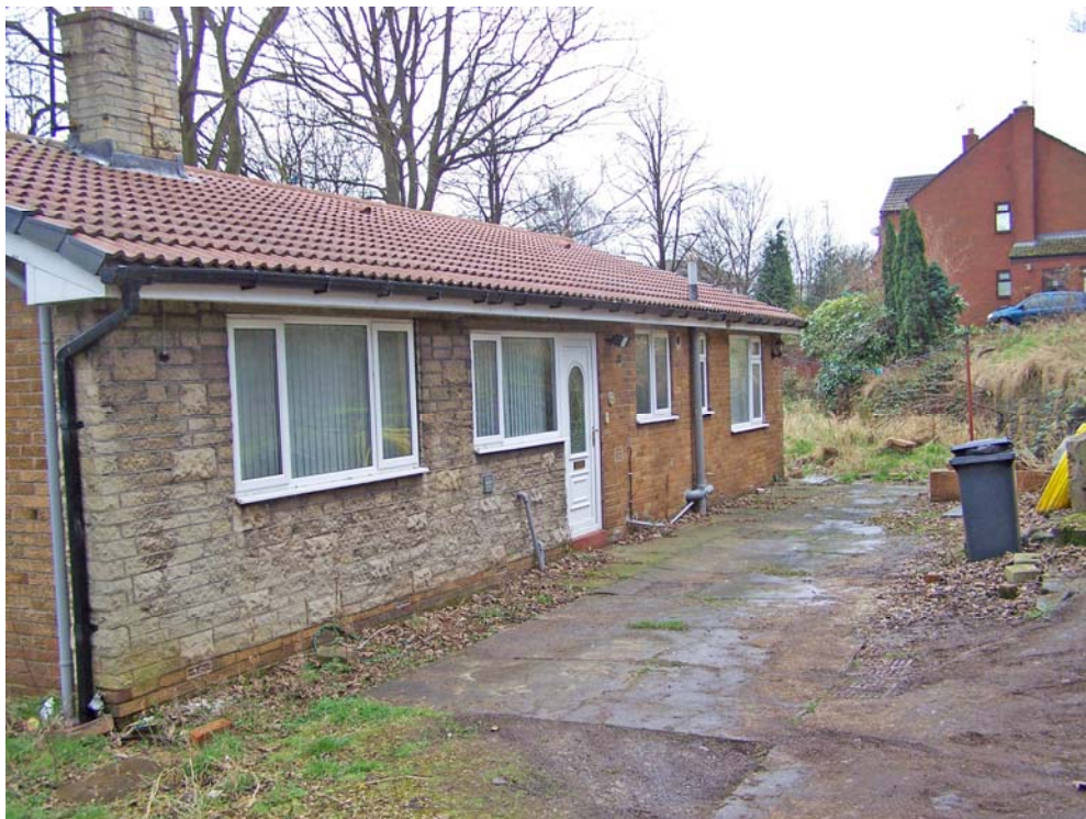
Plate 2: Southwest facing elevation of 5 Station Road, looking east.
