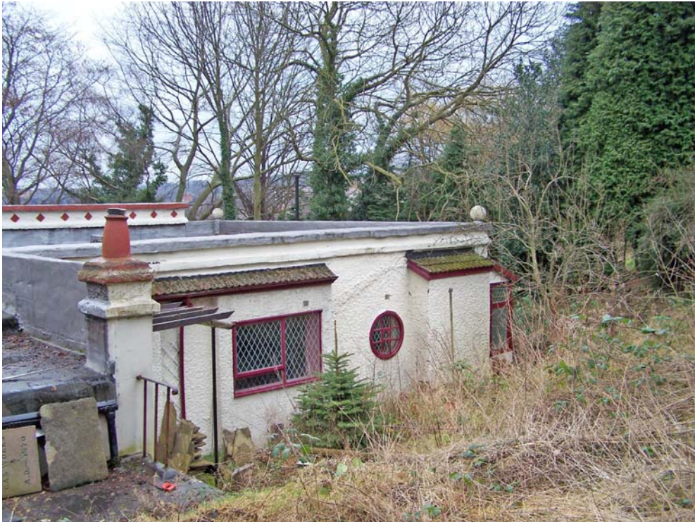
Plate 8: View of rear of property, looking east.
