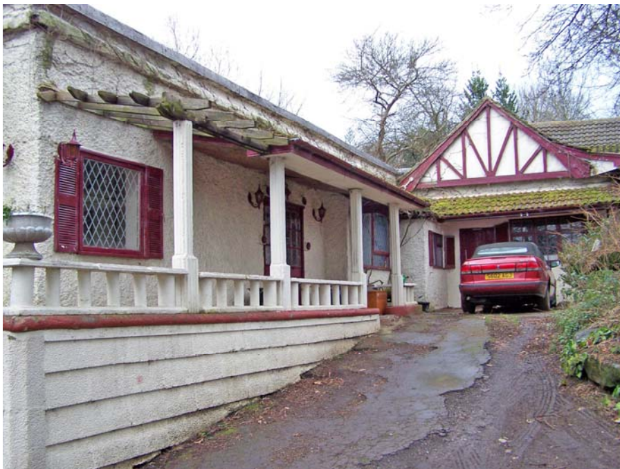
Plate 6: View of northwest facing elevation of 7 Station Road showing continuation of balcony to meet rising ground surface, and northeast facing elevation of north wing.
