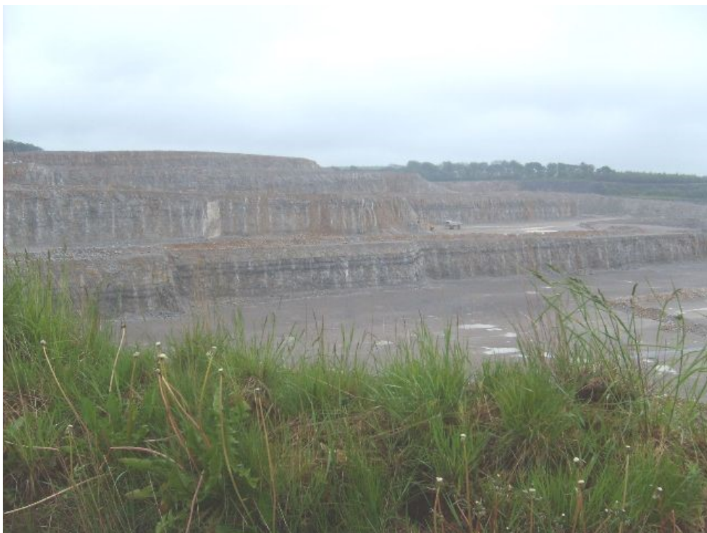
Plate 28 – View facing south of the working faces ('lifts' A-D) of Old Moor Quarry.
