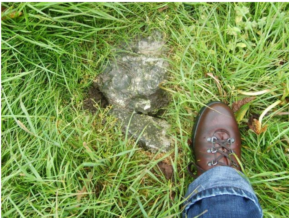
Plate 22 – View of fast limestone cobbles (possibly ginging), which may represent the filled entrance to a former lead shaft (site 79). A void was observed beneath the stones.
