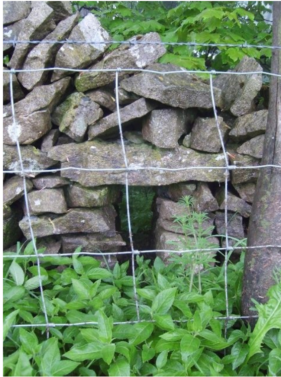
Plate 25 – View taken from the west side of enclosed sycamore copse showing a single rabbit smoot (site 66).
