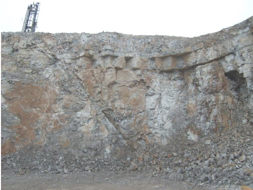
Plate 31 – View facing east of lift 'B', Old Moor Quarry. At centre is a narrow sediment choked fault.
