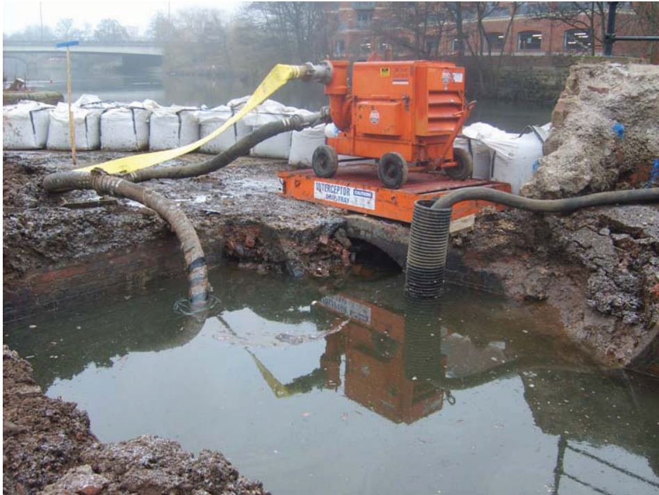
Plate 1: Deep tank associated with the early 20 th -century power station, beneath the raised southern end of the island. Note the brick arched outlet beneath the pump. View north-east.
