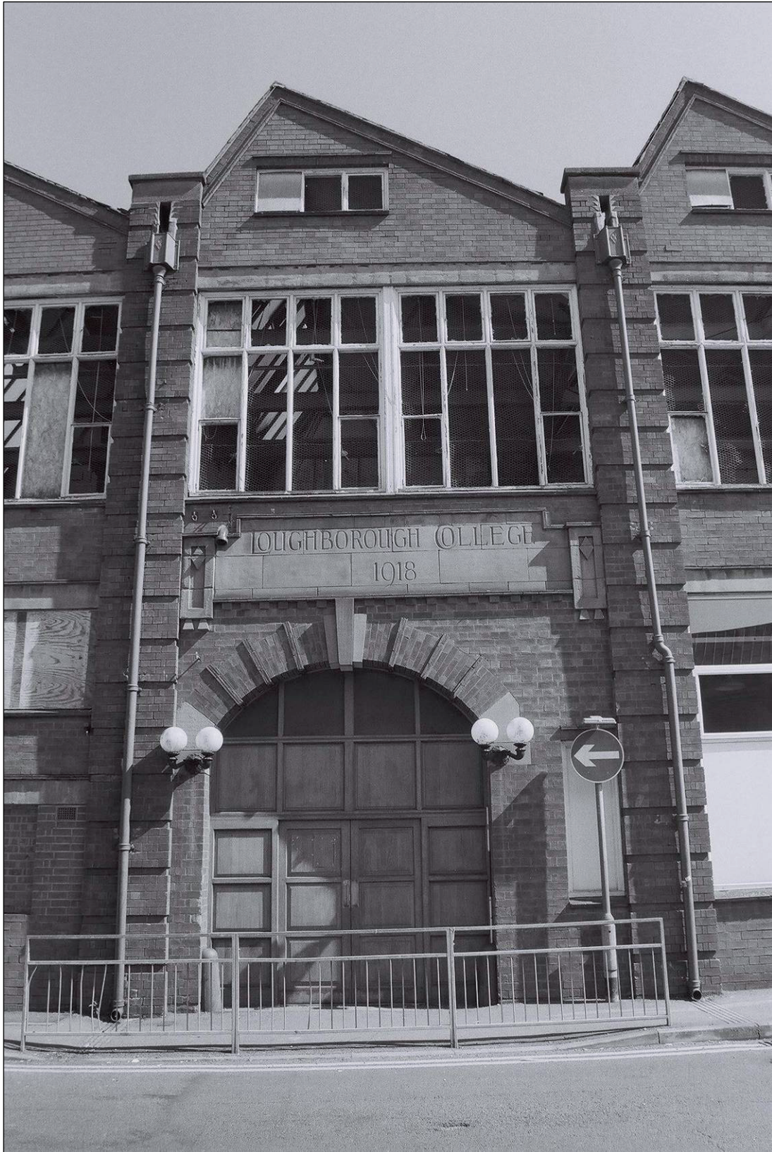
Plate 4: General view of main entrance, building 1 (film 15.14)
