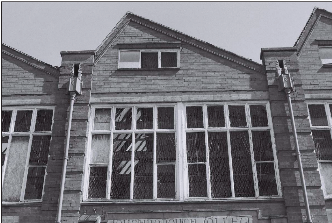
Plate 6: Detail of windows and north light roof of building 1 (film 15.10)
