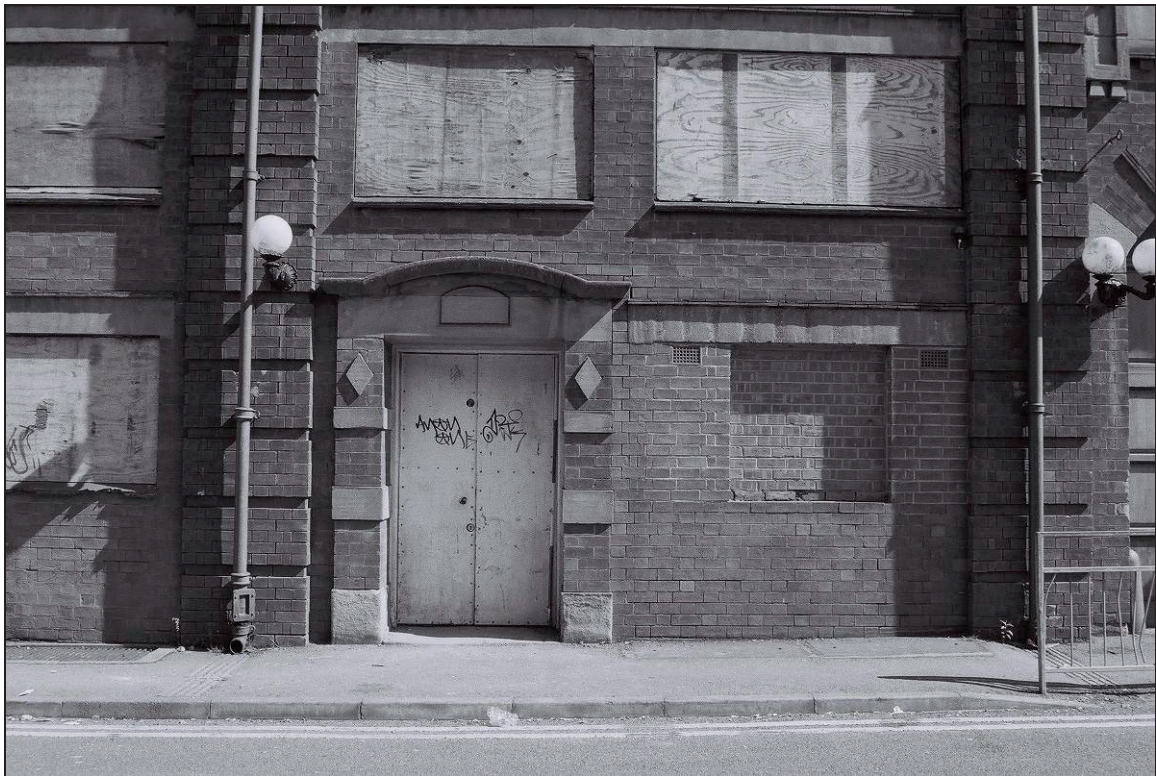
Plate 8: Detail of doorway, principal façade of building 1 (film 15.9)
