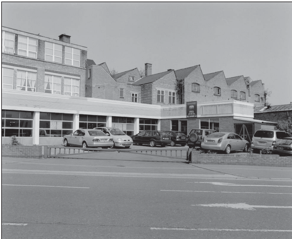
Plate 10: East elevation of building 1 (film 1.9)
