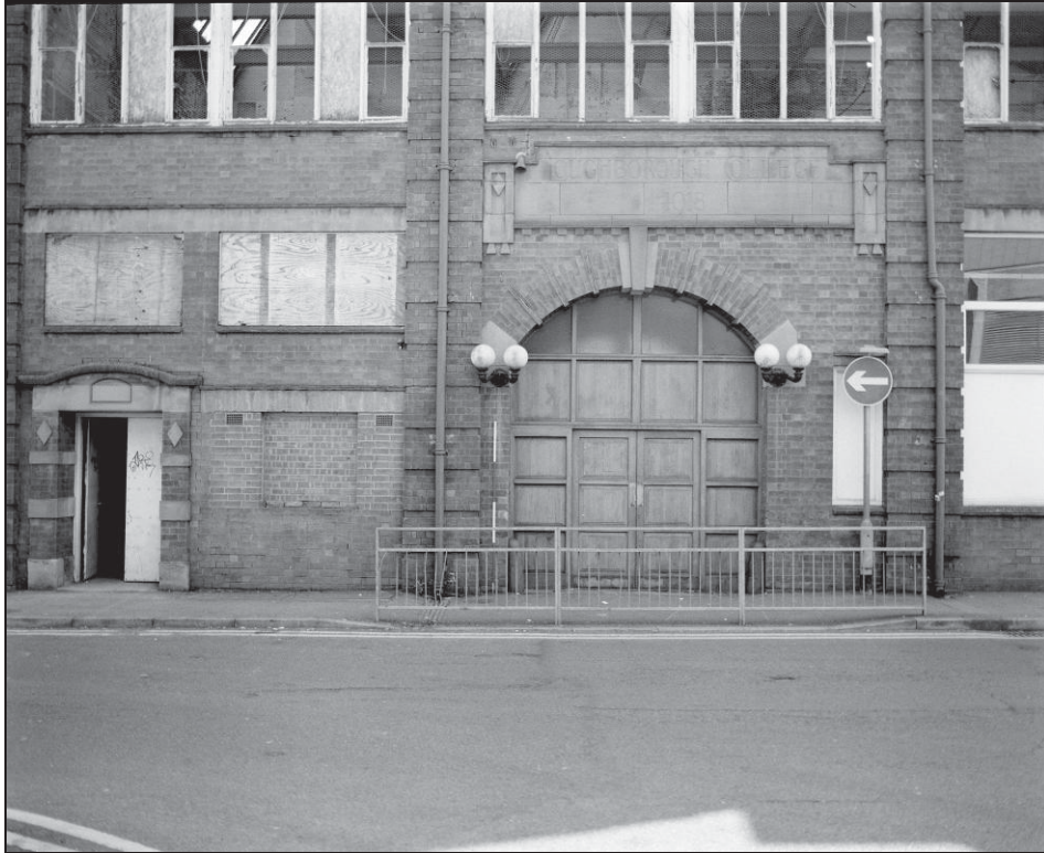
Plate 5: Doorways in west elevation of technical college (film 2.6)
