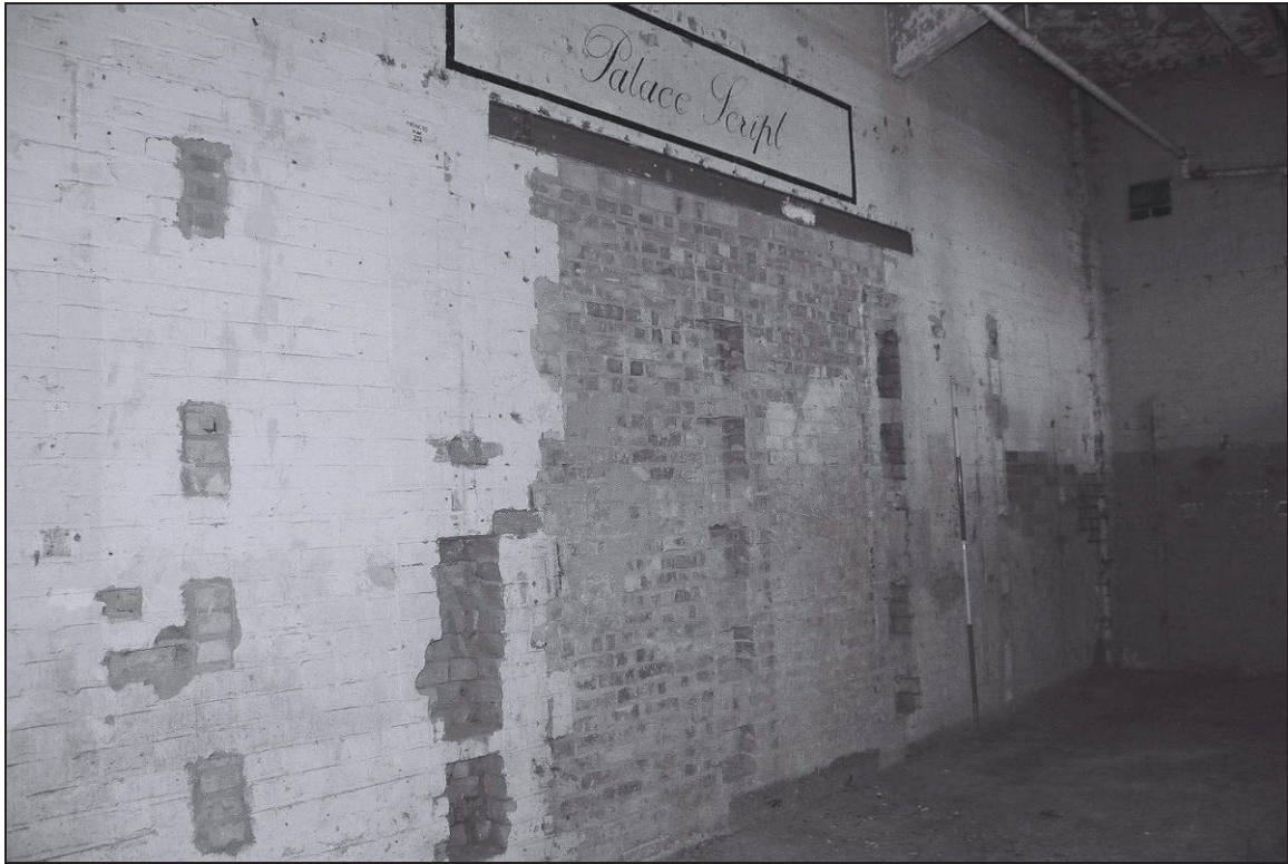
Plate 27: Detail of northwest wall of G4 showing blocked openings (film 12.18)
