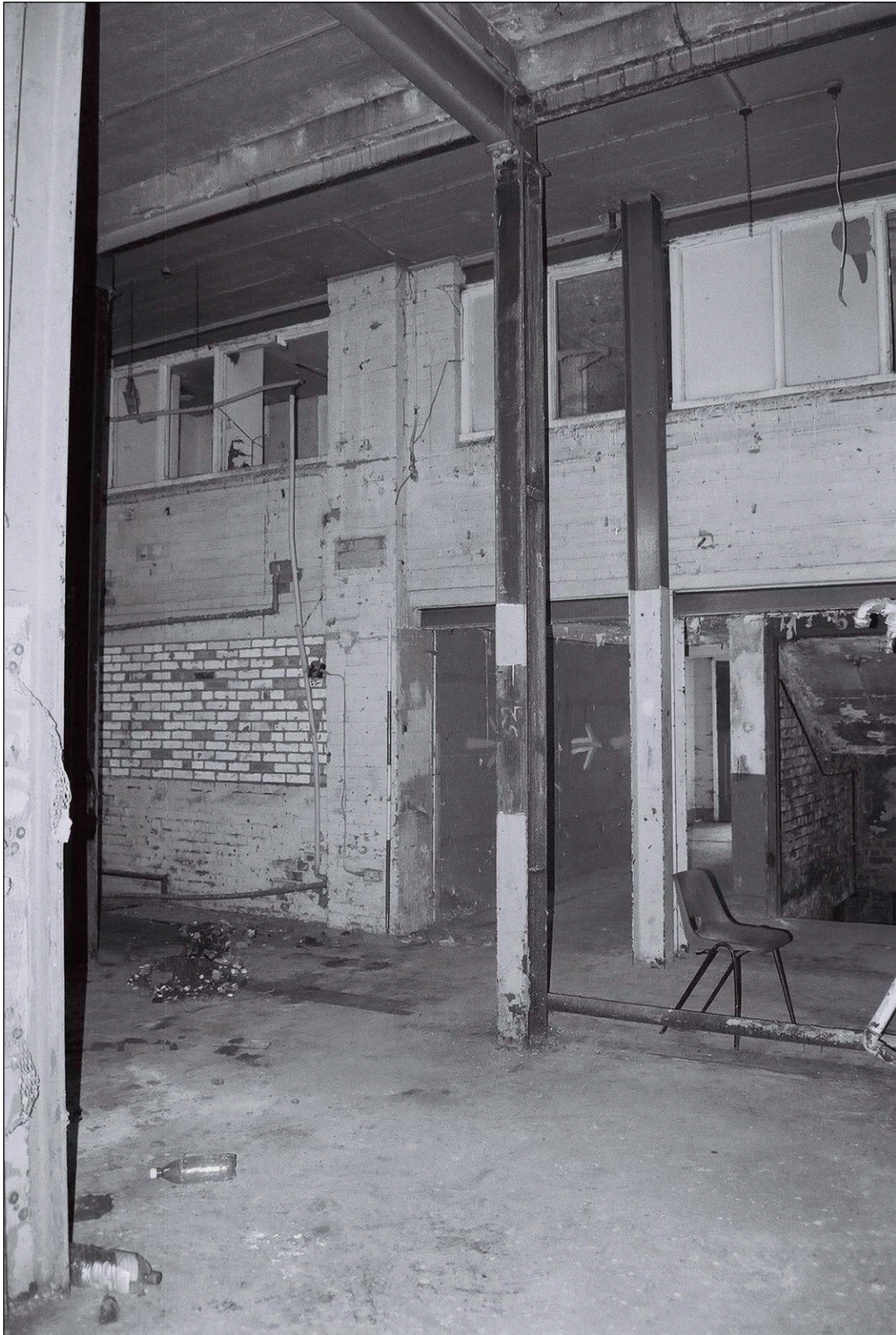
Plate 21: View of overlooking mezzanine floor from G5 (film 12.27)
