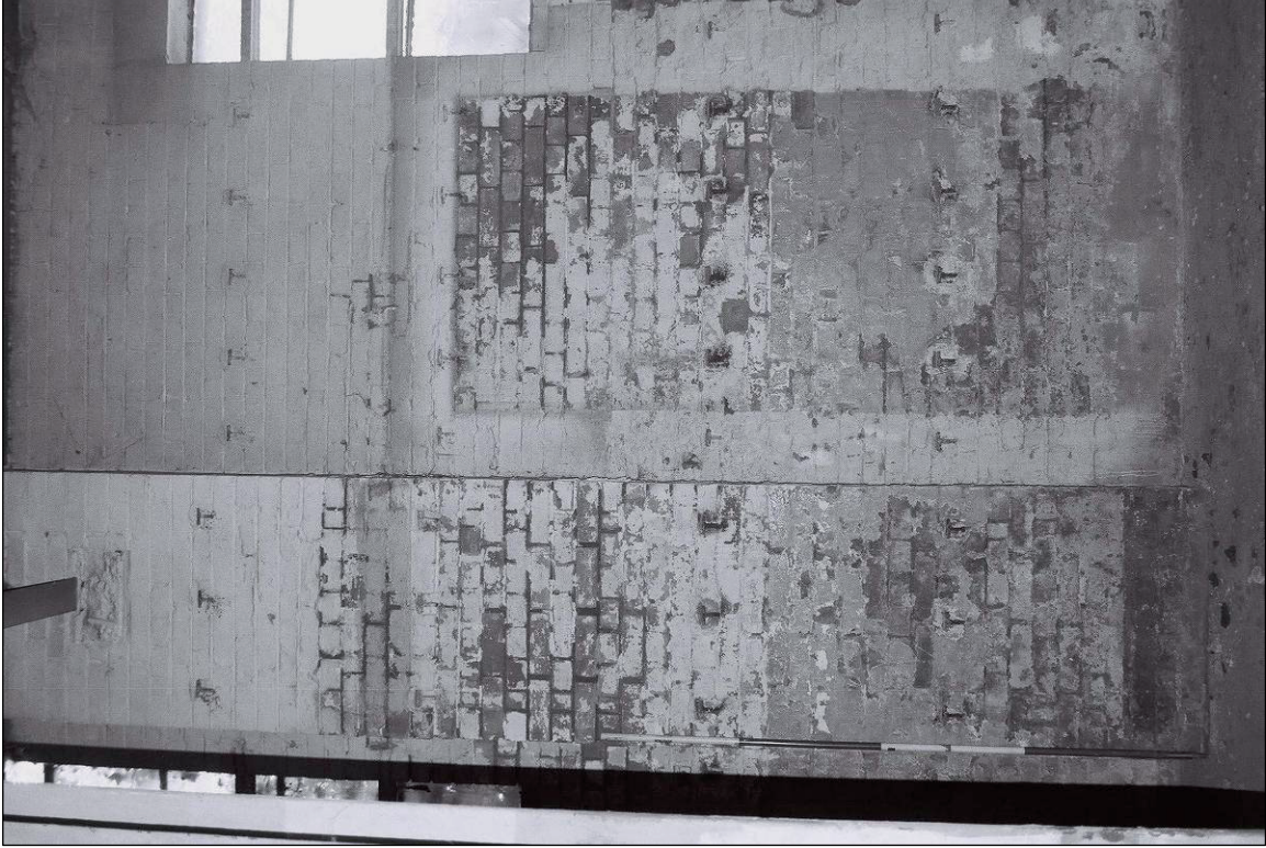
Plate 24: Detail of truncated 'T' bars (4 rows) within southeast wall of G5 (film 12.28)
