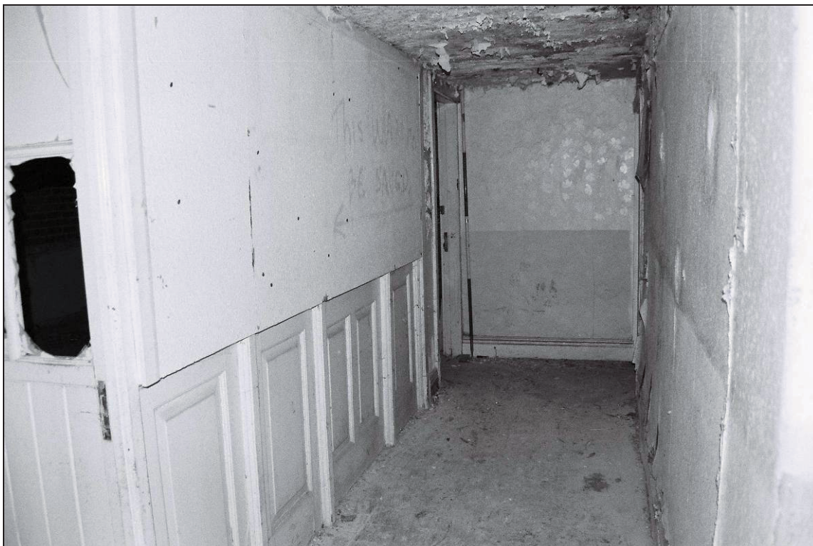
Plate 43: General view of mezzanine corridor showing paneled partition (film 13.12)
