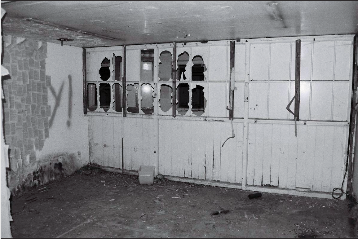
Plate 45: General view of M3 showing glazed partition (film 13.8)
