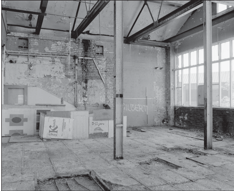
Plate 50: View across room F1 looking towards stairwell (film 8.5)
