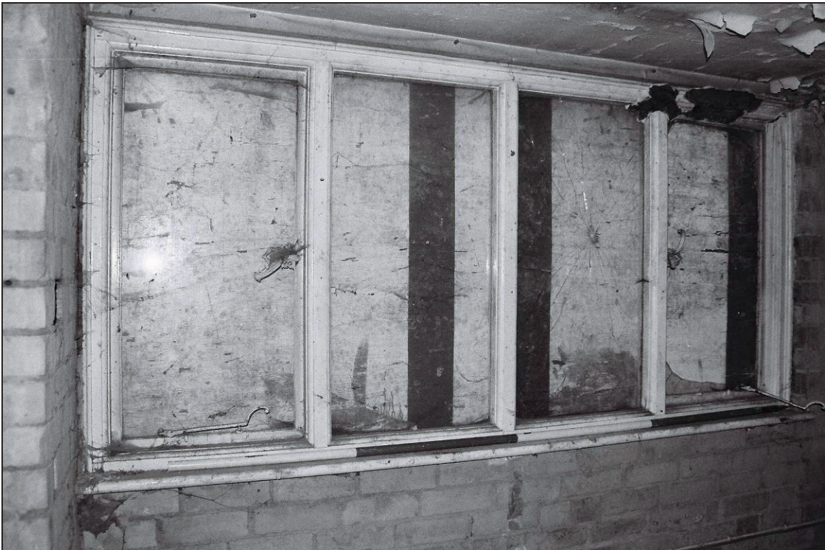
Plate 46: Detail of window, northwest wall of M3 (film 13.6)
