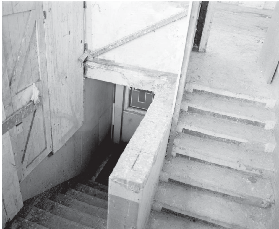
Plate 49: View down stairwell towards mezzanine floor (film 8.1)
