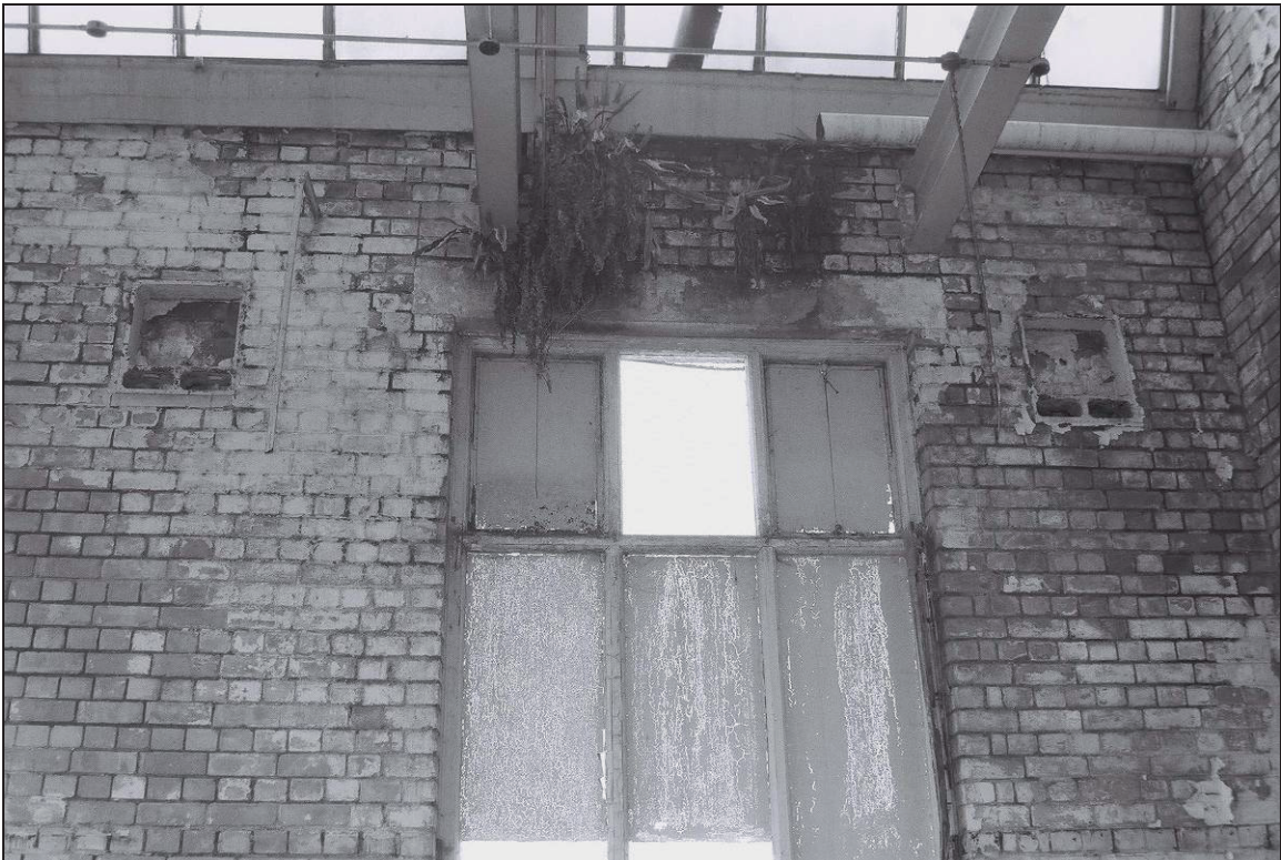
Plate 53: Detail of wall boxes in northeast wall of F1 (film 14.28)
