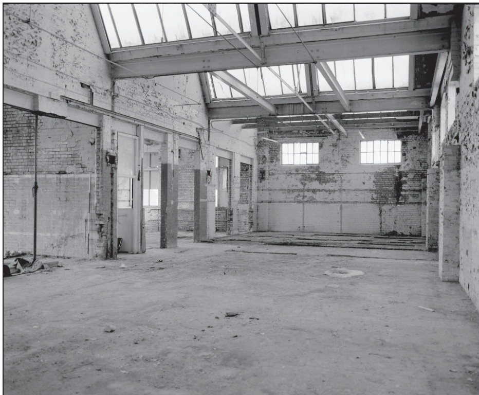
Plate 57: View across room F3 towards stairwell (film 9.4)
