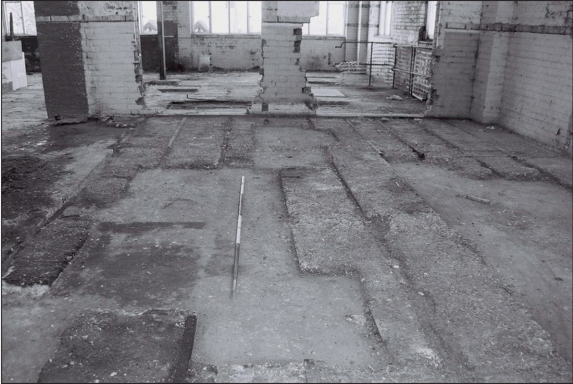
Plate 60: Detail of machine base scars in floor of F2 (film 14.19)
