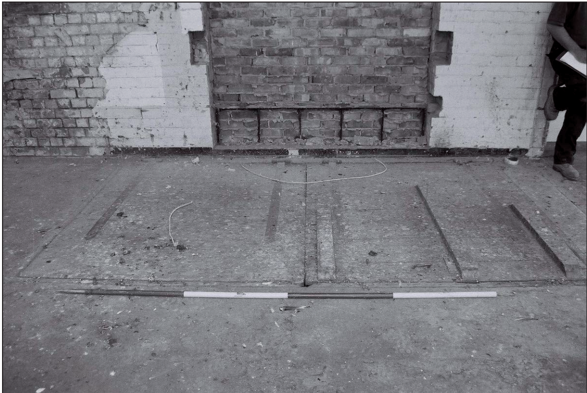
Plate 63: Detail of trap doors in floor of F3 (film 14.7)
