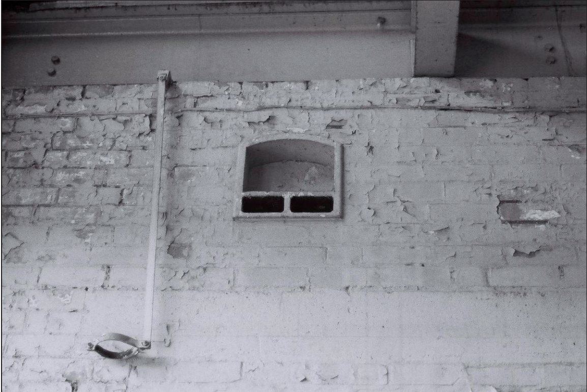
Plate 72: Detail of wall box, north east wall of F4 (film 15.26)
