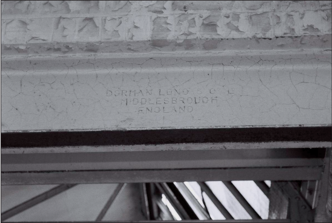
Plate 70: Detail of RSJ maker's name, above openings between F3 and F4 (film 14.1)
