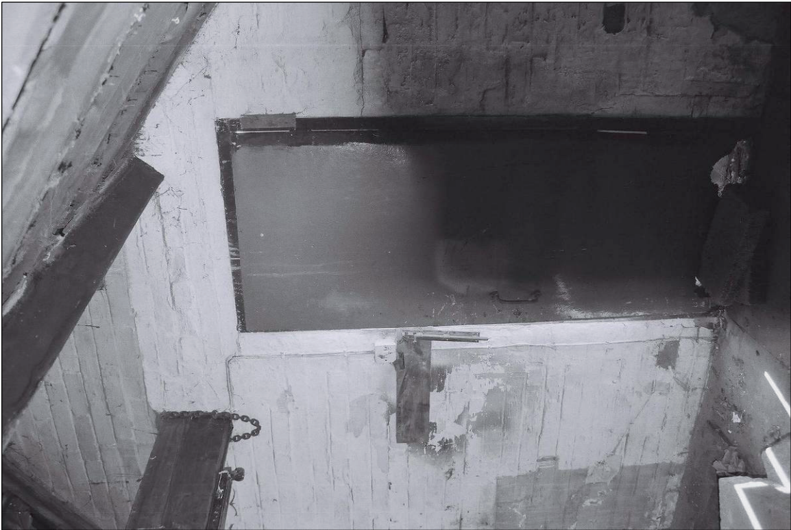
Plate 90: Partition wall and door and beam (first floor) building 2 (film 10.23)
