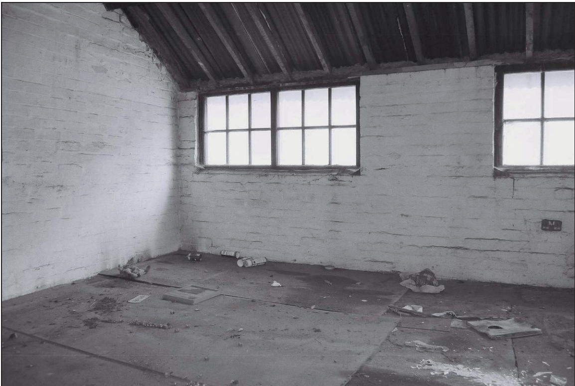
Plate 89: General view of windows on first floor – building 2 (film 10.25)
