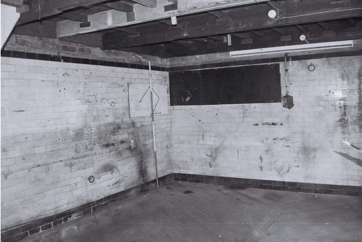
Plate 88: Blocked window in wall of building 2, note inserted glazed tiles (film 10.30)
