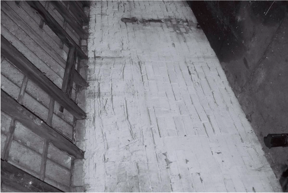
Plate 91: Blocked window/doorway (first floor) building 2 (film 10.22)
