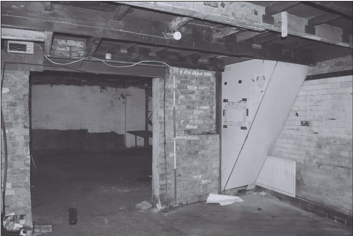
Plate 87: Small room (ground floor) building 2 (film 10.28)
