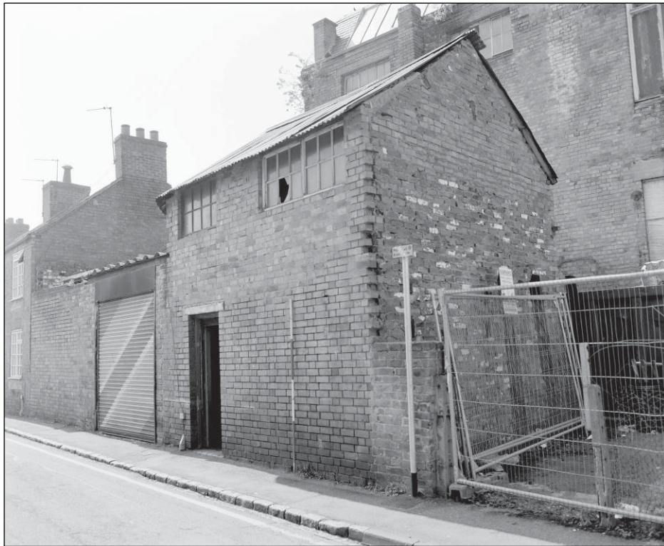
Plate 84: Orchard Street façade of building 2 (film 1.3)
