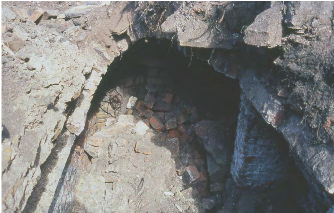
Plate 2: Vaulted cellarage close to corner of Edward Street/Brocco Street, looking east
