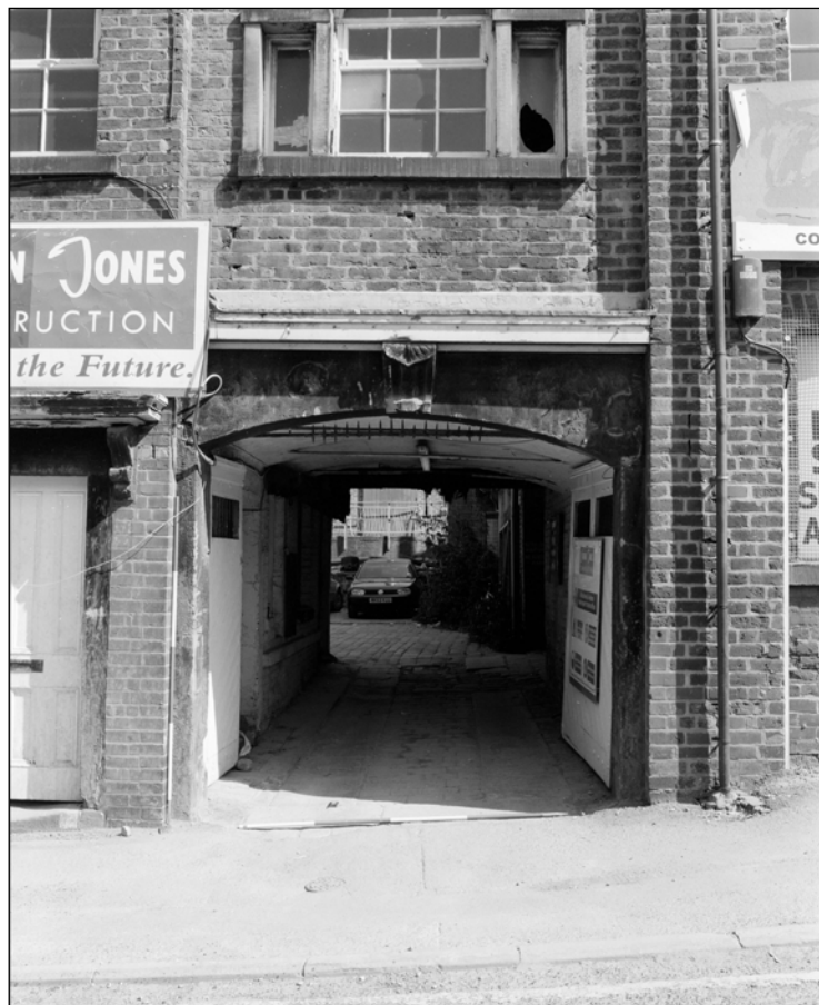
Plate 2: Building 1a: cart passage entrance (Film 10.3)
