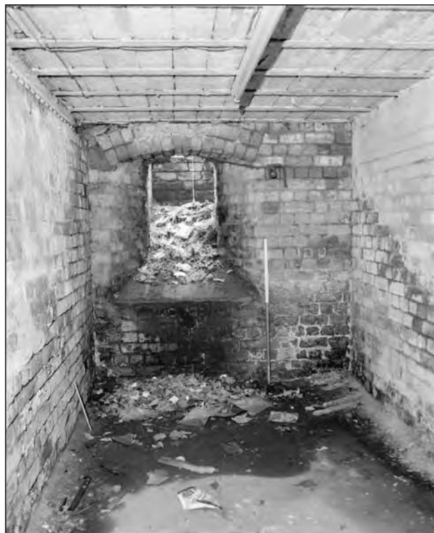
Plate 108: Building 4; sub-basement, general shot of A44a with coal chute (Film 17.1)
