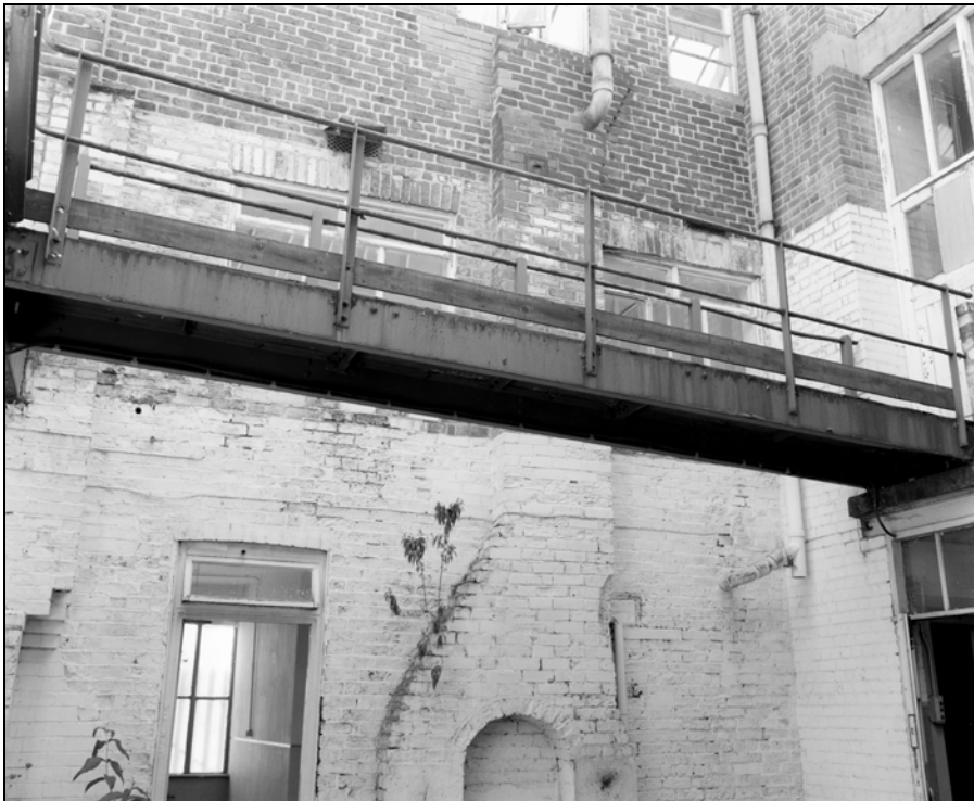
Plate 33: Building 2; west elevation, showing elevated walkway to building 5 (Film 13.8)
