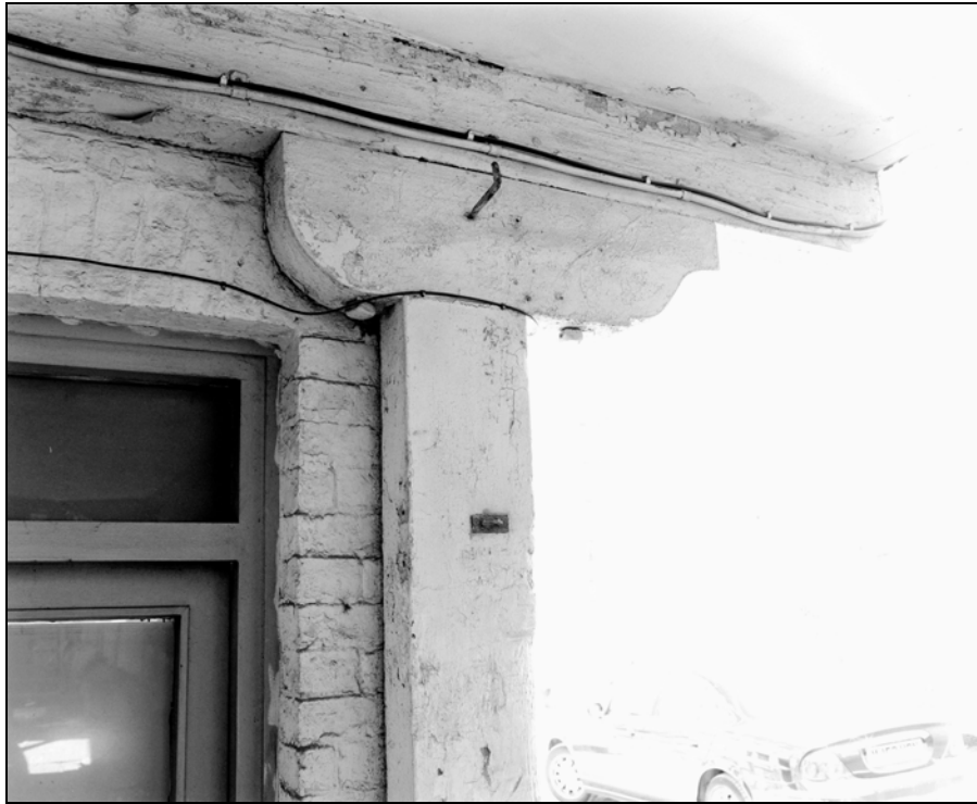
Plate 7: Building 1a, rear of cart passage; timber supporting beams (Film 18.6)
