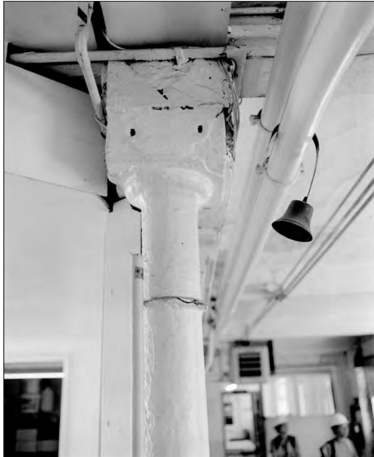
Plate 22: Building 1b ground floor; cast iron column in room A2 (Film 7.7)
