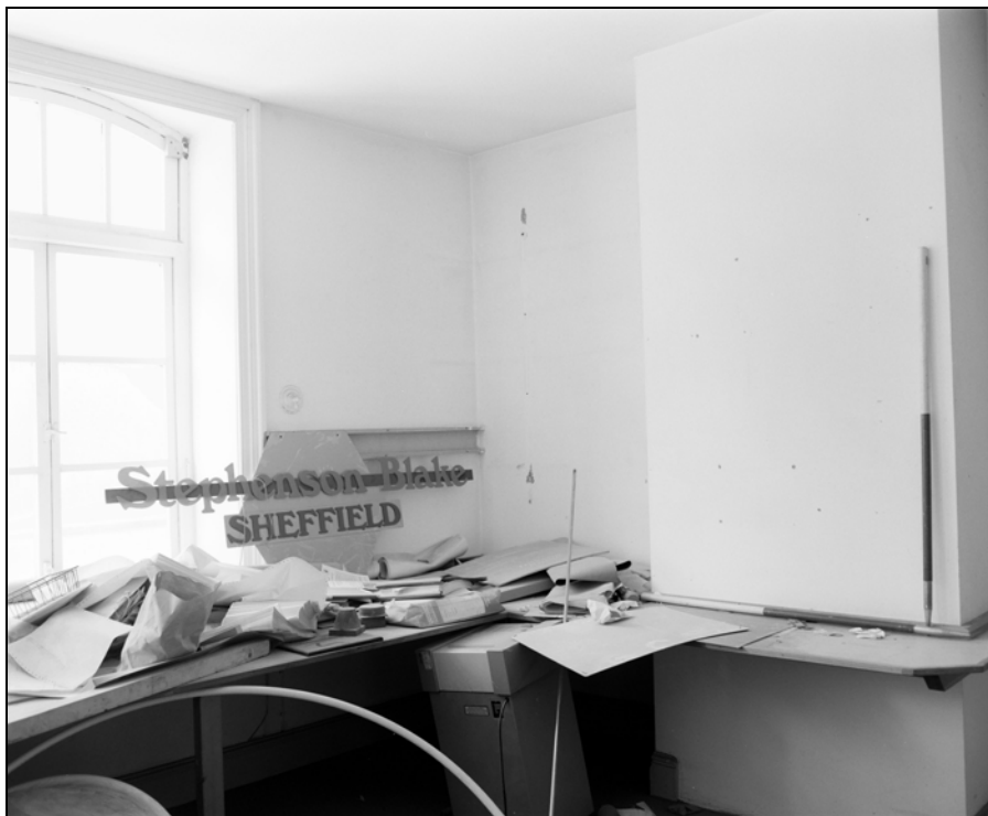
Plate 128: Building 4; ground floor, general shot of A47 with blocked fireplace (Film 7.1)
