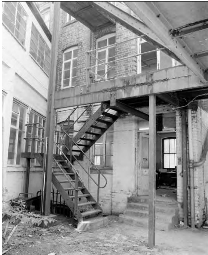
Plate 64: Building 5 (left) and building 3 (right); elevated walkway in west yard (Film 8.9)
