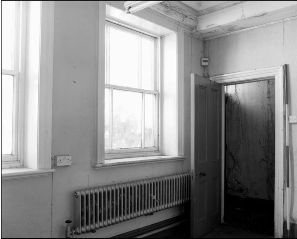
Plate 43: Building 2; ground floor, general shot of A12, showing architectural details (Film 17.7)
