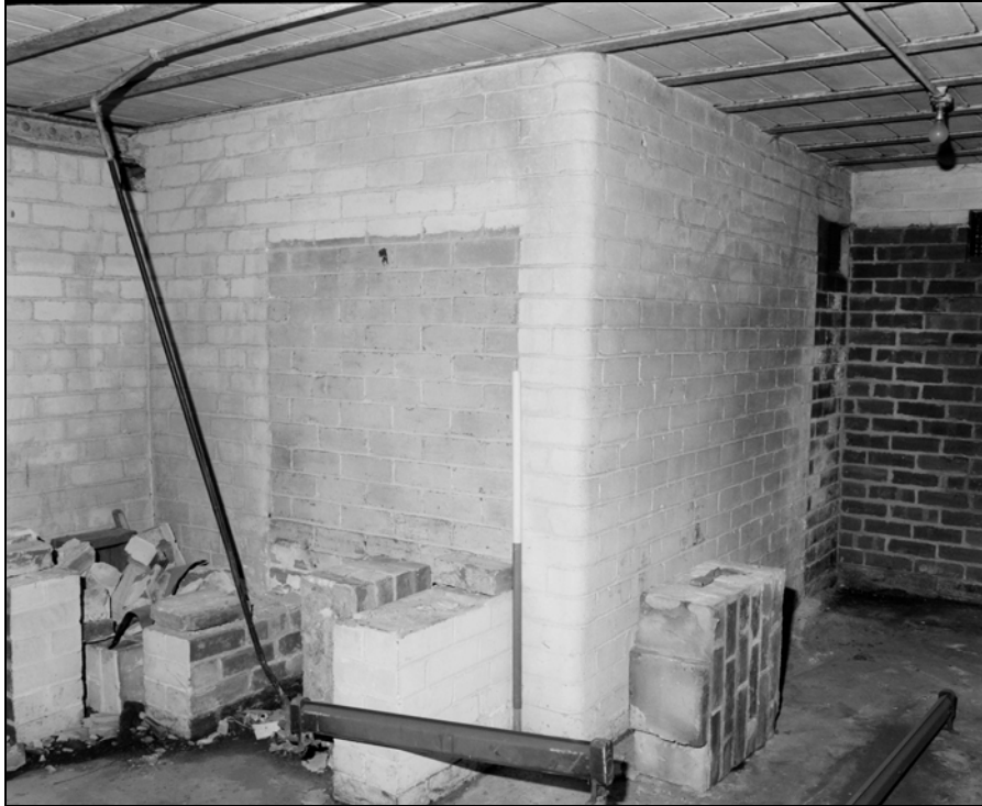
Plate 101: Building 4; sub-basement, general shot of A42a, removed shelving (Film 15.8)
