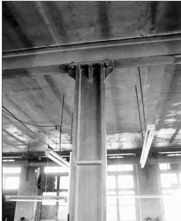
Plate 131: Building 4; first floor, detail of cast iron column in A14 (Film 3.02)
