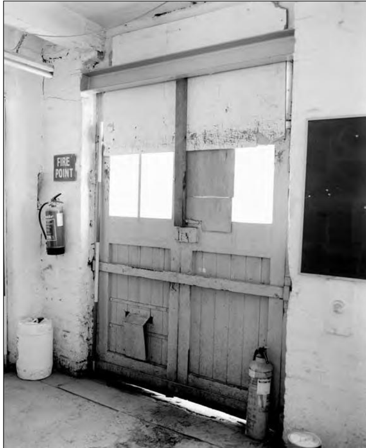
Plate 21: Building 1b ground floor; taking-in door, room A2 (Film 7.9)
