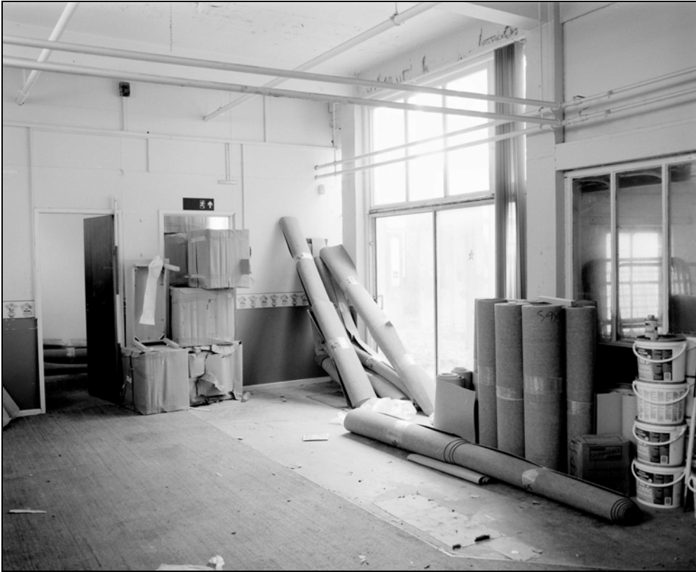
Plate 140: Building 5 ground floor, room A9; general view to west (Film 12.1)
