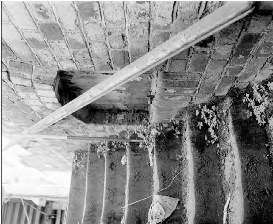
Plate 94: Building 4; rear basement passage, worn steps to sub-basement (Film 16.09)
