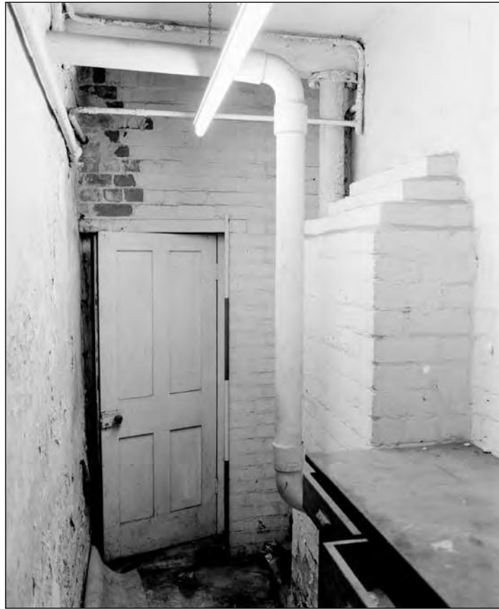
Plate 41: Building 2; ground floor, flue in passage behind A12 (Film 11.7)
