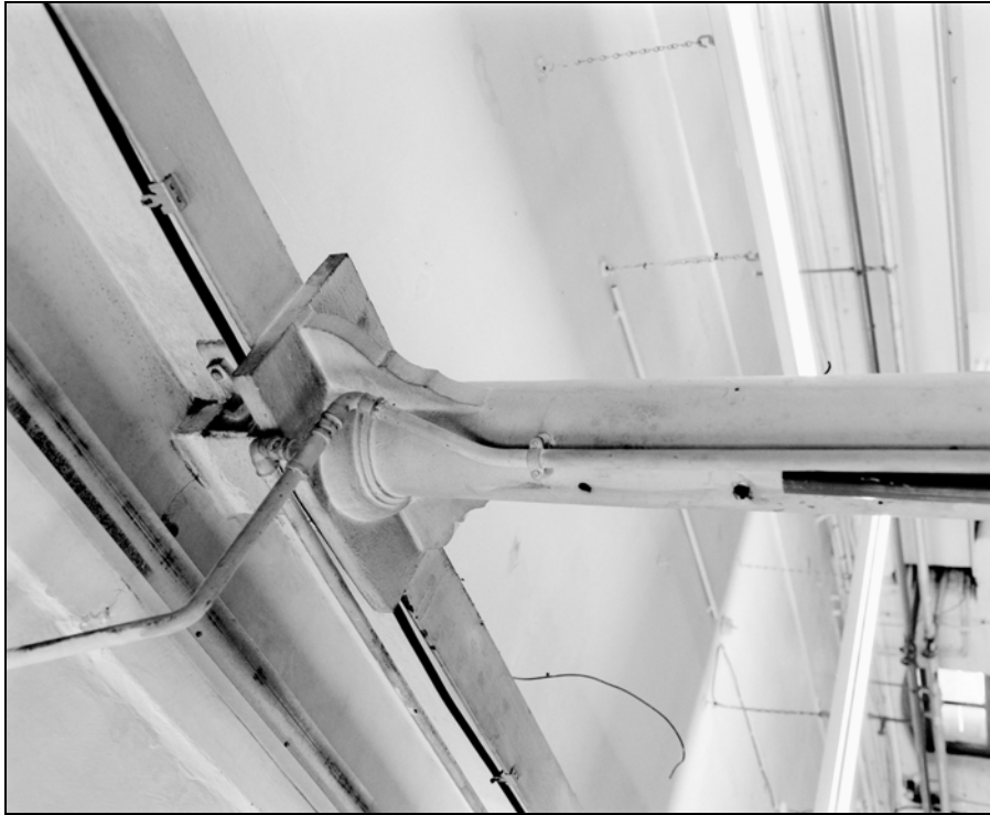
Plate 77: Building 3; ground floor, column detail in A7 (Film 8.5)
