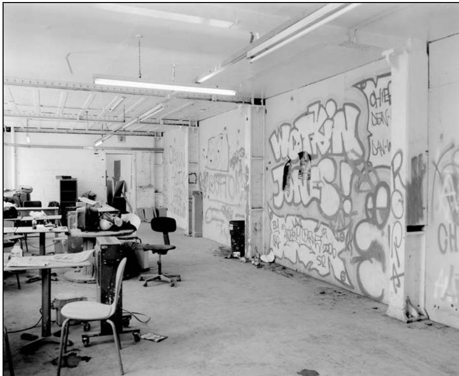
Plate 124: Building 4; ground floor, A3 looking north-east, cast iron columns (Film 7.4)
