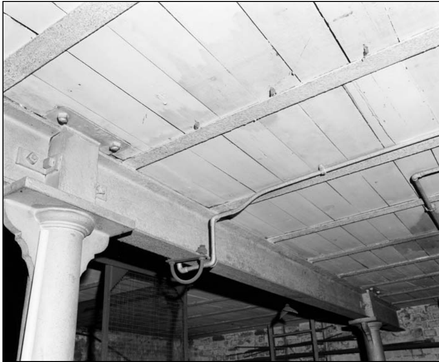
Plate 65: Building 3; basement, ceiling detail in A52 (Film 12.4)
