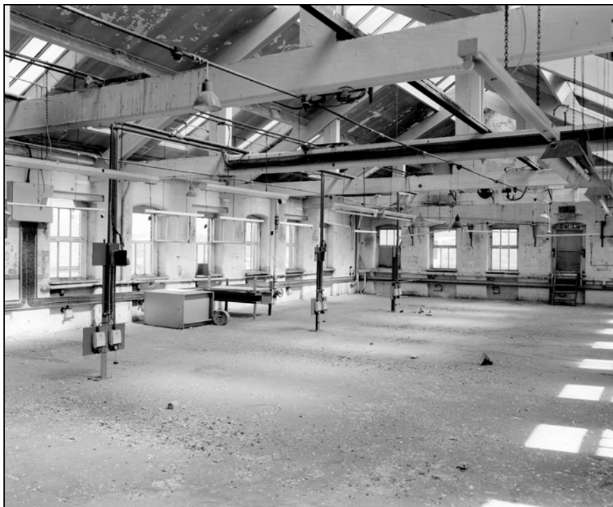
Plate 133: Building 4; second floor; general shot of A34 looking north (Film 1.1)
