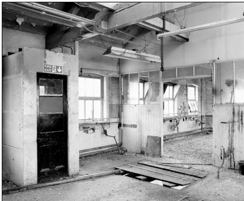
Plate 83: Building 3; second floor, general shot of A30; A29 beyond partition (Film 6.1)
