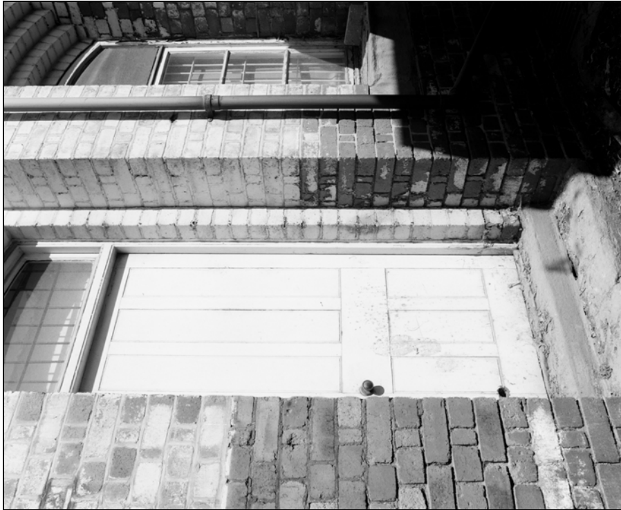
Plate 92: Building 4: rear basement passage, door to eastern room A45 (Film 14.7)
