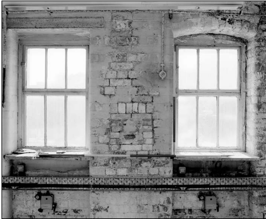
Plate 136: Building 4; second floor, detail of window & blocking in pier, A34 (Film 1.4)
