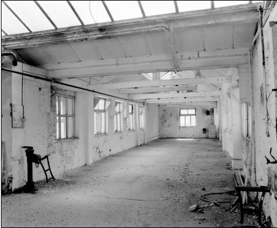
Plate 59: Building 2 second floor; room A32b viewed from room A32a (Film 1.10)
