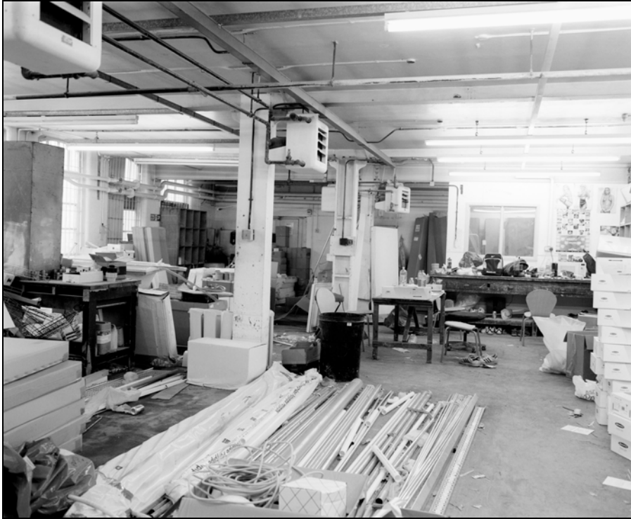
Plate 119: Building 4; basement, general shot of A38 looking south (Film 6.7)
