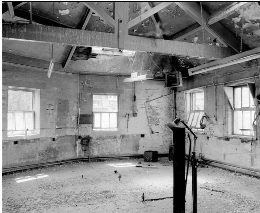
Plate 85: Building 3; second floor, general shot of A29 (Film 6.4)
