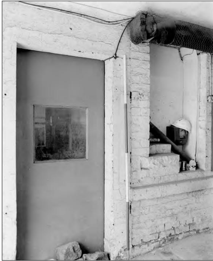
Plate 12: Building 1a, rear of cart passage; door & blocked window on east side (Film 10.7)
