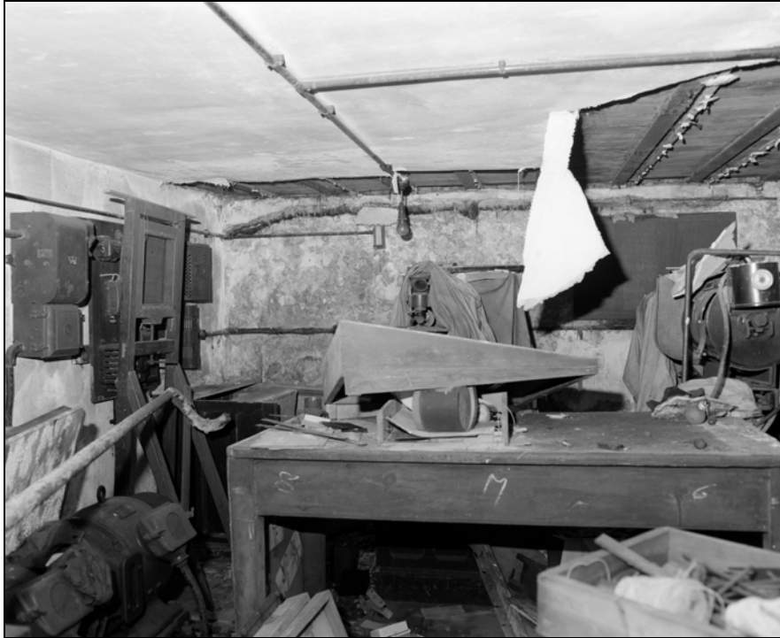
Plate 107: Building 4; sub-basement, room A43a looking north-east (Film 16.7)
