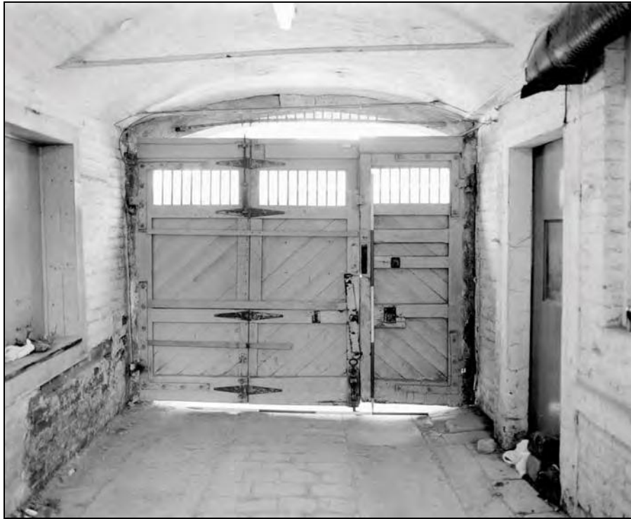
Plate 10: Building 1 cart passage, doors, jack-arch ceiling (Film 18.5)
