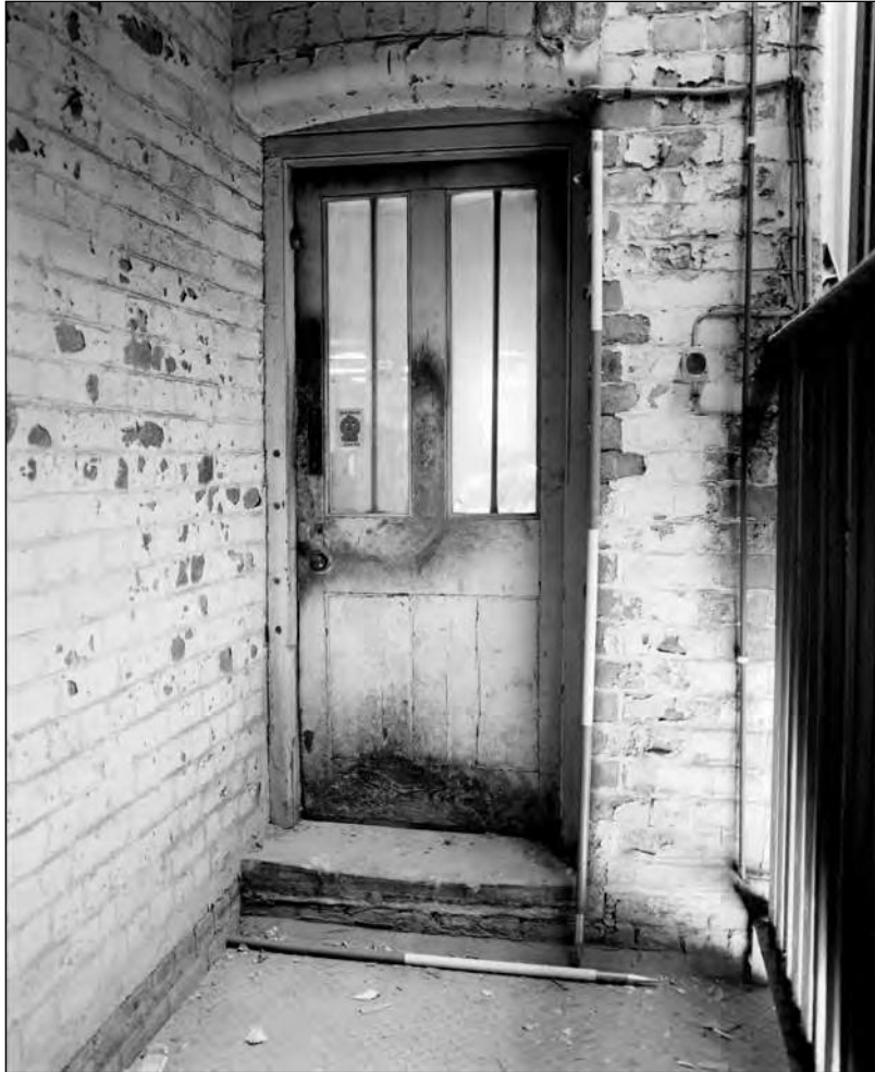
Plate 129: Building 4; first floor, entry from stairwell (Film 2.10)
