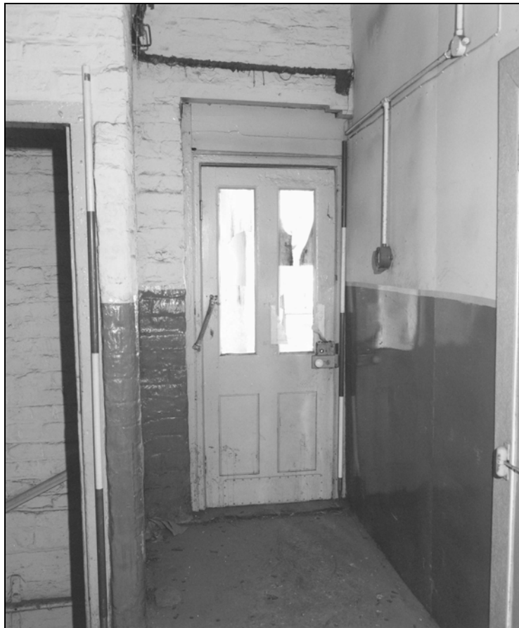
Plate 52: Building 2; first floor, stair-head and east door in A19 (Film 5.10)
