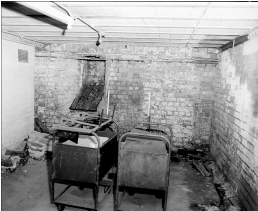
Plate 102: Building 4; sub-basement, general shot of A42b with coal chute (Film 15.5)
