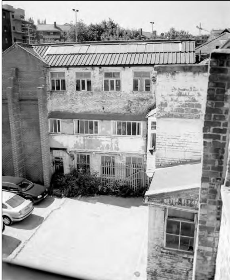
Plate 29: Shot of building 2 from roof of stair tower (Film 2.6)
