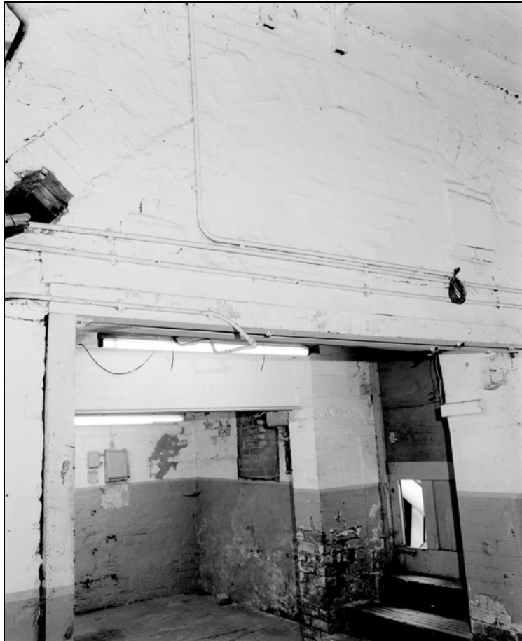
Plate 45: Building 2; ground floor, blocked arch over entrance to A13 (Film 11.3)
