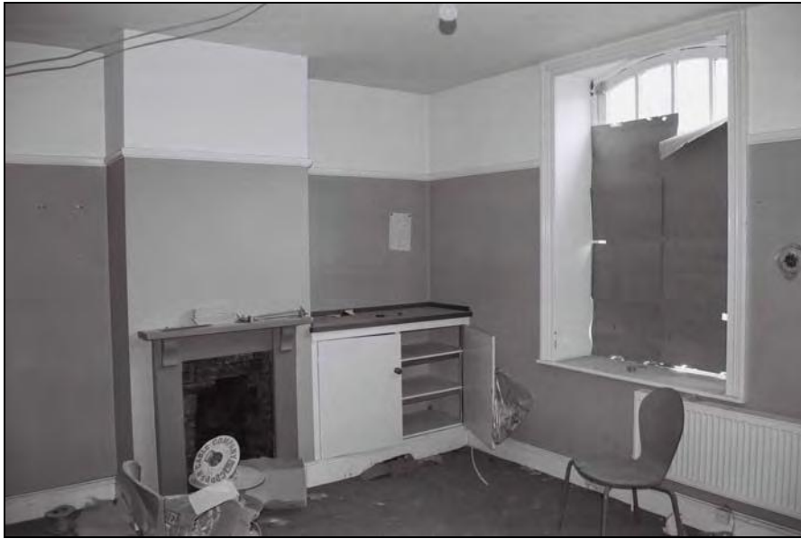
Plate 127: Building 4; ground floor, room 46 looking north-east (Film 19.26)
