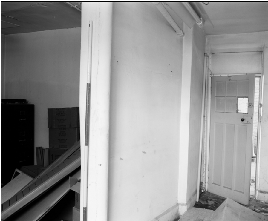
Plate 37: Building 2; ground floor, A5, cast iron column and yard door (Film 8.2)
