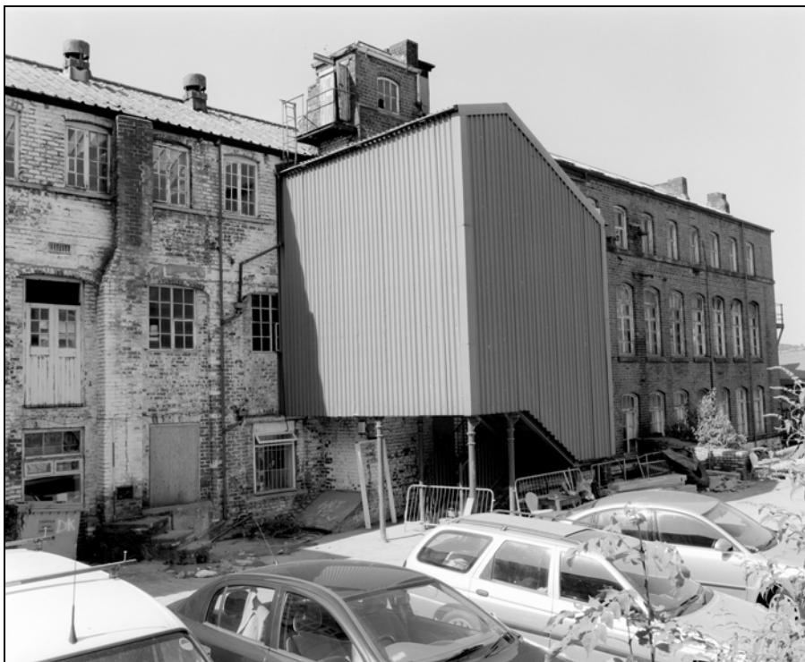
Plate 6: Rear of buildings 1b, 4 and enclosed stairwell (Film 9.5)
