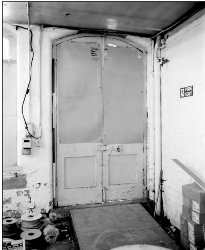
Plate 120: Building 4; basement, A38, detail of street doors (Film 6.8)
