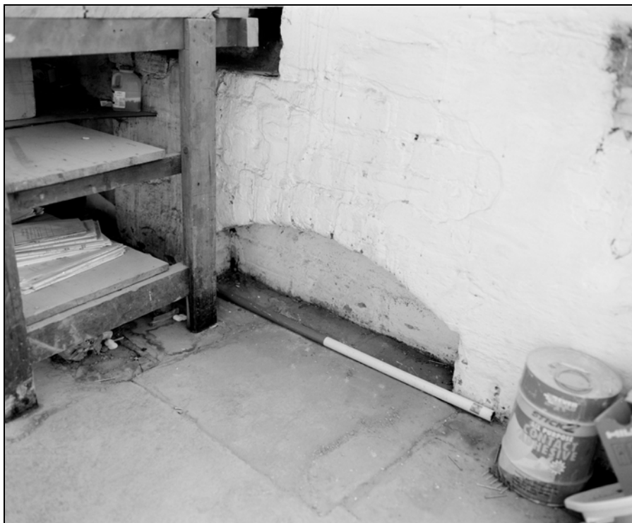
Plate 23: Building 1b ground floor; recess in A2 north-west wall (Film 7.8)
