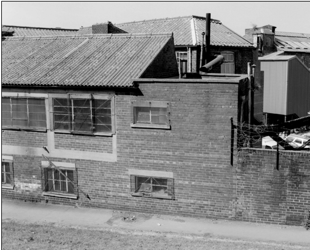
Plate 138: Building 5; view of Kenyon Alley facade (Film 9.9)
