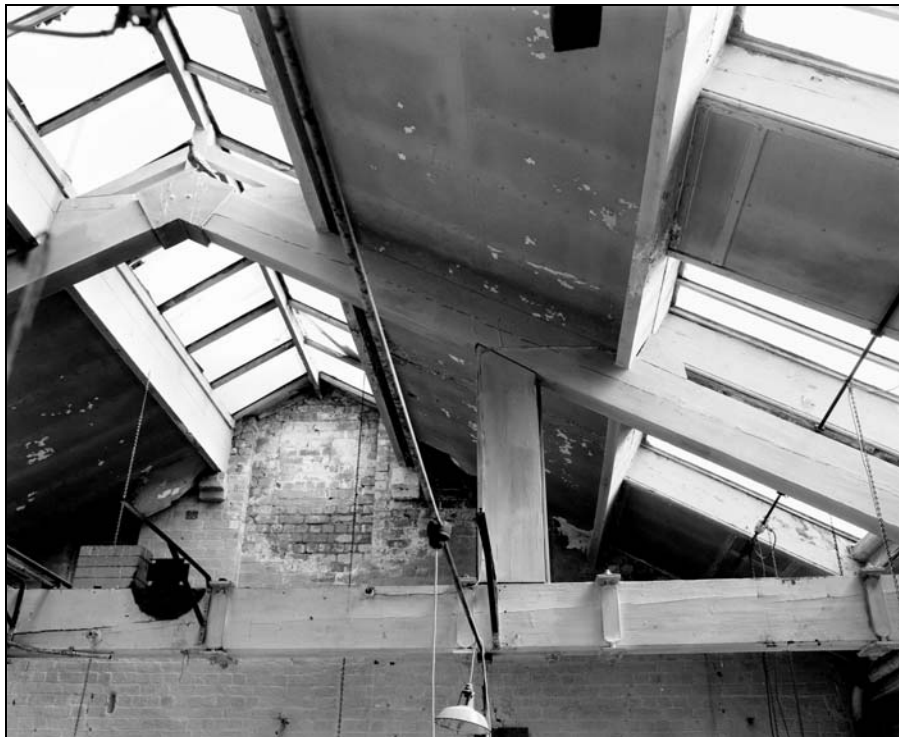
Plate 135: Building 4; second floor, detail of truss in A34 (Film 1.3)
