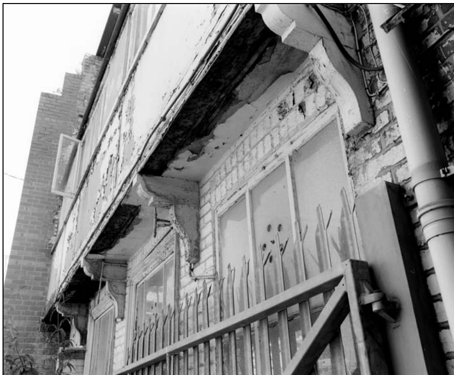
Plate 31: Building 2, east elevation, jettied first floor (Film 9.4)
