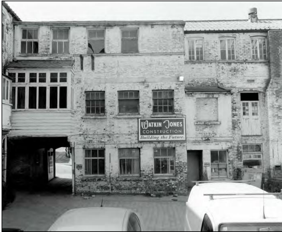
Plate 5: Buildings 1a,1b rear elevations, jettied room A18 (Film 9.6)
