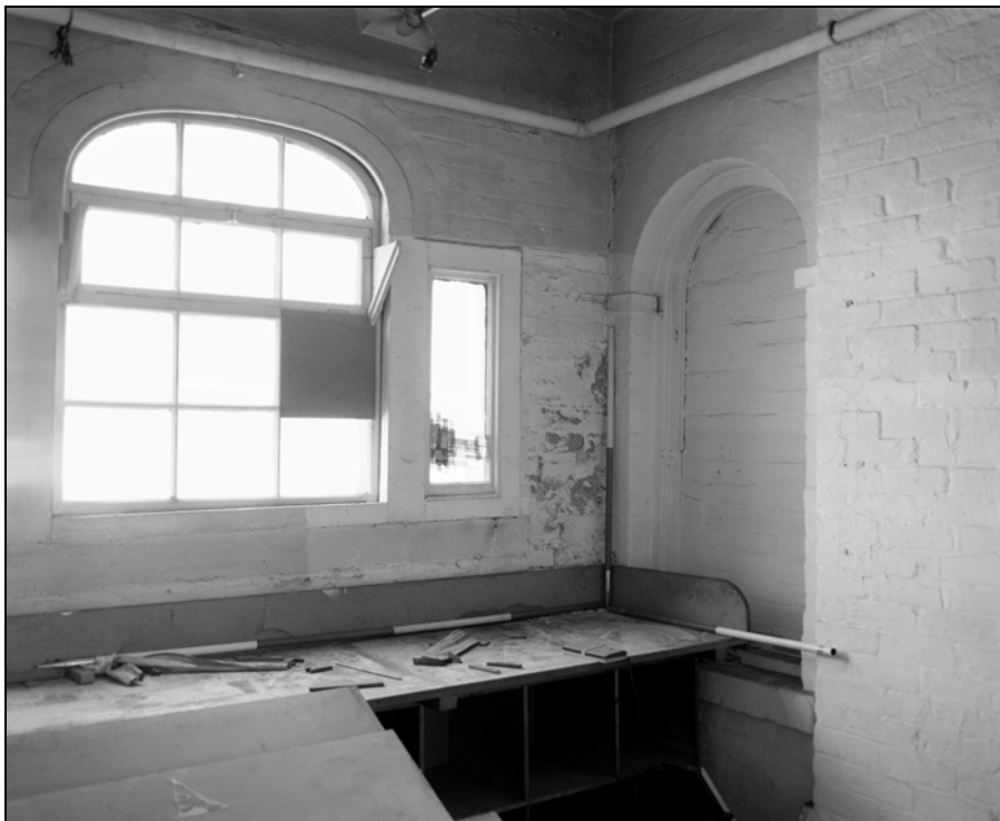
Plate 18: Building 1a, first floor, A18a; Venetian and blocked arched Windows (Film 4.2)
