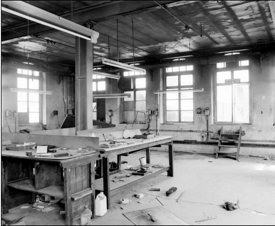
Plate 130: Building 4; first floor, north-east end of room A14 (Film 3.01)
