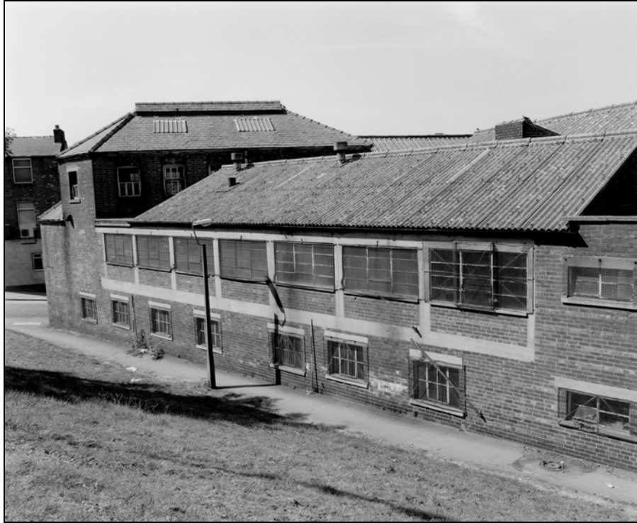
Plate 63: Building 3 and building 5; Kenyon Alley elevations (Film 9.10)
