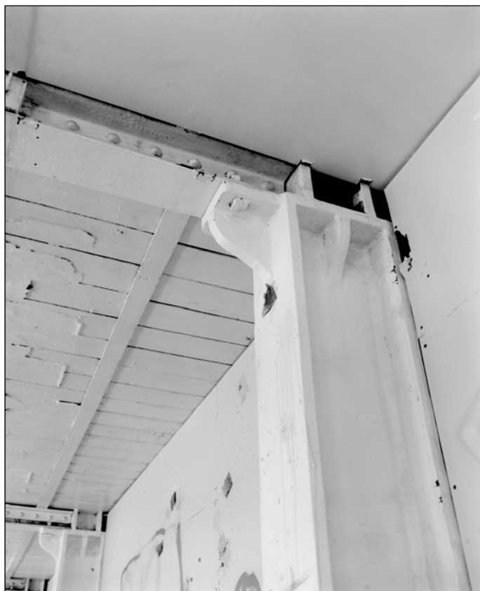
Plate 125: Building 4; ground floor, detail of cast iron column, A3 (Film 7.3)
