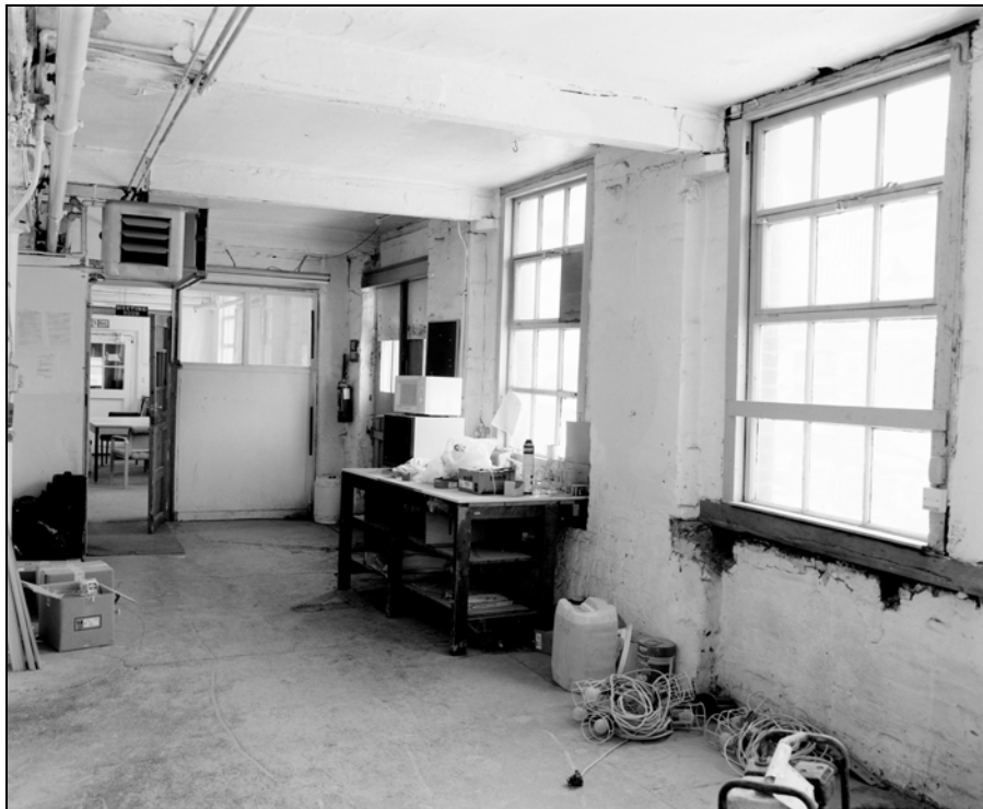
Plate 20: Building 1b ground floor; room A2, looking north-west towards A1 (Film 7.6)
