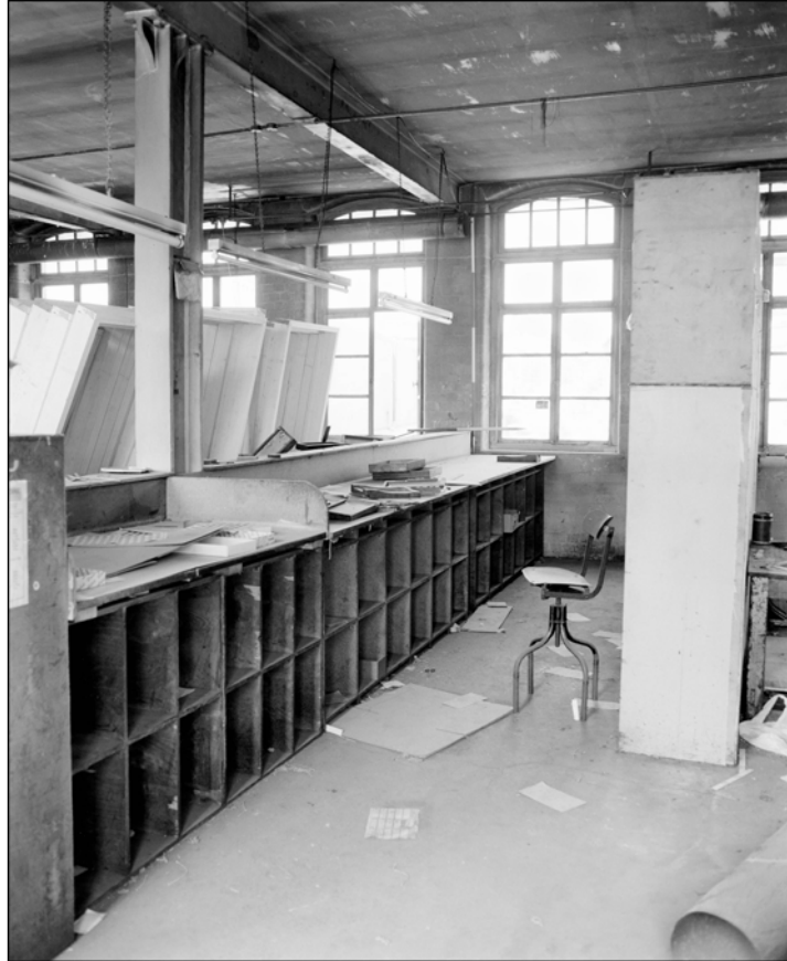
Plate 132: Building 4; first floor, west side of room A14 (Film 3.03)
