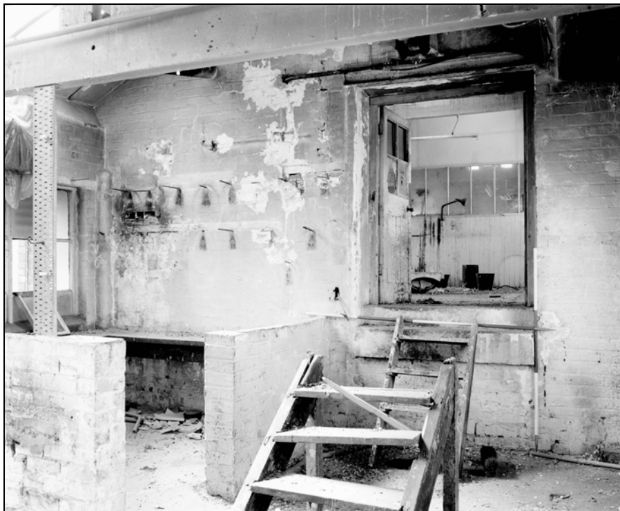
Plate 58: Building 2 second floor; A32a corner pen and steps to A30 (Film 2.5)
