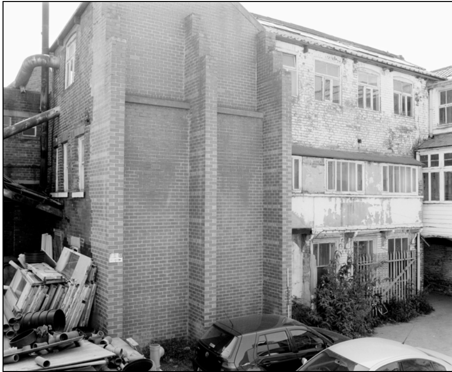
Plate 30: Building 2; general external shot of east elevation and inserted gable (Film 9.7)
