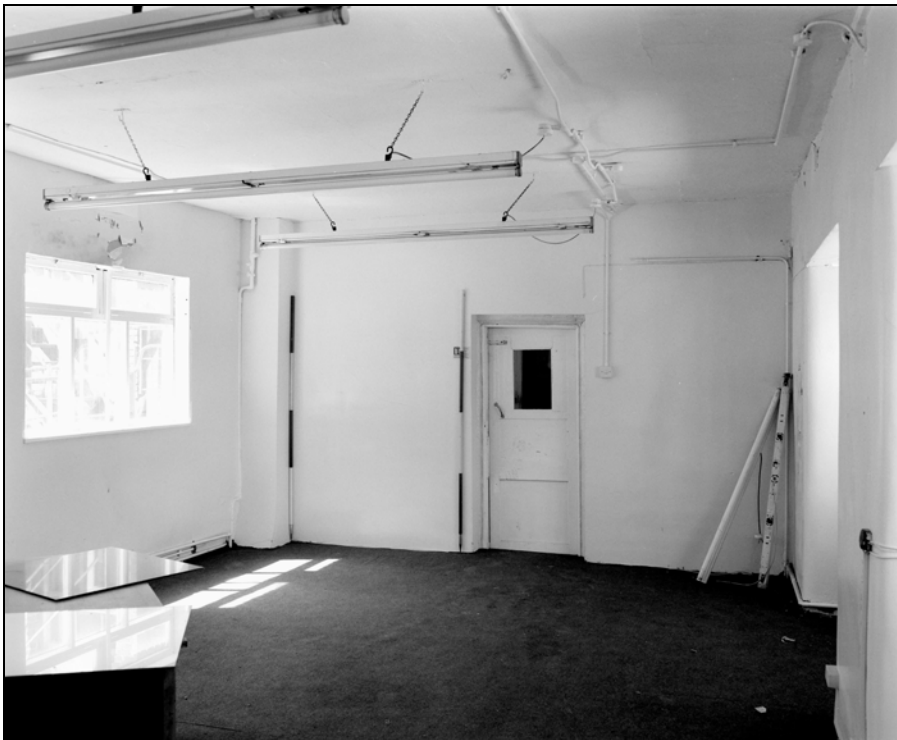
Plate 54: Building 2; first floor, general shot of A28 (Film 5.9)
