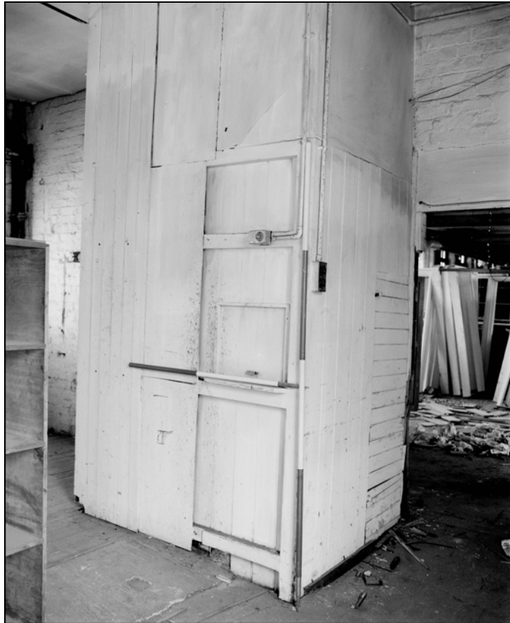
Plate 26: Building 1b, first floor; lift shaft in A15 (Film 3.4)
