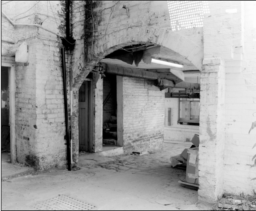
Plate 32: Building 2, west elevation, arch to cart passage (Film 8.8)
