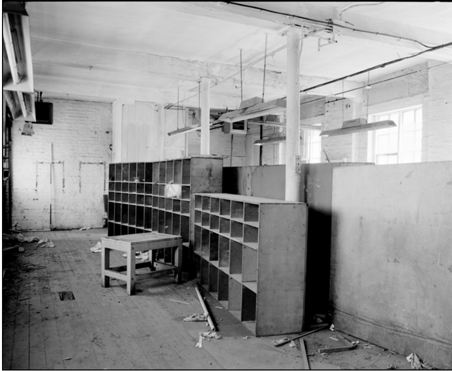
Plate 24: Building 1b, first floor; room A15 looking north-east (Film 3.6)
