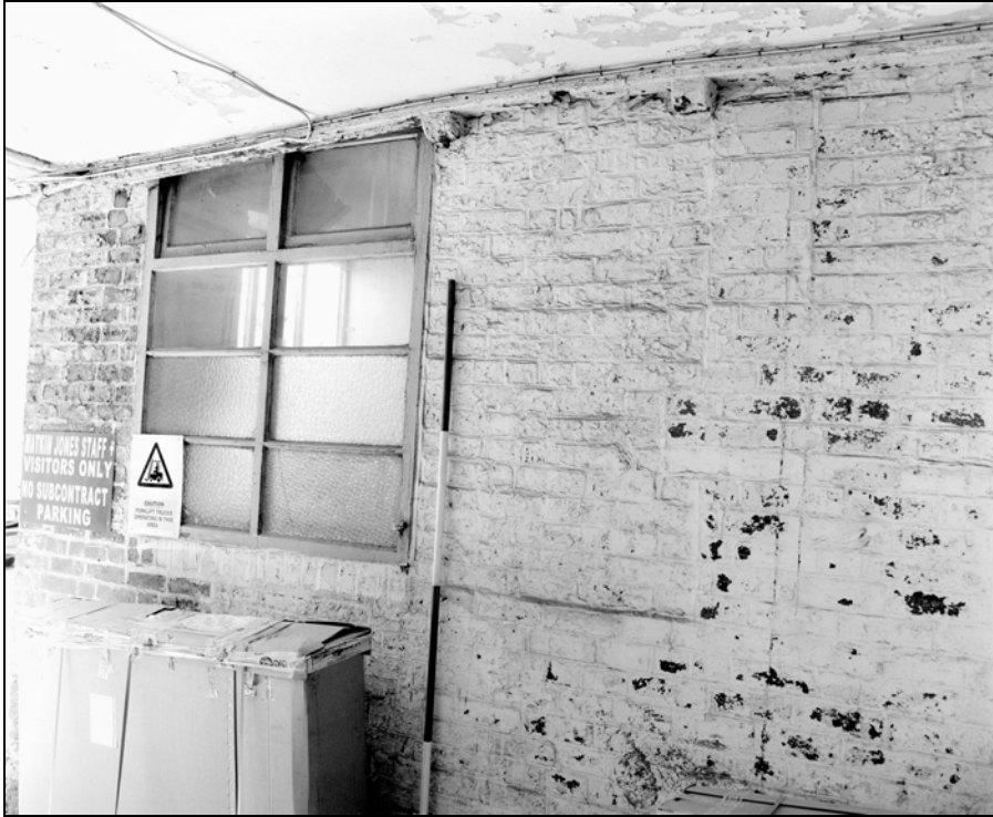
Plate 36: Building 2, cart passage, south elevation, detail of window and blockings (Film 13.10)
