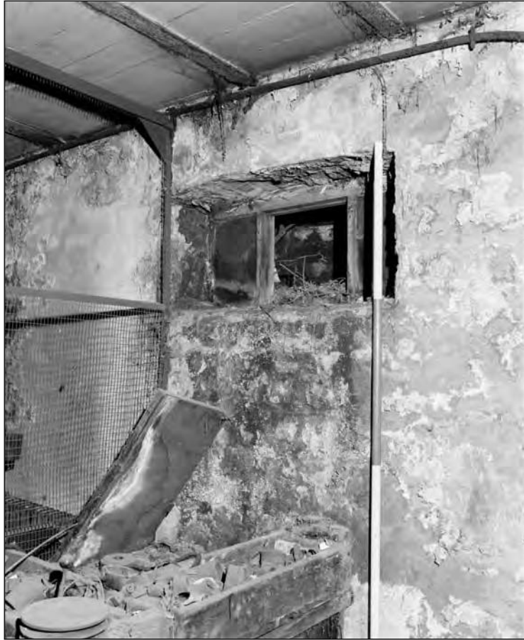
Plate 67: Building 3; basement window in A52 (Film 12.6)
