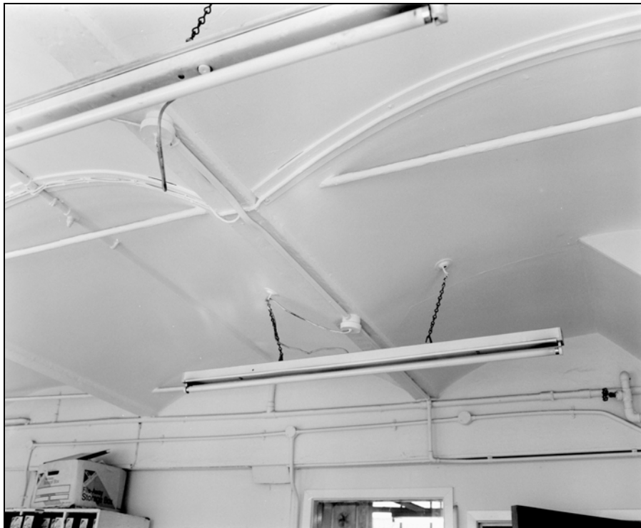
Plate 14: Building 1a ground floor; jack-arches in room A48 (Film 11.2)
