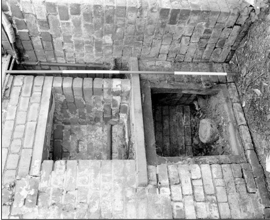
Plate 93: Building 4: rear basement passage; recess with grating (Film 14.4)
