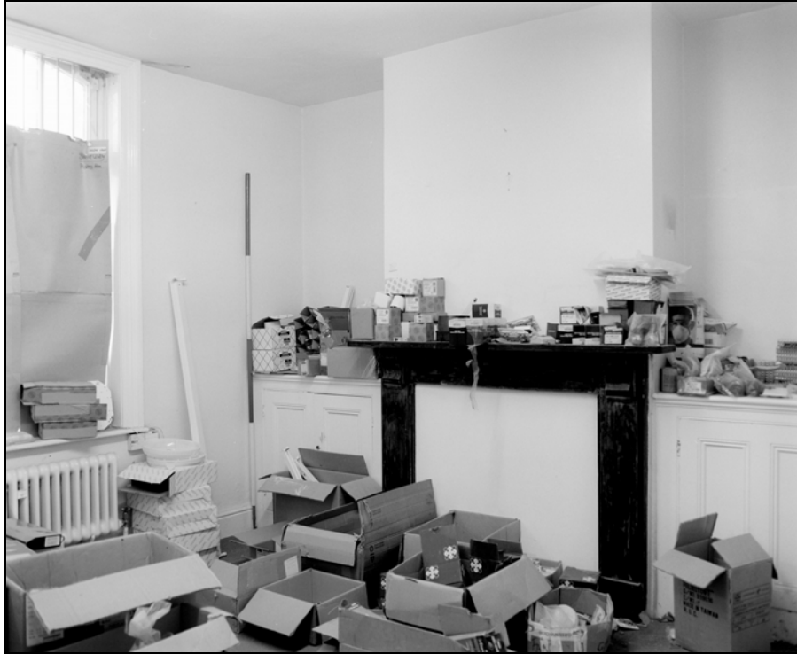
Plate 121: Building 4; basement, general view of A40, showing original fireplace and cupboard (Film 16.10)
