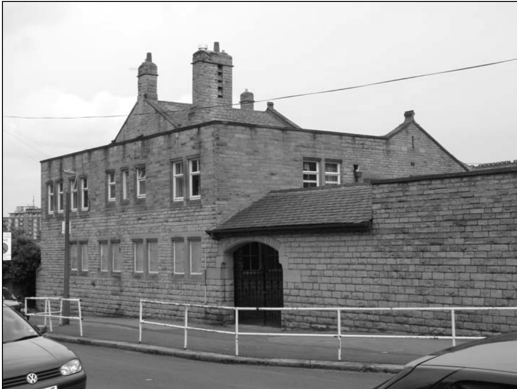
Plate 5 – West facing elevation (film 1.05)
