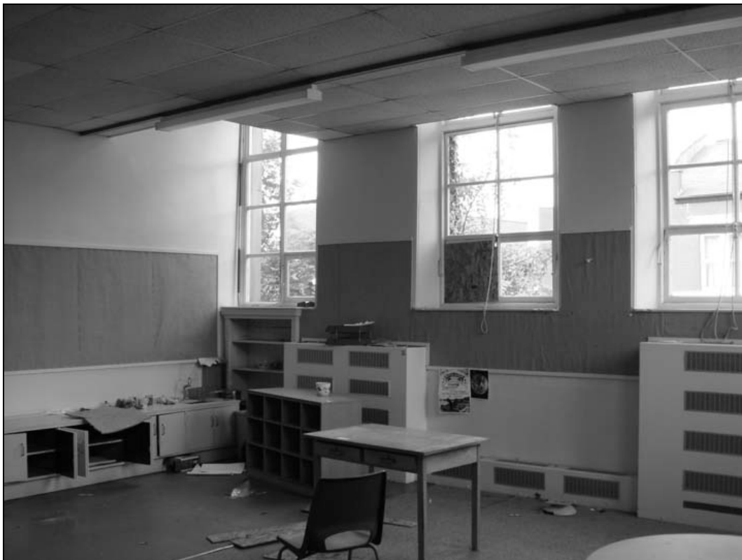
Plate 16 – General view of room G6 (film 2.29)
