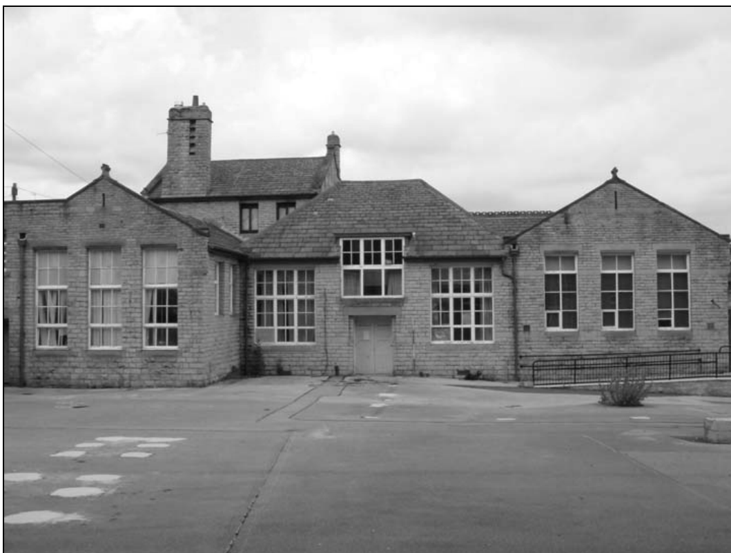
Plate 8 – Detail of south facing elevation (film 1.08)
