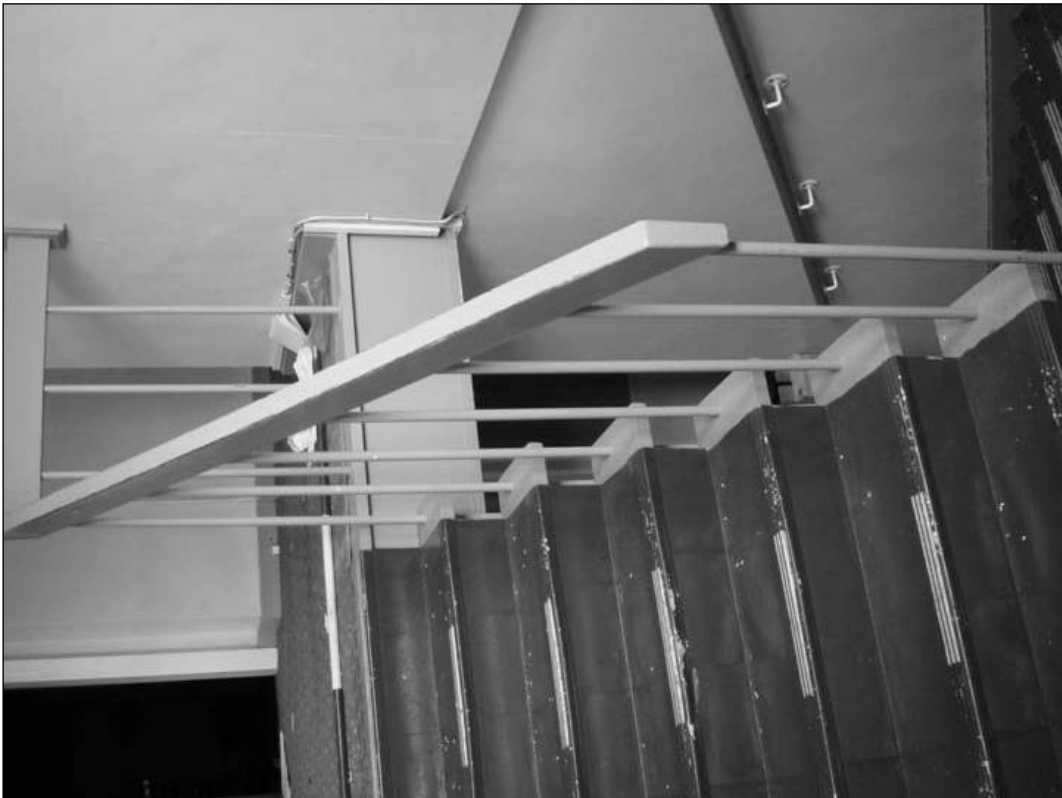
Plate 28 – General view of staircase between G12 & F1 (film 2.17)
