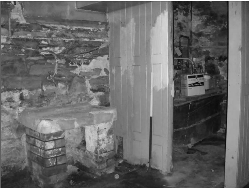
Plate 10 – Detail of stone sink and wooden screen in cellar B1 (film 2.08)
