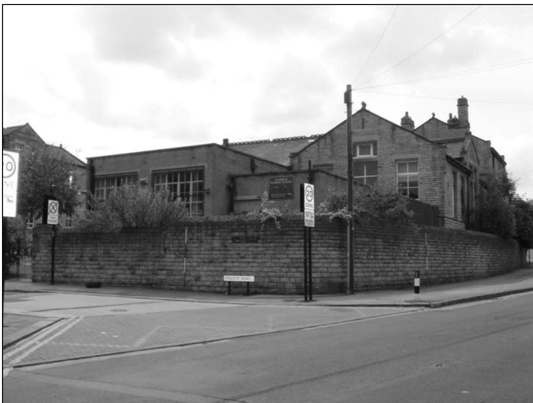
Plate 2 – General view of Sharrow Infants School, looking southwest (film 1.02)
