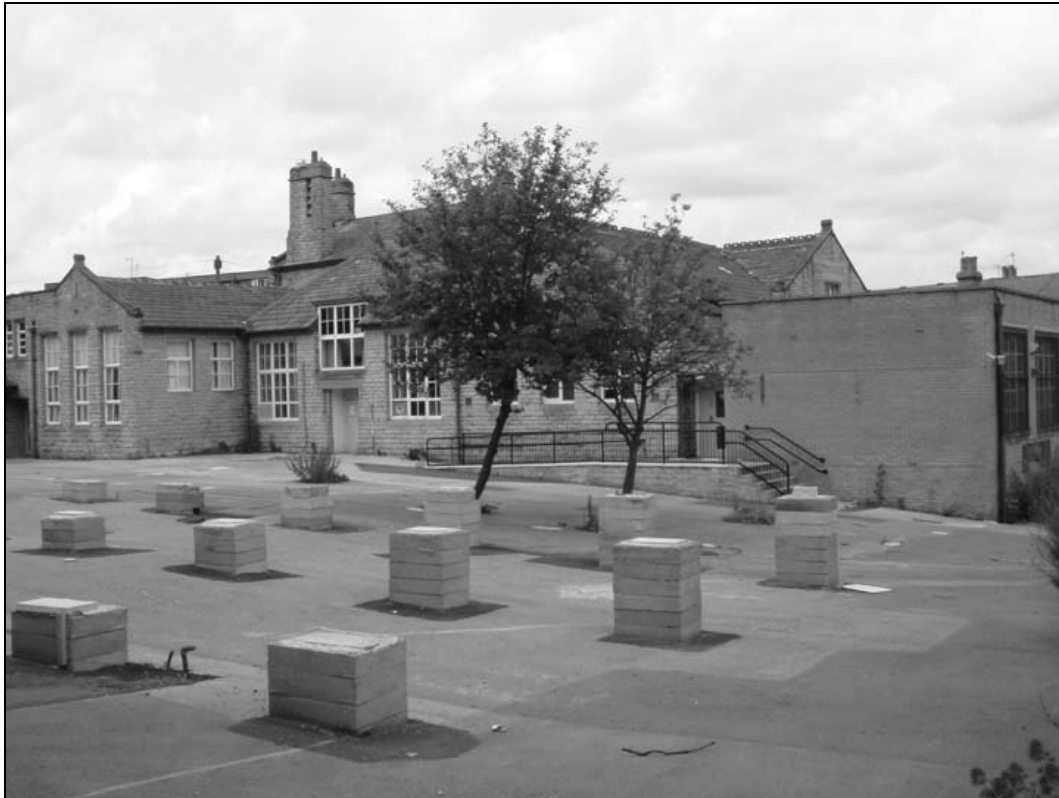
Plate 7 – General view of building from playground, looking northwest (film 1.07)
