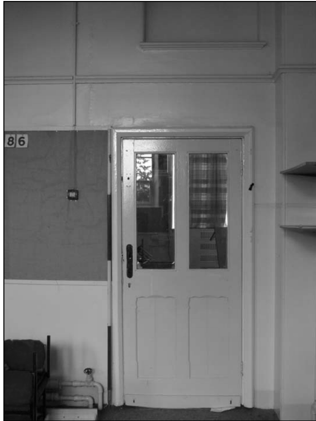
Plate 19 – Detail of paneled door in G8; note blocked window above (film 2.27)
