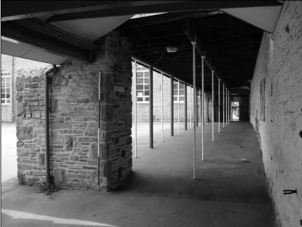
Plate 9 – General view along covered walkway adjacent to western boundary wall (film 1.09)
