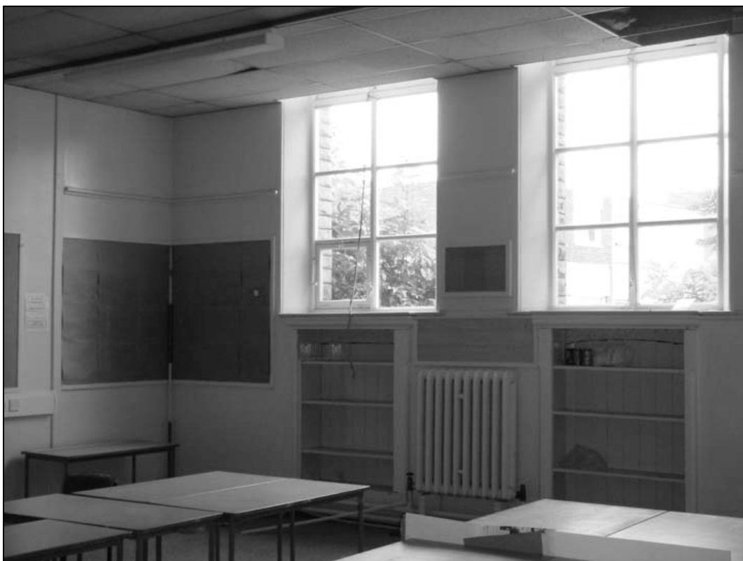
Plate 18 – General view of G8; note fitted cupboards beneath windows (film 2.26)
