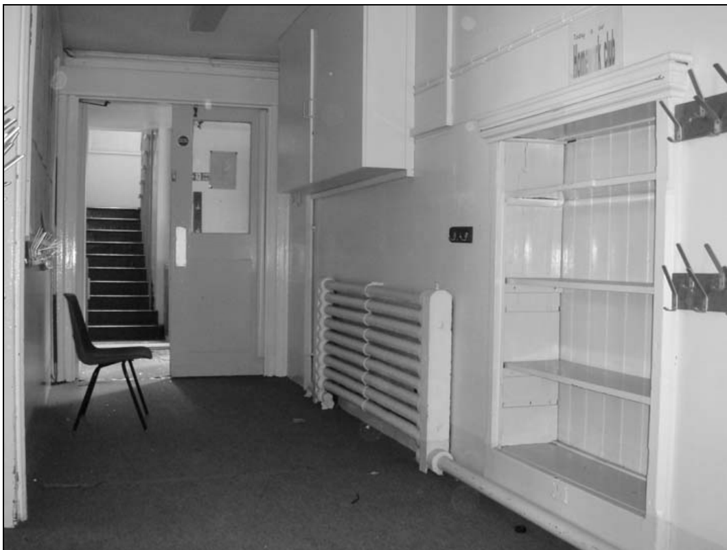
Plate 22 – General view of corridor G10; note radiator and recessed cupboard (film 2.23)
