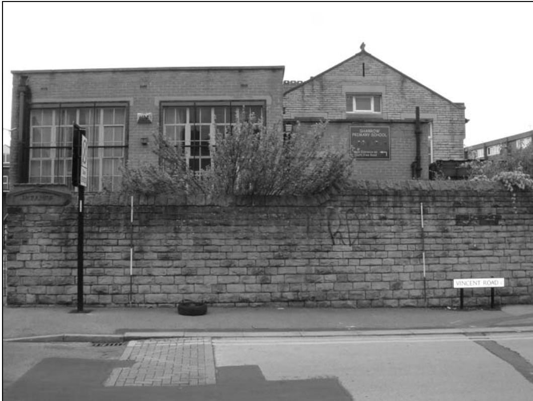
Plate 1 – East facing elevation of Sharrow Infants School (film 1.01)
