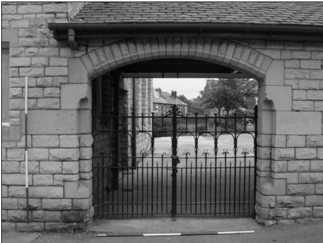
Plate 6 – Detail of iron gate in western boundary wall (film 1.06)
