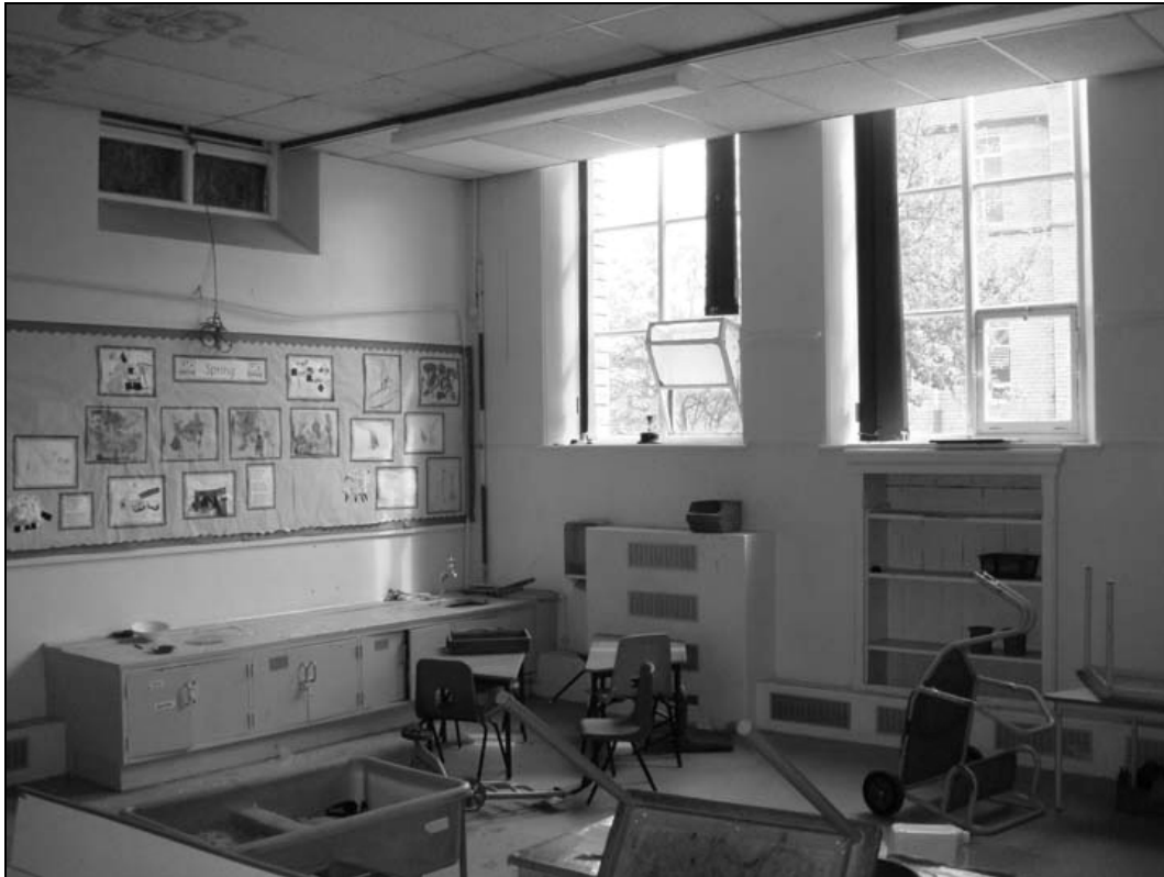
Plate 15 – General view of G3; note cast iron window hopper (film 2.32)
