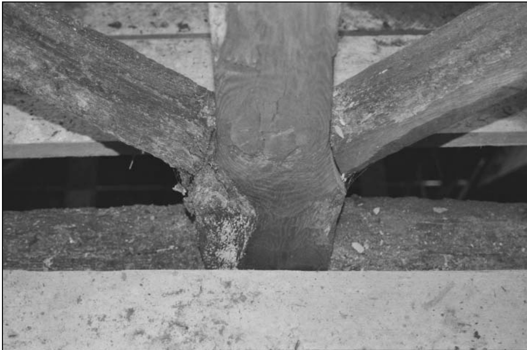
Plate 64 - Detail of joggled king post in northern end of building (film 2.06)
