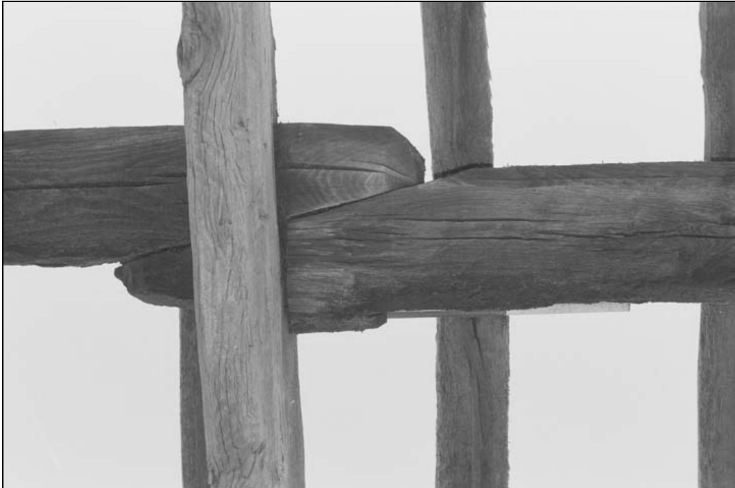
Plate 71 – Detail of lapped scarf joint of purlins (film 4.20)
