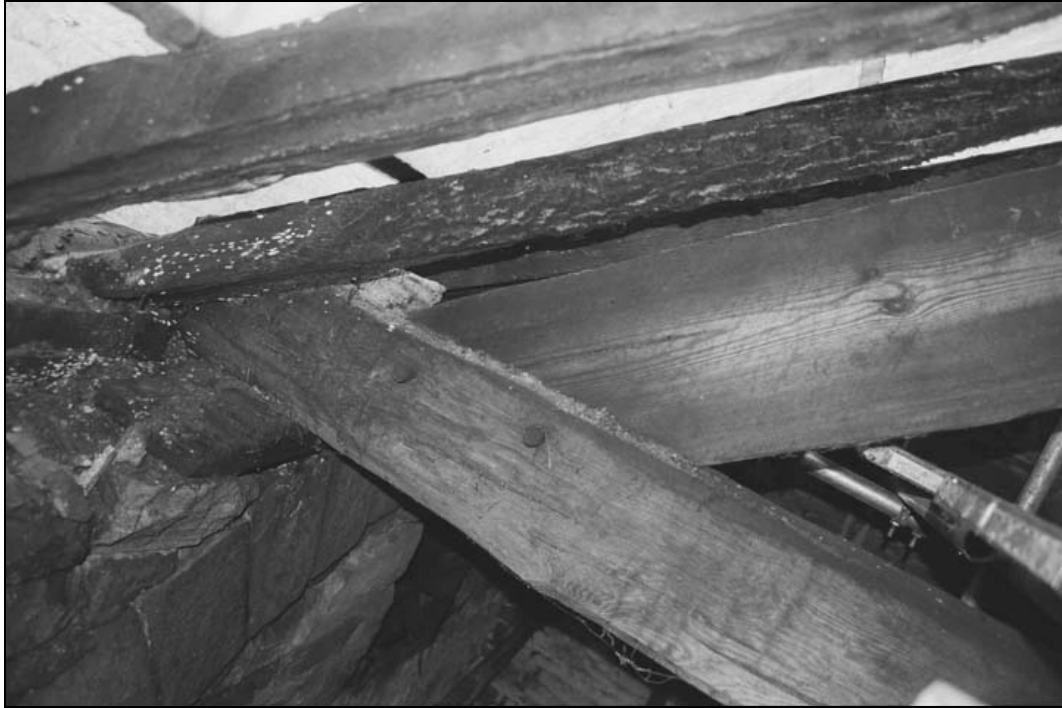
Plate 65 – Conjunction of principal and tie beam in northern part of building (film 2.02)
