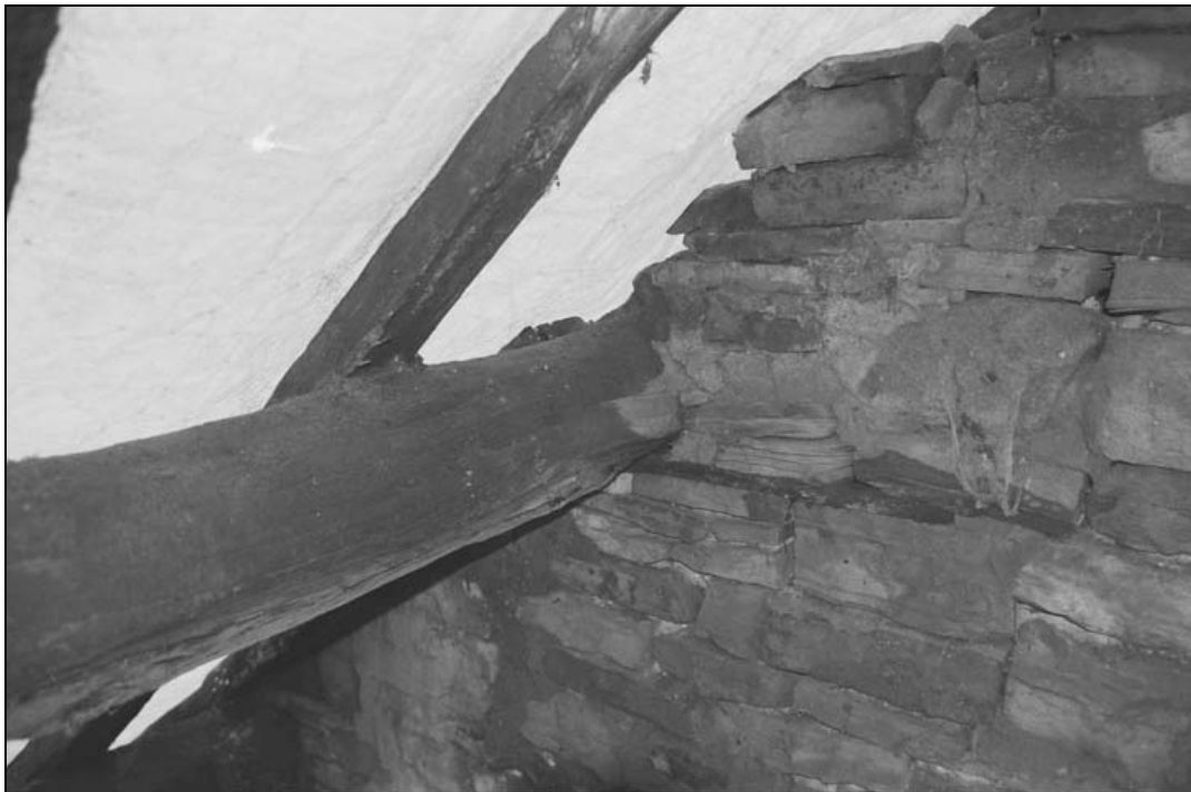
Plate 62 – Detail of purlin in northern end of building (film 2.25)
