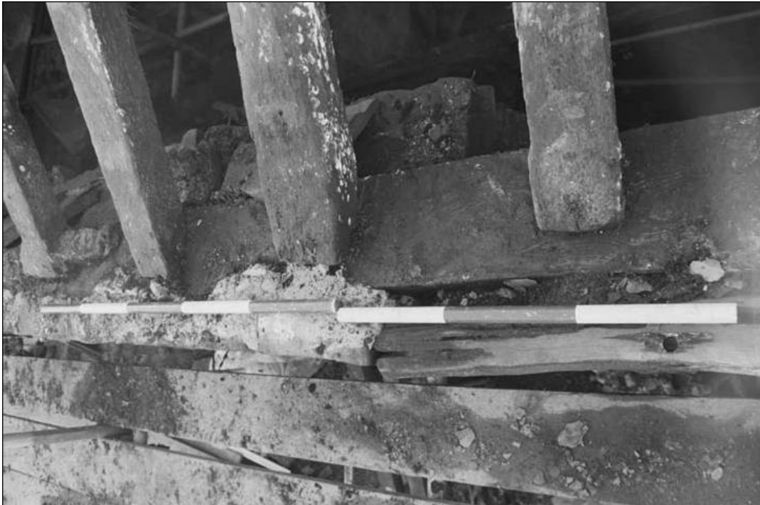
Plate 43 – Detail of wall plate of eastern wall (film 3.31)
