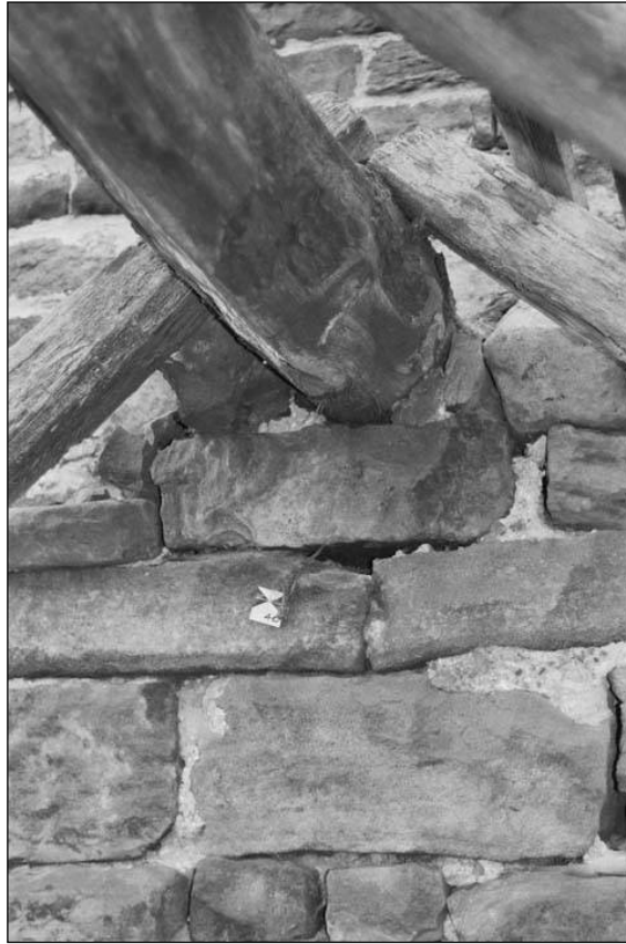
Plate 79 – Conjunction of southern end wall and ridge piece (film 3.05)
