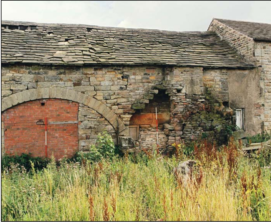
Plate 35 – General view of west facing elevation (film 1.06)
