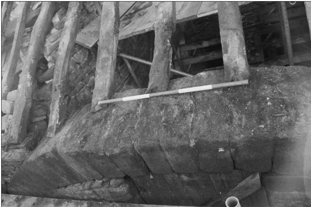
Plate 46 – Detail of common rafters resting on arch in east wall (film 3.14)
