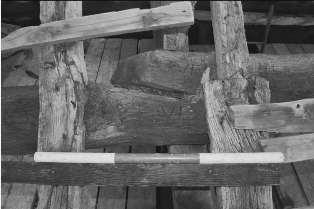
Plate 55 – 'VI' carpenter's marks, purlin ends (film 4.22) – 0.60m scale rod
