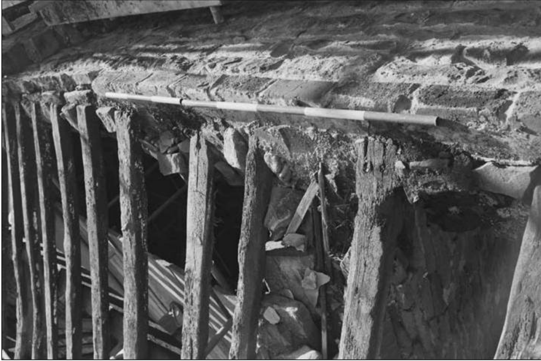
Plate 54 – Detail of wall plate in west wall (film 4.31)
