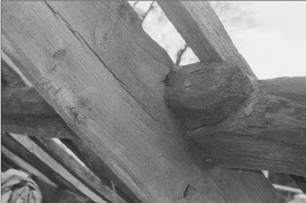
Plate 77 – Detail of notching-in of purlins in southernmost truss (film 3.03)
