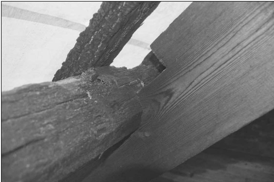
Plate 72 – Halved joint of purlin and principal, northern part of building (film 2.30)
