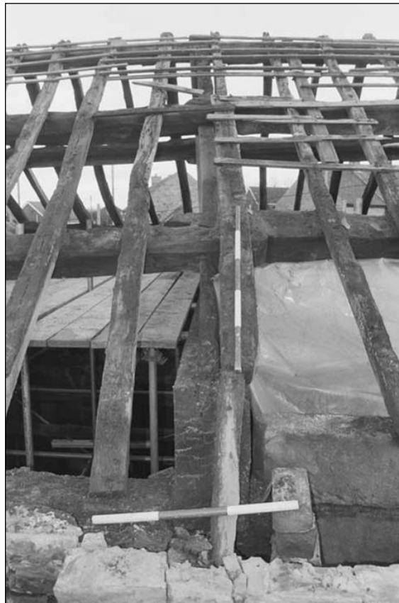
Plate 56 – View along southernmost truss (film 4.23)
