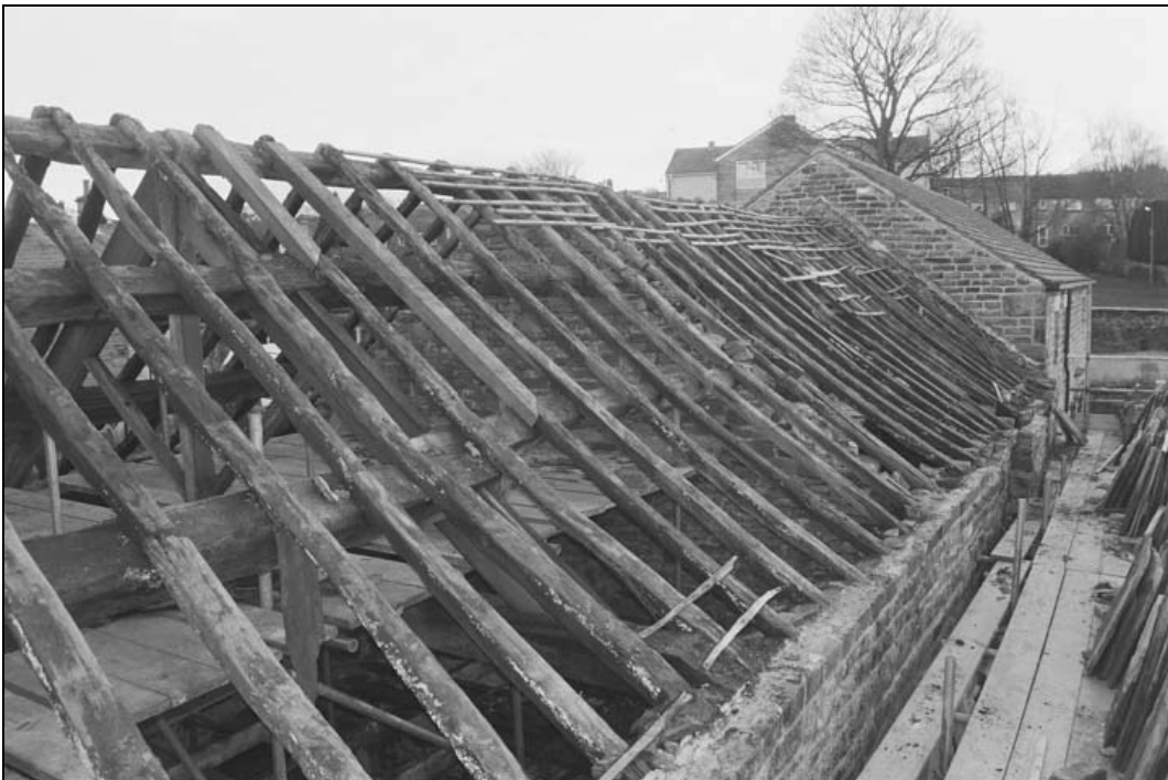
Plate 50 – General shot of roof (film 4.26)
