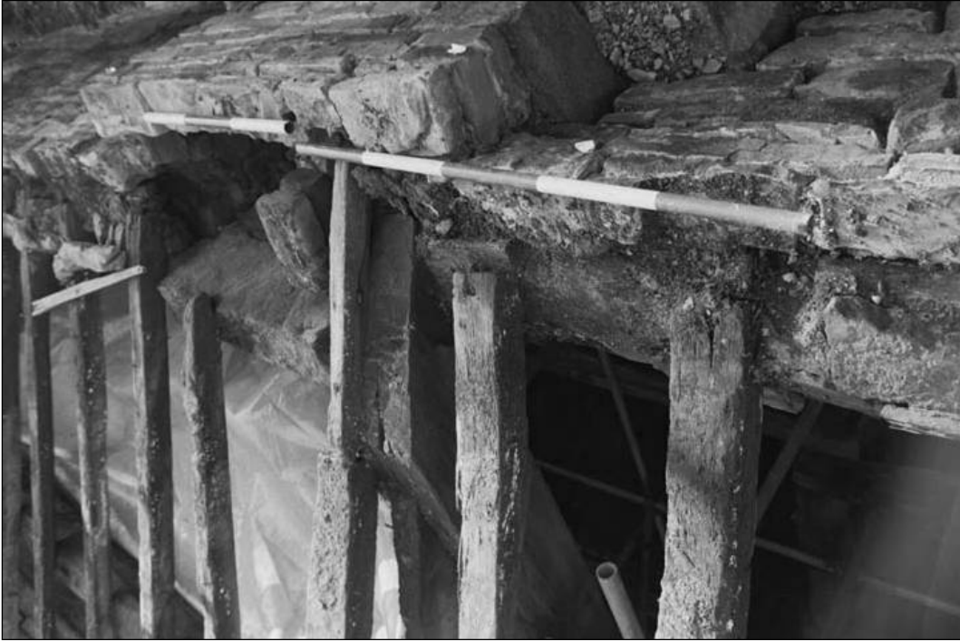
Plate 57 – Detail of wall plate, west wall (film 4.33)
