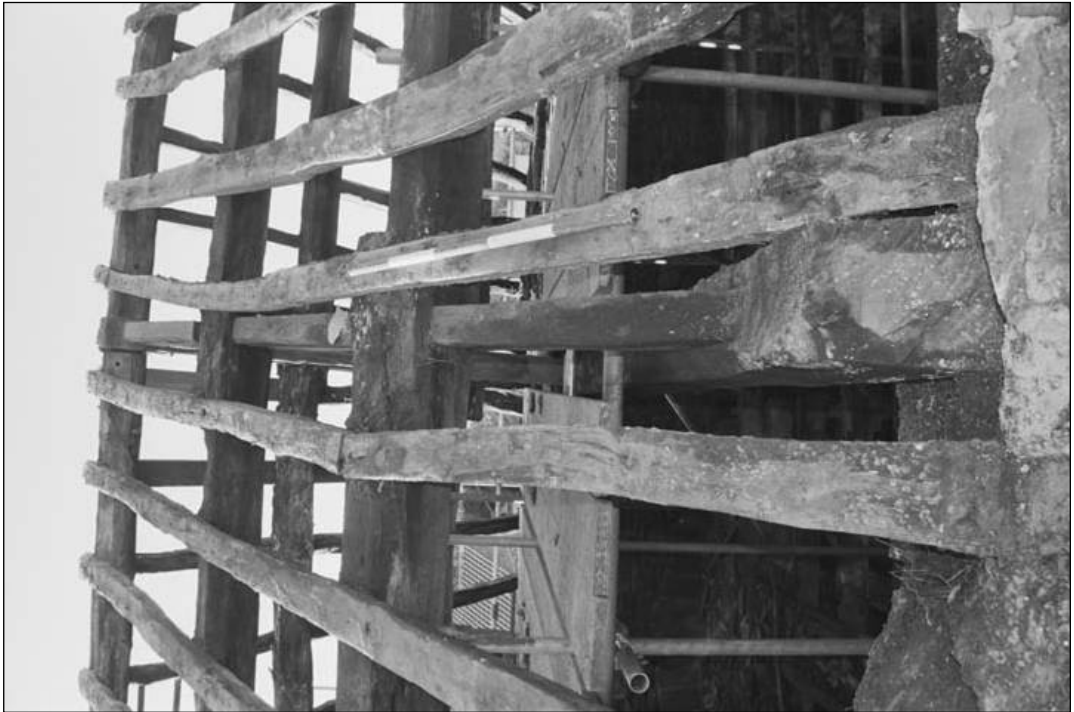
Plate 47 – General view along northernmost truss (film 3.12)
