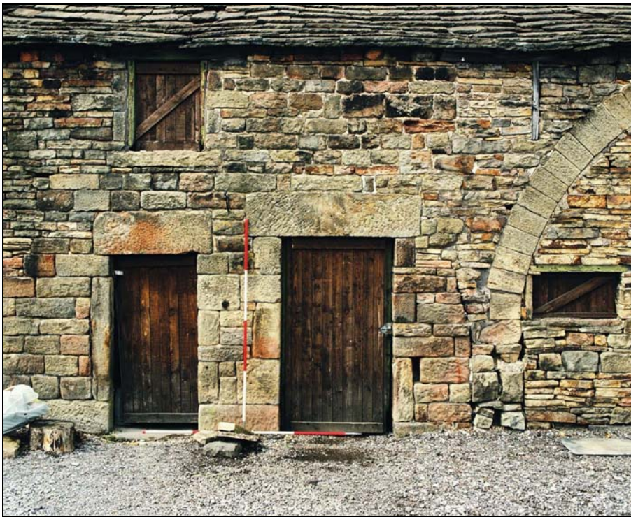
Plate 30 – Detail of rebuilt walling replacing external lehr chimneys in east facing elevation (film 1.02)
