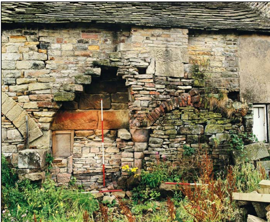
Plate 36 – Detail of fragmentary remains of lehrs in west elevation (film 1.07)
