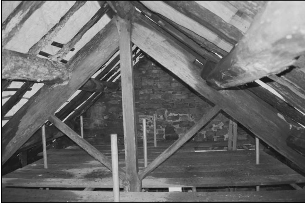
Plate 63 – Detail of roof truss in northern end of building (film 2.11)
