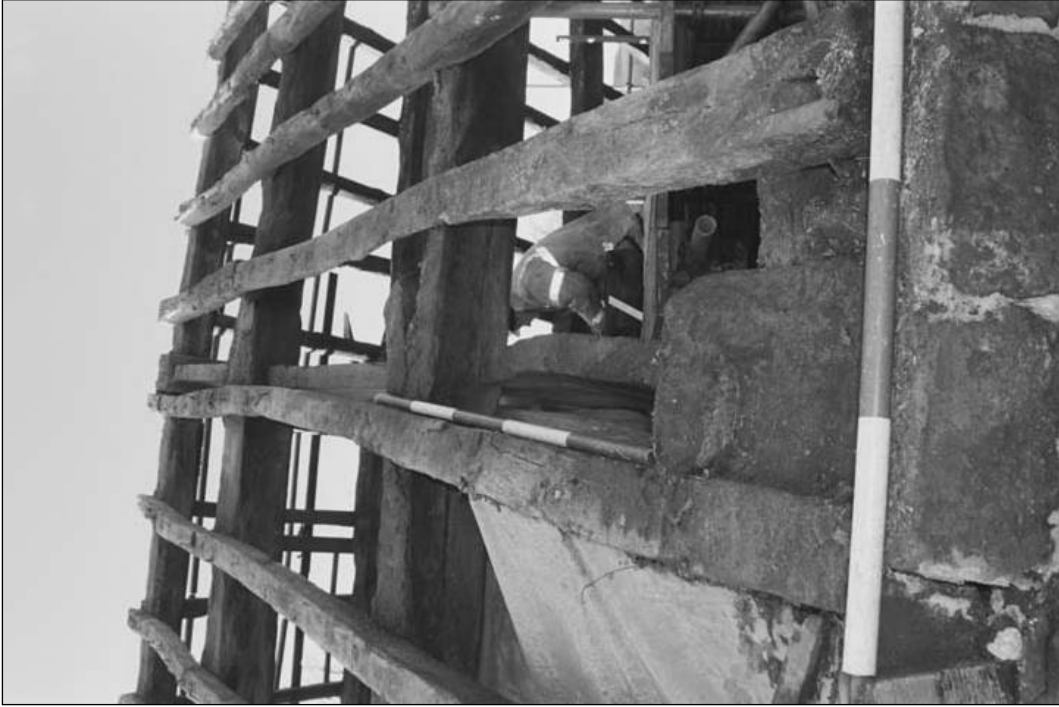
Plate 44 – Conjunction of south tie-beam and wall plate (film 3.20)
