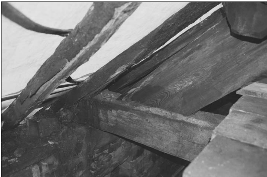
Plate 78 – Conjunction of tie beam and principal, northern part of building (film 2.05)
