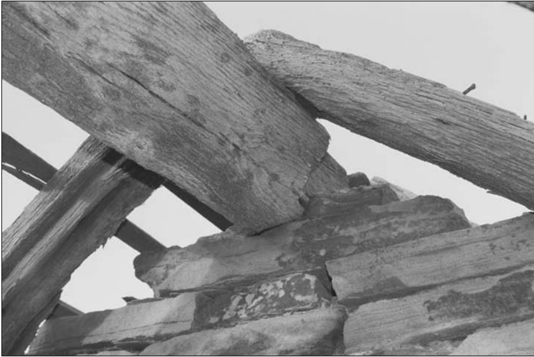
Plate 73 – Detail of ridge and gable wall (film 3.01)
