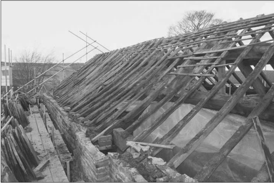
Plate 49 – General shot of roof (film 4.21)
