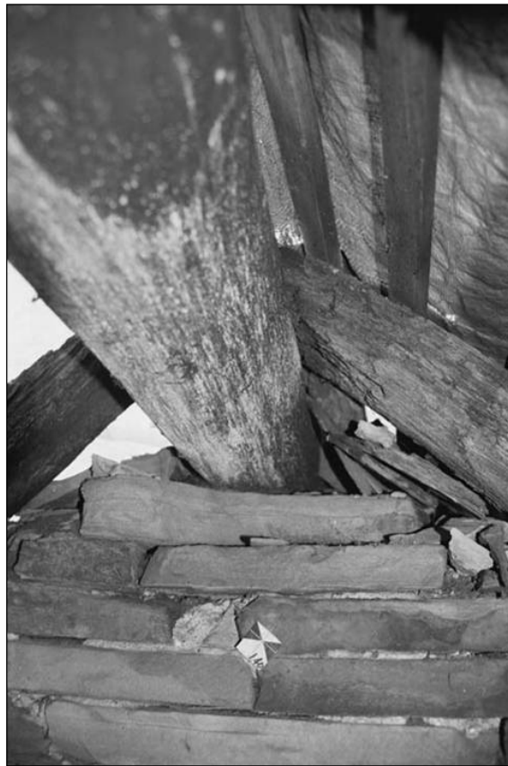
Plate 74 – Conjunction of ridge and gable in northern part of building (film 2.19)
