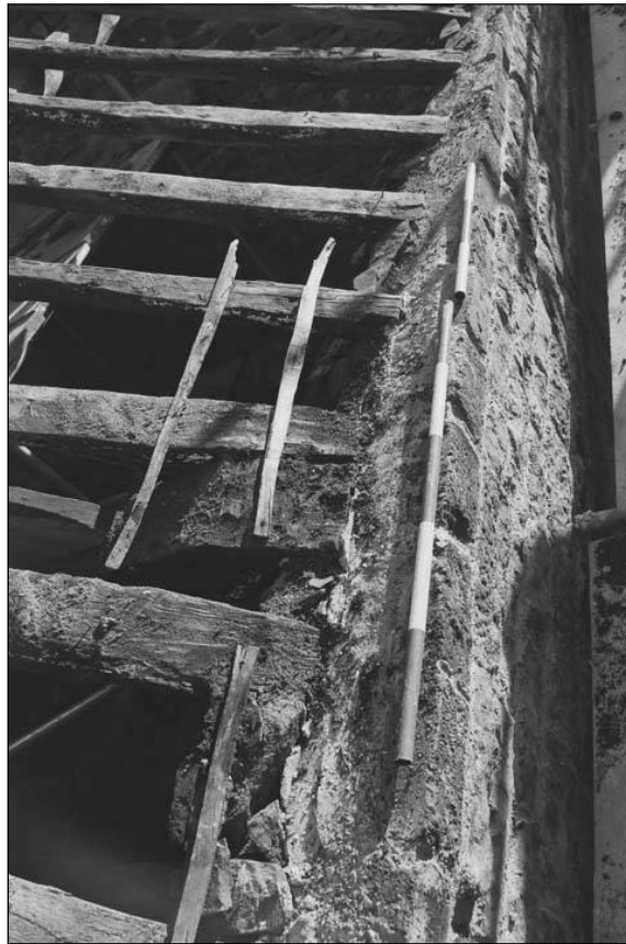
Plate 52 – Detail of wall plate in west wall (film 4.29)
