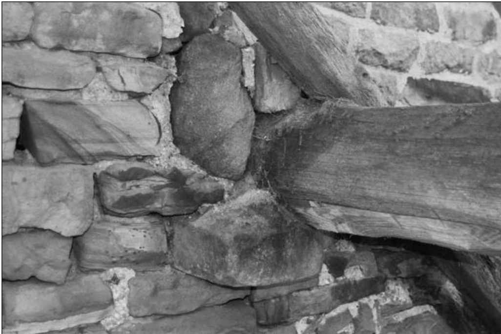
Plate 80 – Detail of corbel supporting purlin in southern end wall (film 3.04)
