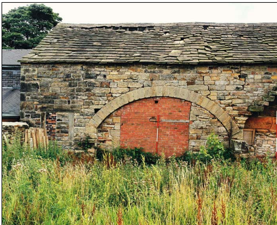
Plate 34 – General view of blocked arch in west facing elevation (film 1.05)
