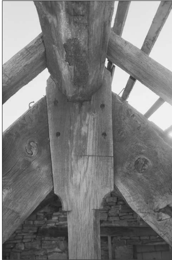
Plate 75 – Detail of king post of southernmost truss (film 3.07)
