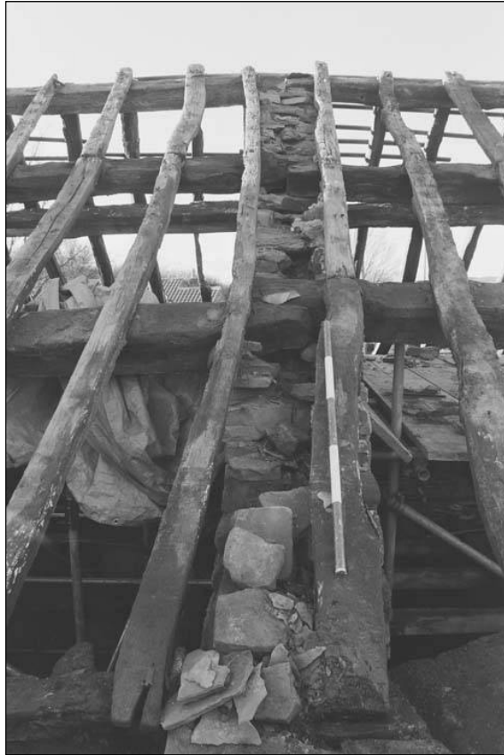
Plate 45 – General view along central wall from east side (film 3.15)
