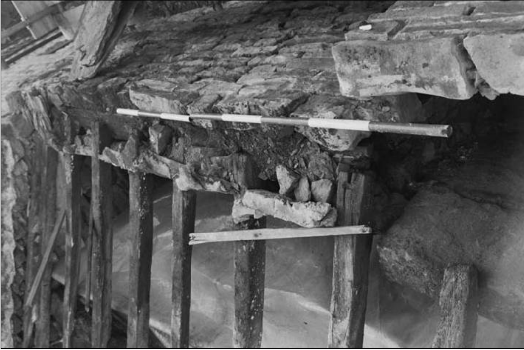
Plate 59 – Detail of wall plate in southernmost end of the western wall (film 4.34)
