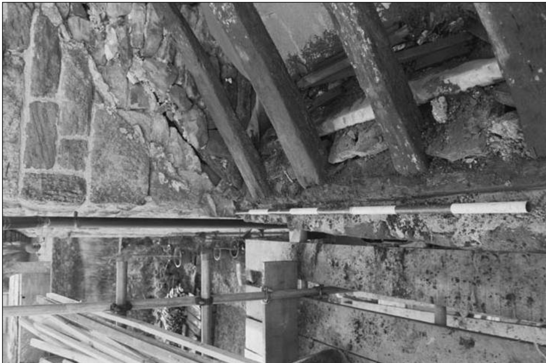
Plate 39 – Detail of wall plate, southernmost end of east wall (film 3.34)
