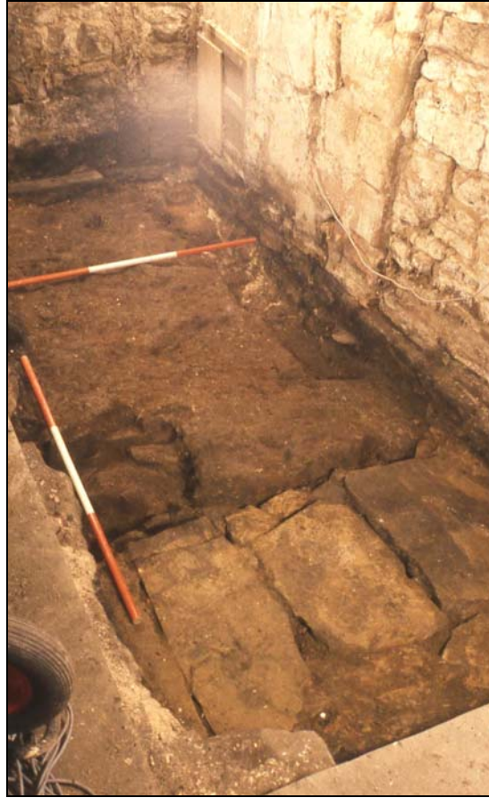
Plate 7 – 1986 excavation: slabs covering subsidiary furnace flue (facing northwest) © David Barrett
