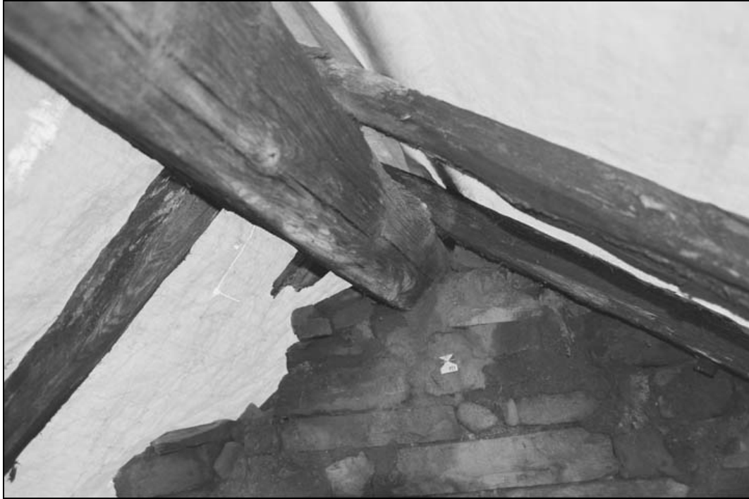
Plate 61 – Detail of ridge piece in northern end of building (film 2.26)
