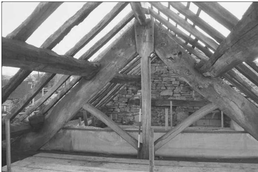
Plate 76 – Elevation of southernmost truss (film 3.09)
