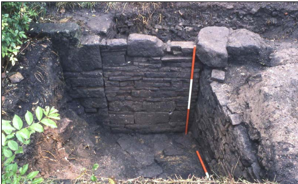
Plate 2 – 1986 excavation: later blocking of furnace flue (facing east) © David Barrett
