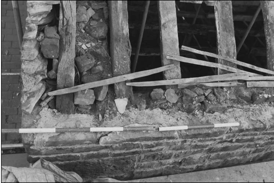
Plate 51 – Detail of wall plate, west wall (film 4.27)
