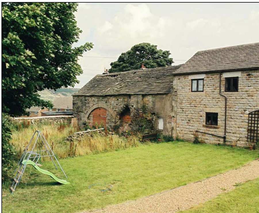
Plate 38 – General view of west facing elevation (film 1.09)
