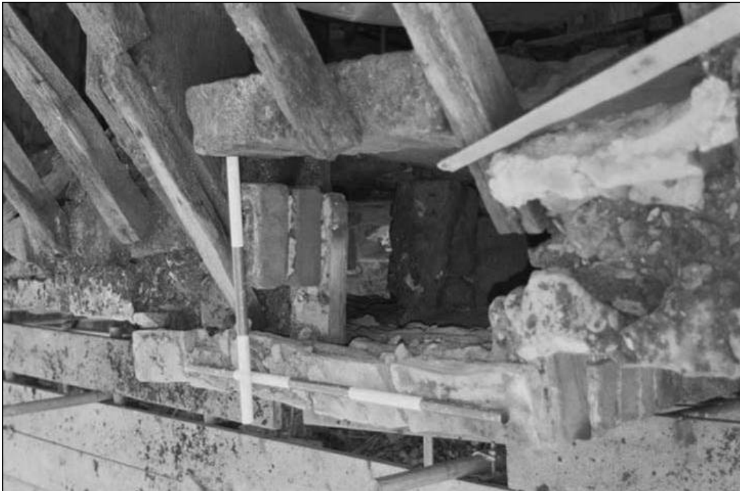
Plate 58 – Detail of chimney in west wall (film 4.24)
