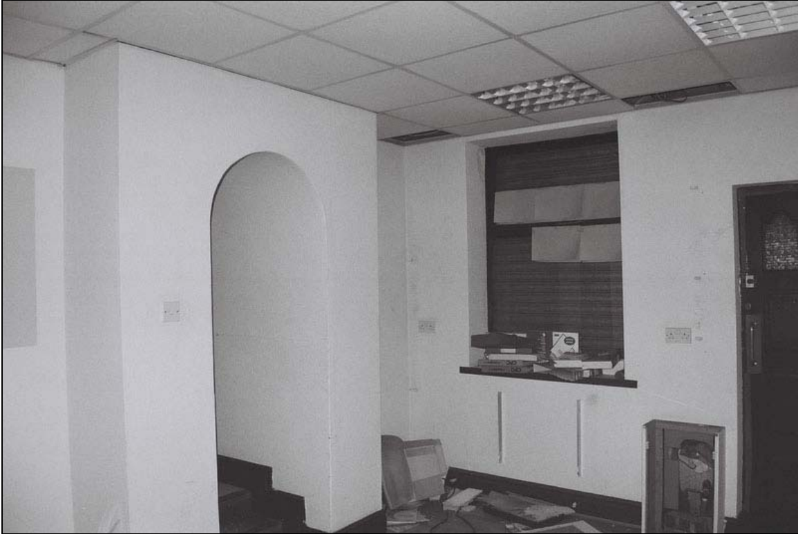
Plate 7: General view of room G2 looking north west (film 1.6)
