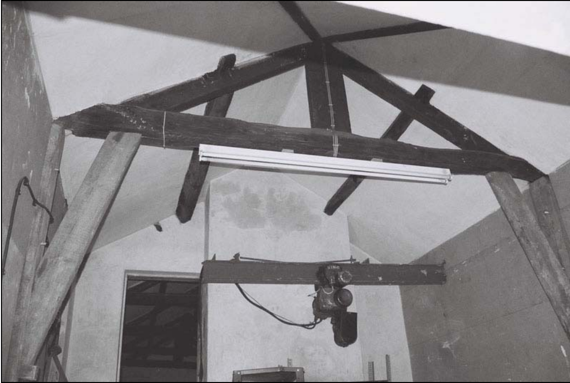
Plate 20: General view of room S5, note crane for taking in door and king post truss with later timber brackets (film 1.23)
