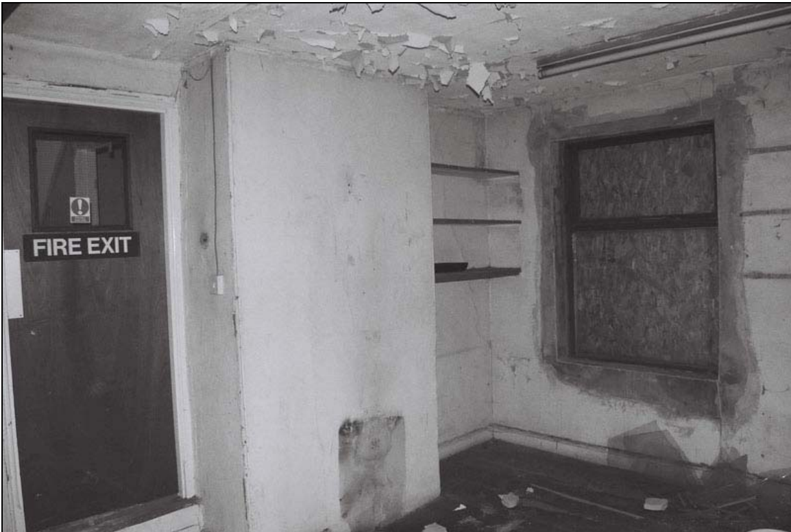
Plate 13: General view of room F2 looking north west (film 1.15)
