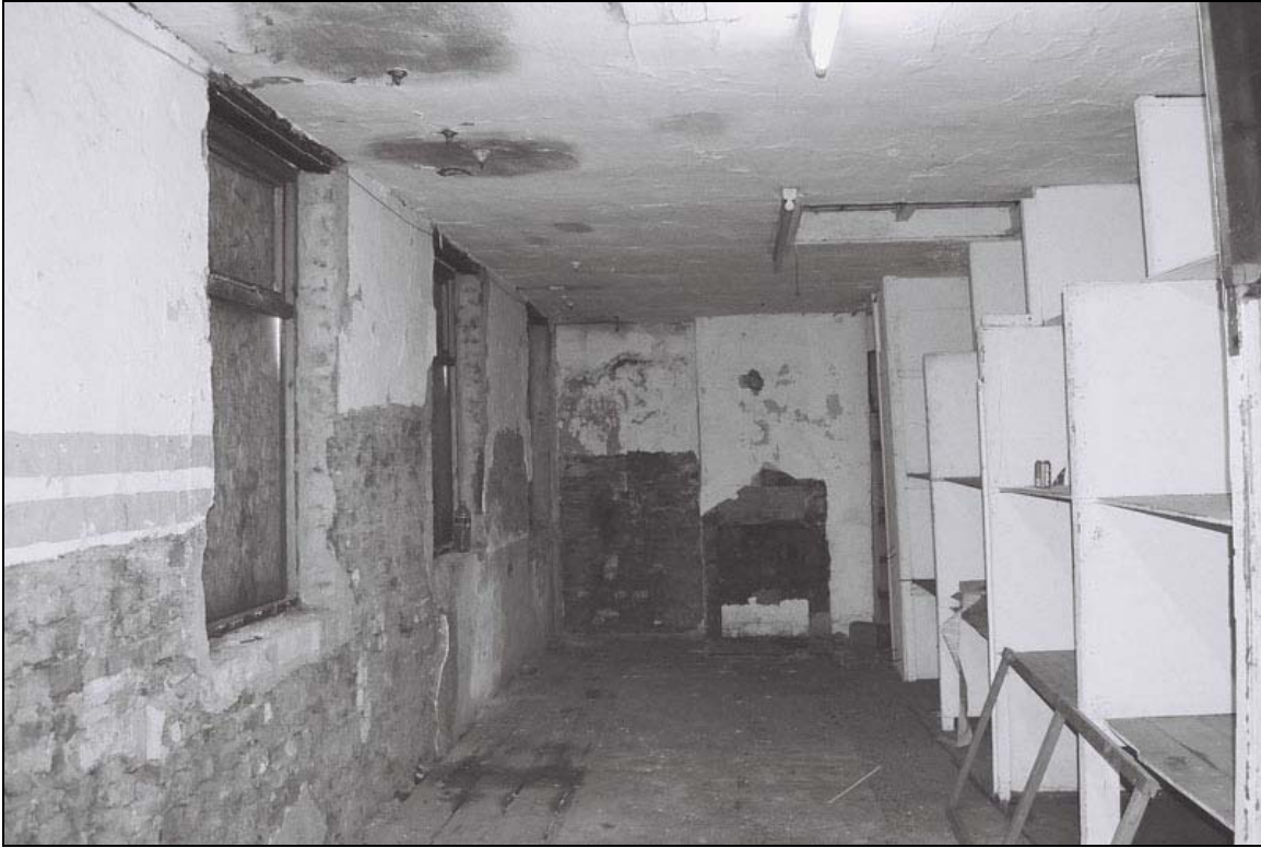
Plate 24: General view of room F9 looking south, note blocked fireplace (film 1.13)
