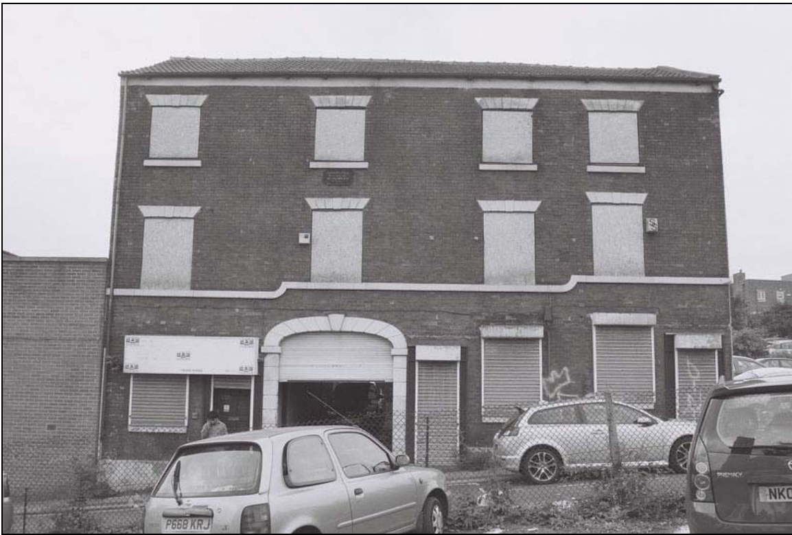
Plate 3: General view of north elevation of building (film 1.30)
