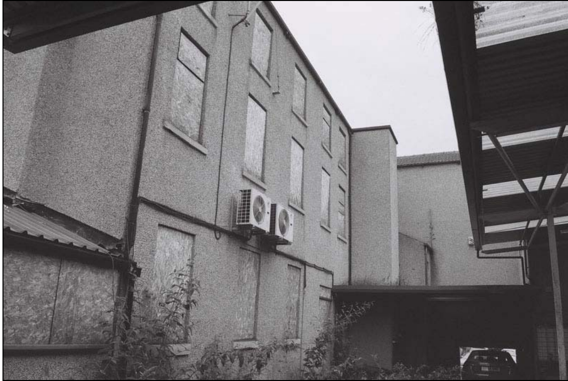
Plate 22: General view of east elevation of building, note rendering and converted doorway situated on ground floor (film 1.34)
