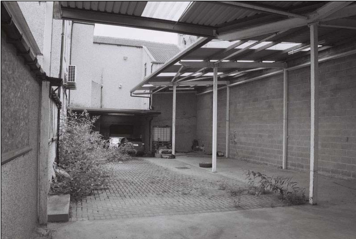
Plate 5: General view of central yard, note modern brick and concrete floor (film 1.33)
