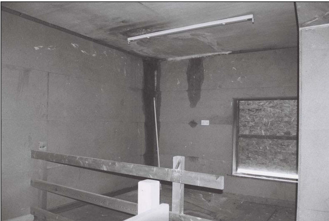
Plate 19: General view of room S1 looking north (film 1.22)
