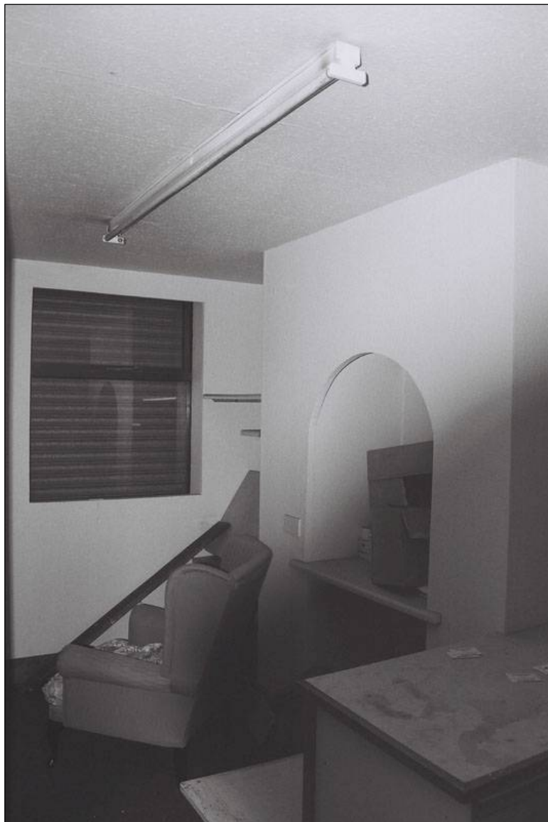
Plate 9: General view of room G3 looking north east (film 1.27)
