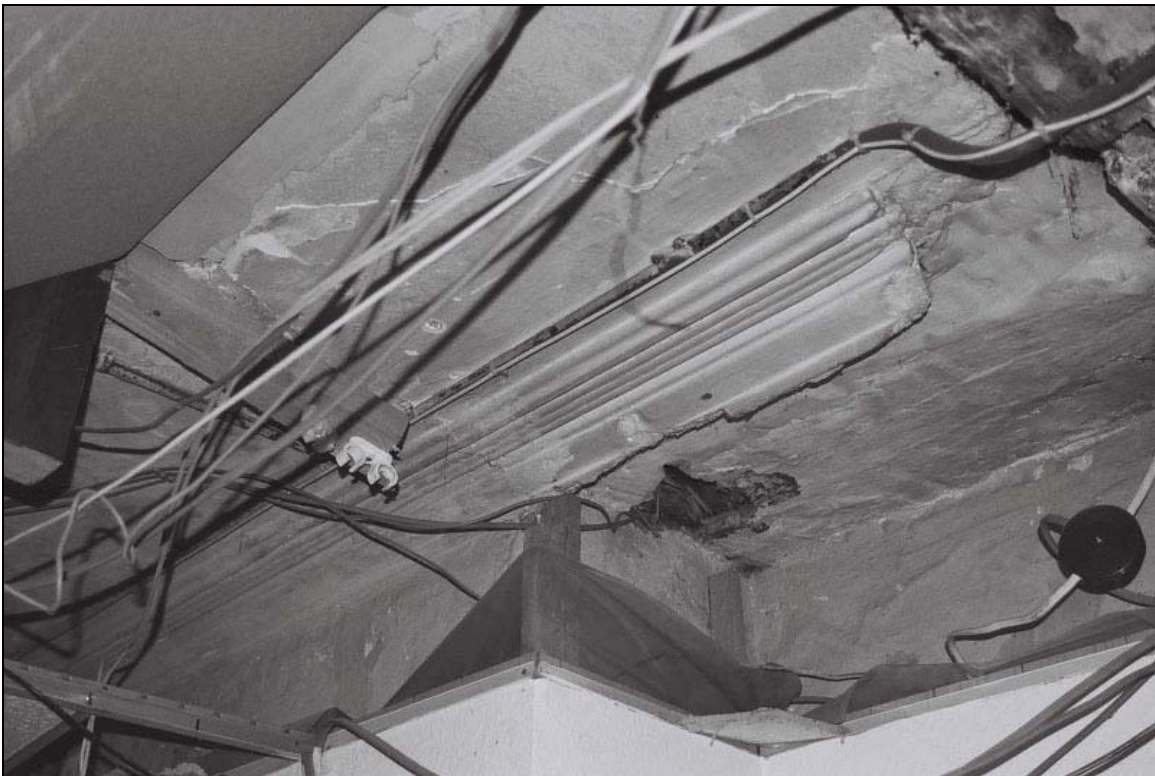
Plate 11: Room G1, detail of plaster cornice above suspended ceiling (film 1.5)
