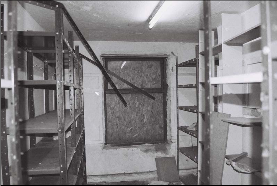
Plate 14: General view of room F3 looking north (film 1.16)
