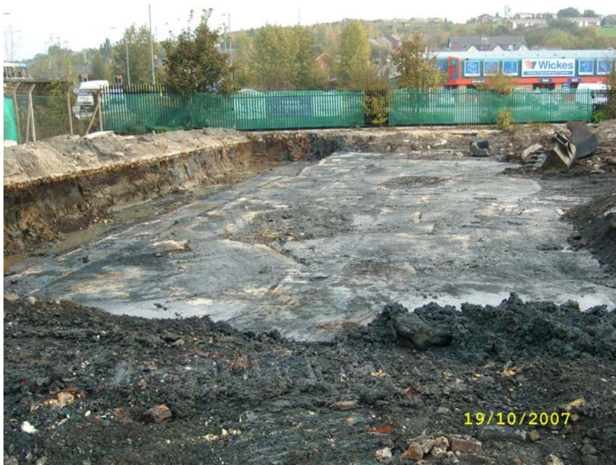
Plate 12: Area A4 – view of concrete slab
