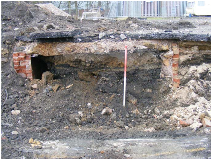
Plate 20: Walls [043] and [044] recorded within Area B2-A, probably associated with the Booster House
