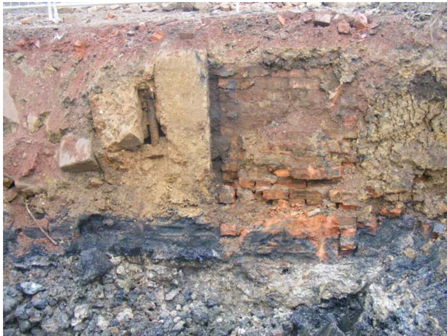
Plate 8: Sandstone block [010] with a vertical iron bar and concrete wall [011] associated with the Exhauster House
