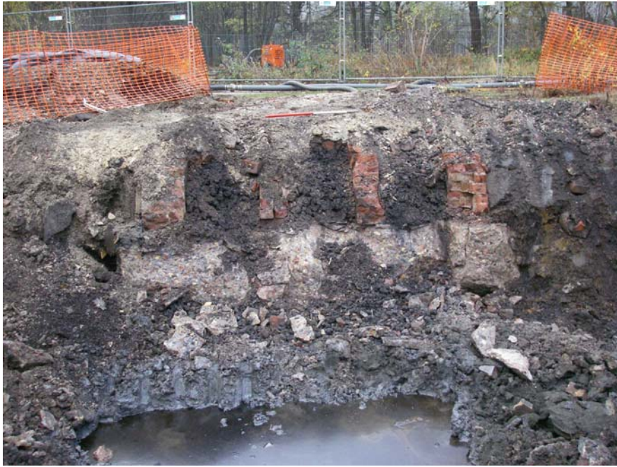
Plate 13: Four red brick walls [027] built on a 0.8 – 1m thick gas works concrete slab within Area A6
