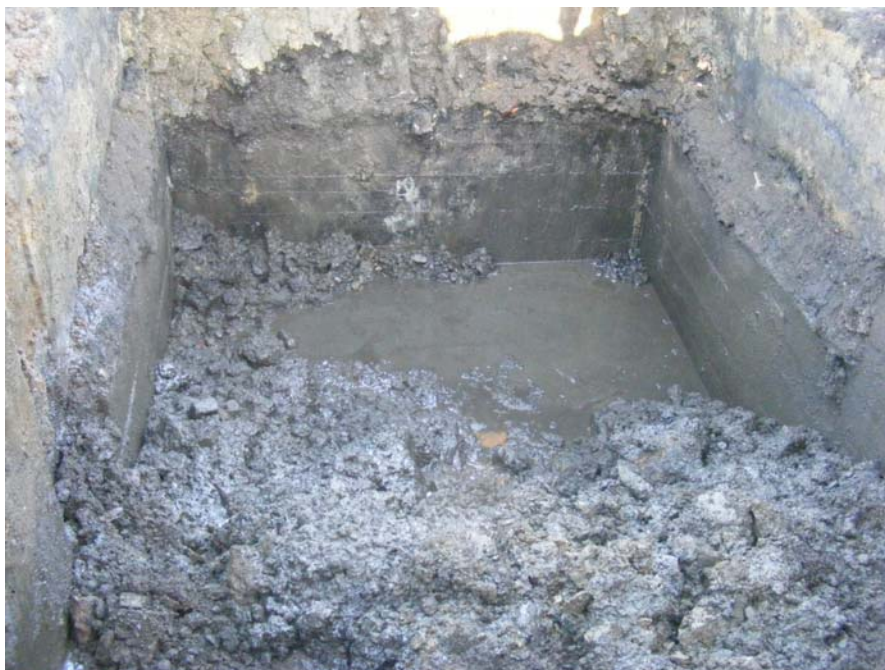
Plate 4: A large concrete 'hopper' [005] recorded to the north-east of the Retort House
