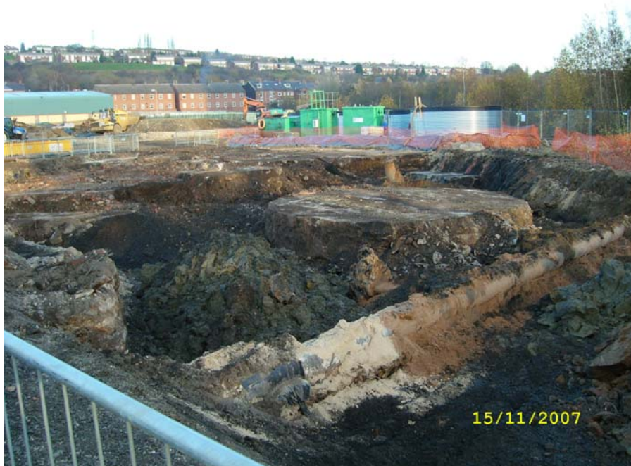
Plate 18: Concrete fuel tank base within area B2
