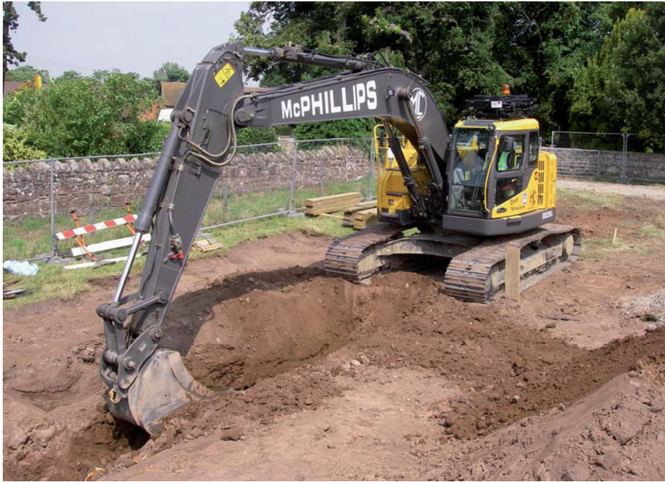
Plate 1 Excavating pipe trench looking north-west
