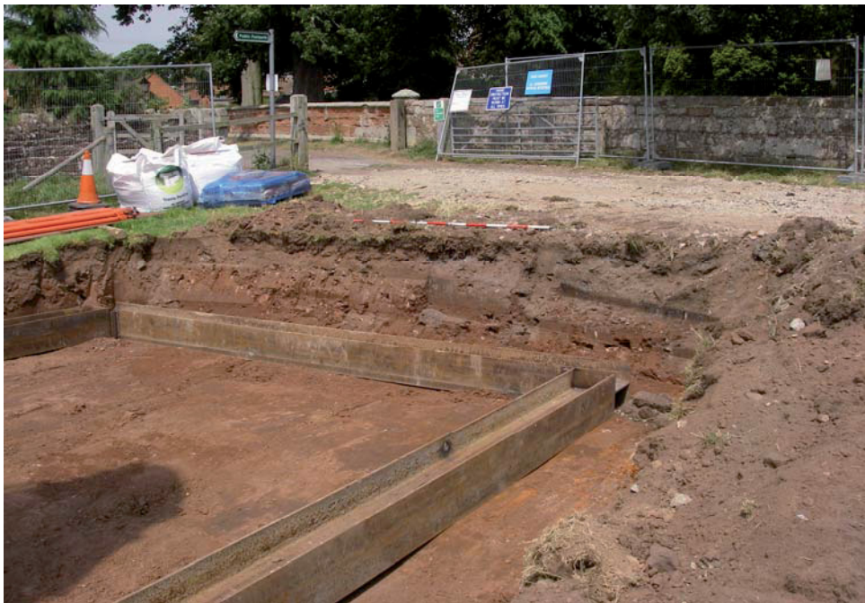
Plate 2 Trench for overflow chamber in north-west corner excavated to 1.20m depth
