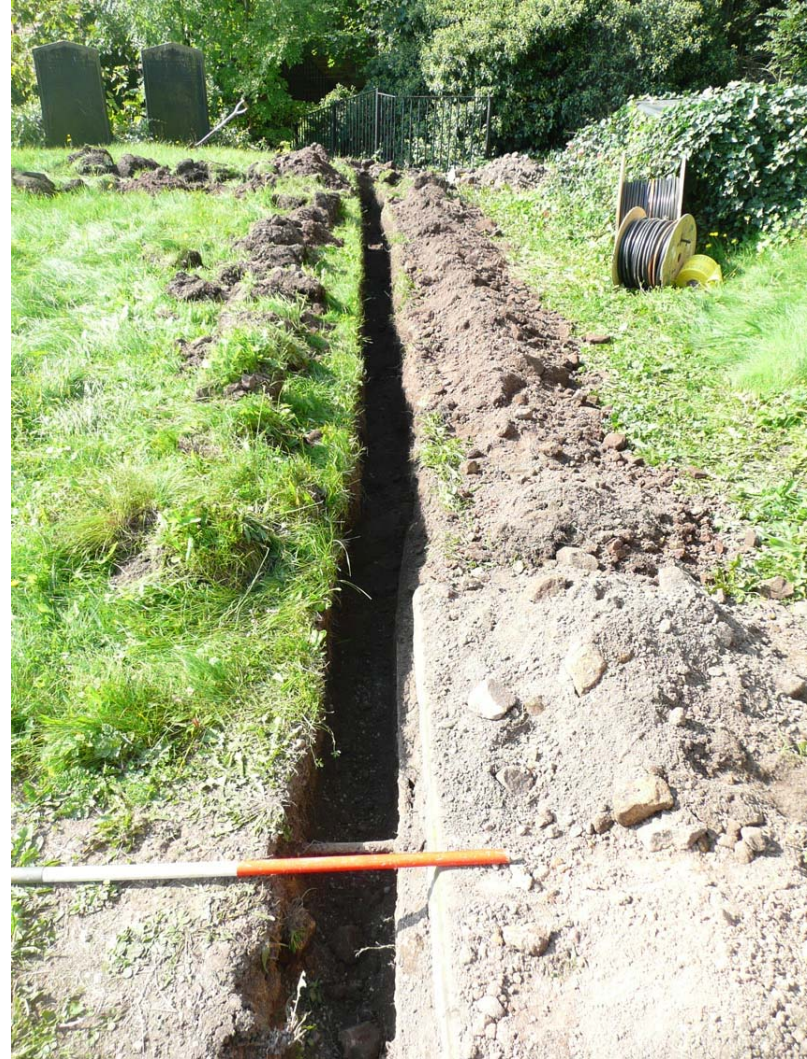
Plate 2 Trench to the south of the church
