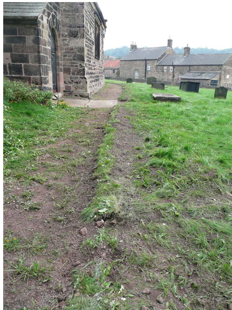
Plate 8 Backfilled trench to south of the church
