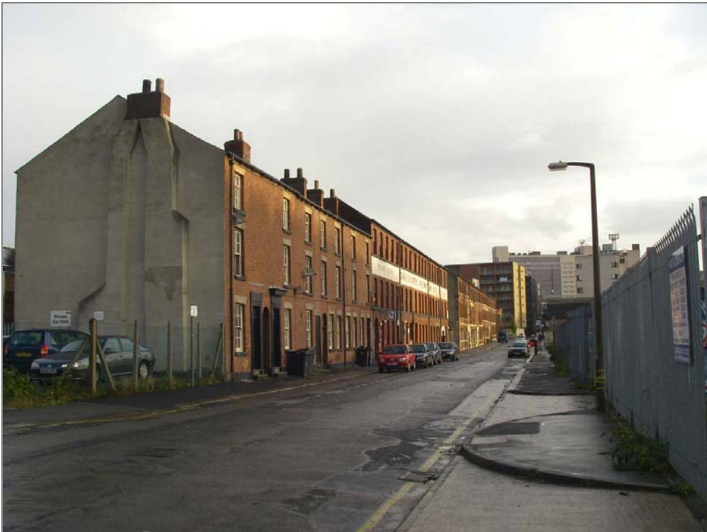
Plate 1 – View northeast along Milton Street showing the range of Grade II and Grade II* Listed Buildings opposite the application area
