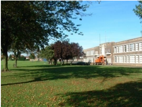
Plate 1: Pre-excitation shot of southern extents of development site, looking north
