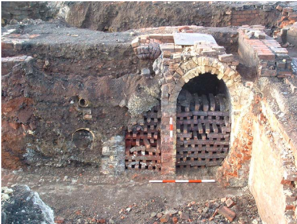
Plate 22: Facing site W. Showing a profile through the Alpha gas regenerative furnace. Note the brick arch extending to the right of the photograph suggesting further chambers to the north. Note also the difference in the widths of the hot air chamber to the left and the cold air chamber to the right.
