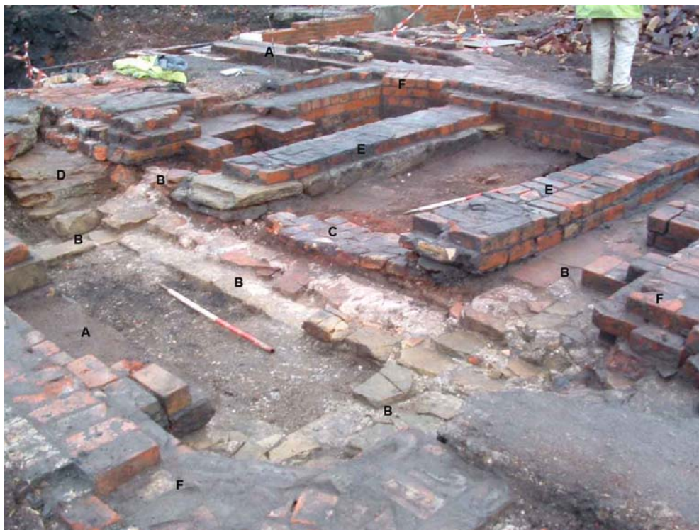
Plate 18: Facing site SE. Showing the cross struts (B) between the large stone walls (A) forming a possible early boiler base. The heavy heat damage is noticeable as pink discolouration and was also evident on the brick furnace floor (C). Note also the north western corner of Chimney III (D) and the phase 3 boiler base (F) with the boiler support cross struts (E).
