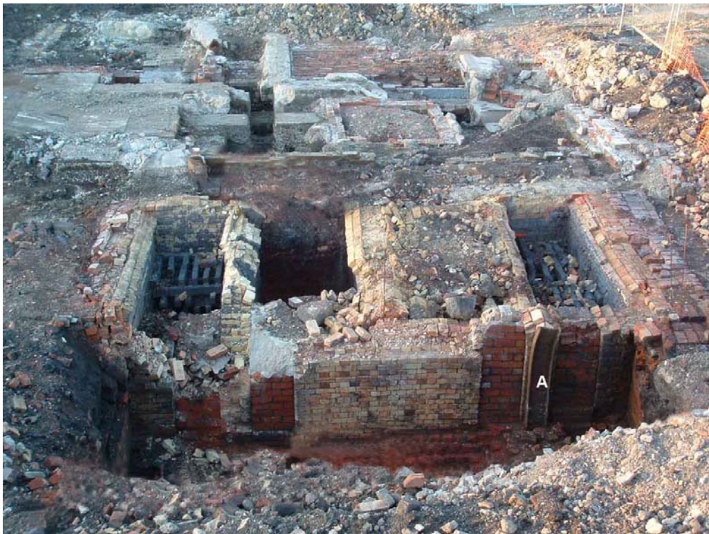
Plate 4: Facing site N. Showing the gas regenerative furnace in trench B3 after excavation. Note the four chambers. The two outer 'hot air' chambers were narrower and showed a higher degree of vitrification than those of the 'cold air' chambers in the middle. The in/out-let flue cellar was located in front of the furnace and the engine room was located immediately beyond. Note the structural support girder (A).
