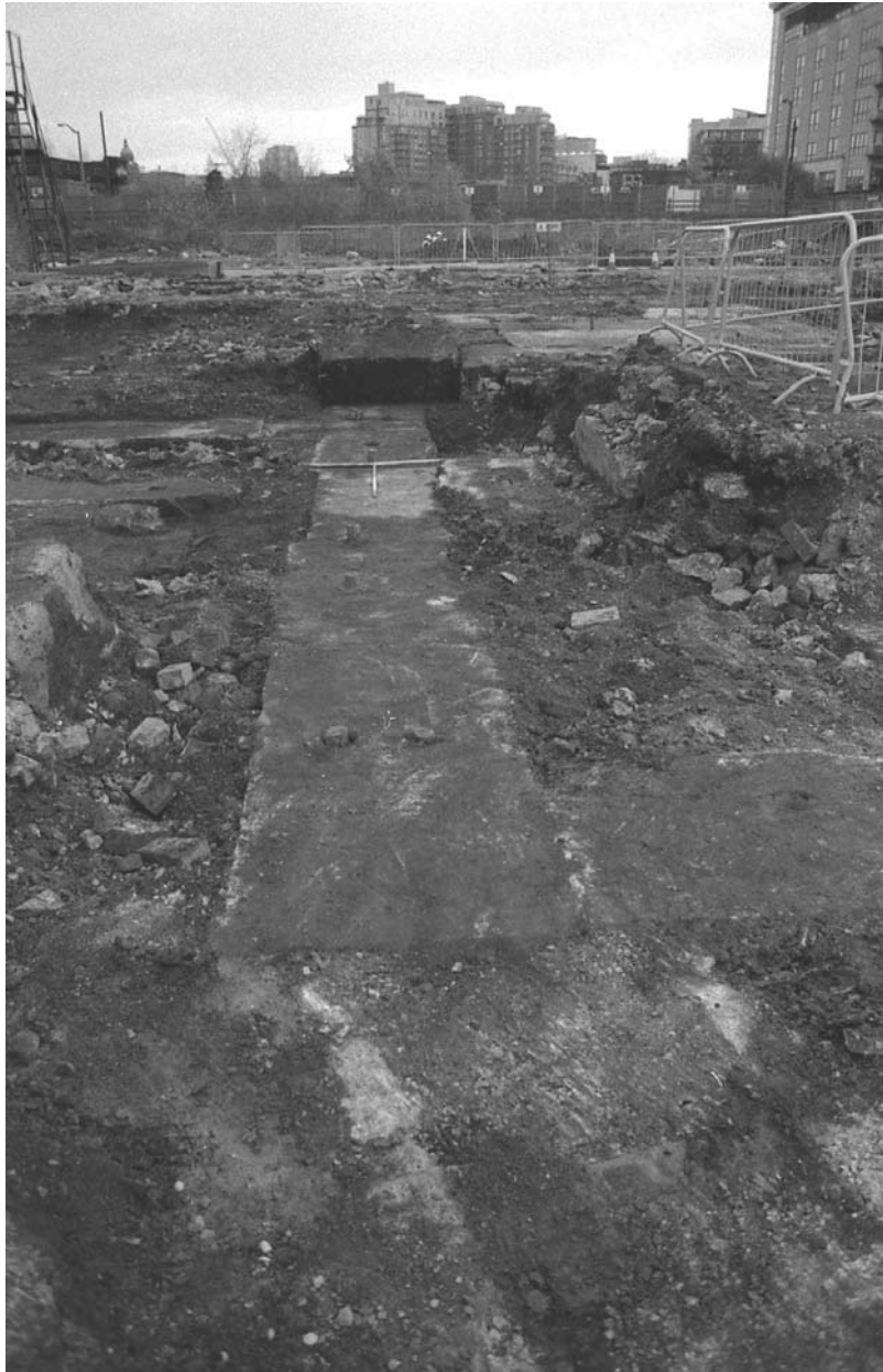
Plate 13: Facing site E. Showing part of the possible rolling mill stand 6020/6035 looking towards Trench C. This structure was uncovered in Strip and Record Area 1b and was linked to the bases uncovered in Trench C.
