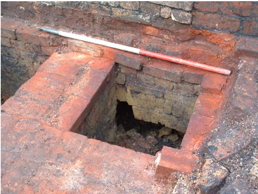
Plate 6: Facing site NW. Showing one of the flue voids entering the gas regenerator's eastern cold air chamber from the flue cellar. Note the arch built into the fabric of the connecting wall.
