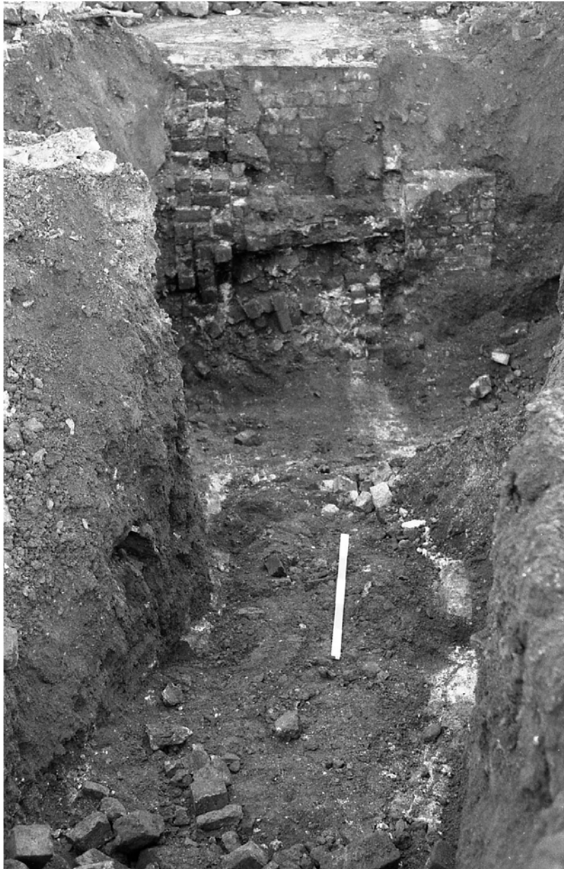
Plate 33: Facing site S. Showing the partially excavated curving flue 6058 and squared brick chimney 6059 (top of picture) which were uncovered during the early watching brief. It is possible that these structures may be linked to the earliest puddling phase of operation under Stephen Witham.
