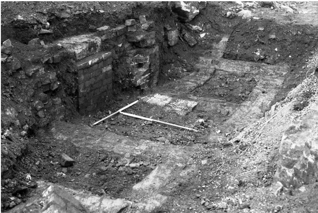
Plate 32: Facing site NE. Showing the structure 6160 uncovered during the Strip and Record Area 2a. This structure is depicted as early as 1888 and may have associations with the iron puddling process.
