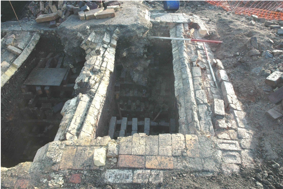
Plate 5: Facing site S. Showing the lattice or 'checkerboard' bricks within the western cold and hot air chambers.
