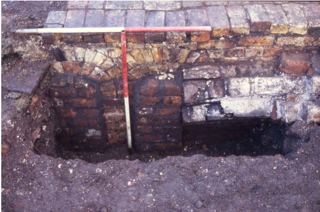
Plate 25: Facing site E. Showing the brick blocked access arches from the cellar located at the west of the Beta regenerative furnace.
