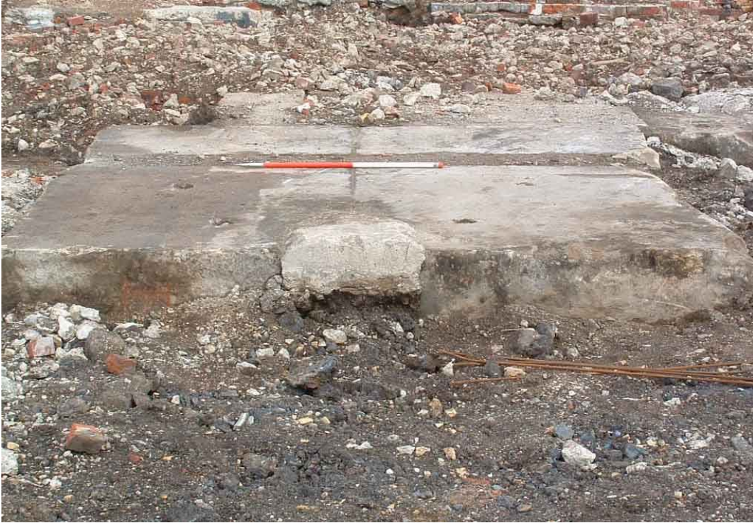
Plate 7: Facing site E. Showing the engine mounting 6105 with trapezoidal fixing bolts. Uncovered as part of strip and record Area 3, Trench B3 (behind) was backfilled for safety purposes.
