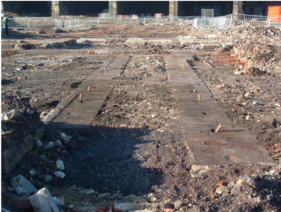
Plate 1: Facing site N, showing engine mounting [6099] exposed during the strip and record on Area 3. This mounting was located almost centrally within Building E1 and may well have had three separate machines above it. Note that the large crane base was located in the lower left corner and the open sided engine house from trench B3 was located just to the northeast of the scale.
