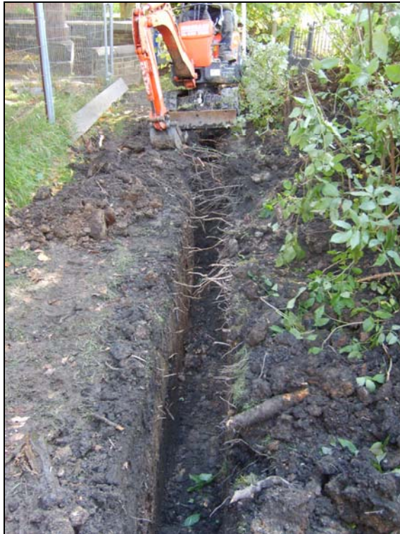
Plate 3 – Mechanical excavation of remainder of trench, south facing.
