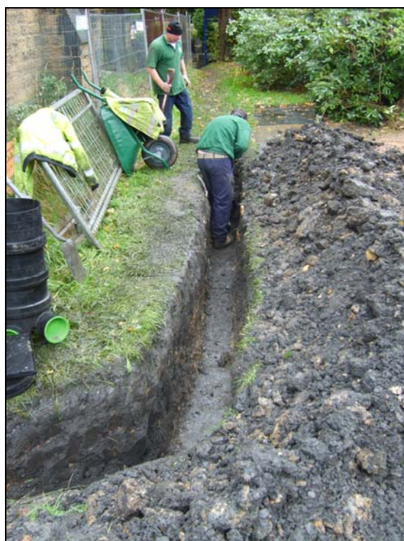
Plate 2 – Continued hand excavation of pipe trench, south facing.
