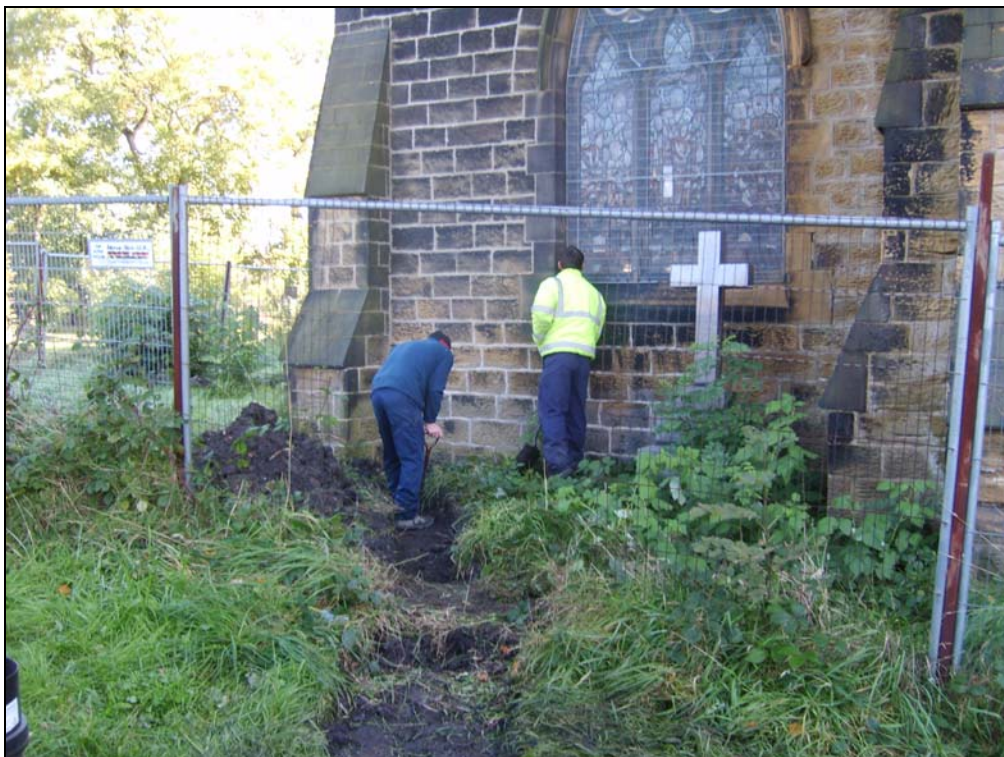
Plate 1 – Hand excavation of pipe trench, northeast facing.
