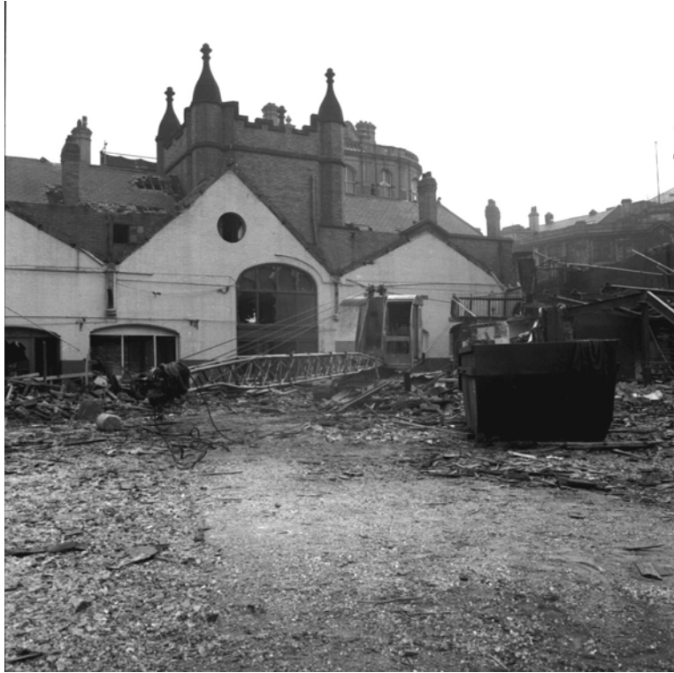
Plate 9 Photograph, facing east towards the Imperial Arcade, showing the interior demolition of the second, 1888, market Hall in 1971. (Courtesy of Rotherham Archives)
