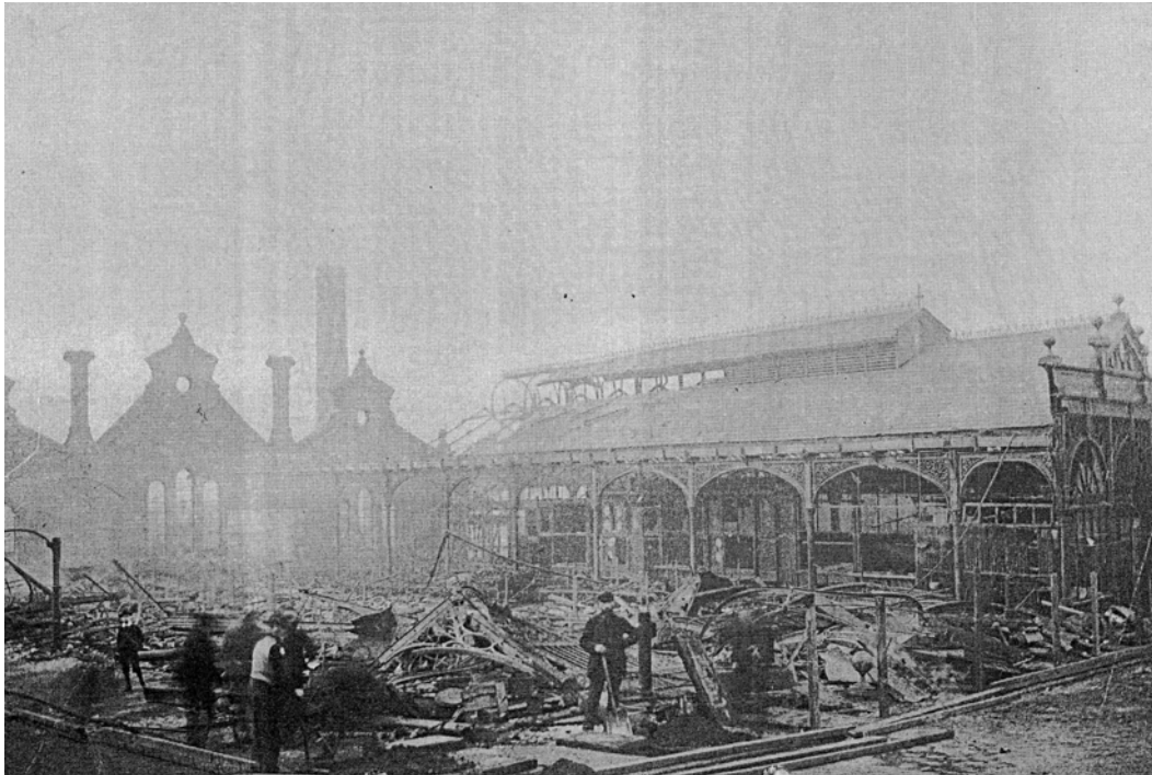
Plate 6: The first Market Hall after the fire of 1888. Note the surviving columns, possibly placed on the first phase brick pillars and the intact western façade (rear left). (Courtesy Rotherham Archives)
