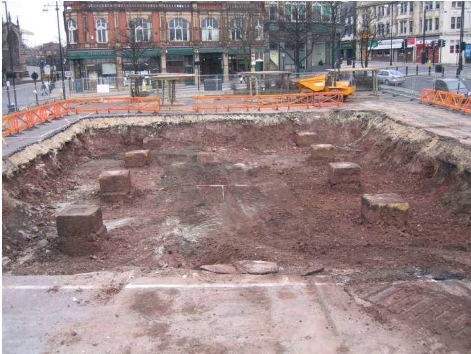
Plate 23: Facing E showing Trench 5 prior to the excavation of the L-shaped sondage. Note the sandstone blocks which would have probably supported the cast roof support columns. Note also the 'Imperial Buildings', built in 1907 to replace 'The Shambles' (top).
