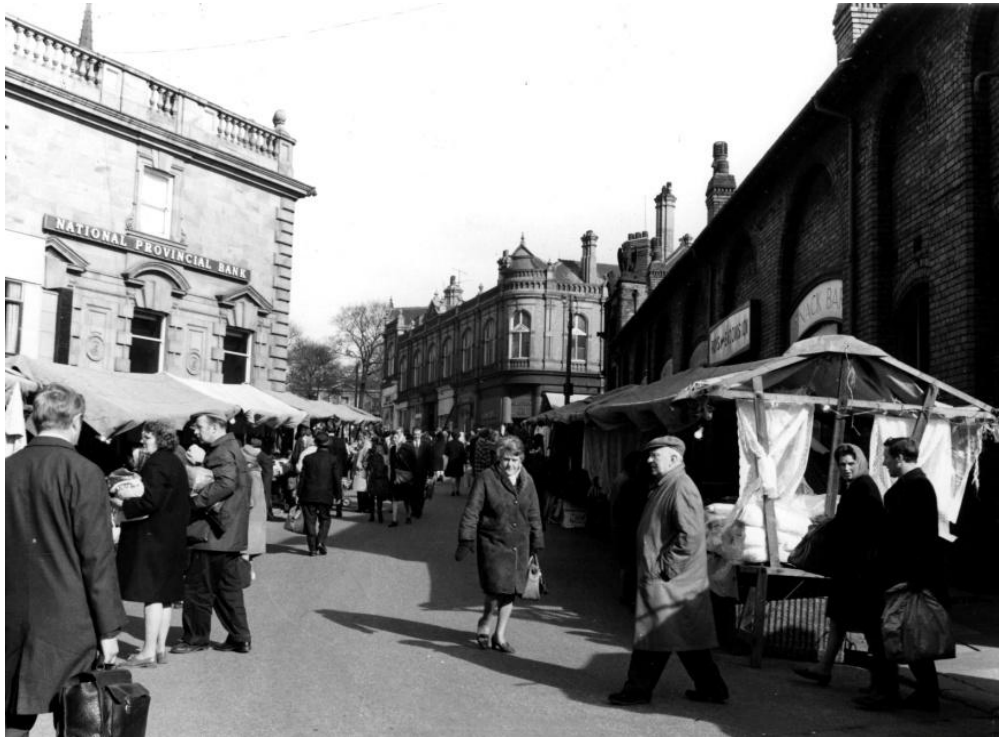
Plate 21: Historic archive photograph, facing ESE, showing the northern market wall (right) (RALSS, photo no. 02988). Note the brick arches that may have been supported on substantial brick pillars.
