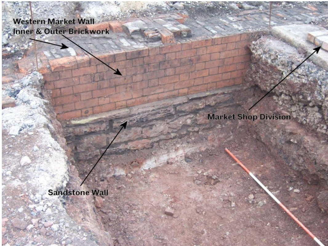
Plate 13: Facing WNW showing several features within the Trench 6 section.
