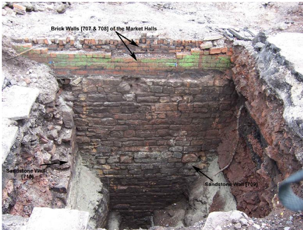
Plate 15: Facing E showing the western market hall wall [707, 708 and 709] with buttress [710] uncovered within Trench 7.
