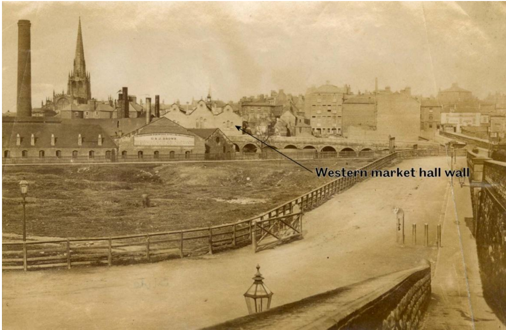
Plate 26: Historic archive etching, facing E, showing the first market hall (RALSS, photo no. 01324). Note that there is no large square turreted tower visible behind the western market hall walling.
