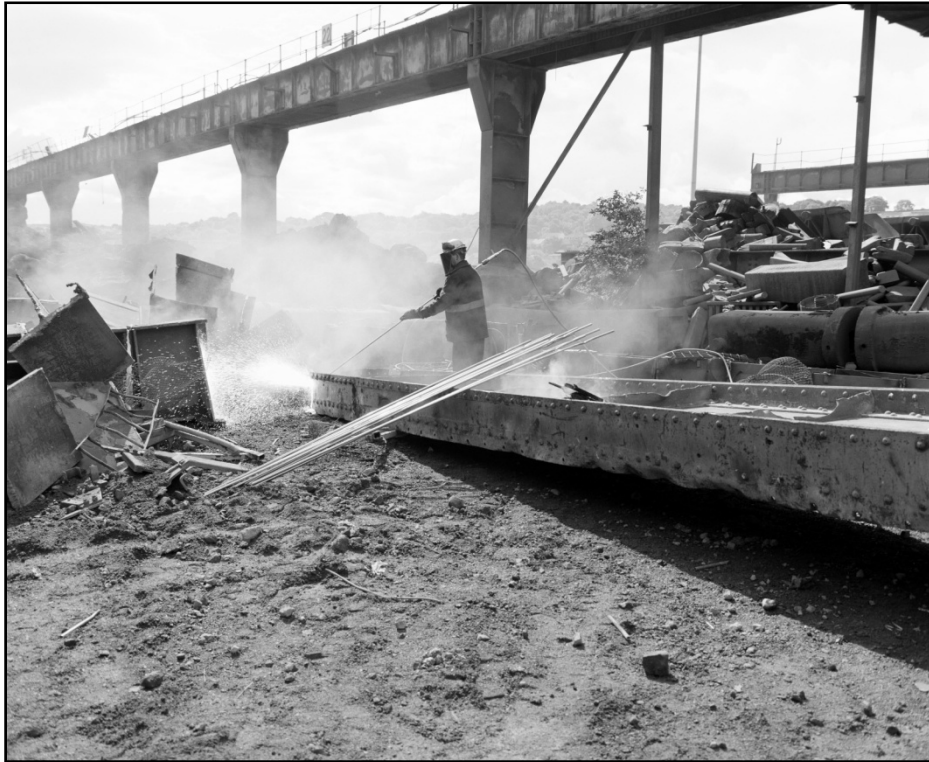
Plate 11: Cutting scrap with thermal lance (film 13:10)
