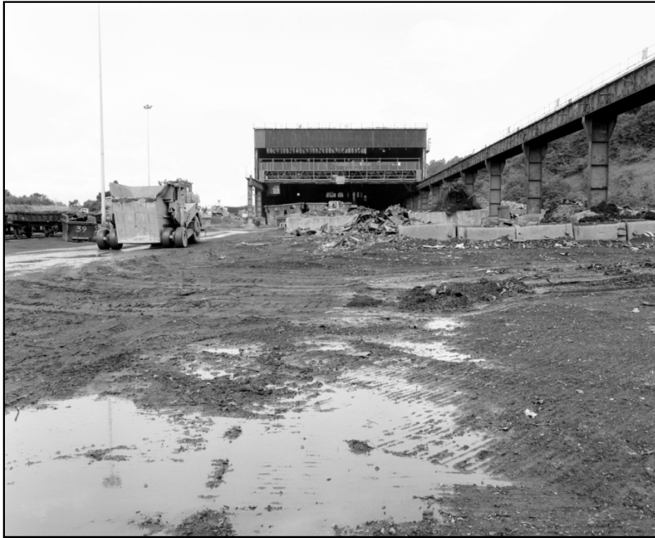
Plate 3: General view across A2, noting truncated gantries and Kress carrier (film 12:10)
