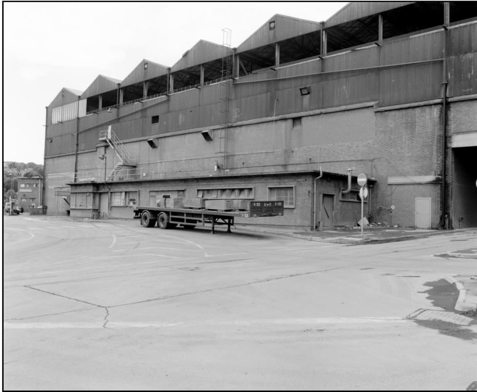
Plate 21: Detail of east elevation of building A1 (film 12:2)
