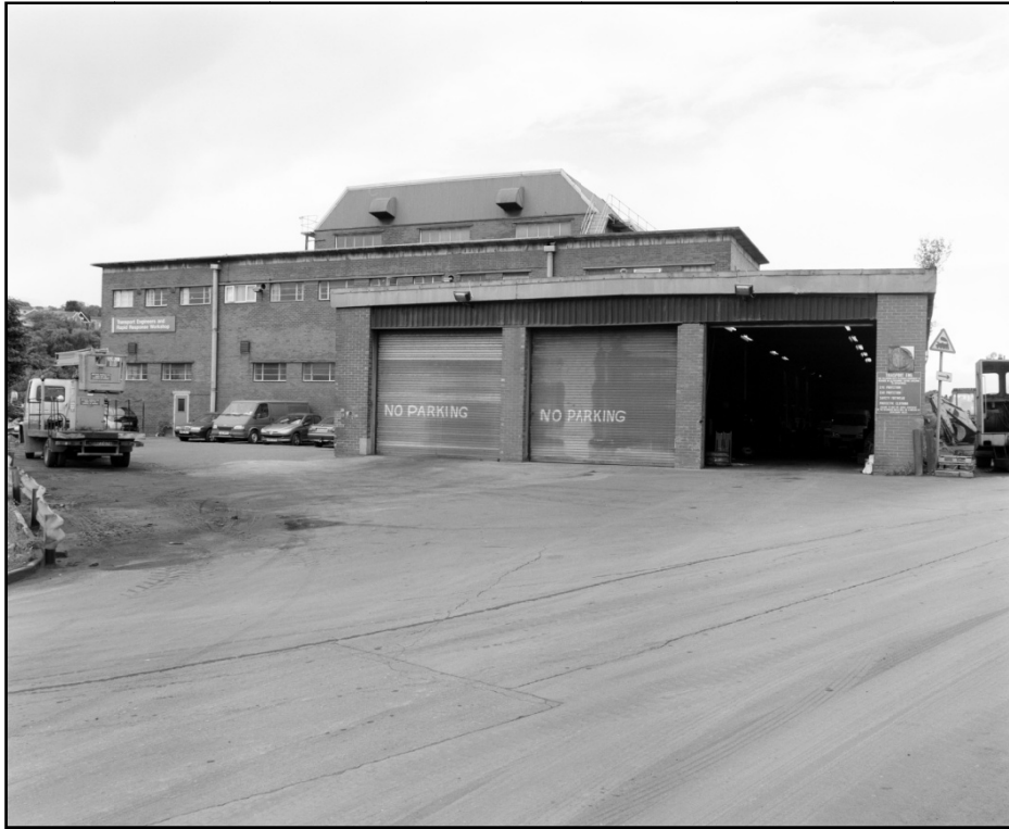
Plate 33: General view of west elevation of building A6 (film 15:9)
