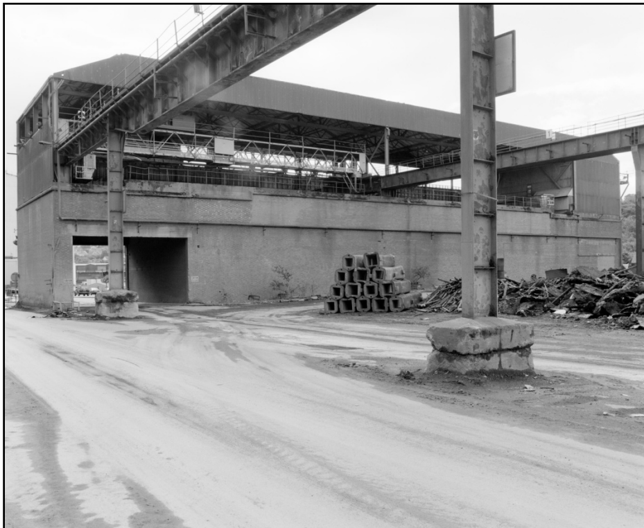
Plate 22: General view of west elevation of A1, noting travelling crane in first floor (film 12:3)
