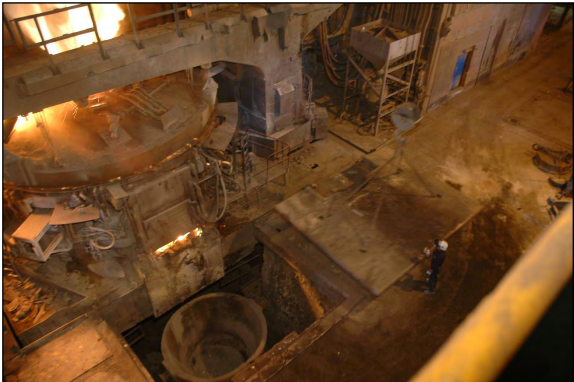
Plate 55: When in position the slagging pit cover plate is replaced then the slagging door is opened
