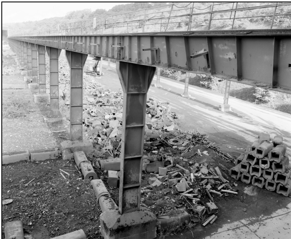
Plate 4: Detail of gantry across A2 (film 10:10)
