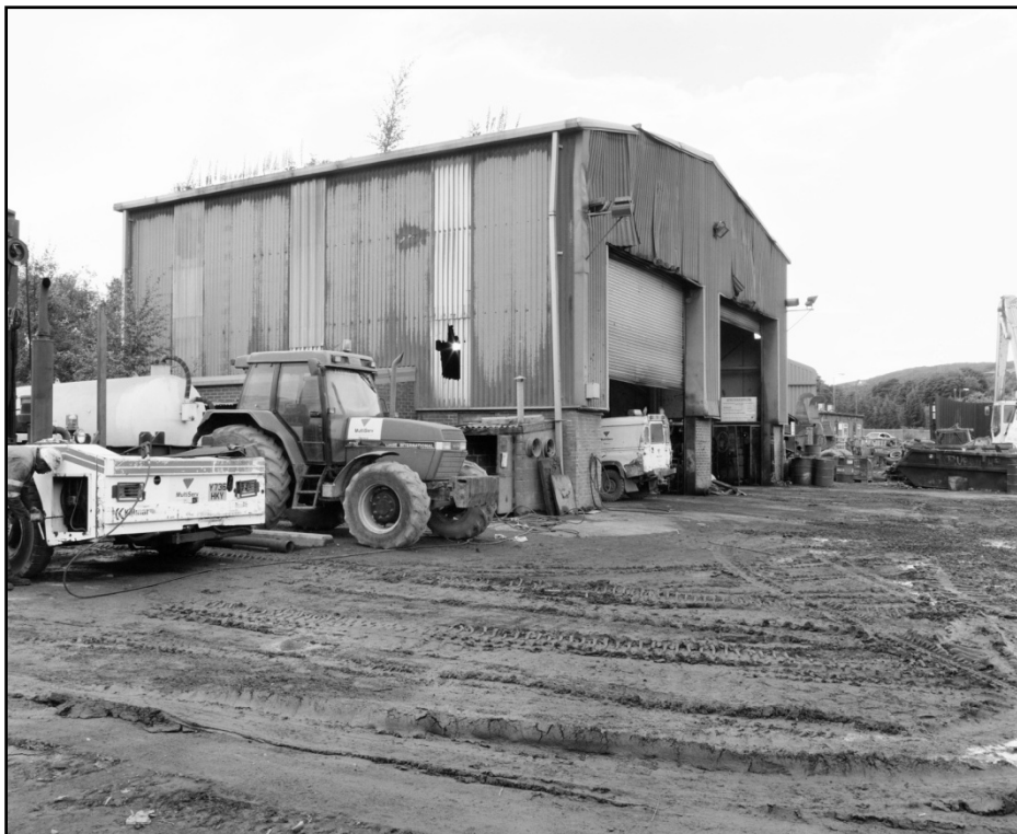
Plate 32: General view of Kress maintenance building A5 (film 15:2)
