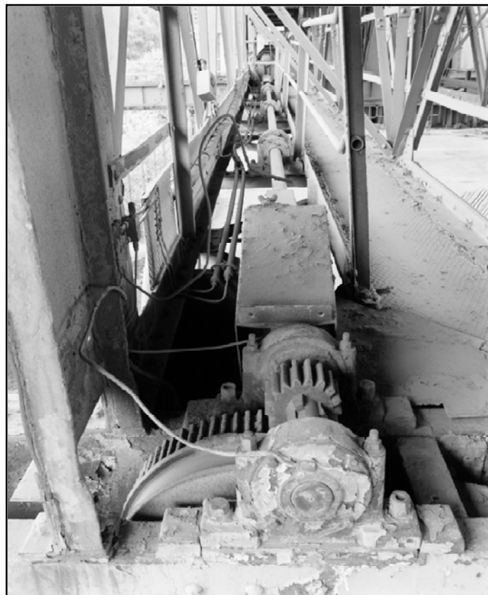
Plate 24: Detail along drive shaft of travelling crane (film 11:8)
