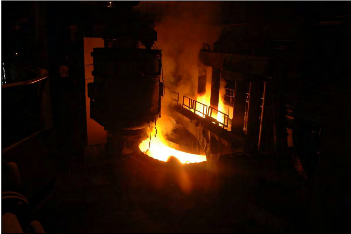
Plate 46: As the roof continues to open the charging basket is manoeuvred into position
