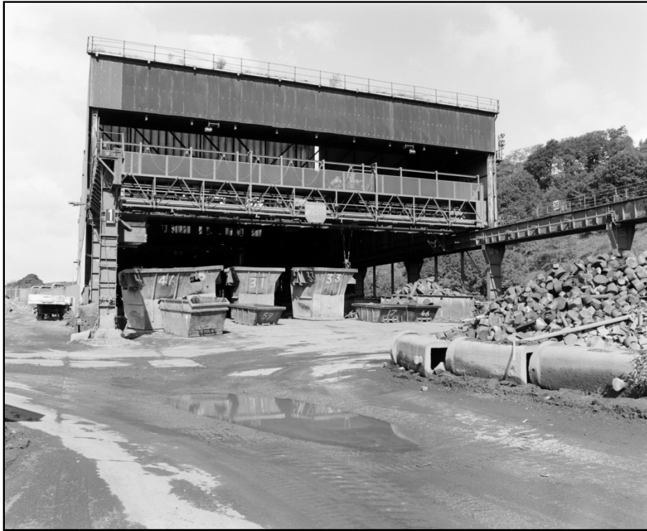
Plate 15: General view of southeast end of building A3 (film 13.8)
