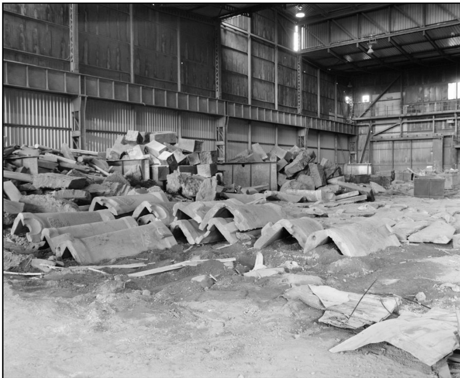
Plate 16: Interior of A3 looking west, noting ingot moulds for recycling (film 14:1)
