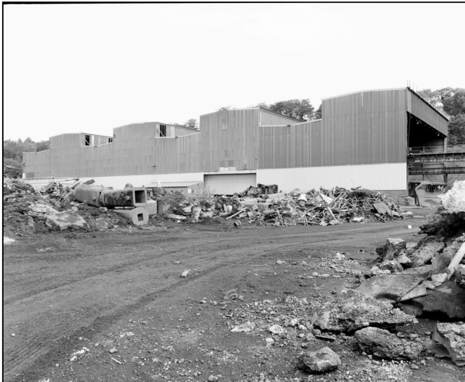
Plate 14: Southwest elevation of building A3 (film 13:3)
