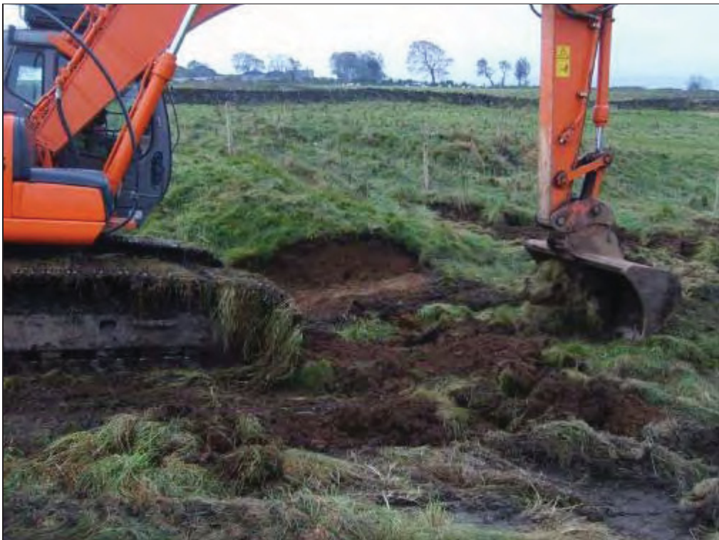
Plate 2 – Easement excavation in Field 2
