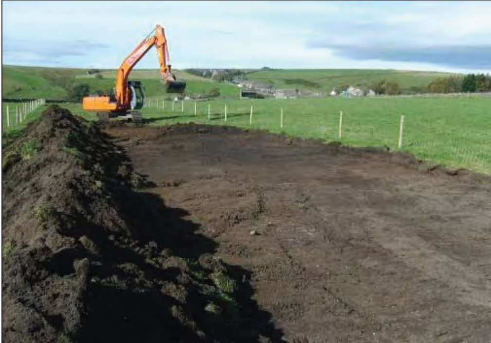
Plate 1 – Easement excavation in Field 1
