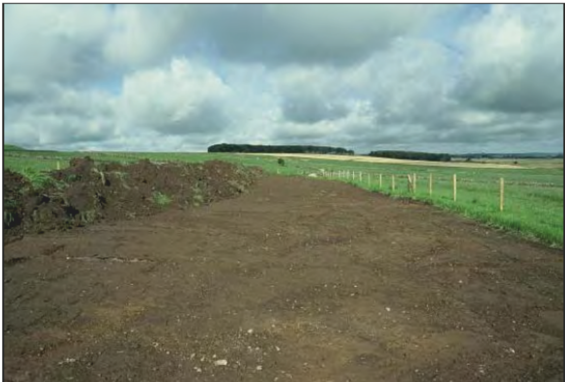
Plate 26: Excavated pipeline easement in field 2, viewed facing north-west.
