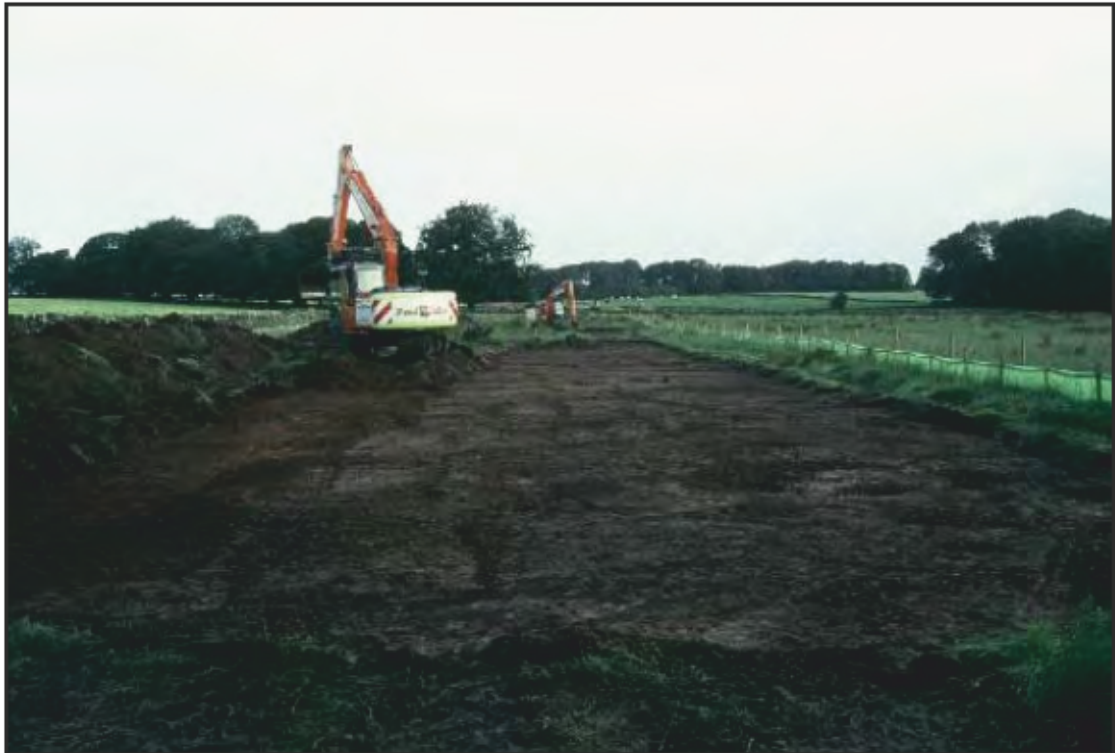
Plate 29: Working shot of easement excavation in field 5, viewed facing south.
