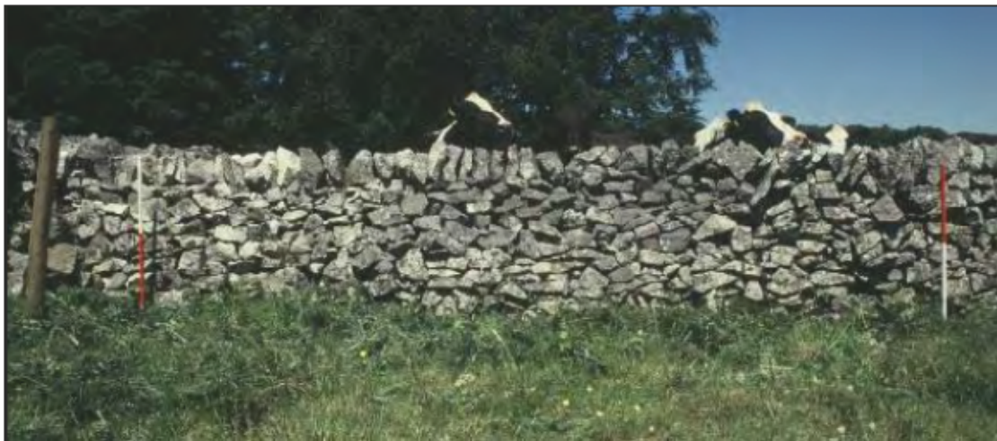
Plate 17: Field boundary 5, West end, viewed facing north.
