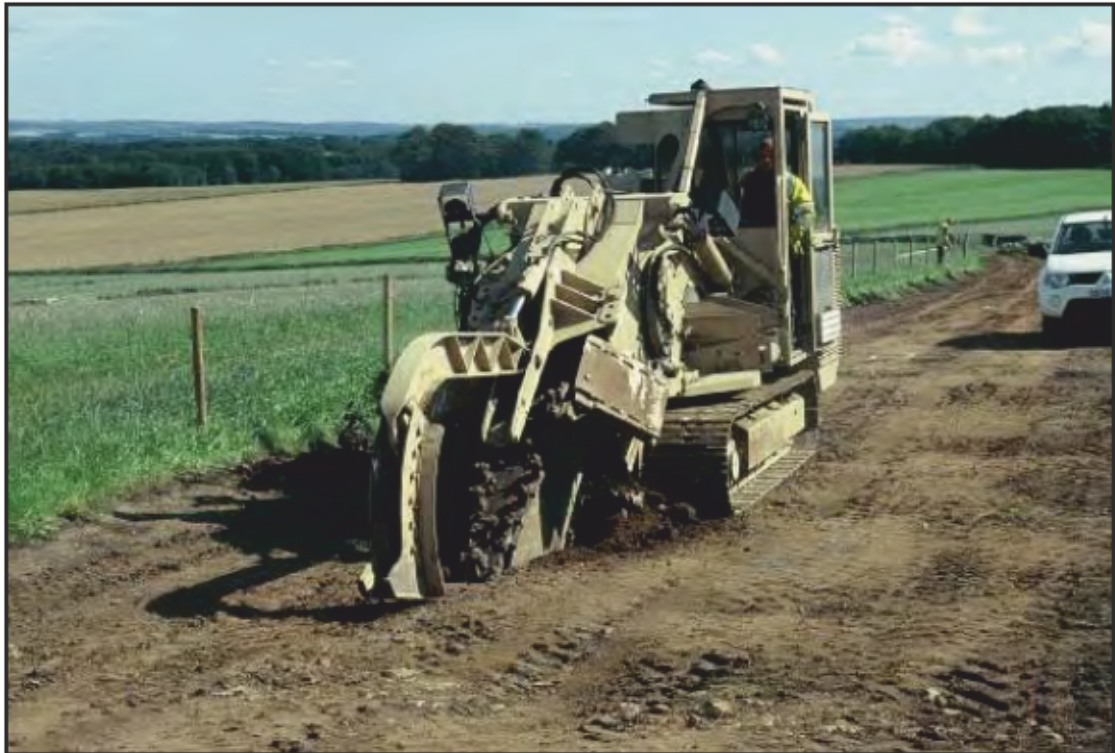
Plate 31: Commencement of pipeline excavation in field 1, viewed facing north-east.
