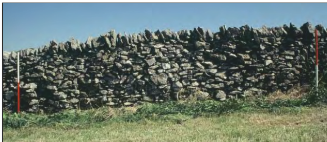
Plate 1: Field boundary 1, west end of photographed section, viewed facing southeast.
