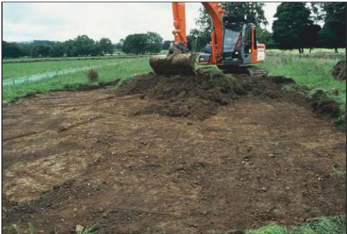
Plate 28: Working shot of easement excavation in field 4, viewed facing south.
