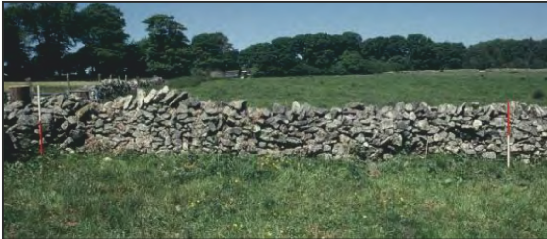
Plate 13: Field boundary 4, west end, viewed facing north.
