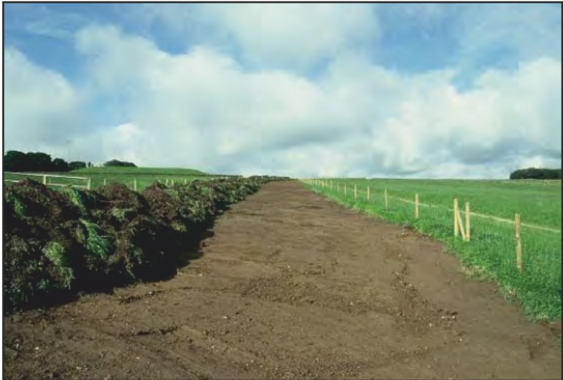
Plate 25: Northern end of pipeline easement, viewed facing north-west.
