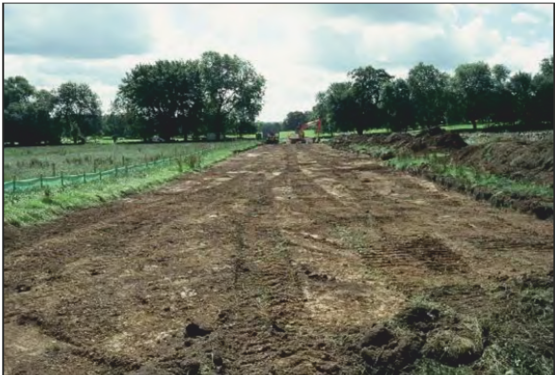
Plate 30: Working shot of easement excavation in field 6, viewed facing south.
