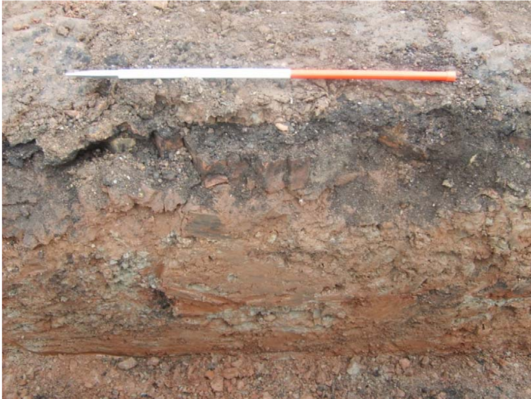
Plate 1: View of north facing section of foundation trench showing tarmac and red brick surface. Top layer is modern demolition material, deposited after the concrete raft was removed.
