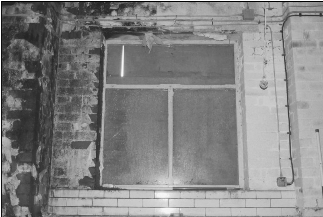
Plate 77: Detail of chamfered timber framed window in south wall of room 4 (film 10.32)
