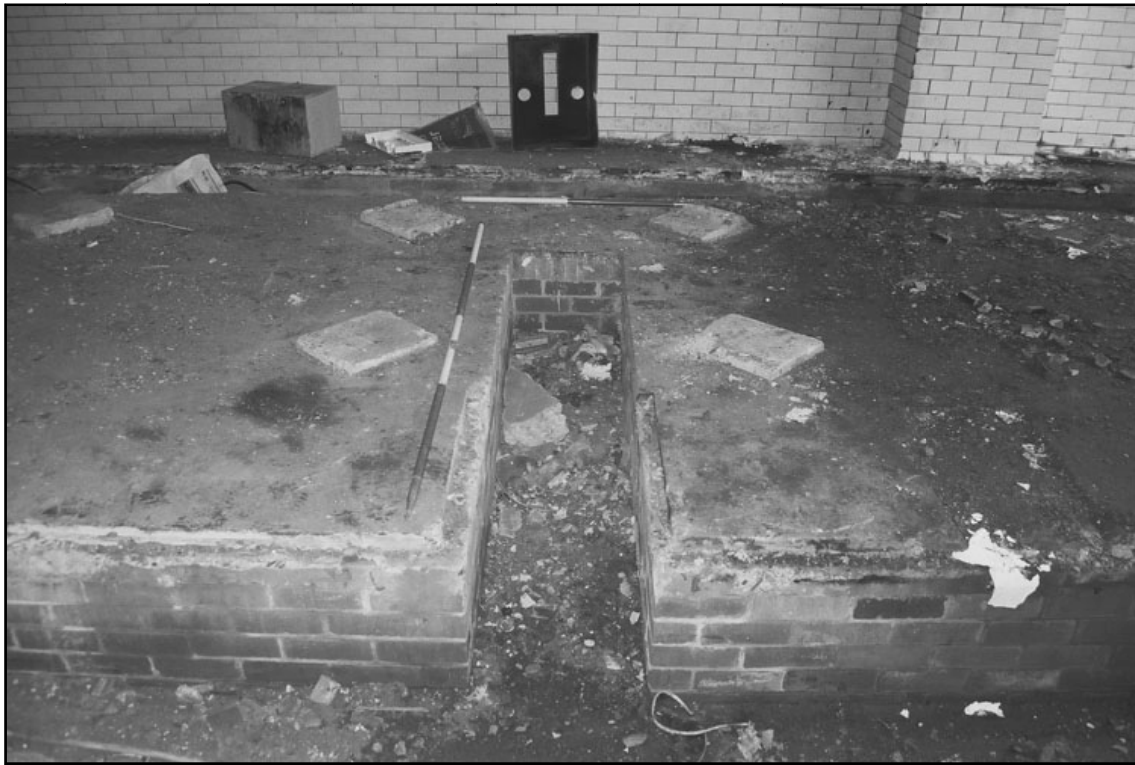
Plate 83: Detail of concrete pads around branch duct in room 4 (film 10.31)
