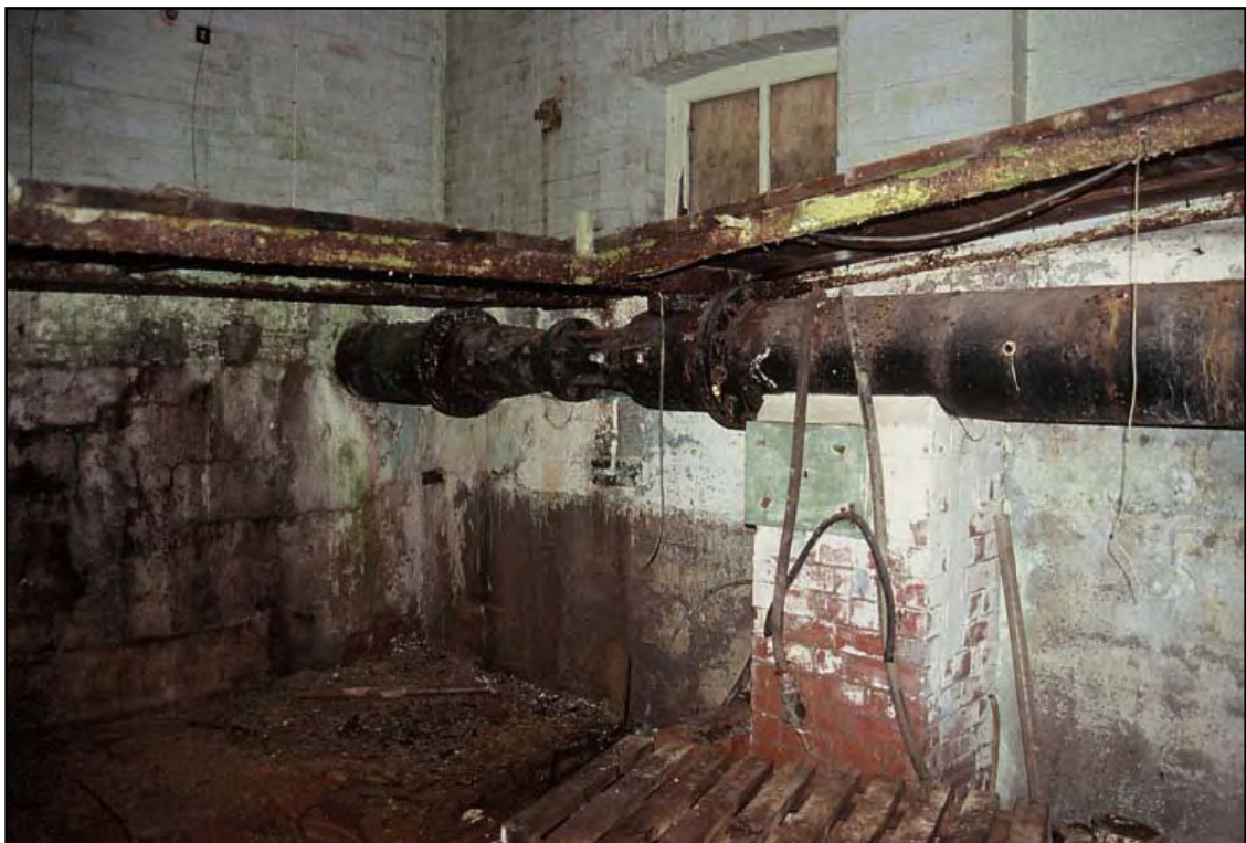
Plate 62: Detail of 8" water main in room 2, noting valve (slide 14)
