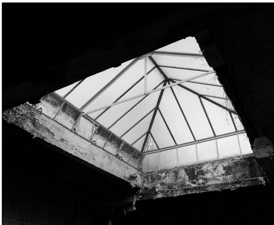
Plate 87: Detail of reinforced glass lantern skylight above room 4, looking northeast (film 9.05)
