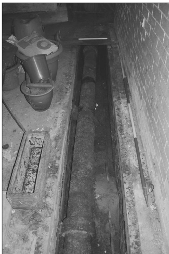
Plate 52: Detail of 8" water main inlet within floor of room 1 (film 6.32)
