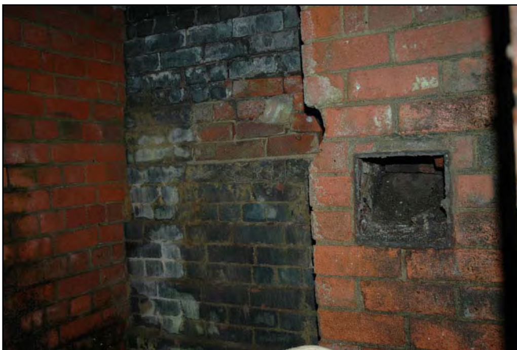
Plate 9: Detail of flue in southeast corner of generator chamber beneath yard
