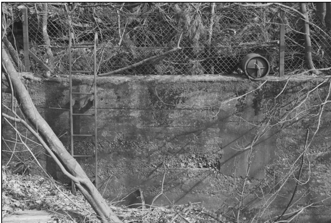
Plate 26: Detail of inlet pipe and ladder on east wall of south tank (film 1.23)
