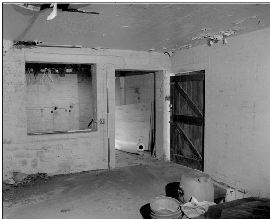
Plate 47: General view of room 1 looking west; note inserted doorway in stone faced wall (film 7.06)
