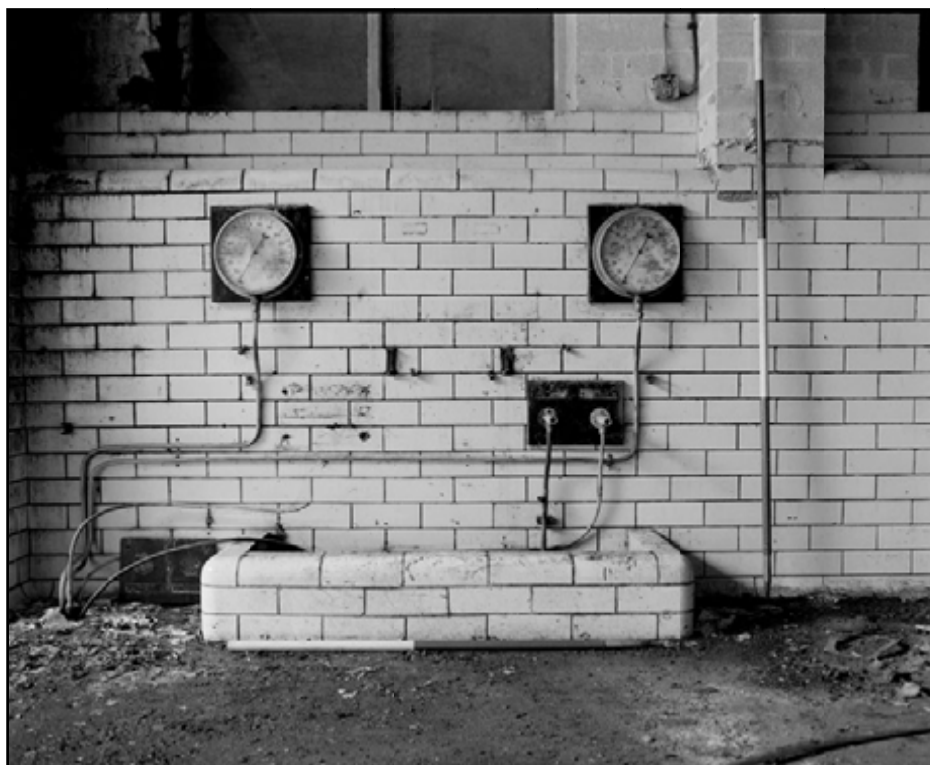
Plate 78: Detail of glazed brick floor basin against south wall of room 4 (film 9.03)
