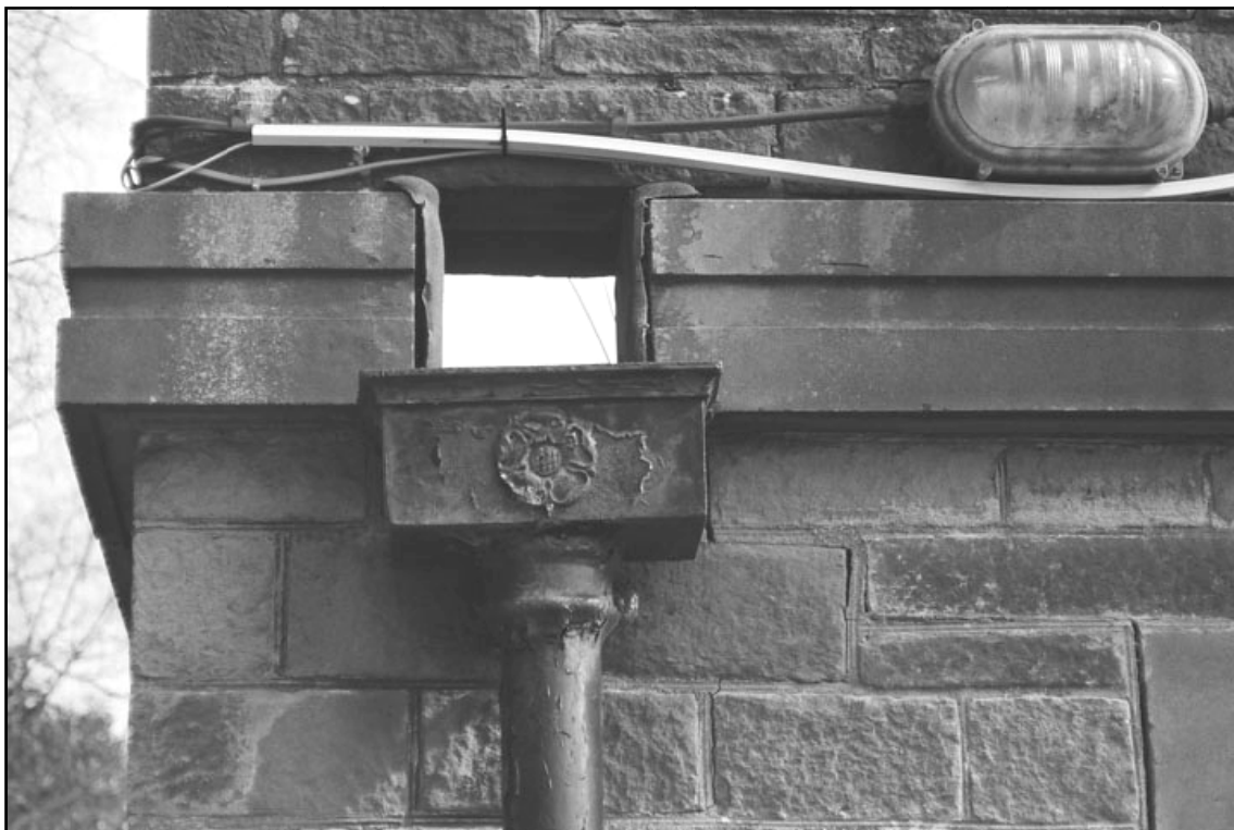
Plate 46: Detail of cast iron hopper on west elevation of filter house (film 1.30)
