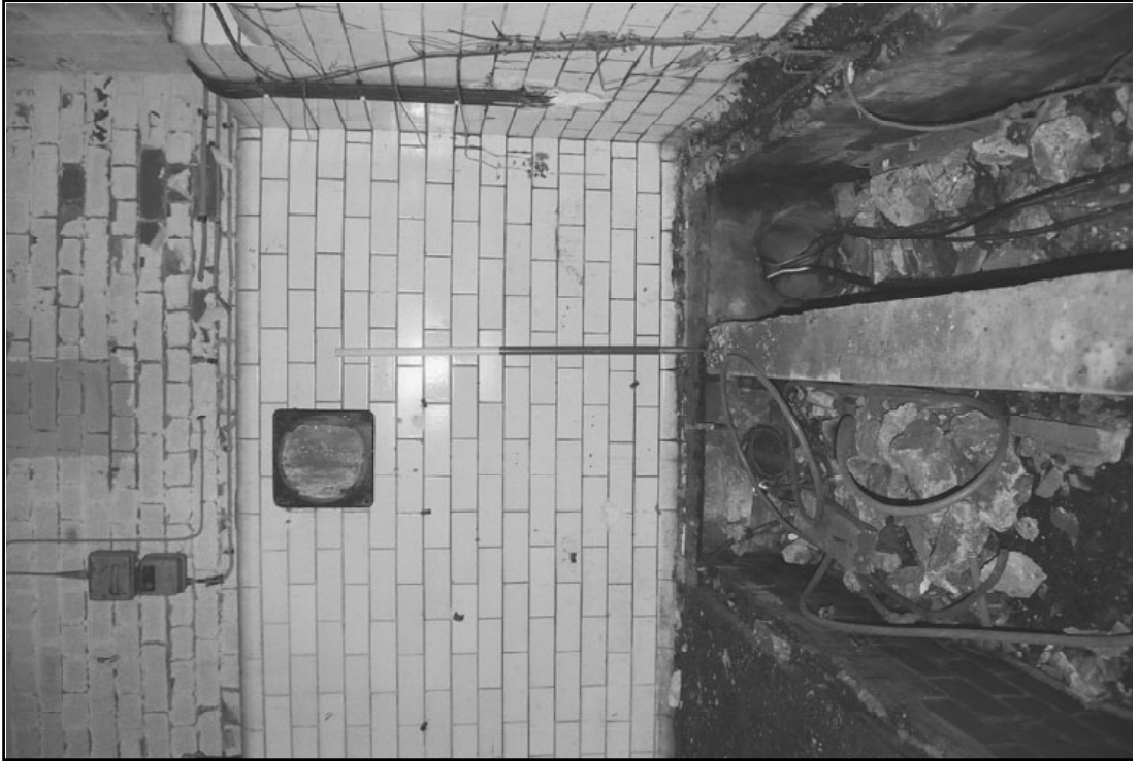
Plate 86: Detail of ducts and board for gauge against southern wall of room 4 (film 10.34)
