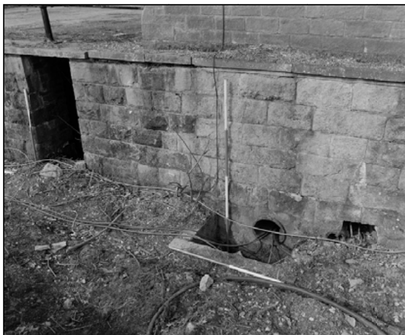
Plate 21: Detail of wash-out outlet from filter house; note entrance into generator chamber to left (film 5.09)
