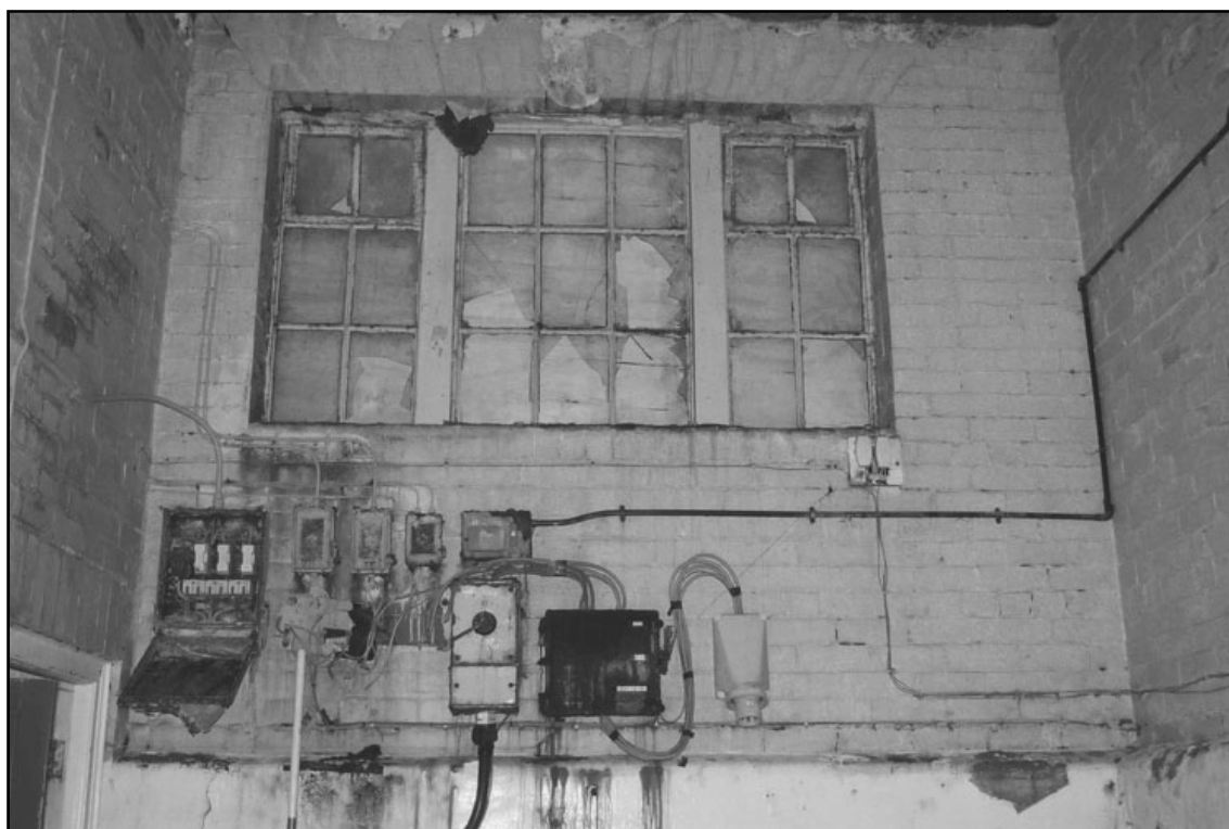
Plate 64: Detail of iron framed window and electrical junction boxes on east wall of room 3 (film 6.16)
