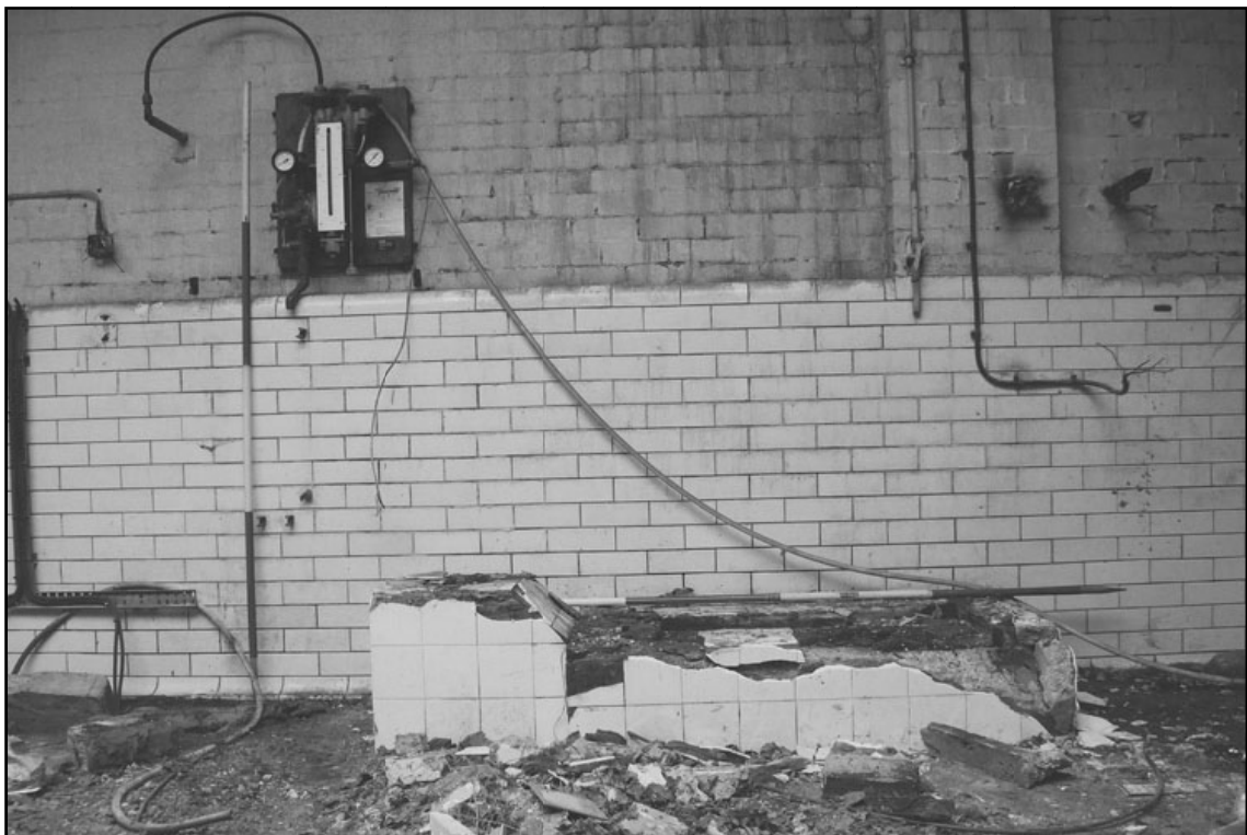
Plate 80: Detail of tiled concrete machine base against southern wall of room 4 (film 6.03)
