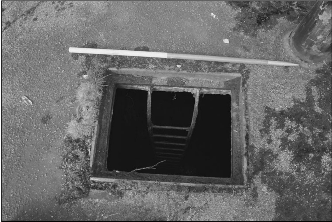
Plate 19: Detail of manhole with ladder into reservoir (film 1.07)
