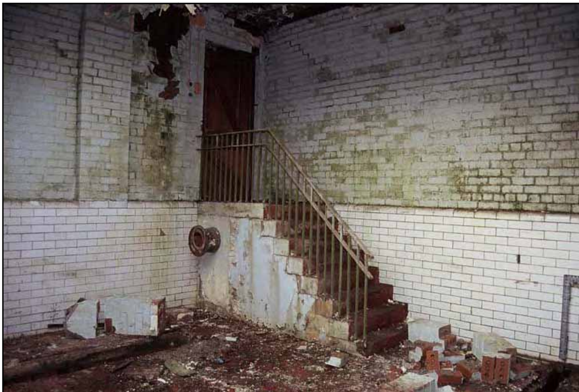
Plate 74: General view of staircase in northeast corner of room 4; note truncated 8" water main beneath (slide 3)
