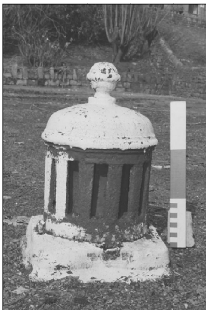
Plate 12: Detail of ornate cast iron vent above reservoir (film 1.16)
