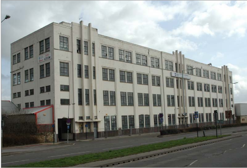
Plate 5 – Osborn Mushet Tools, street frontage structure probably built during the 1940s, on site of Morton Wheels dam. Looking north-east from Penistone Road.
