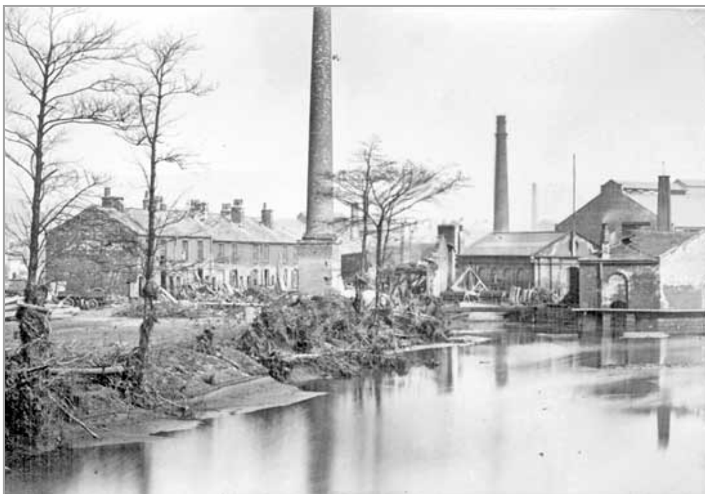
Plate 1 – Looking north-east towards mill dam, cottages, works chimney and part of Philadelphia Steel Works, following 1864 Sheffield Flood (Picture Sheffield y00945).
