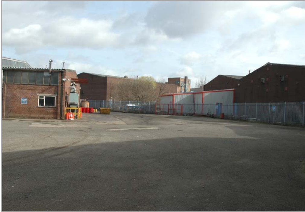
Plate 9 - Yard at east of site. Dam located from left to centre of yard, with sites of Morton Wheels and Philadelphia Works at right of yard. Site of large chimney in Plates 1 and 2 located within footprint of building at centre-left.
