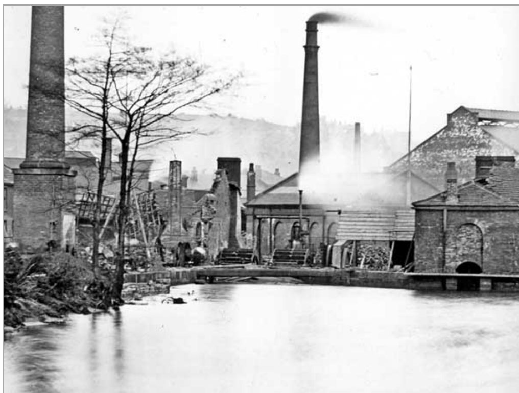
Plate 2 – North-east corner of dam following 1864 flood, showing sluice leading to two water wheels at centre. Remains of gable wall to left of wheels suggests wheelhouse destroyed during flood. North Wheel of post-medieval Morton Wheels located formerly in area of small building at right (Picture Sheffield w00450).
