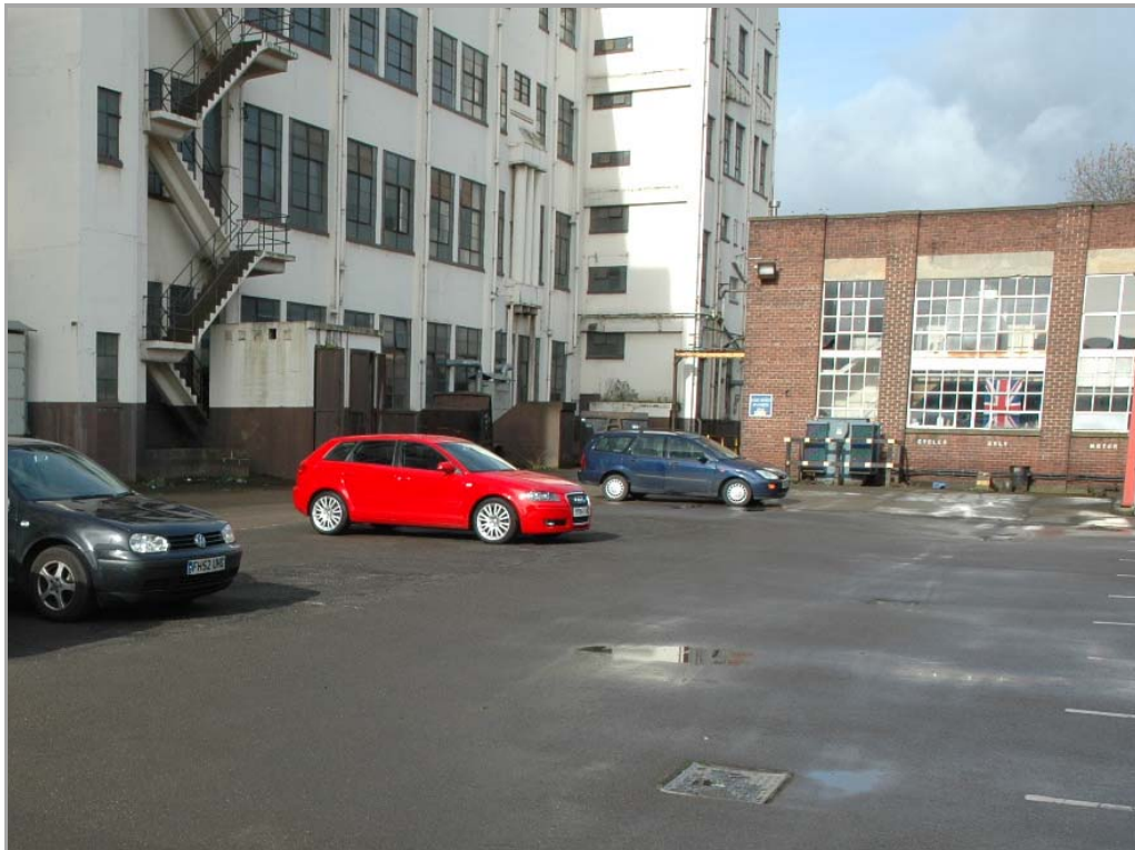
Plate 6 – Works yard to rear of Osborn Mushet Tools building, looking south-west. Mill dam located formerly in area occupied by Osborn building and yard, with goit running north-east through site of single-storey building at centre-right.
