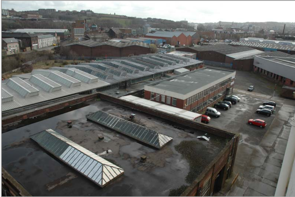
Plate 7 - Looking north-east from roof of Osborn Mushet Tools. 16 th -century Morton Wheels and 19 th -century Philadelphia Works stood in area at centre-right, with mill dam in yard at lower right. Buildings at left occupy site of goit.
