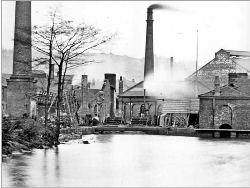
Plate 2 – North-east corner of dam, showing sluice leading to two water wheels at centre. Remains of gable wall to left of wheels suggests wheelhouse destroyed during flood. North Wheel of post-medieval Morton Wheels located formerly in area of small building at right (Picture Sheffield w00450).
