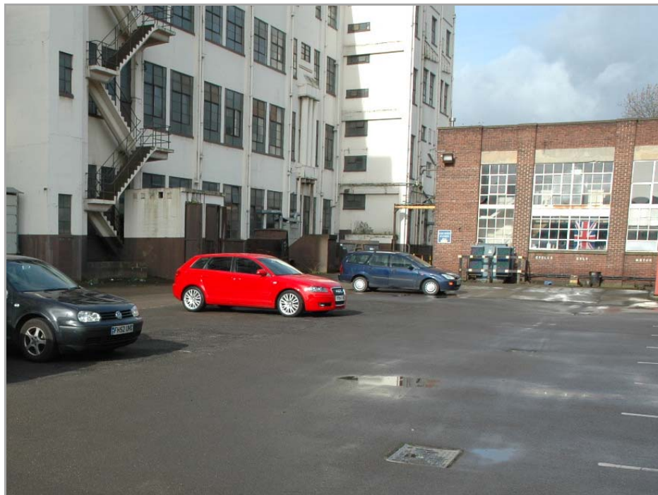
Plate 6 – Works yard to rear of Osborn Mushet Tools building, looking south-west. Mill dam located formerly in area occupied by Osborn building and yard, with goit running north-east through site of single-storey building at centre-right.
