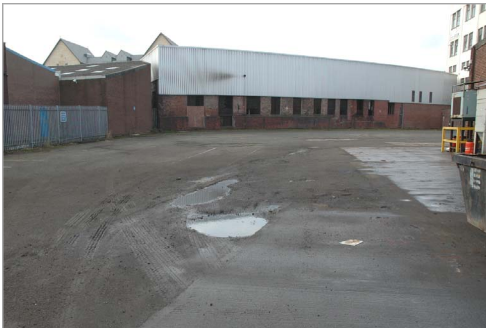
Plate 8 - Yard at east of site. Mill dam wall and tail goit located formerly in area towards centre of shot. Morton Wheels located formerly in upper part of yard, with Philadelphia Works situated in foreground.
