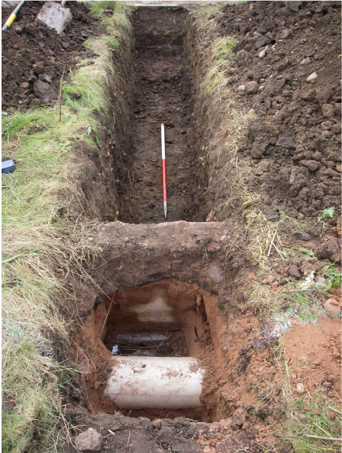
Plate 1 – Area 2. Trial hole 4A; looking east
