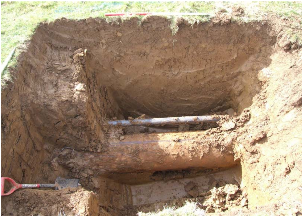
Plate 2 – Trial pit 4 – looking south
