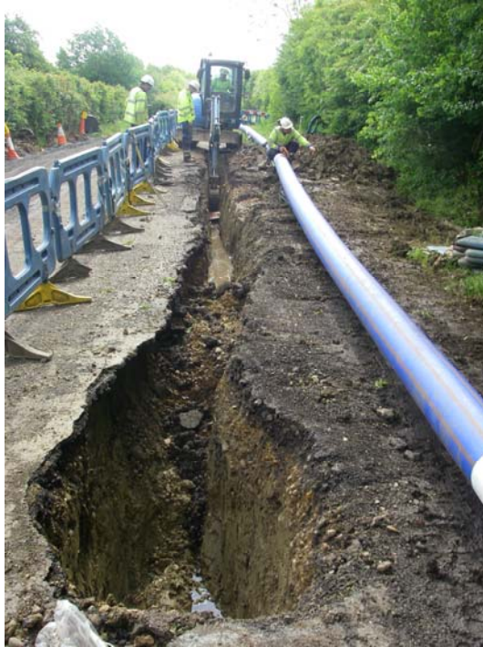
Plate 1 – View of Trench B looking east
