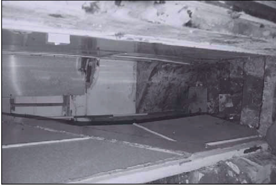
Plate 14: General view of cellar steps from G3 (film 7.9)
