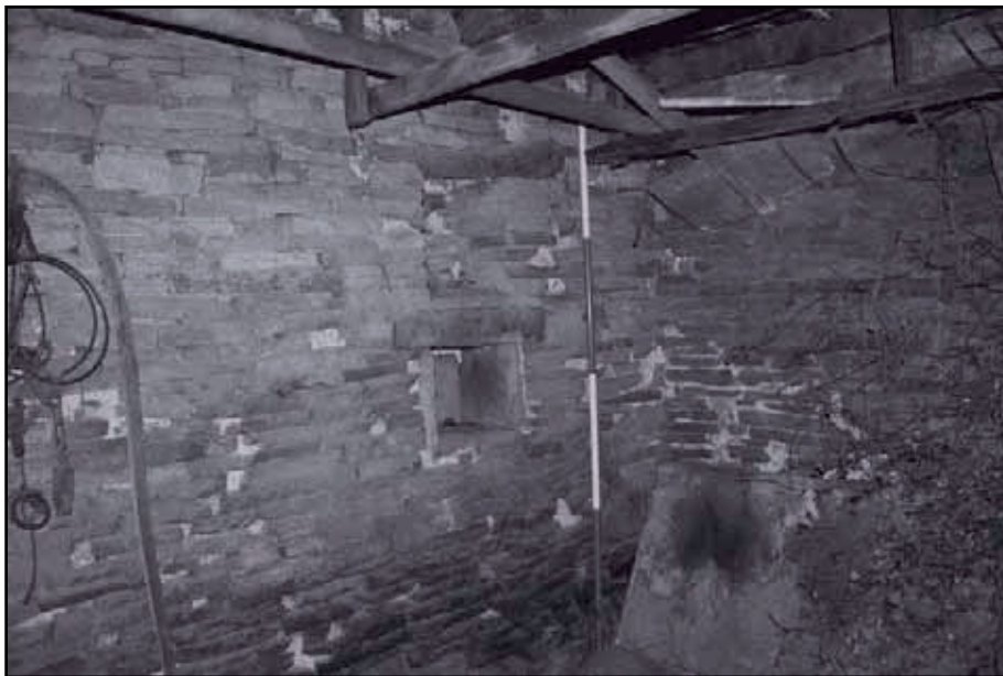
Plate 56: General view of G11, noting 'keeping holes' (film 1.09)
