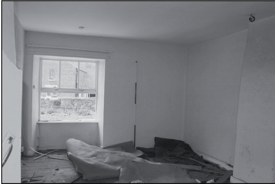
Plate 39: General view of F10, looking northwest (film 6.28)
