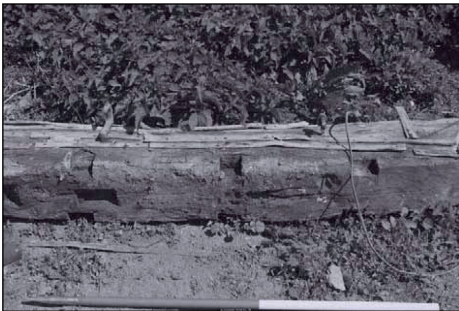
Plate 62: Detail of cogging for ceiling joists, disused mortise and iron hooks on tie beam from East Range (film 8.14)
