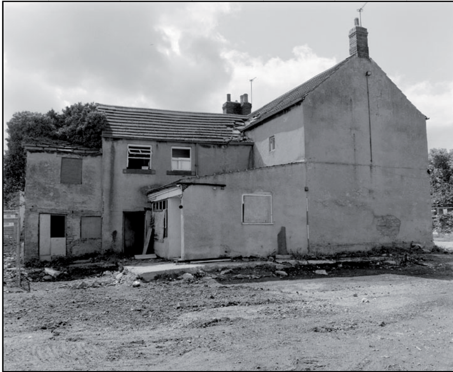
Plate 25: General view of north elevations of Thorpefield farm (film 3.6)
