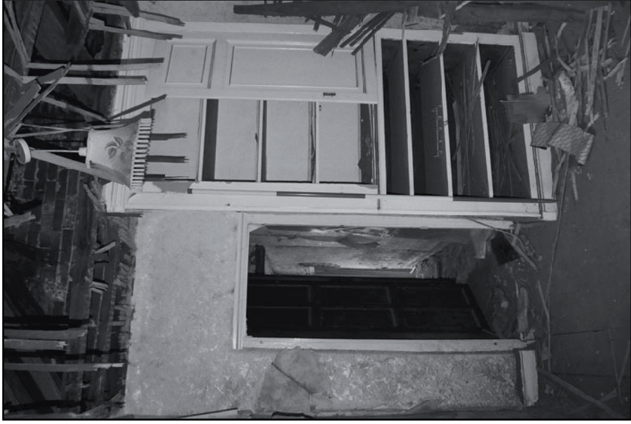
Plate 36: General view of F6, looking southwest (film 6.1)
