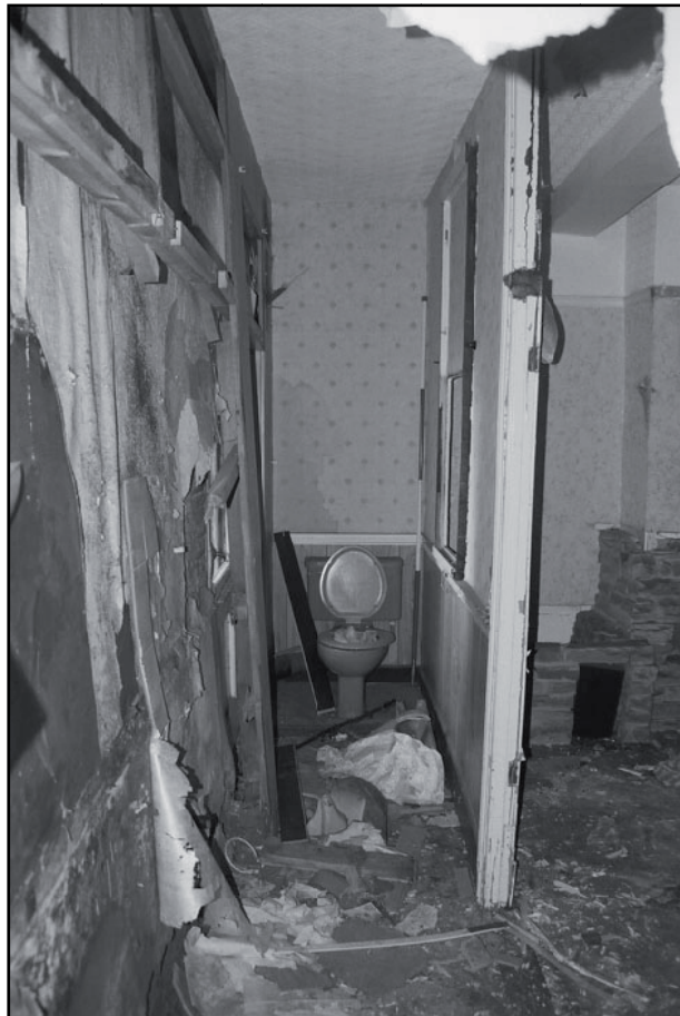
Plate 28: General view of partitioned WC in southeast of G5 (film 5.10)
