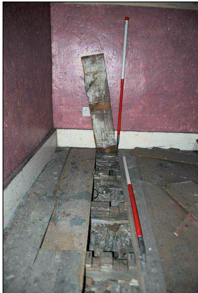
Plate 20: Detail of whitewashed reverse of floor board in F4 (slide 10)
