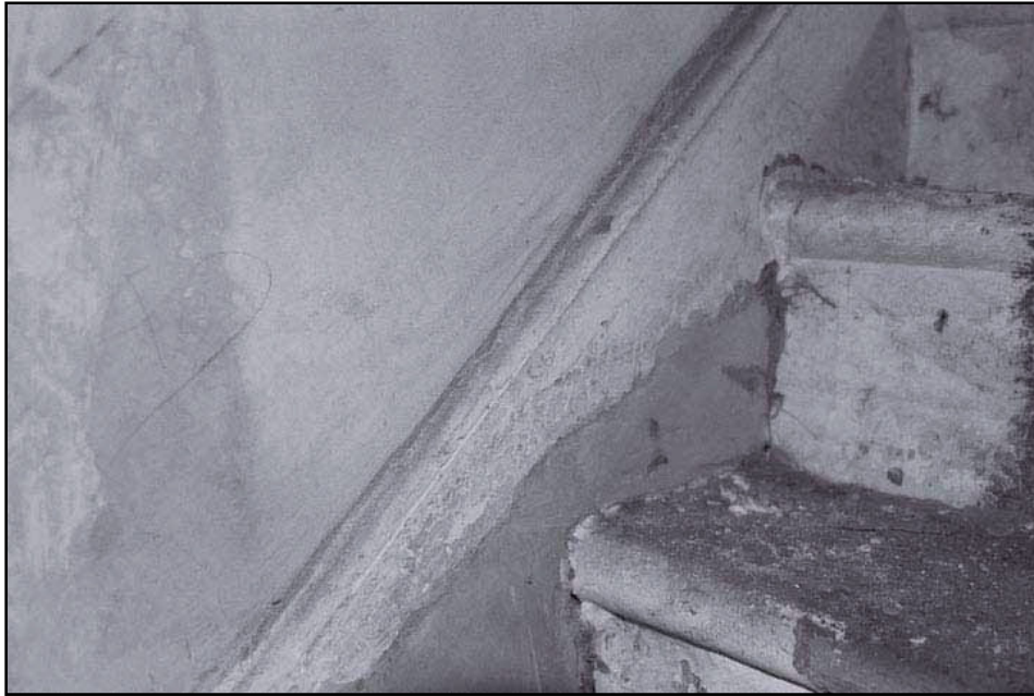
Plate 15: Detail of stone staircase (film 7.21)
