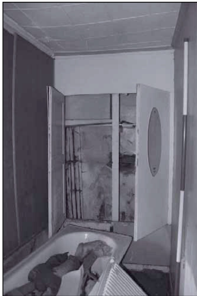
Plate 18: General view of F1, looking north (film 7.29)
