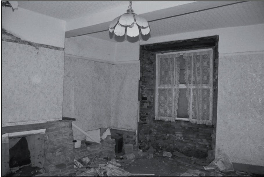
Plate 27: General view of room G5 (film 5.08)
