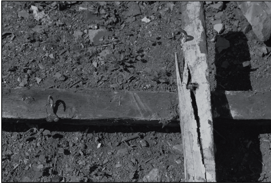
Plate 49: Detail of timber beam built into east elevation of east range with wrought iron hooks (film 8.28)
