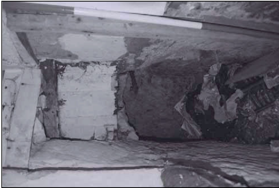
Plate 7: General view of vaulted access to cellar (film 7.7)
