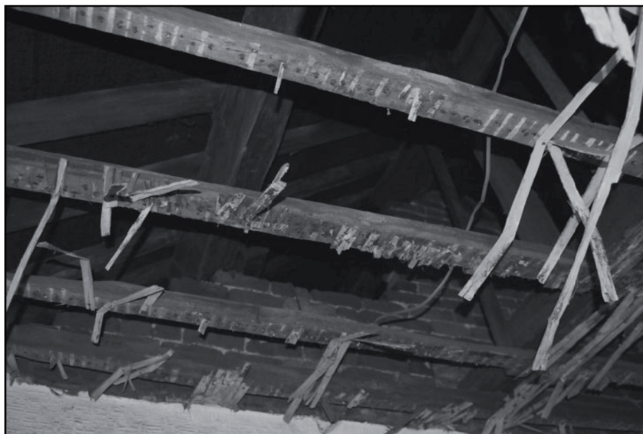
Plate 38: Detail of north wall of F5 noting lathe and plaster ceiling and piers supporting roof purlins (film 6.06)
