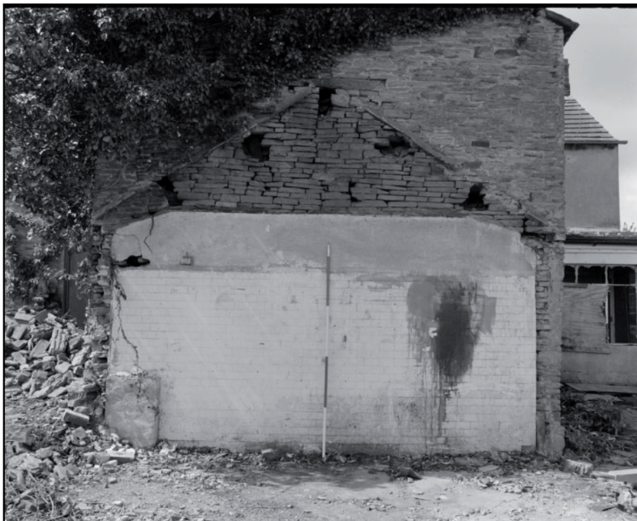
Plate 48: Detail of east elevation of East Range, noting scars from removed extension (film 4.5)
