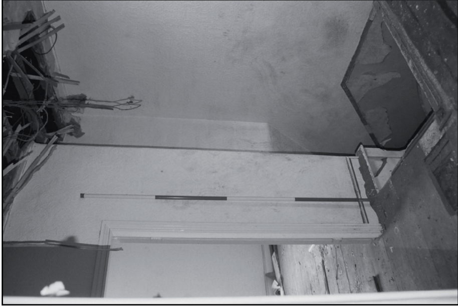
Plate 42: General view of F9, looking northwest (film 6.26)
