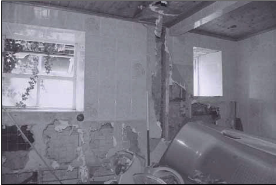
Plate 57: General view of F12, looking southwest (film 6.16)
