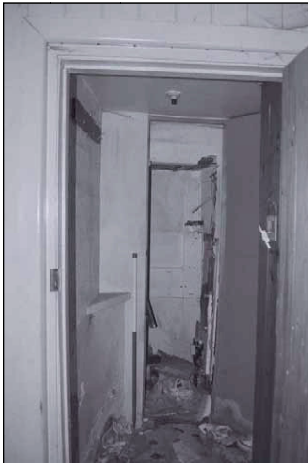
Plate 12: General view of G2 from G1 looking east (film 7.11)
