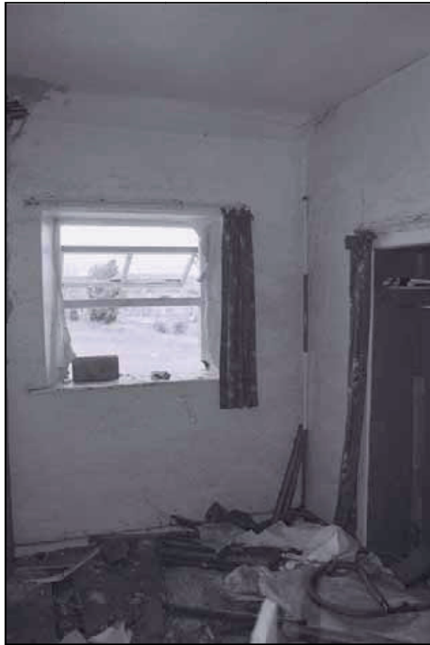
Plate 59: General view of F14 looking north (film 6.12)
