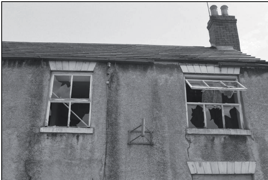
Plate 24: Detail of windows on west elevation (film 1.24)
