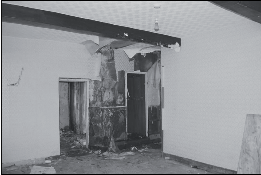
Plate 31: General view of G10, looking southeast (film 5.17)
