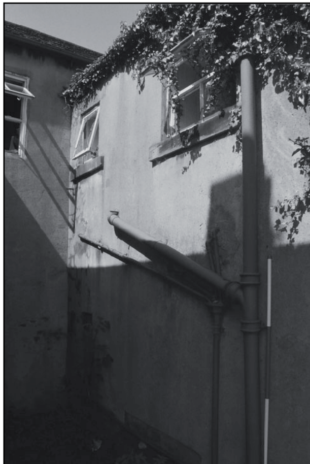
Plate 50: General view of south elevation of east range (film 1.12)
