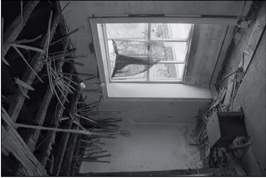
Plate 35: General view of F5, looking southwest (film 6.8)
