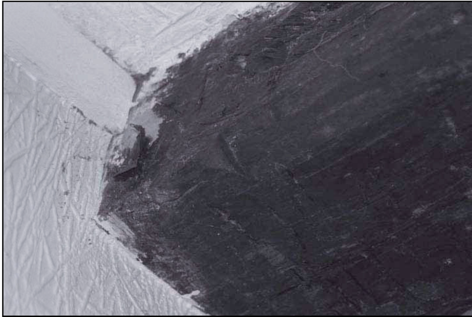
Plate 11: Detail of lambs-tongue stop on ceiling joist in G4 (film 7.16)
