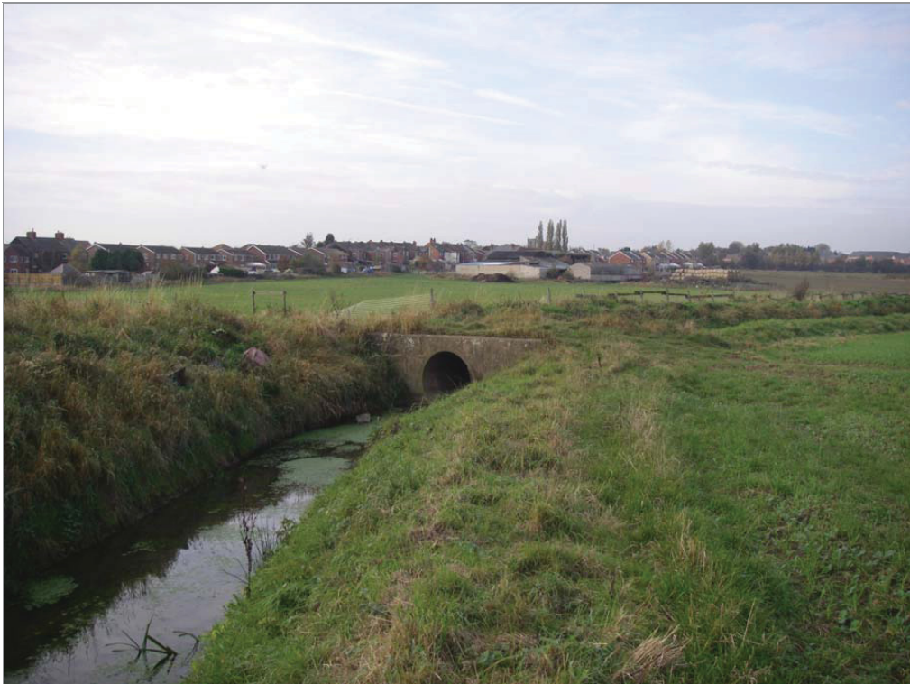
Plate 5 – View west along Crane Well Dike showing concrete bridge
