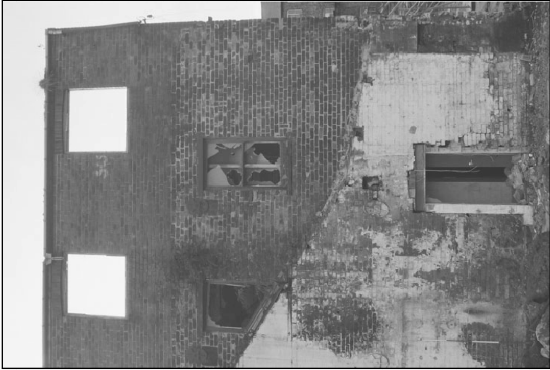
Plate 20: Detail of north elevation of grinding workshop (film 9.34)
