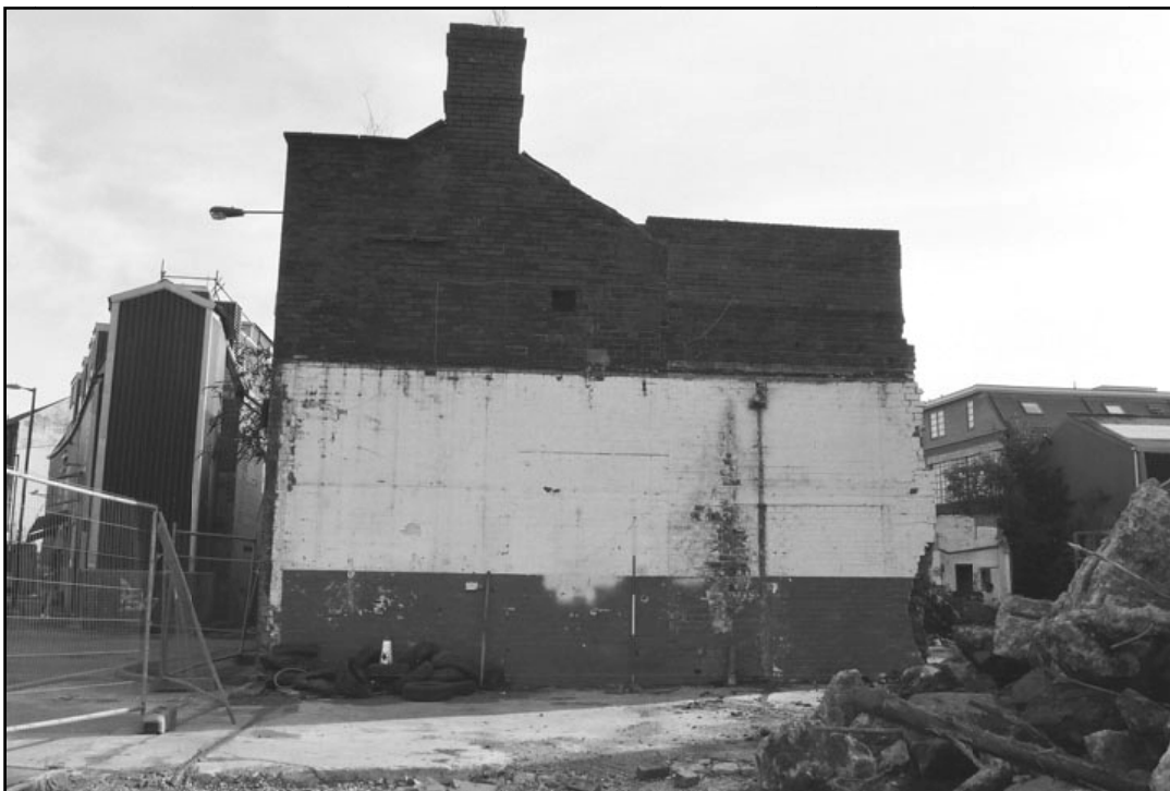
Plate 6: General view of west elevation of office building (film 9.04)
