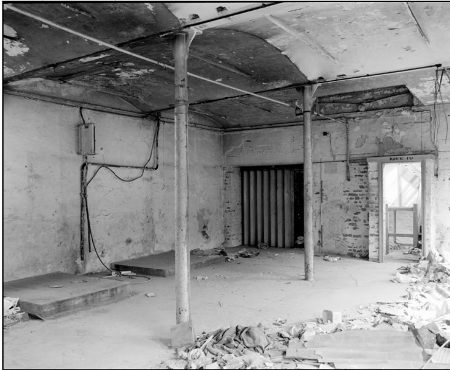
Plate 35: General view of room 2F1, noting concrete machine bases and eastern entrances (film 6.09)
