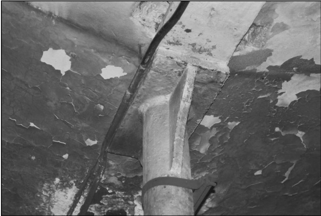
Plate 37: Detail of head of cast iron column supporting brick jack-arches (film 1.28)
