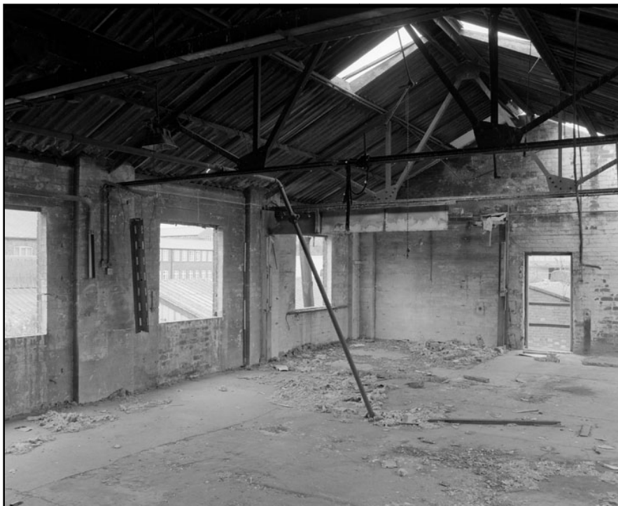
Plate 40: General view of room 2S1, noting angle-iron fink truss (film 7.05)
