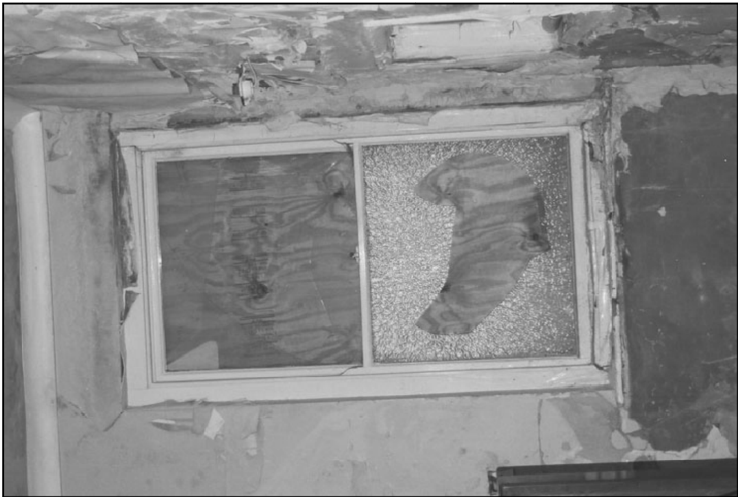
Plate 9: Detail of timber sash framed window in room 1G2 (film 1.18)
