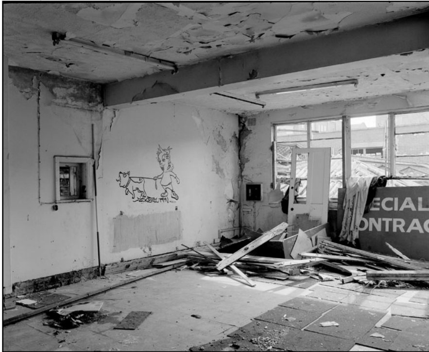
Plate 13: General view of southeast corner of room 1F2 (film 4.03)
