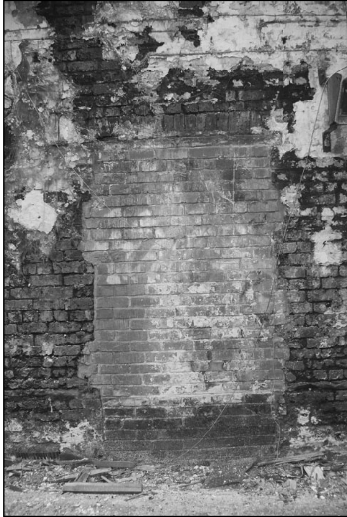
Plate 28: Detail of blocked door inserted through former window (film 1.32)
