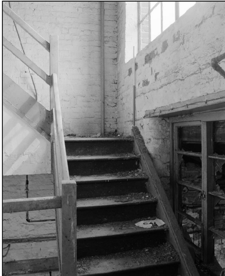
Plate 41: General view of staircase in southern half of stair-tower (film 6.05)
