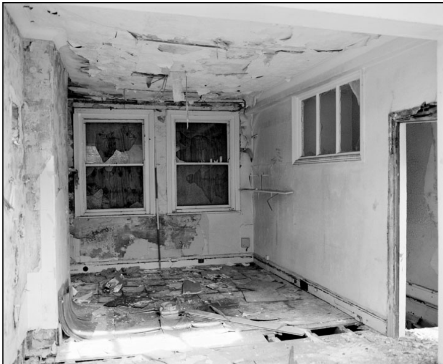
Plate 12: General view of northwest end of room 1F2 (film 3.07)
