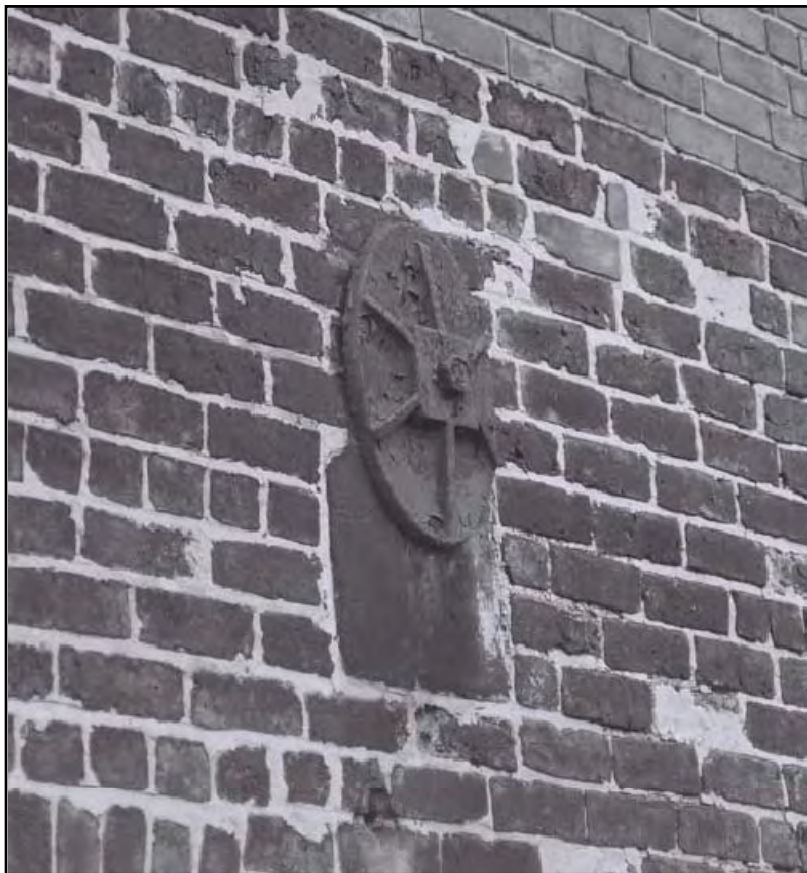
Plate 31: Detail of tie-plate on southern elevation of grinding workshop (film 1.25)
