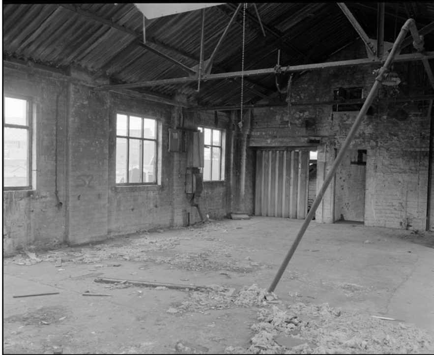
Plate 39: General view of room 2S1 (film 7.07)
