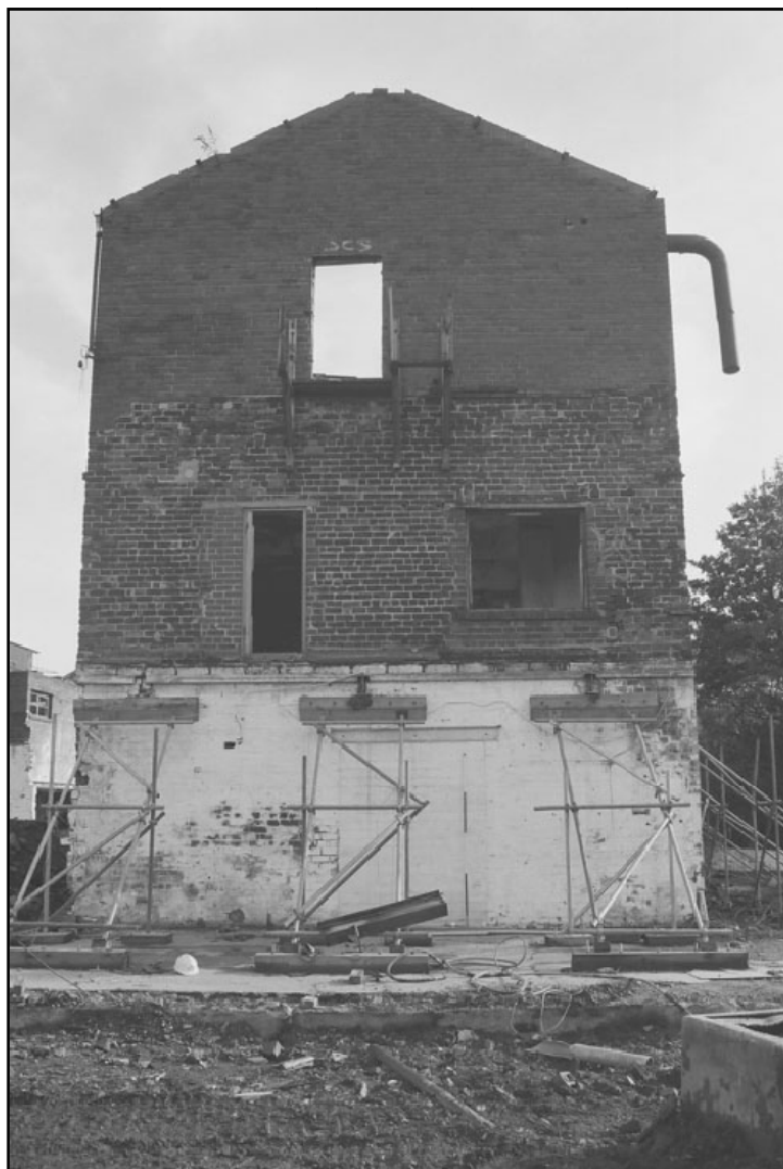
Plate 24: General view of western elevation of grinding workshop (film 9.14)
