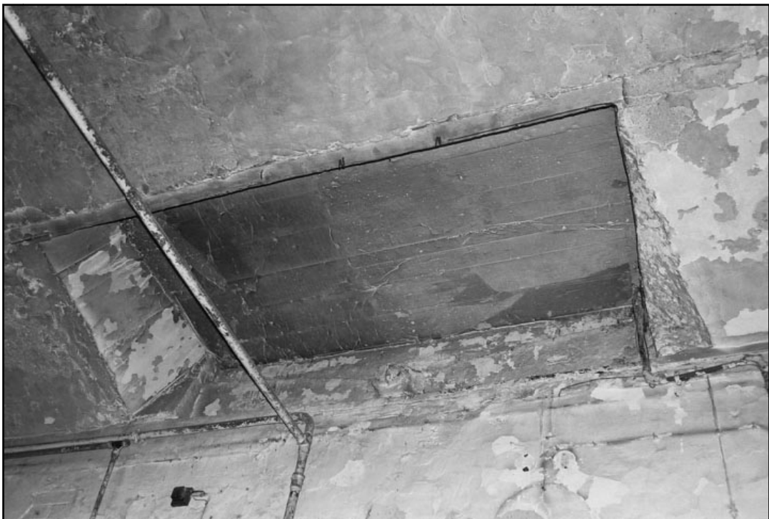
Plate 38: Detail of ceiling hatch with cast iron bracket (film 1.30)
