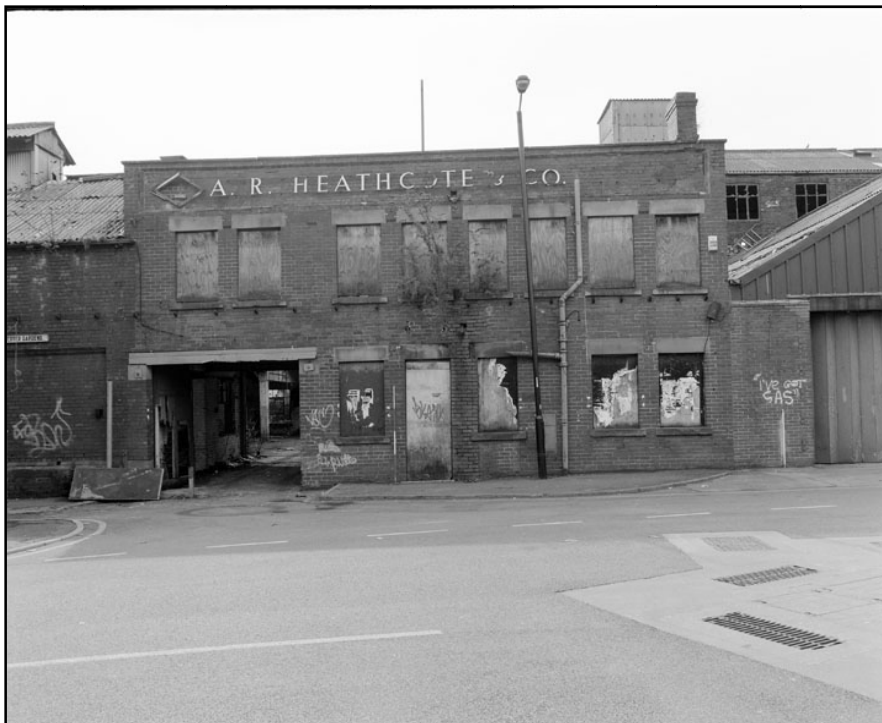
Plate 4: General view of north elevation of office building (film 2.01)
