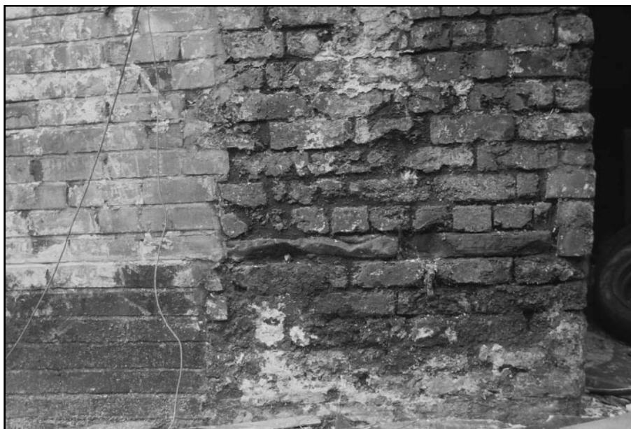
Plate 29: Detail of truncated stone stringcourse below header row in southern wall of grinding workshop (film 1.35)
