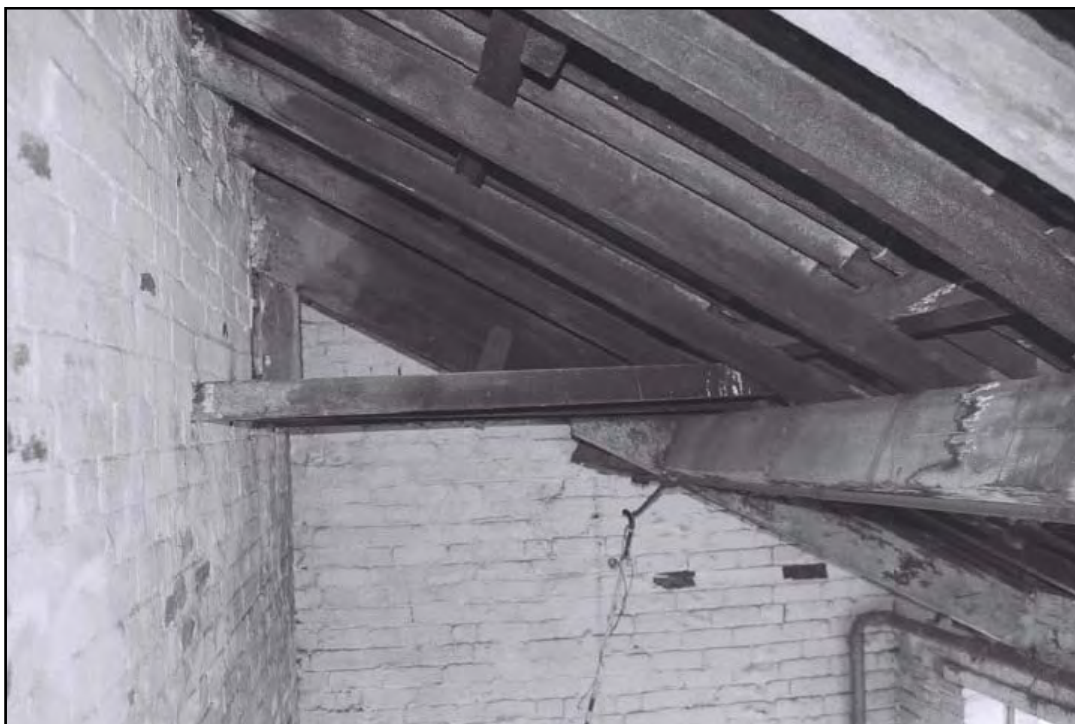
Plate 42: Detail of roof structure of southern half of stair-tower (film 1.22)
