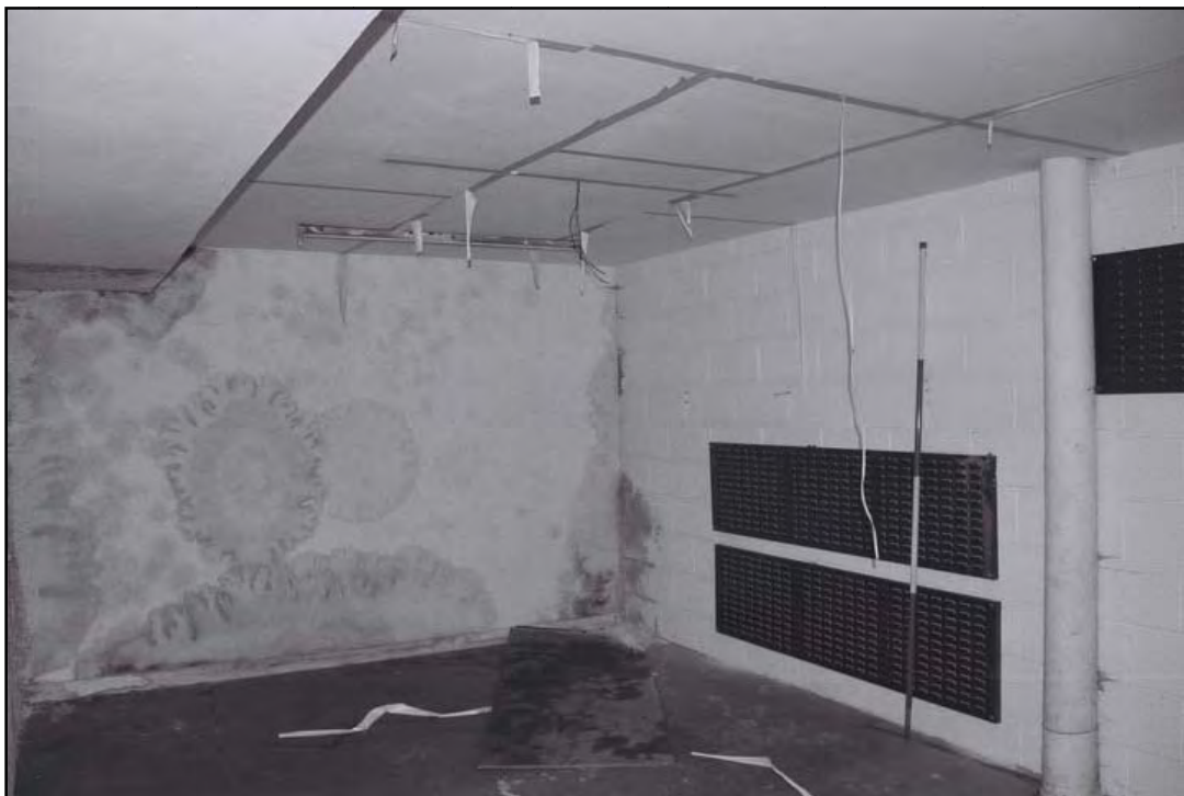
Plate 33: General view of room 2G2 (film 9.10)
