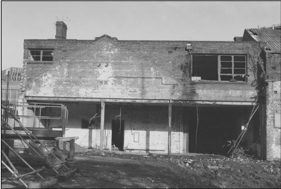
Plate 7: General view of southern elevation of office building (film 9.02)
