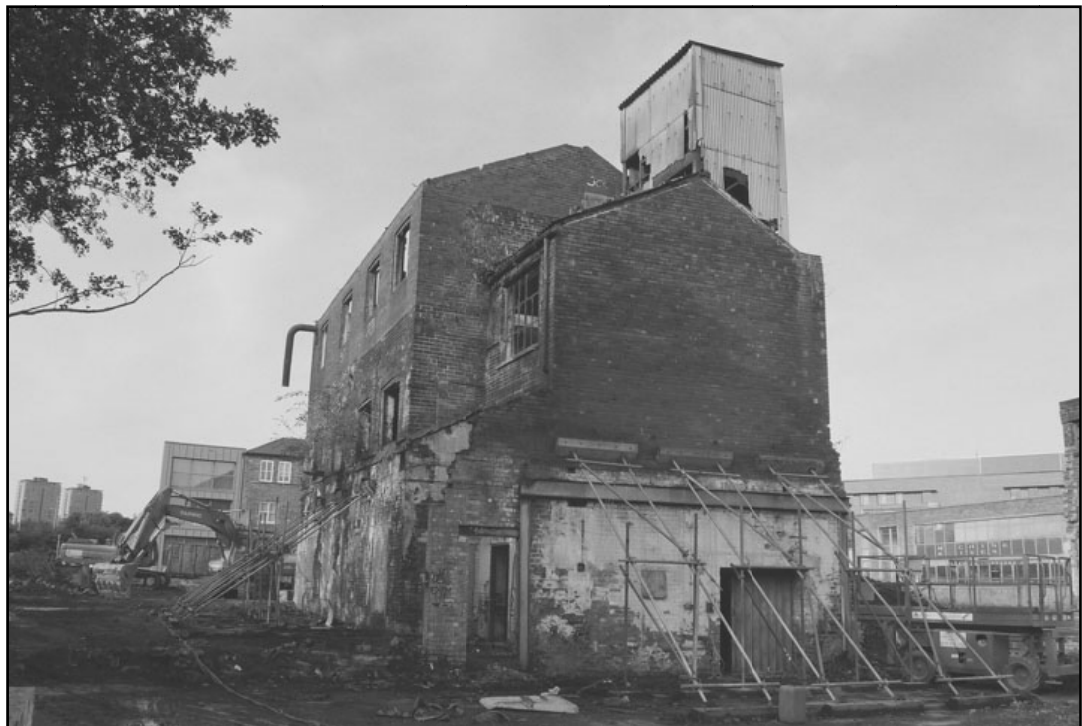
Plate 18: General view of grinding workshop, looking northwest (film 9.22)
