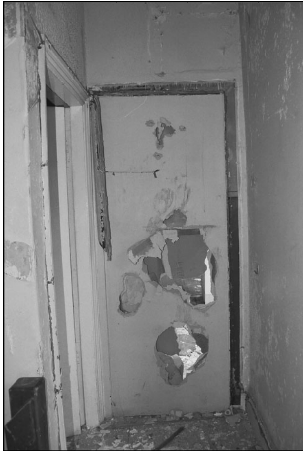
Plate 11: Detail of blocked door at east end of room 1F1 (film 1.04)
