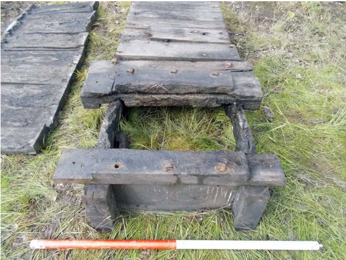
Plate 14. Timber flange plate removed.
