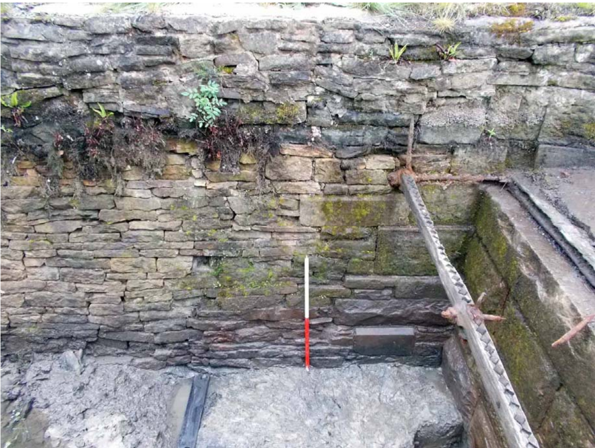
Plate 23. South side wall of canal nearest dam, viewed from north.
