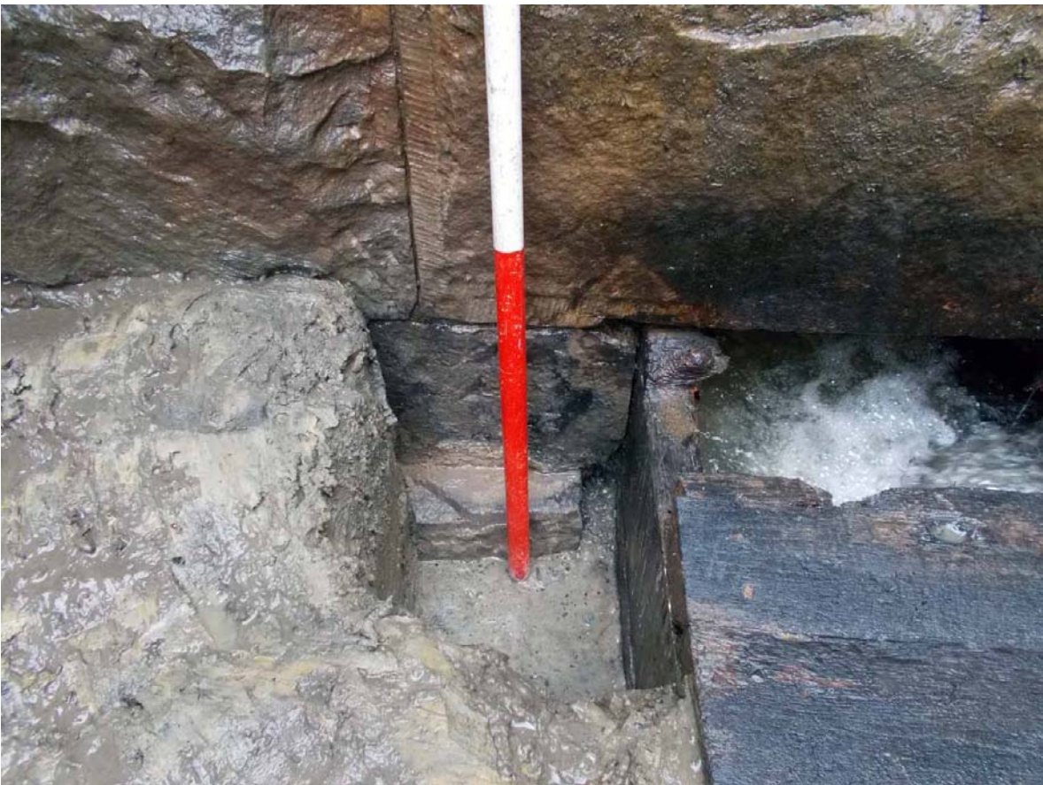
Plate 8. Sondage in puddled clay showing stepped footing of dam, viewed from east.
