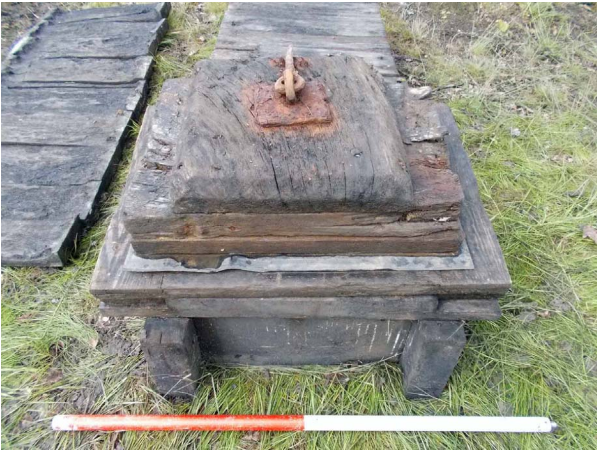
Plate 12. Intake timber plug with rubber seal.
