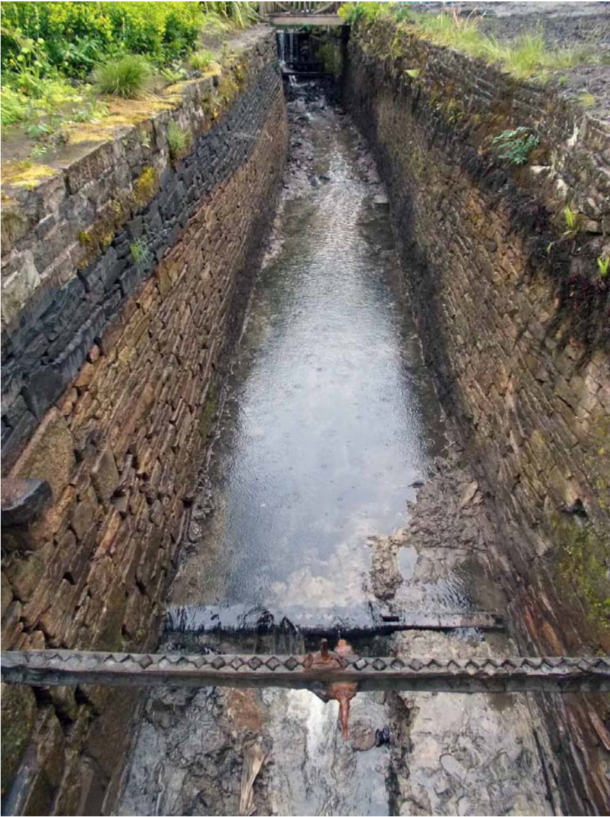
Plate 27. Canal cleared of silt, viewed from west.
