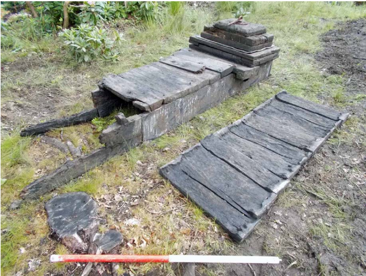
Plate 10. Reassembled ex-situ culvert, note worn base timbers.
