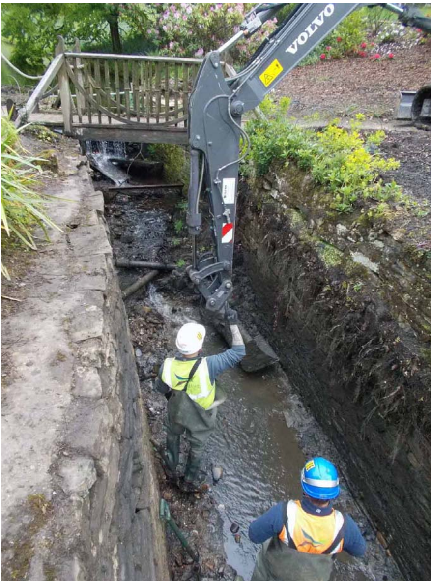
Plate 25. Silt removal from centre of canal, viewed from west.
