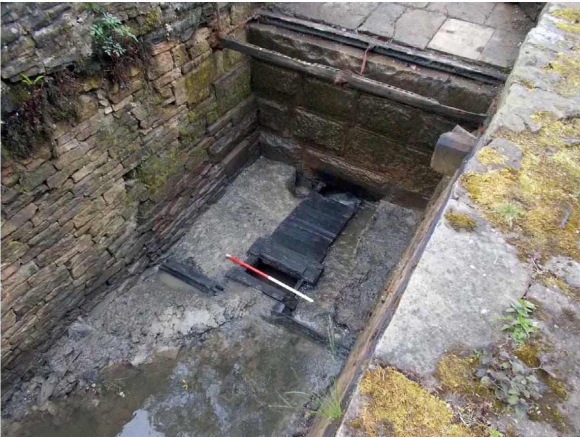
Plate 3. Timber culvert exposed and cleaned up, viewed from east.
