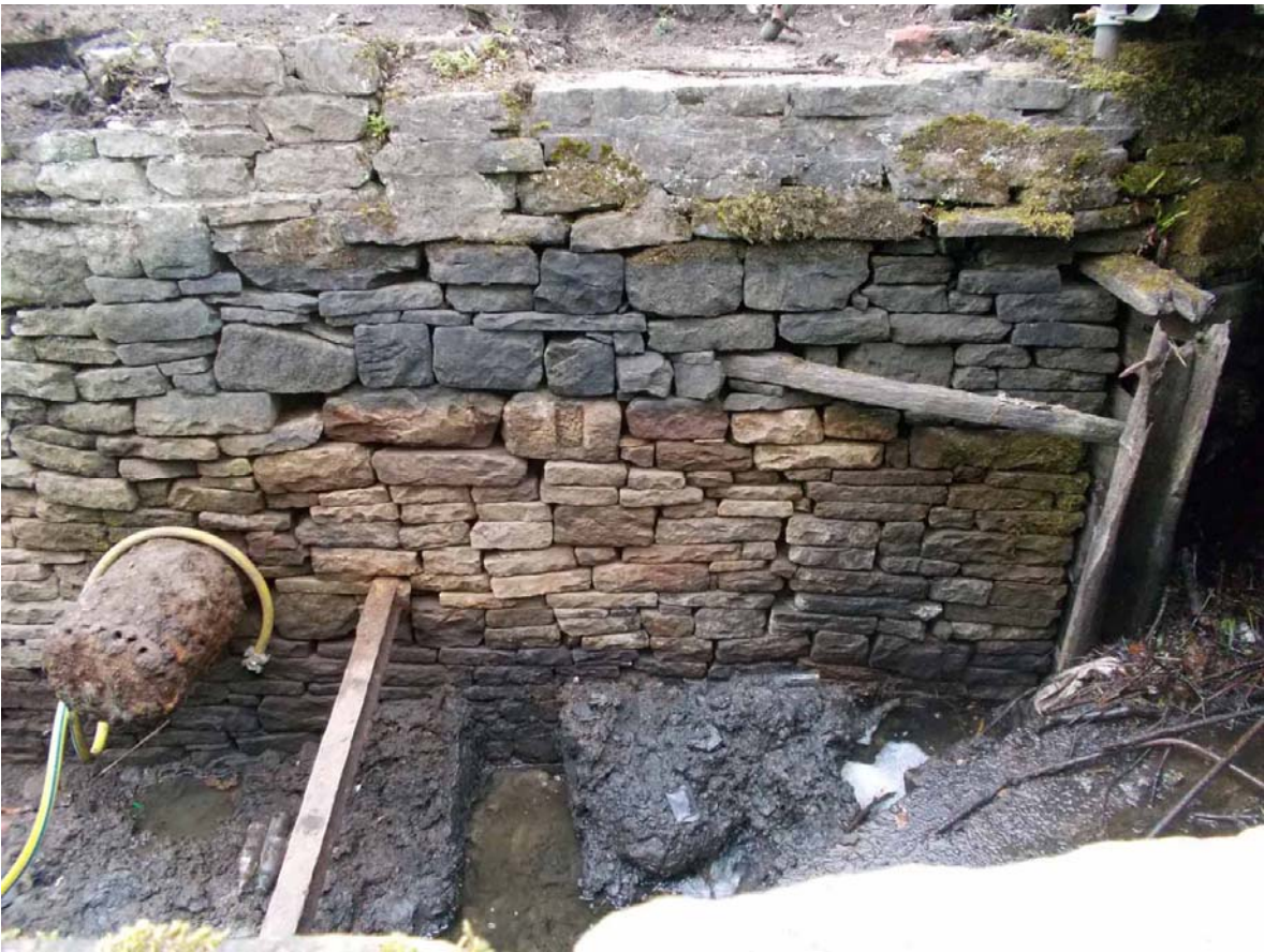
Plate 29. North side wall of canal at east end, viewed from south.
