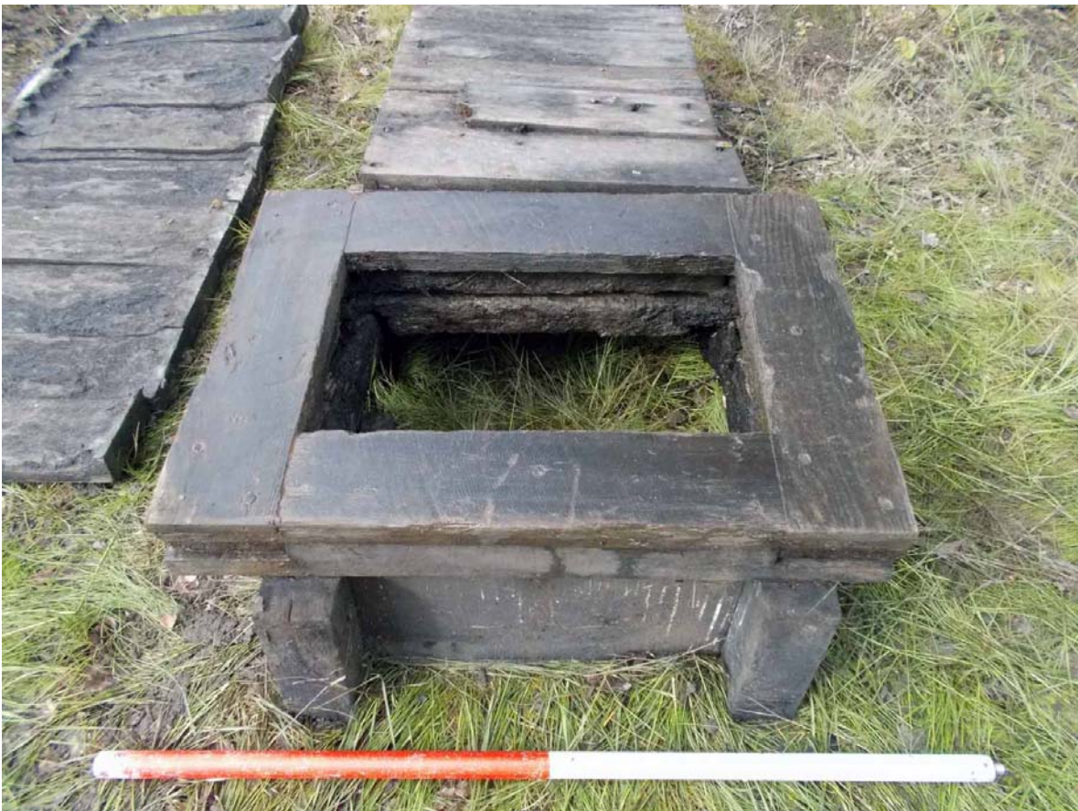
Plate 13. Intake timber flange plate.
