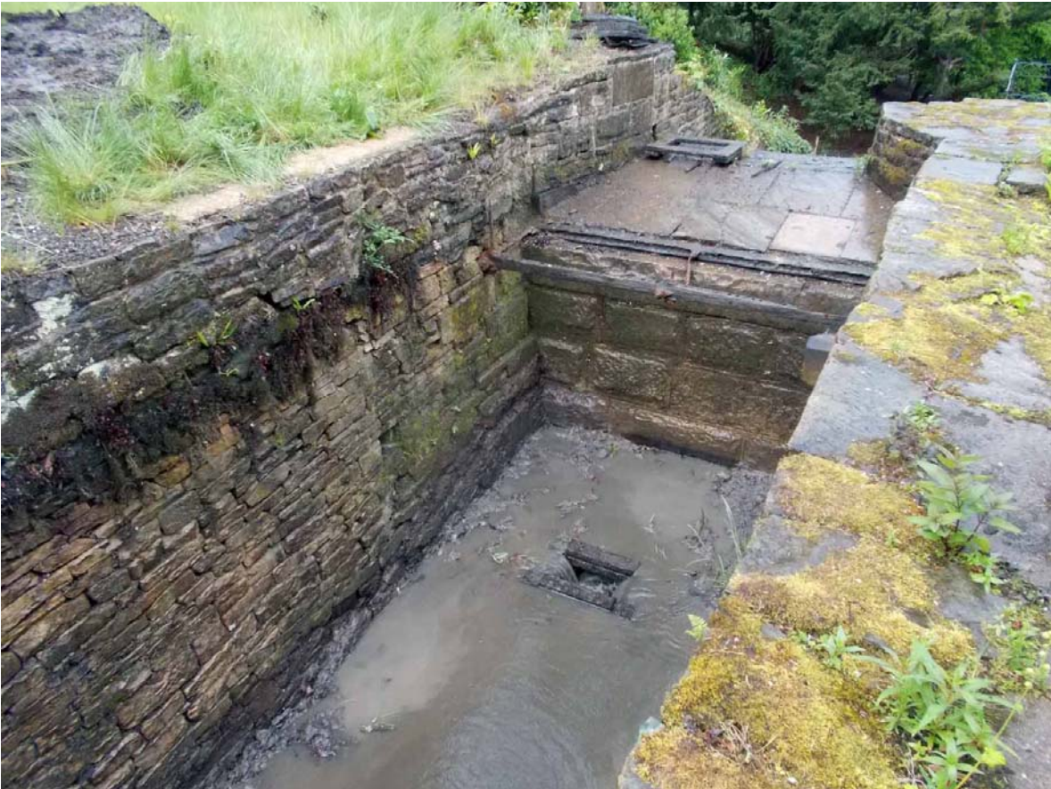
Plate 2. Silt removal completed, viewed from east.
