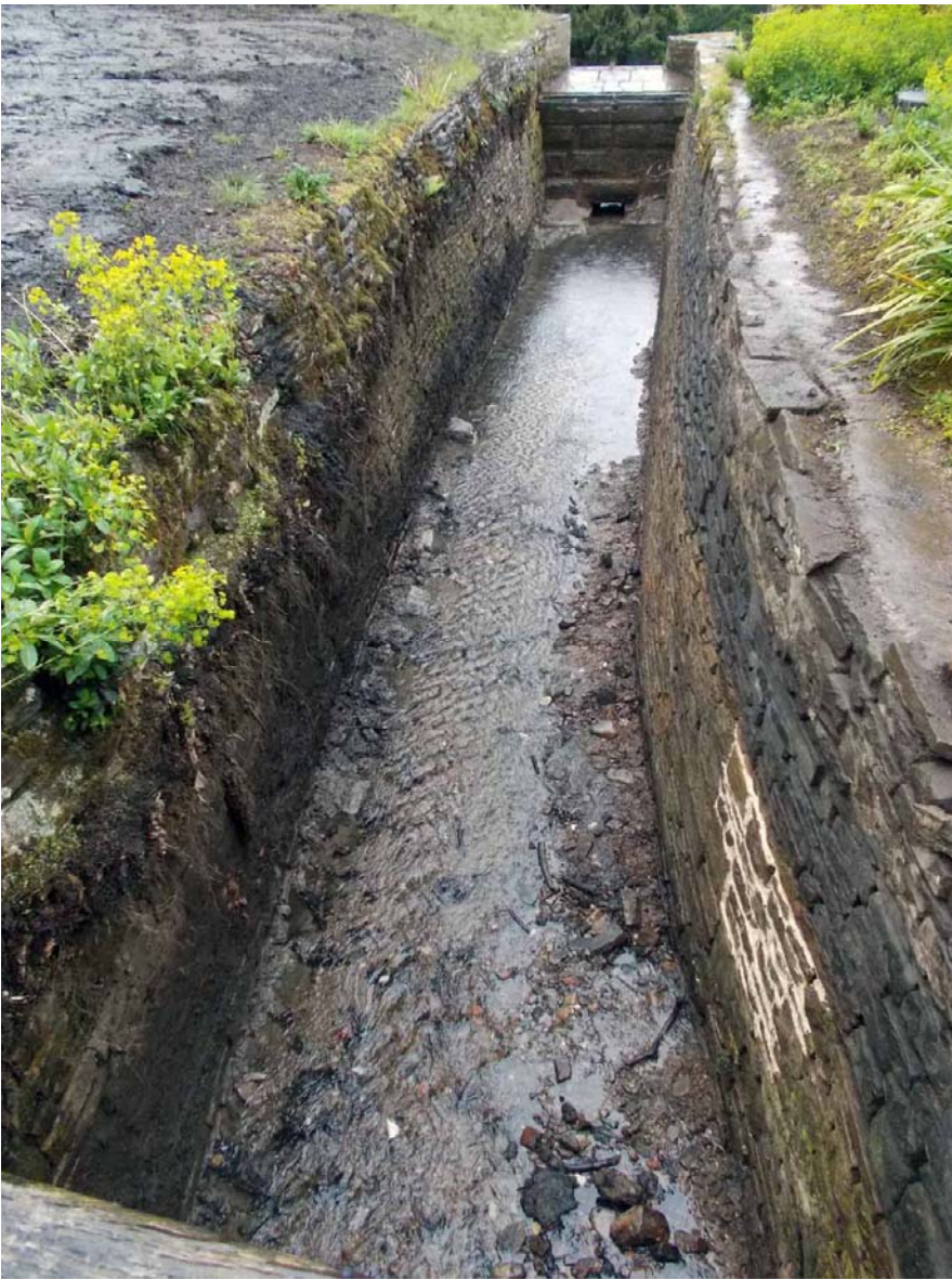
Plate 26. Canal cleared of silt, note puddle clay base, viewed from east.
