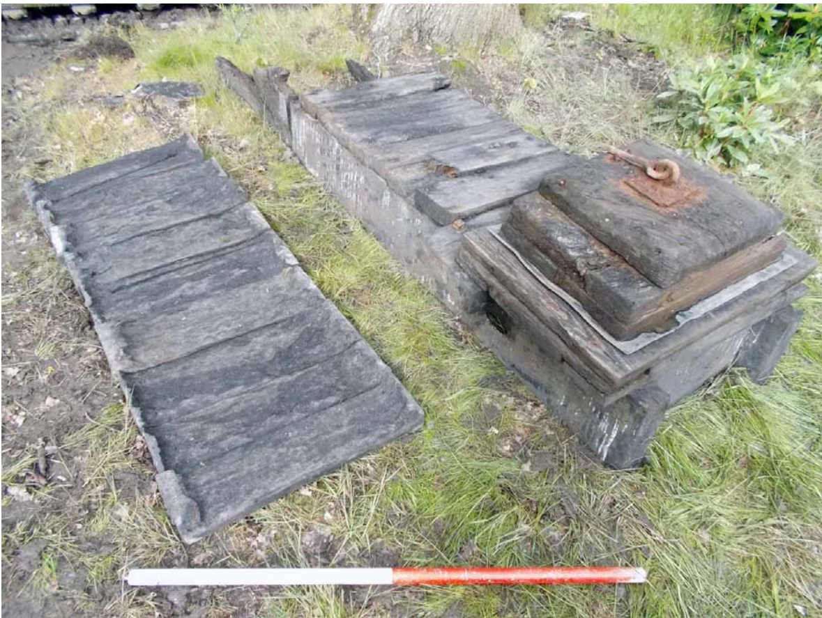
Plate 11. Reassembled ex situ culvert.
