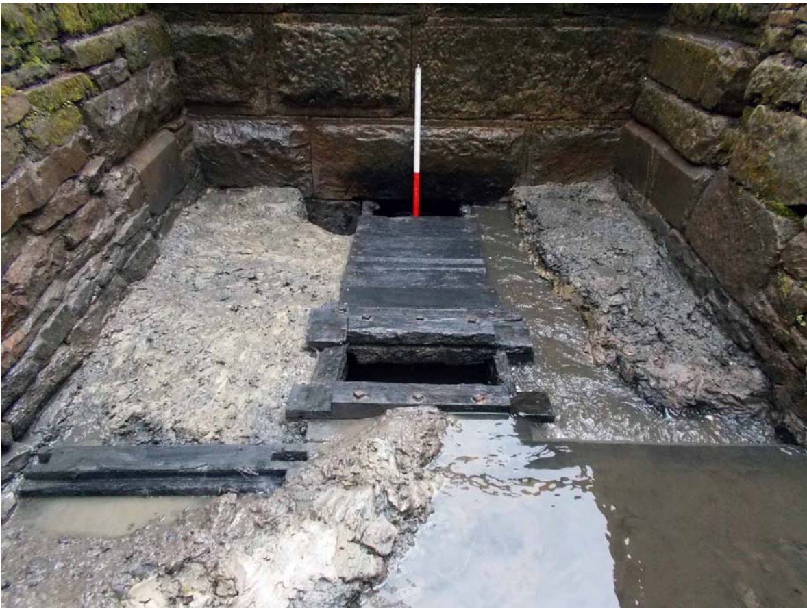
Plate 5. Timber culvert viewed from east.
