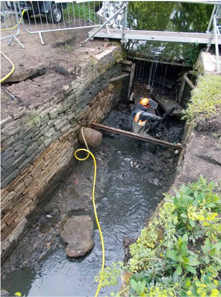
Plate 28. Silt removal at east end of canal, note site of removed bridge, viewed from west.
