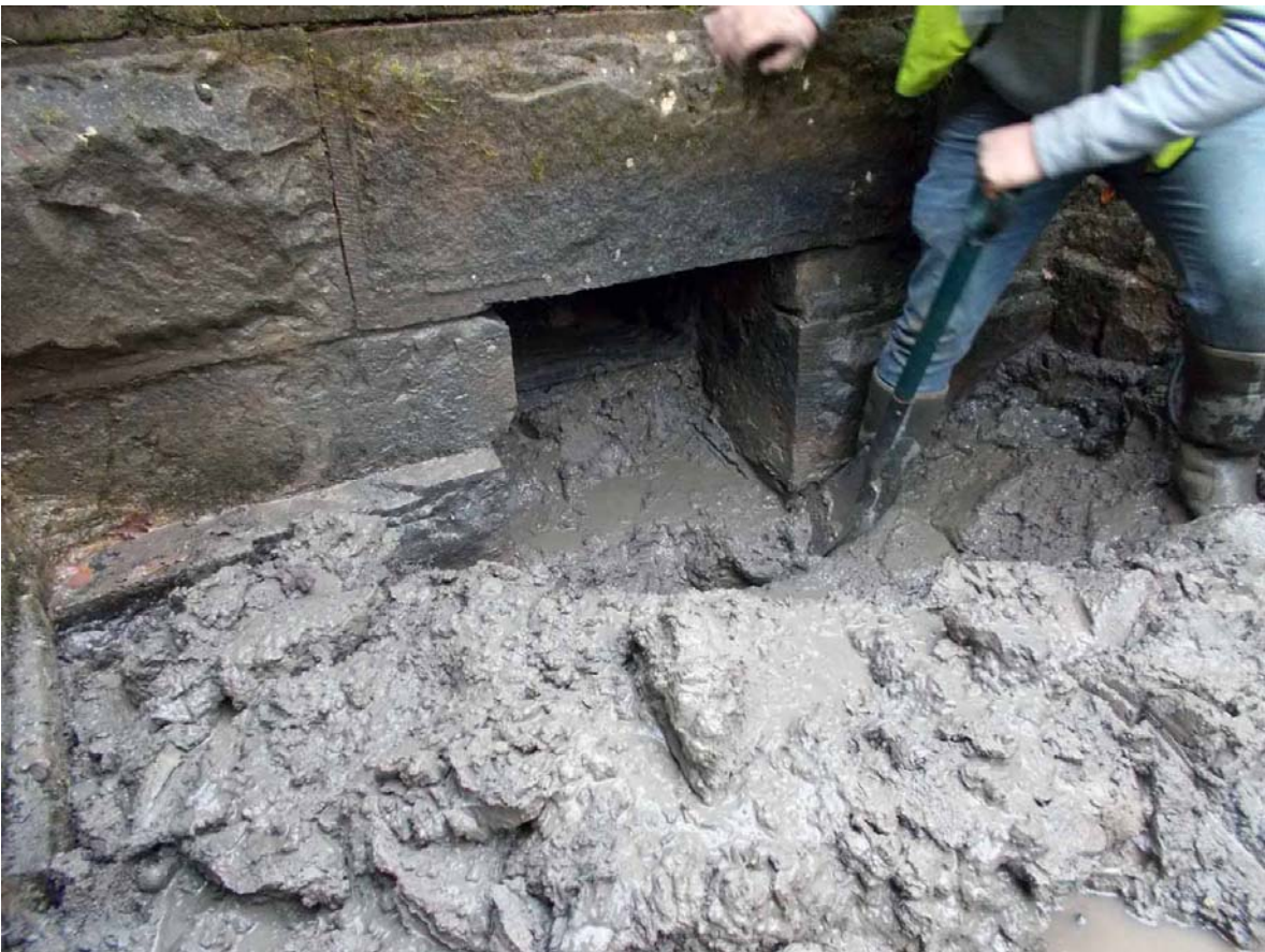
Plate 21. Further excavation within aperture, 30 Oct. 2017, viewed from south-east.
