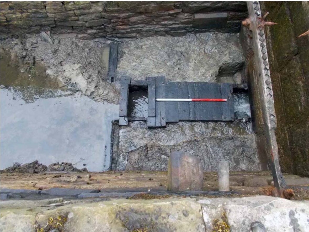
Plate 4. Timber culvert exposed, note surrounding puddled clay, viewed from north.
