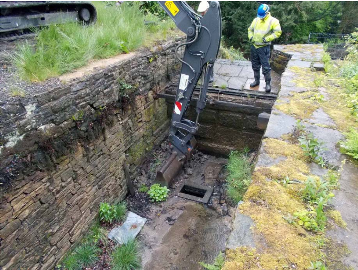
Plate 1. Silt removal at west end of canal, viewed from east.
