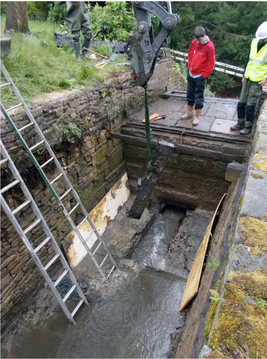
Plate 9. Removal of timber culvert, viewed from east.
