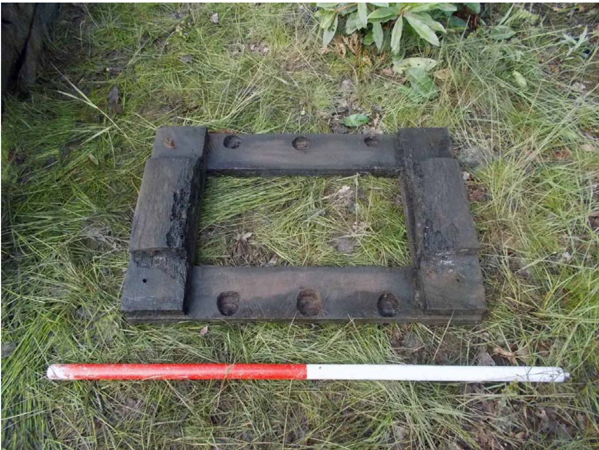
Plate 15. Underside of timber flange plate, note gouged recesses for screw heads.
