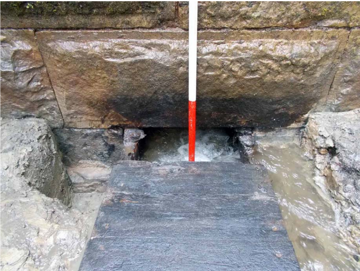
Plate 7. Culvert and aperture in dam base, note missing roof planks, viewed from east.
