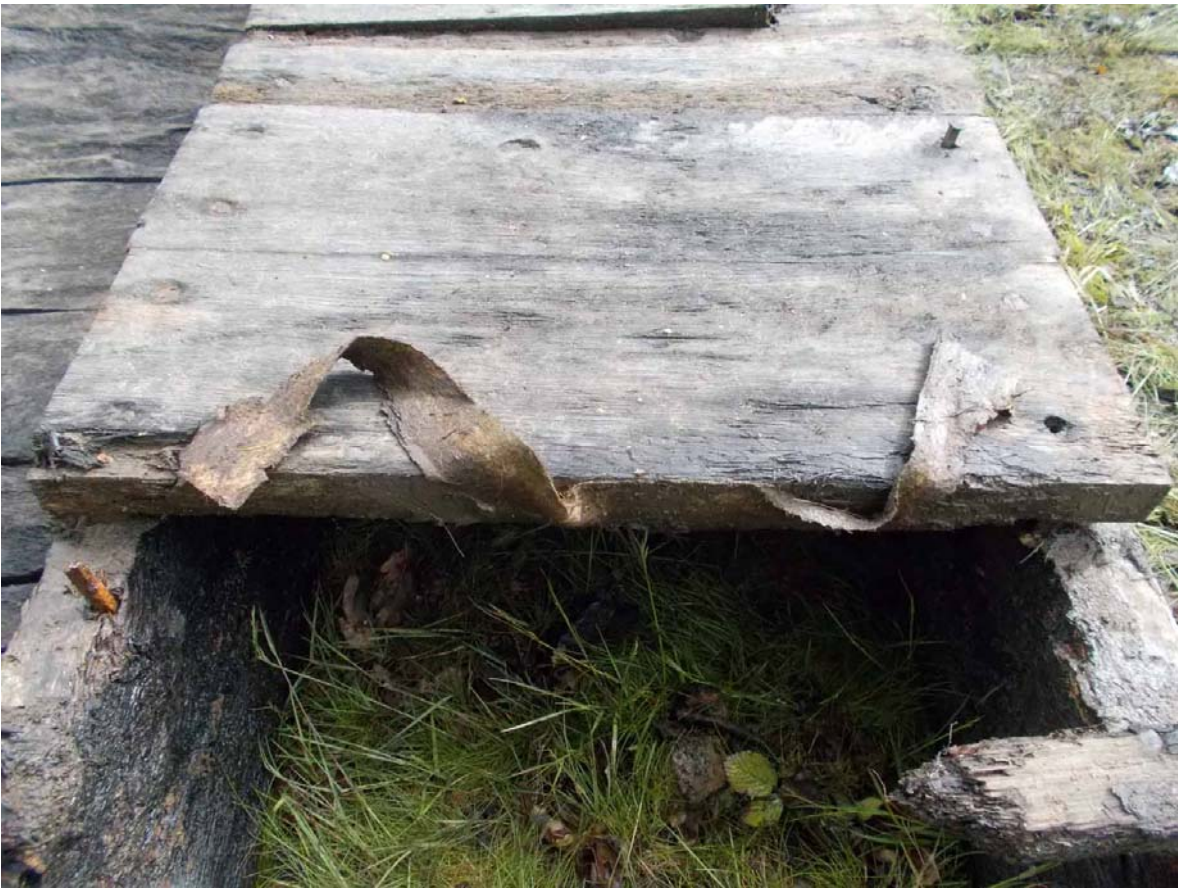
Plate 16. Jointing material between culvert timbers. Possibly a felt strip.
