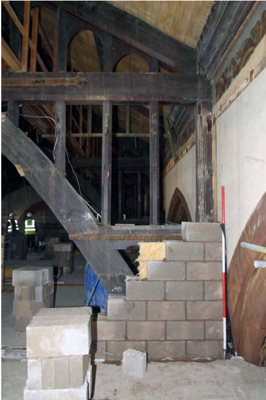
Plate 7. Truss 4/5, east section, lower part, viewed from south.
