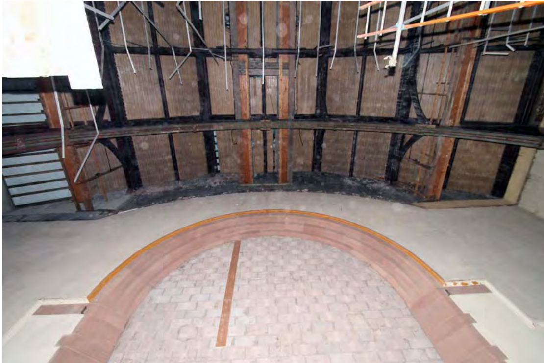
Plate 22. North elevation, infilled arch and roof over, viewed from south.
