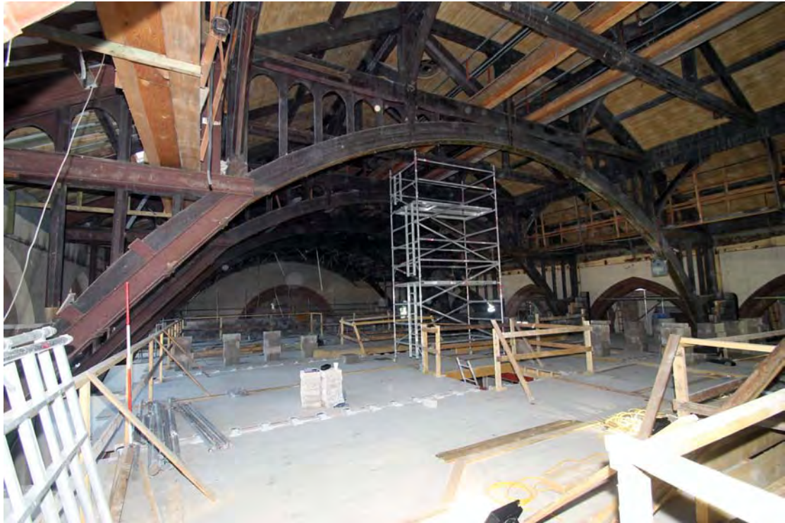
Plate 1. Bay 4/5 truss, viewed from south-west.
