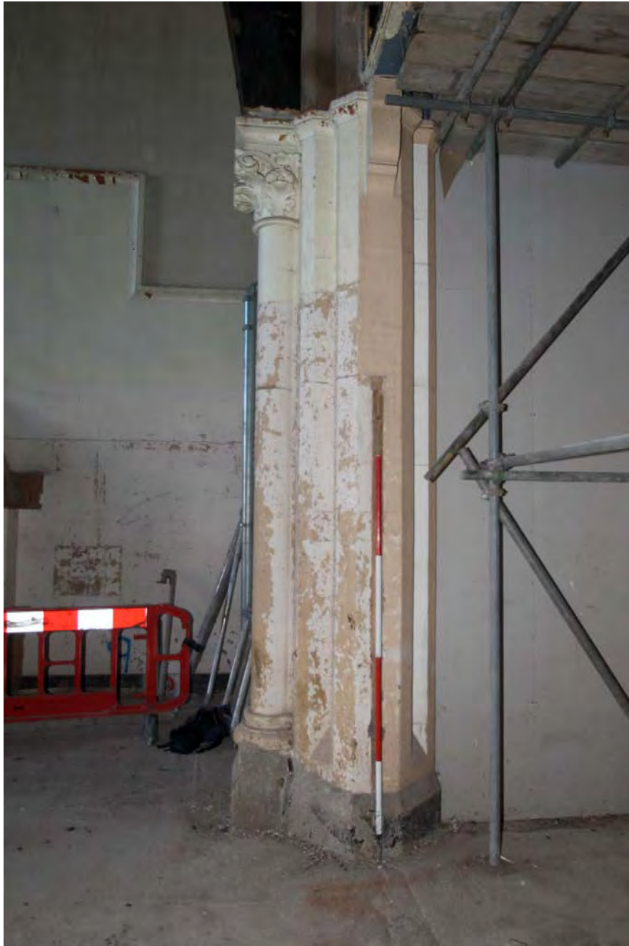
Plate 26. Bay 7/8, eastern elevation, attached column supporting truss base, viewed from south.
