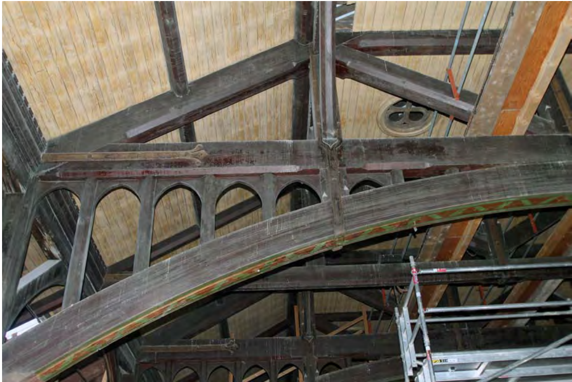
Plate 4. Truss 4/5, west section, upper part, viewed from south.
