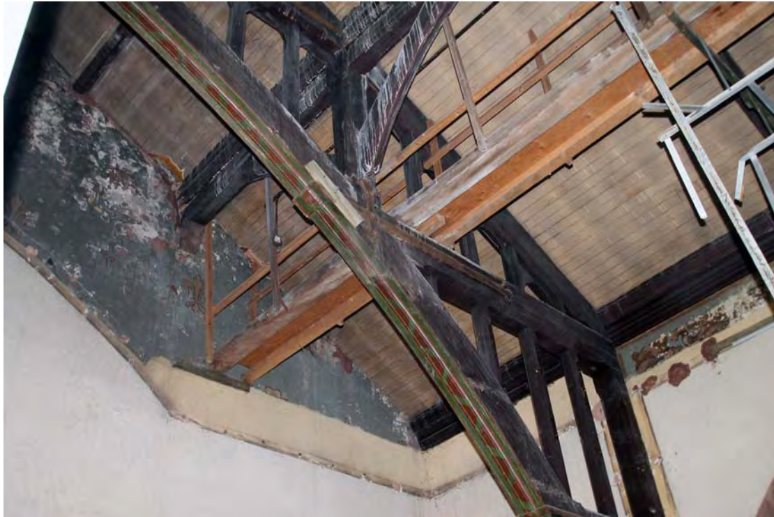
Plate 15. Truss 7/8, east section, viewed from south-west.
