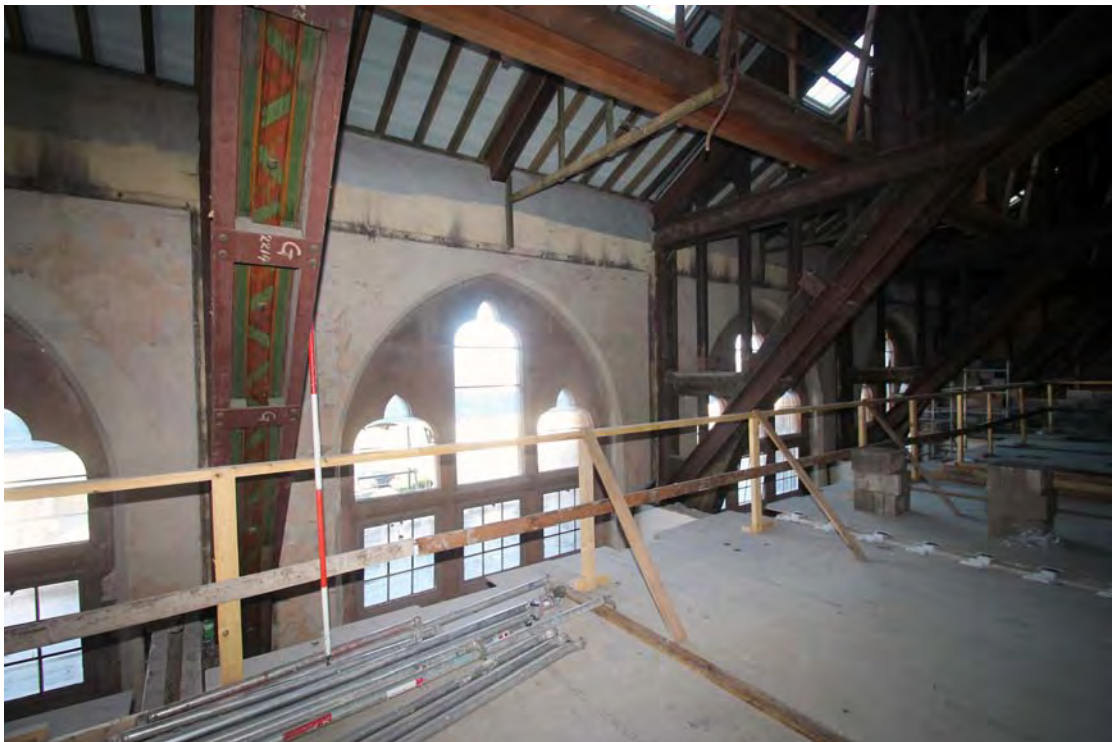
Plate 18. Bay 4, west elevation, window detail, viewed from south-east.
