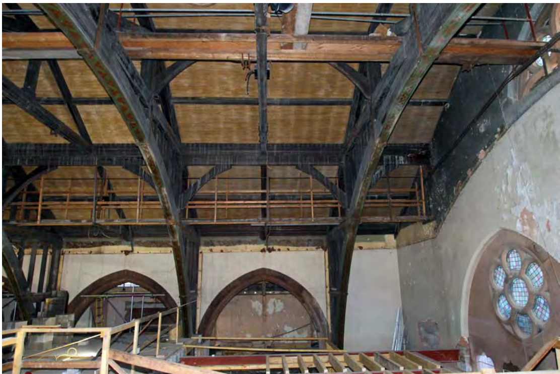
Plate 14. Roof structure within bays 1, 2 and 3, viewed from west.
