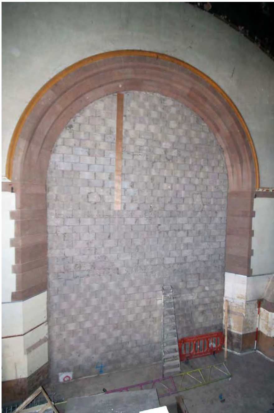
Plate 21. North elevation, infilled arch, viewed from south-west.
