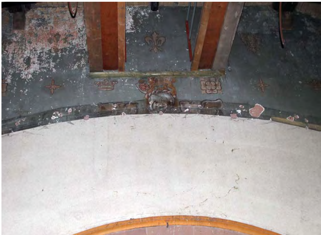
Plate 23. North elevation, remnant of decoration above infilled arch, viewed from south.
