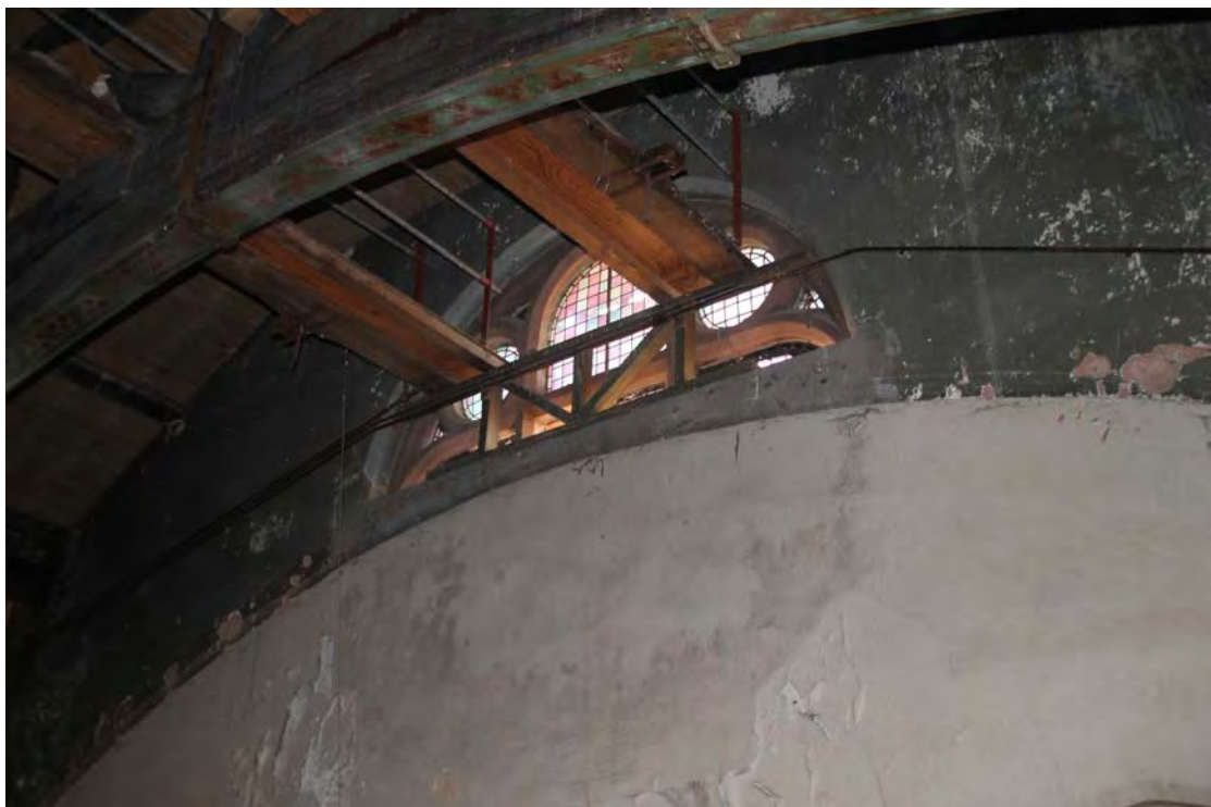
Plate 20. South elevation, upper lunette detail, viewed from north-west.
