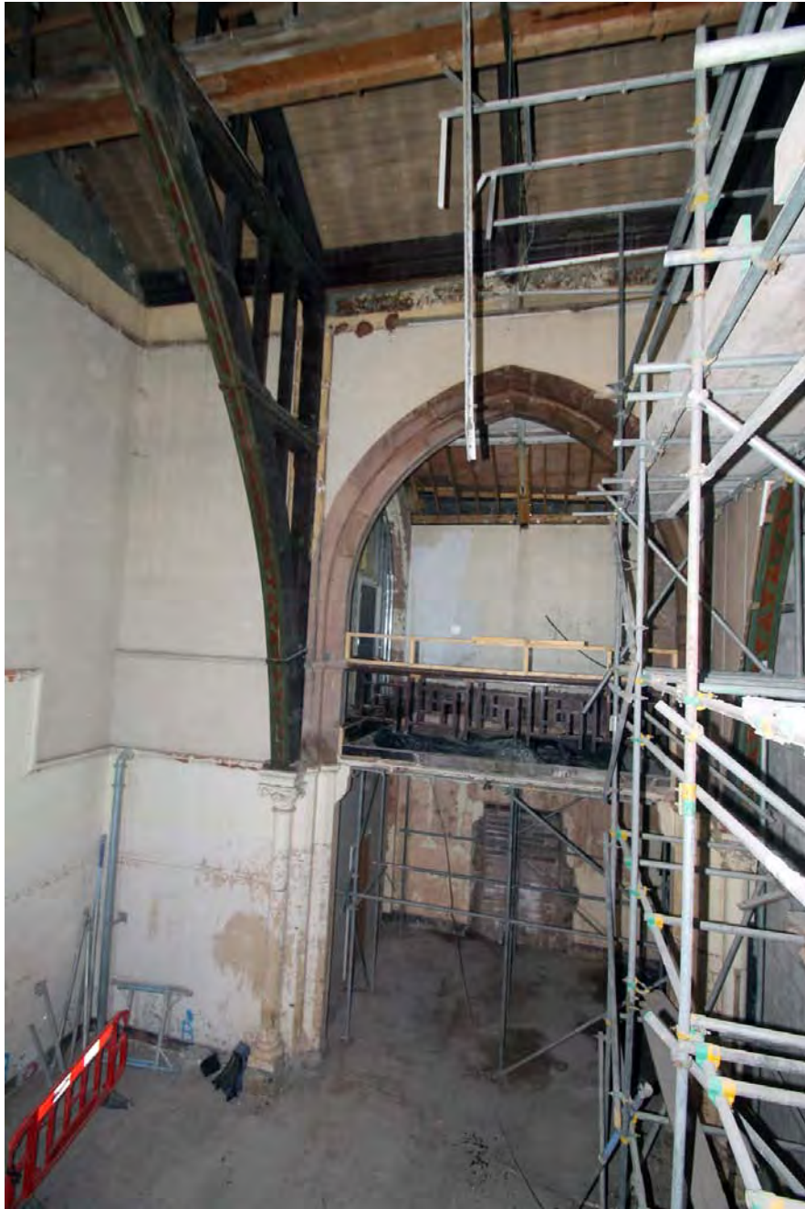
Plate 25. Bays 7/8, east elevation, viewed from west.
