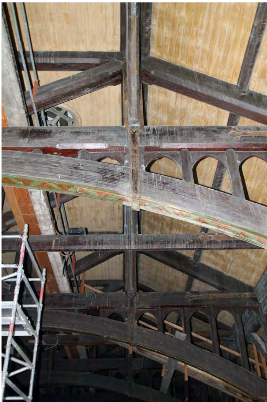
Plate 10. Truss 4/5, east section, detail on upper truss, viewed from south.
