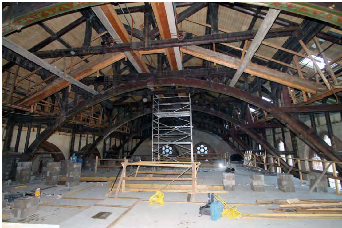
Plate 2. Roof, viewed from north.
