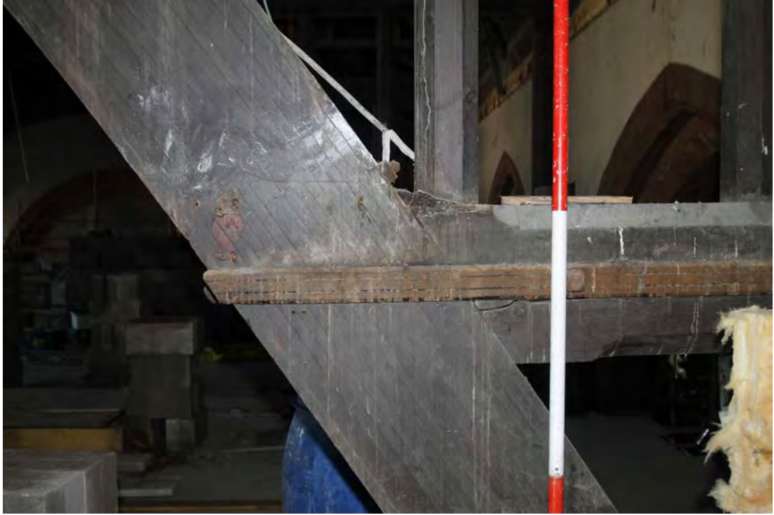
Plate 8. Truss 4/5, east section, lower hammer-beam joint, viewed from south.
