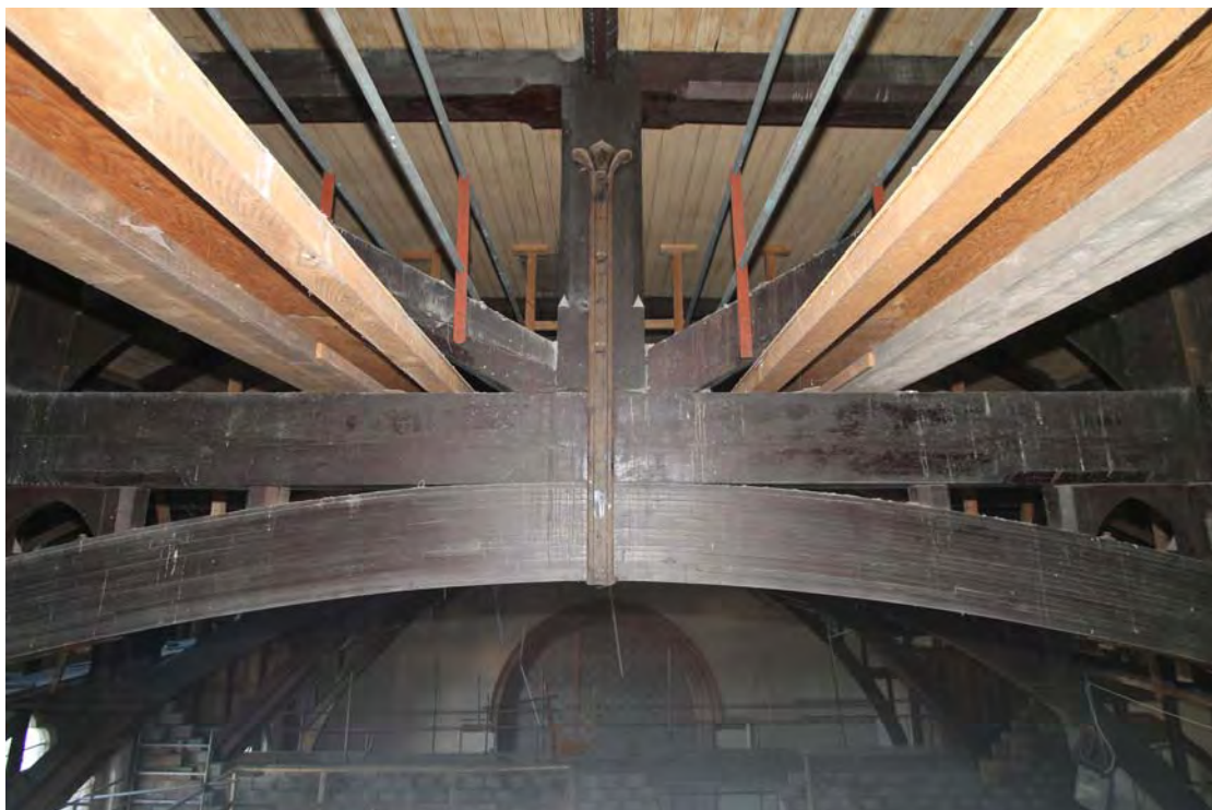
Plate 12. Truss 4/5, central section, viewed from south.
