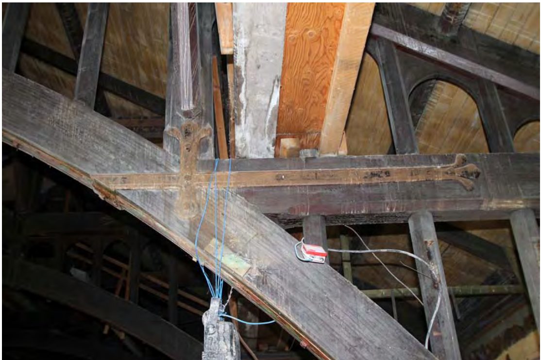
Plate 9. Truss 4/5, east section, upper hammer-beam joint, viewed from south.
