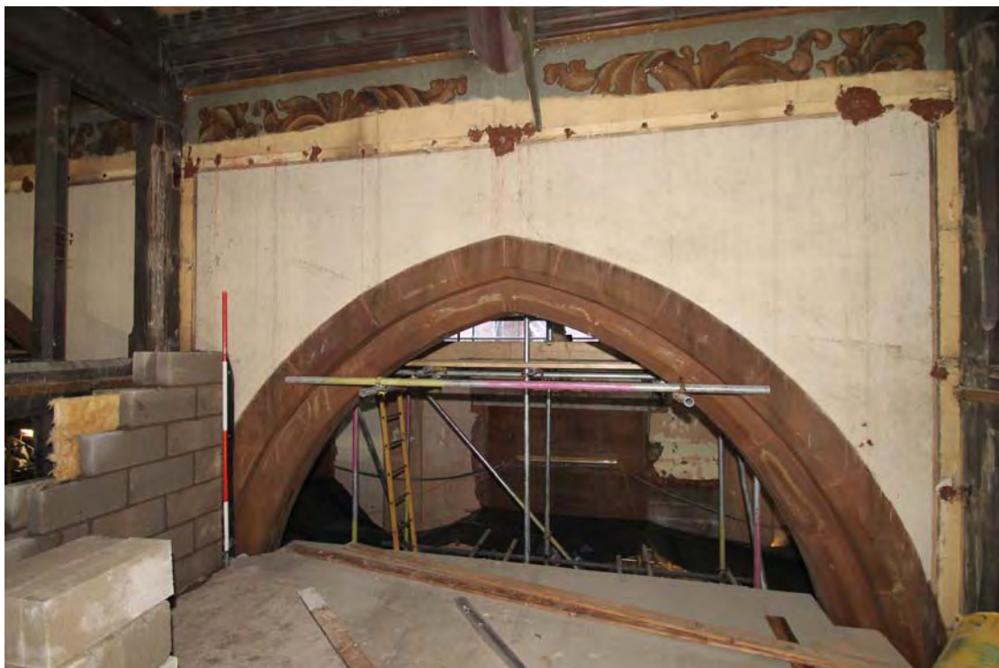
Plate 16. Bay 4, east elevation, upper section of pointed arch, viewed from south-west.
