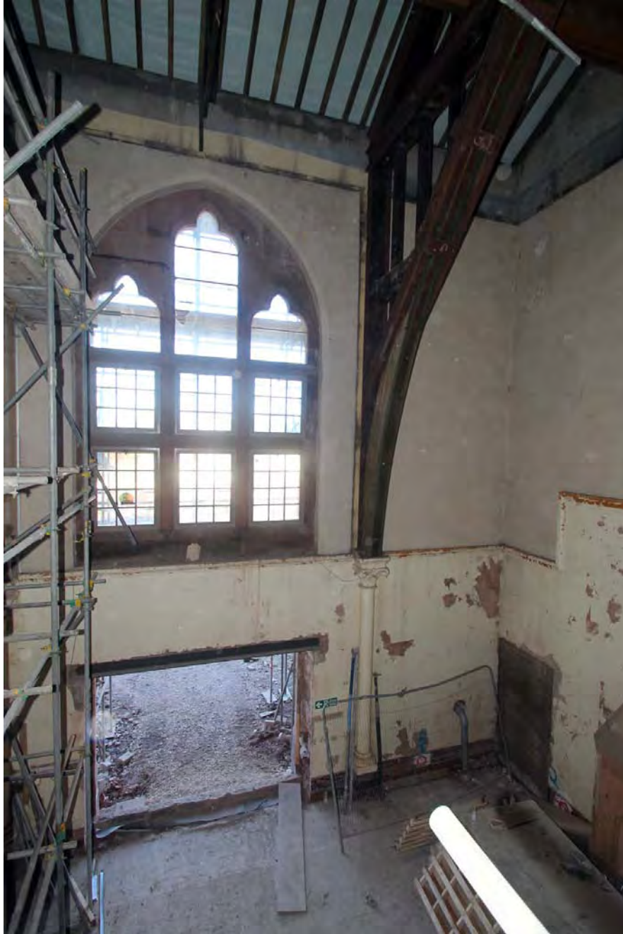
Plate 24. Bays 7/8, west elevation, viewed from east.
