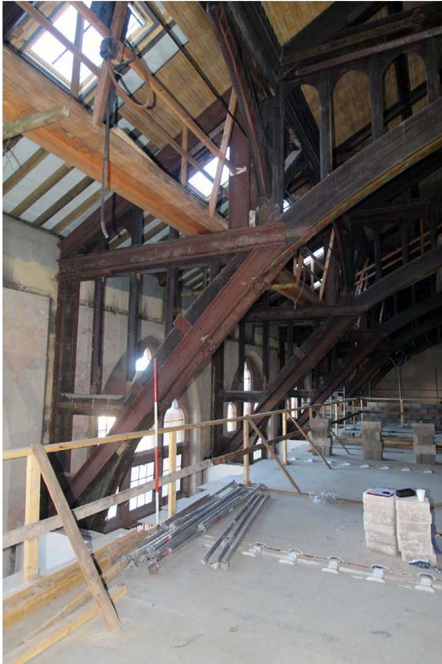
Plate 3. Truss 4/5, west section, lower part, viewed from south-east.
