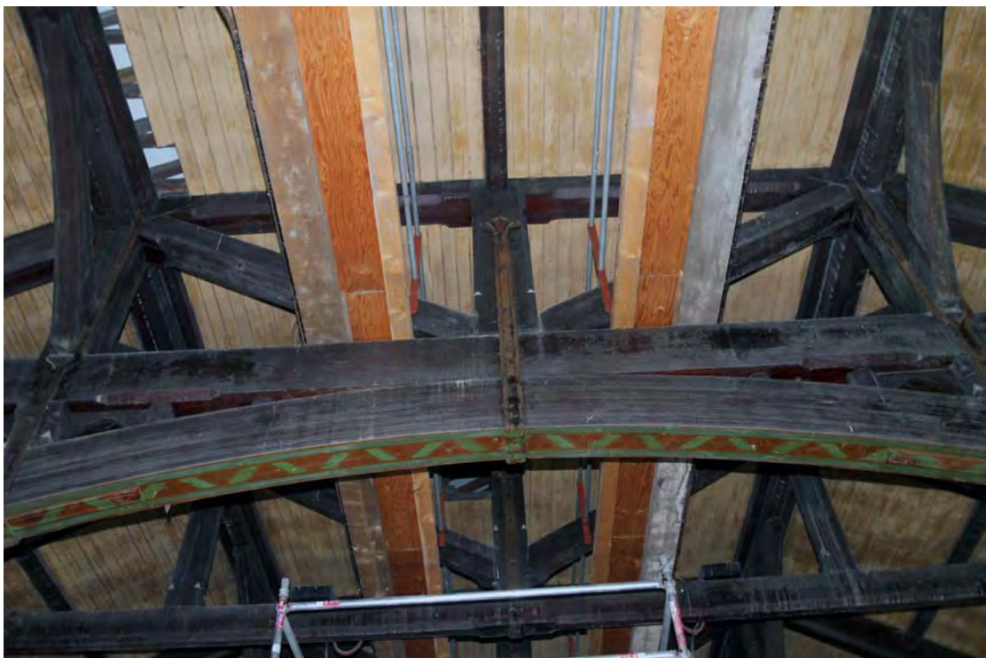
Plate 5. Truss 4/5, central section, viewed from south.
