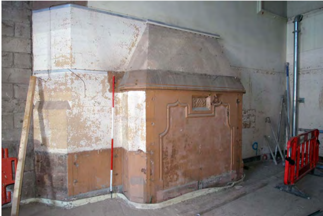
Plate 28. Bay 8, east section of north elevation, blocked fireplace, viewed from southwest.
