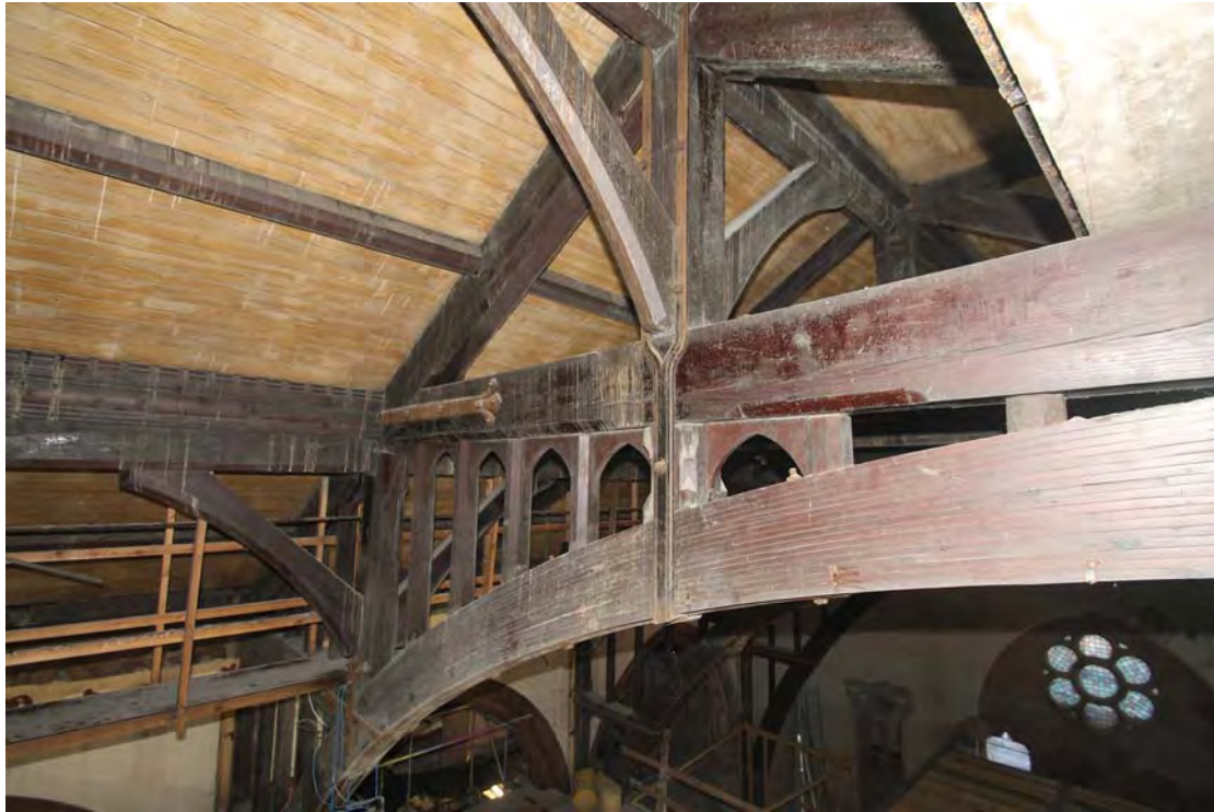
Plate 11. Truss 4/5, west section, detail on uppermost truss, viewed from south-east.
