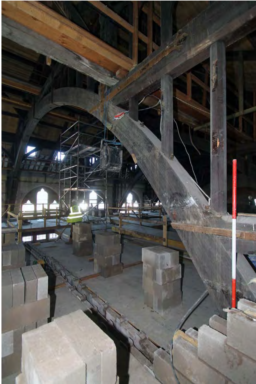
Plate 6. Truss 4/5, viewed from south-east.
