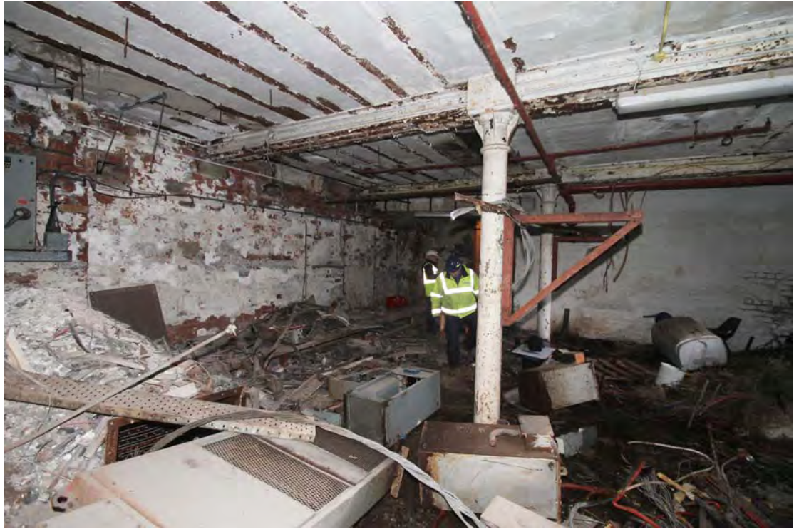
Plate 18. Boiler House ground floor (Building 9), viewed from north-east.
