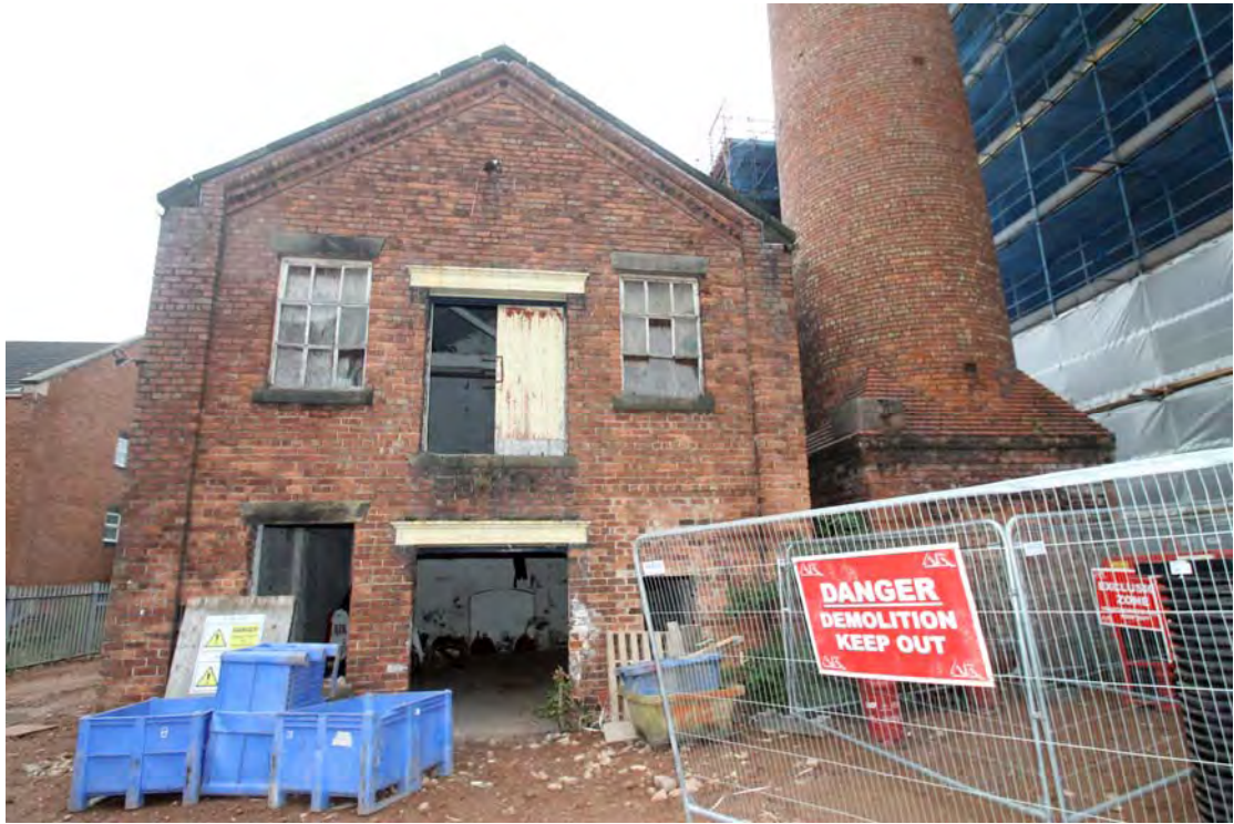
Plate 2. South elevation of Building 19, viewed from south.
