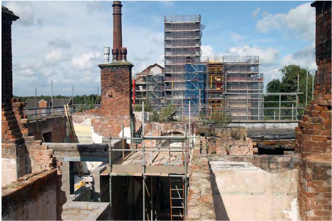
Plate 99. Mansion House, first floor, view northwards across building from pediment.
