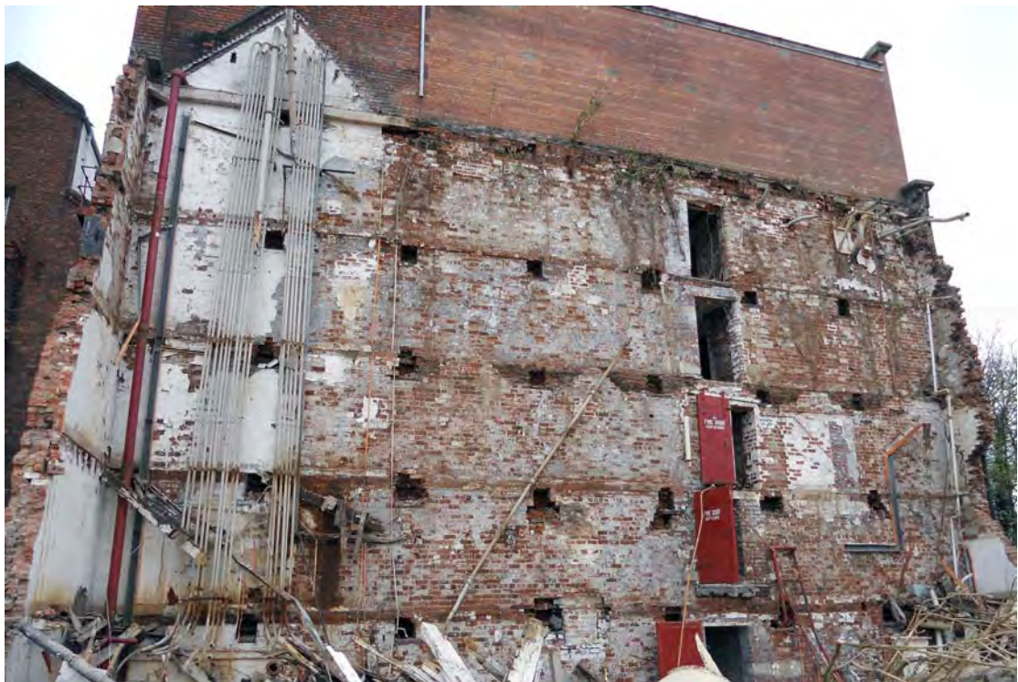
Plate 78. Warehouse Northern Bay (Building 1A), following demolition, viewed from south.
