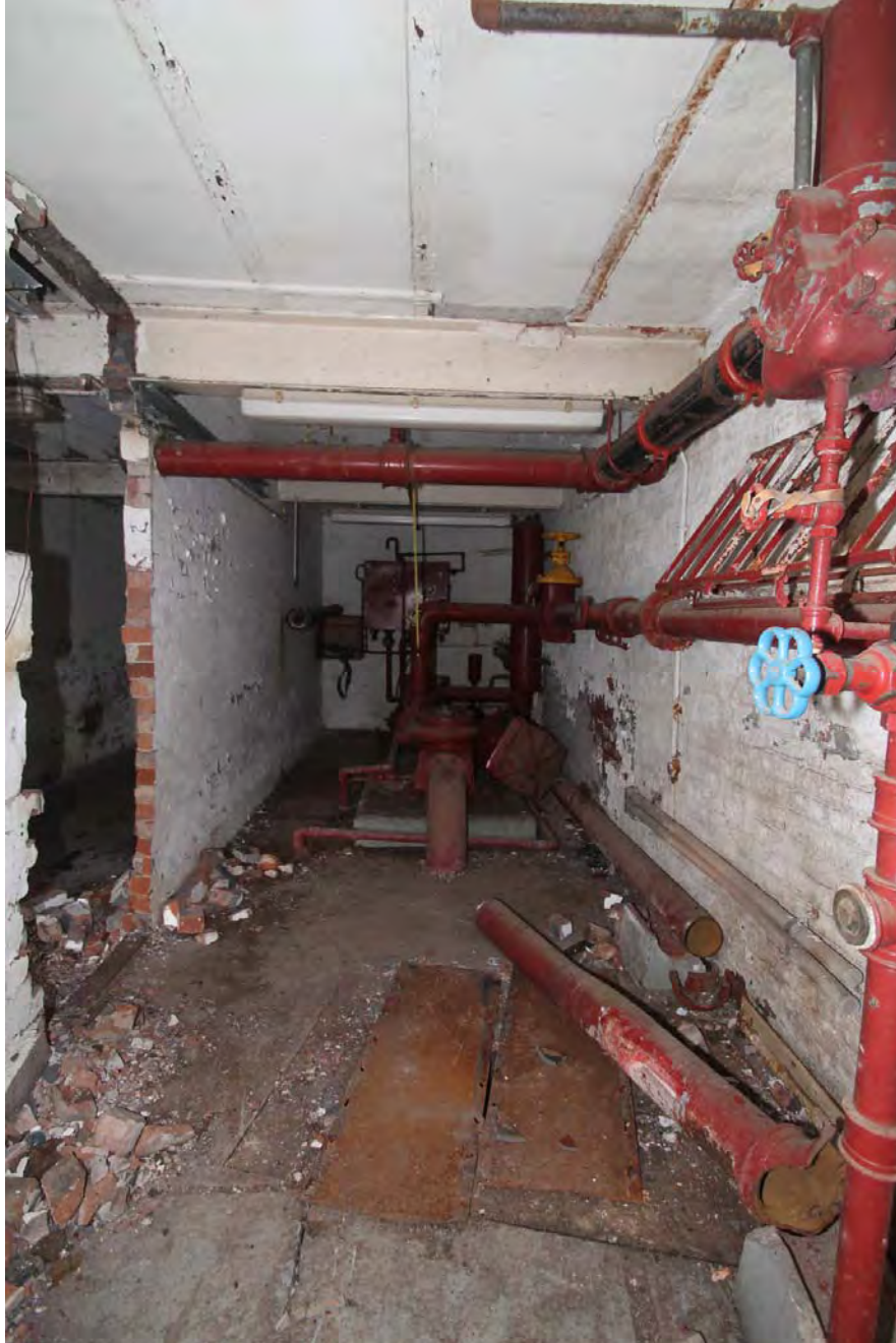
Plate 59. Pumphouse (Building 12), ground floor, viewed from north.
