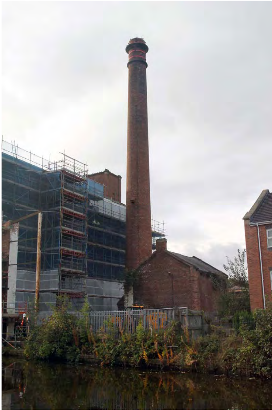
Plate 8. Chimney and Building 19, viewed from north-west.
