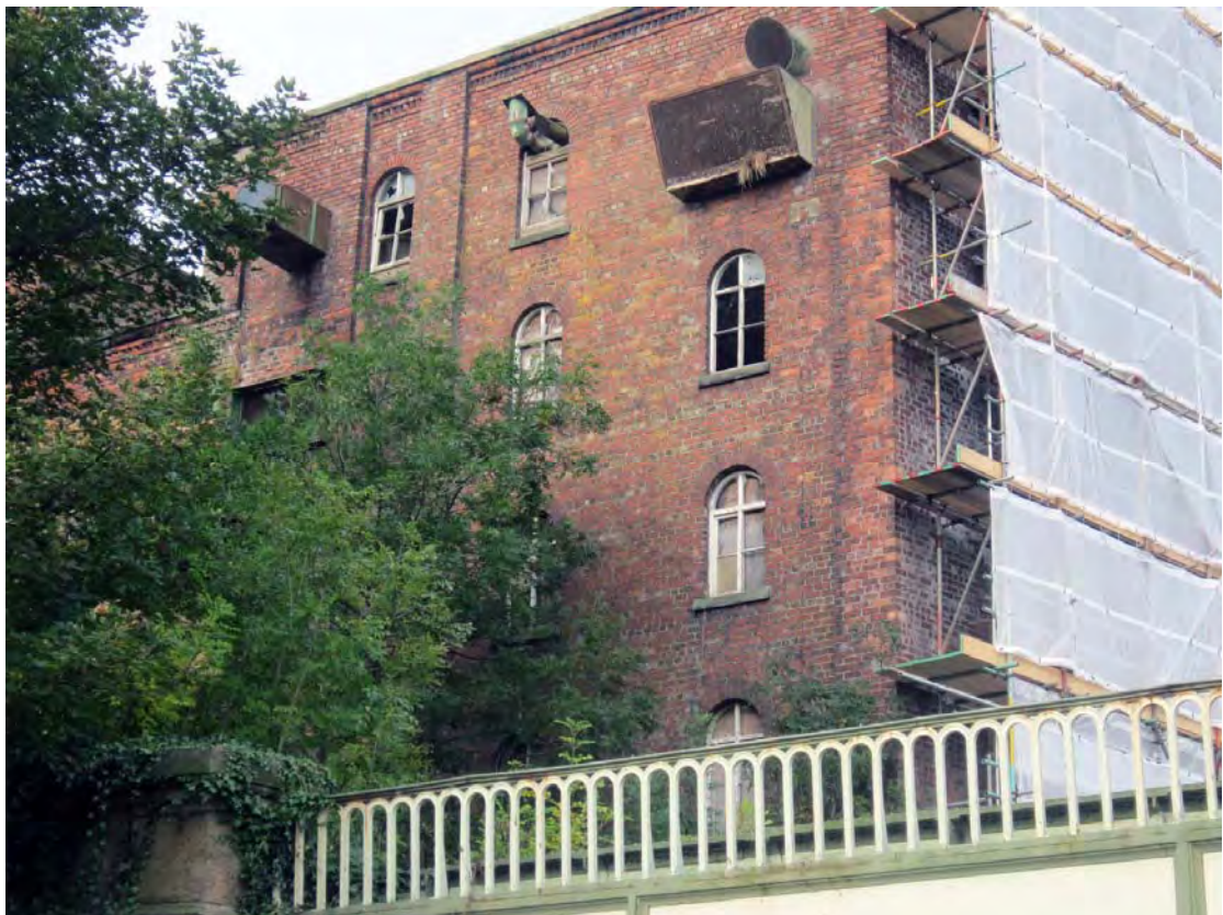
Plate 12. Close up of mill from north-east, Building 9.
