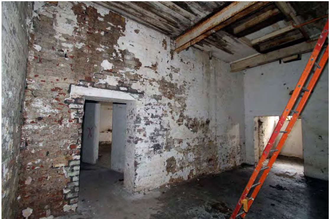
Plate 30. Engine House (Building 8) first floor, viewed from south-west.
