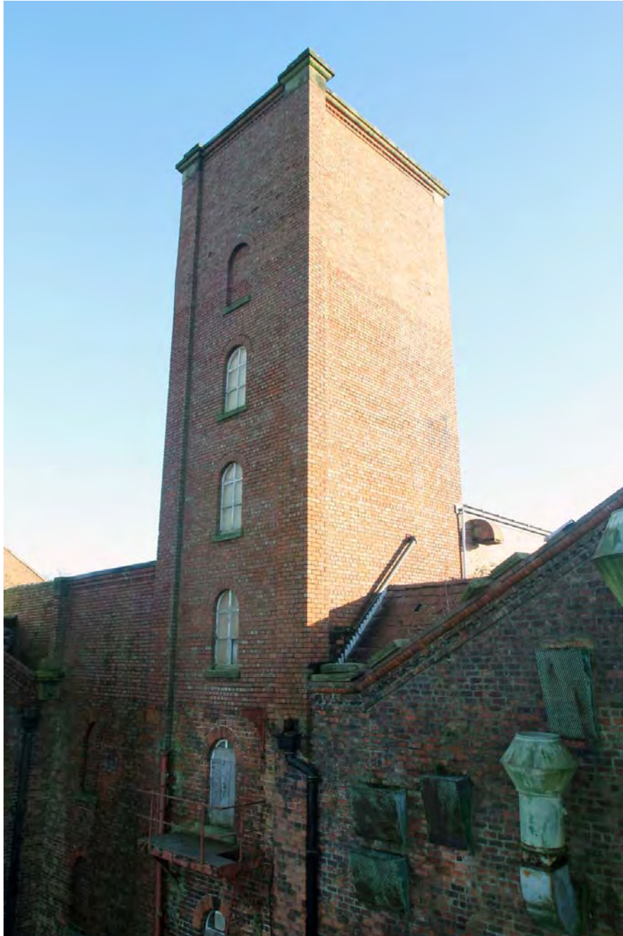
Plate 61. Water Tower (Building 5), viewed from south-west, from cherry picker.
