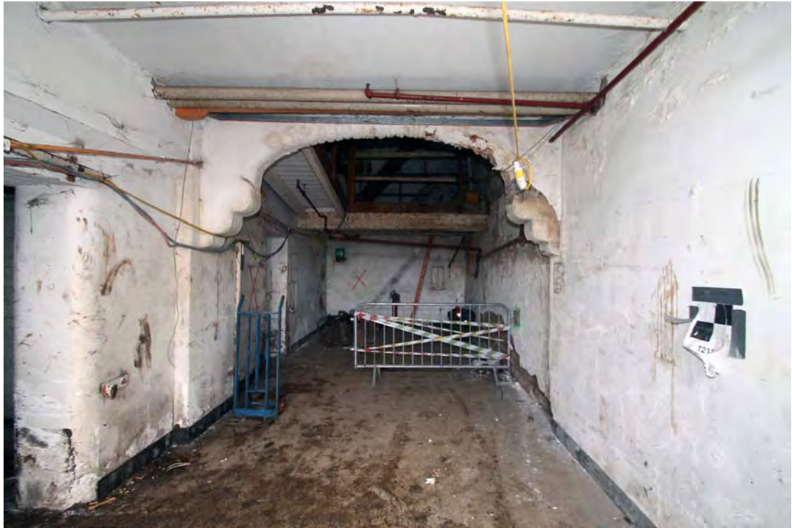
Plate 62. Building 5, ground floor level, east-west passage, viewed from west.
