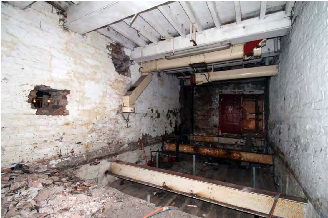
Plate 33. Engine House (Building 8), second floor, viewed from east.
