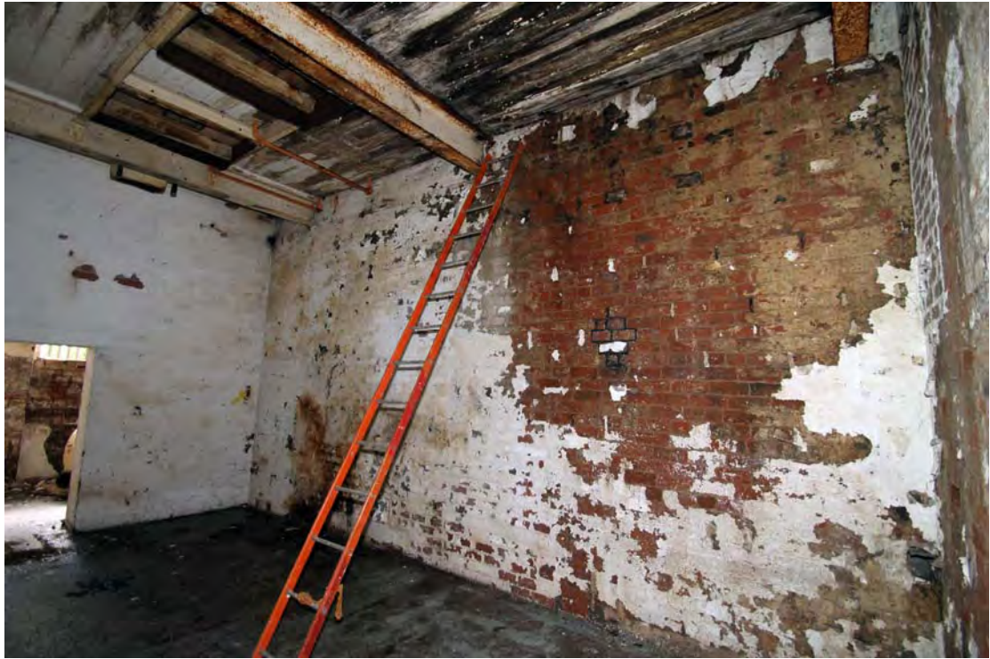
Plate 29. Engine House (Building 8) first floor, viewed from north-west.
