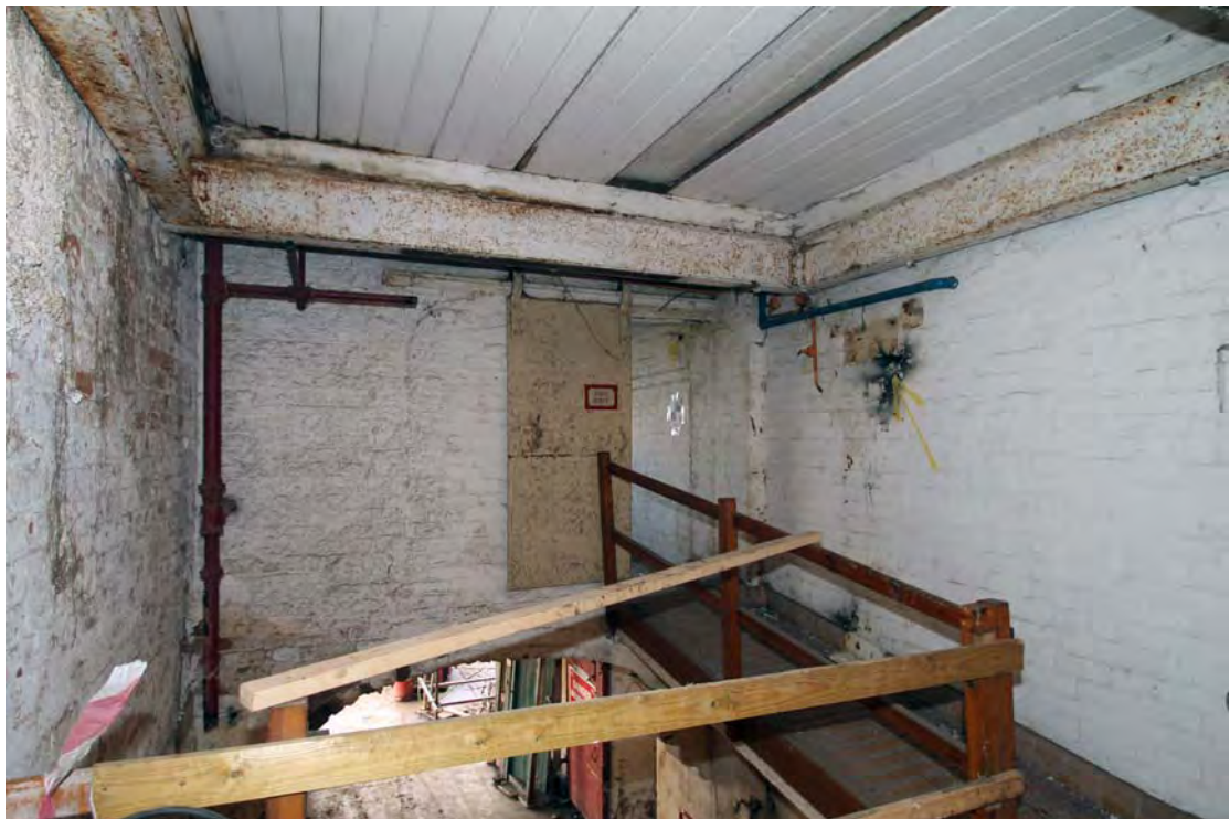
Plate 65. Building 4, first floor level, view from east.
