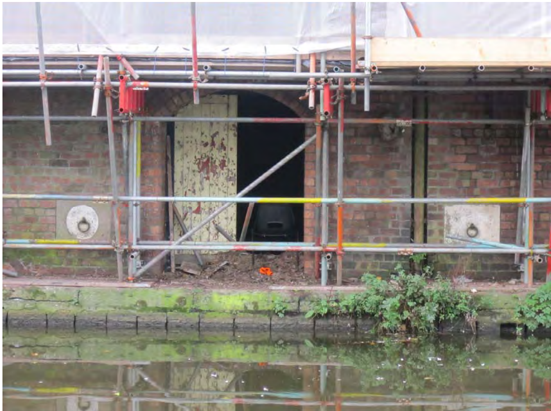
Plate 10. Boiler House central part (Building 9), viewed from north.
