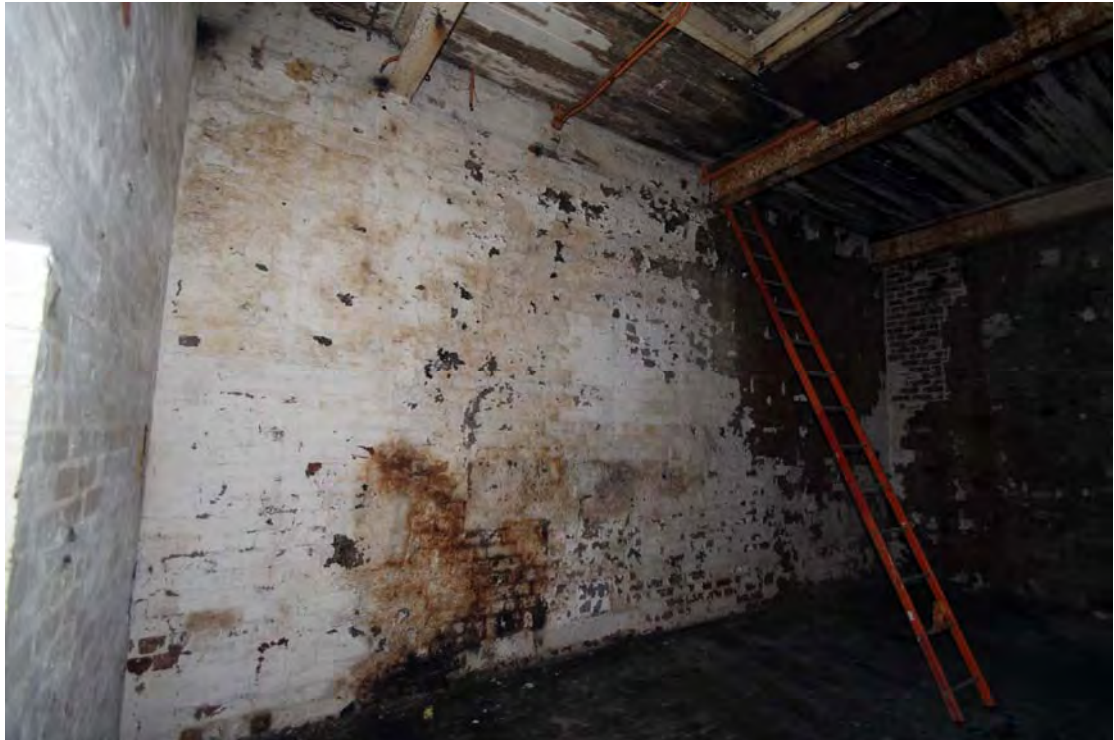
Plate 31. Engine House (Building 8), first floor, viewed from north-east, showing gritstone bed in centre.
