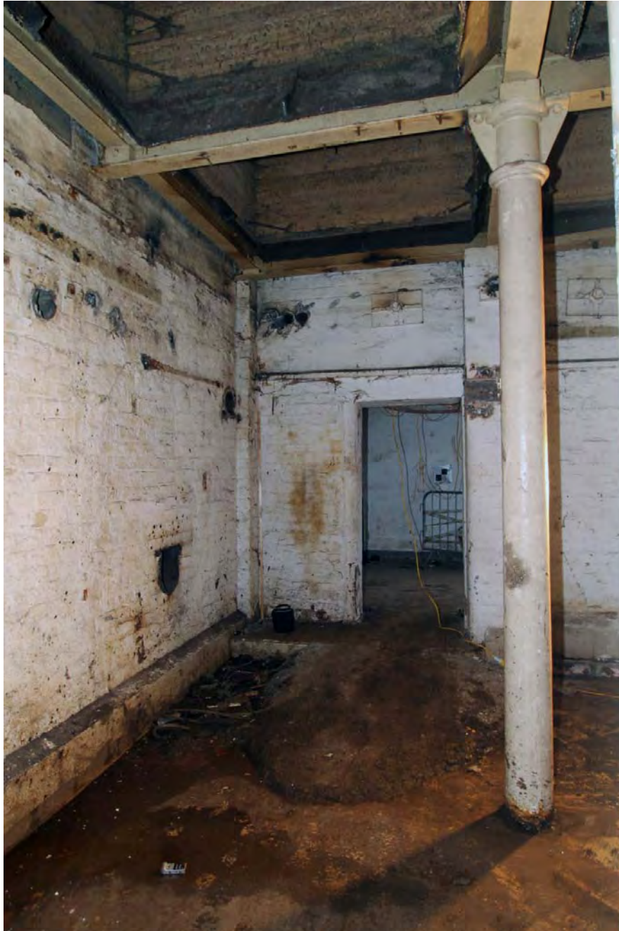
Plate 49. Building 17, ground floor, south end, viewed from north.
