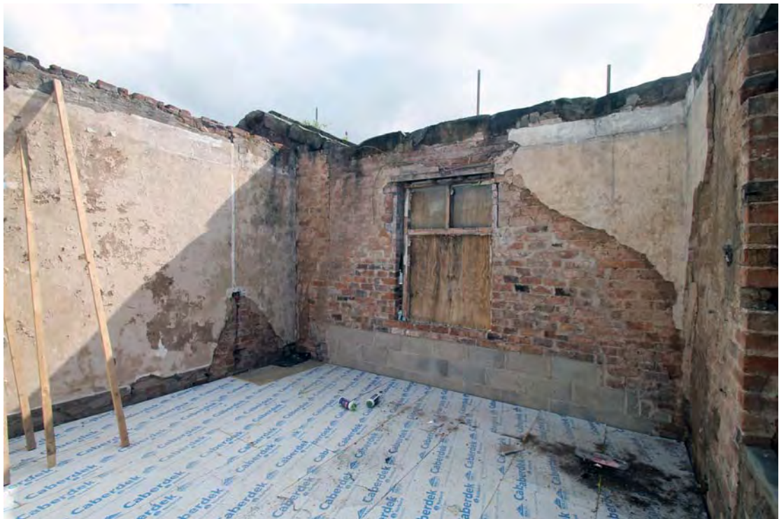
Plate 92. Mansion House, first floor, room F4, viewed from north.
