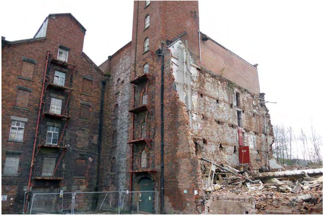
Plate 77. Warehouse Northern Bay (Building 1A), following demolition, viewed from south-west.
