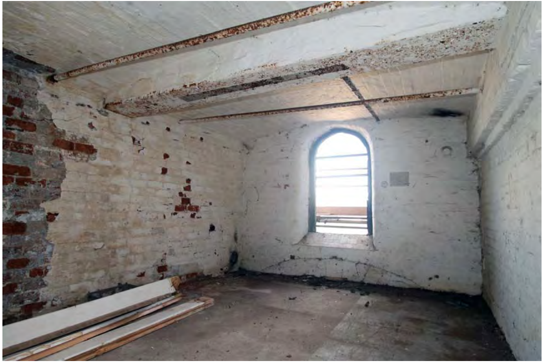
Plate 64. Building 5, first floor level, view from east.
