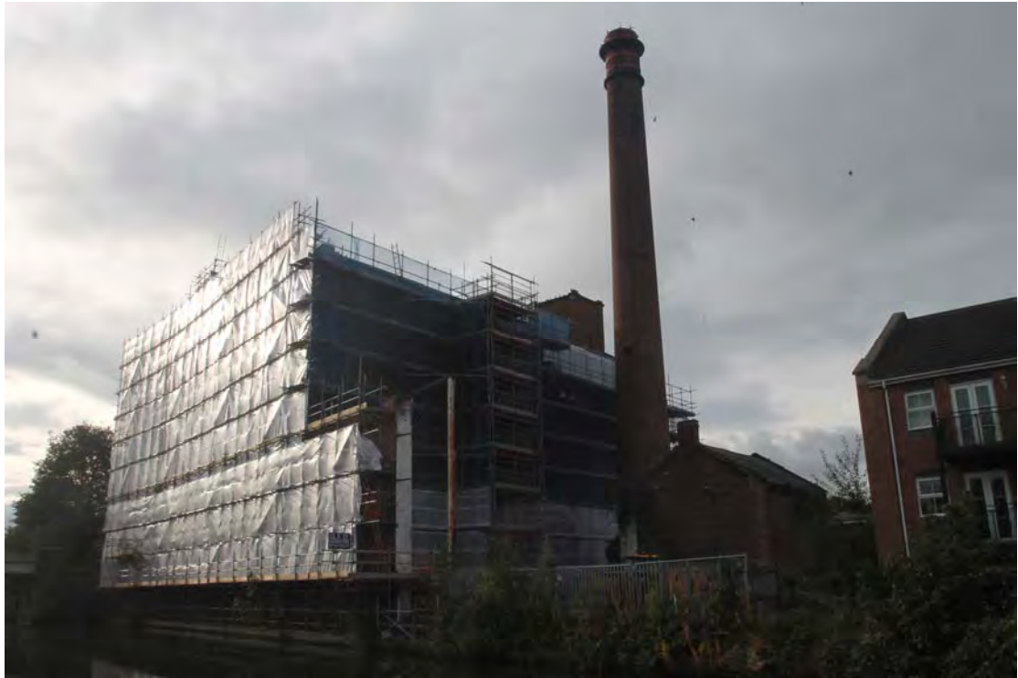
Plate 7. Mill viewed from north-west.
