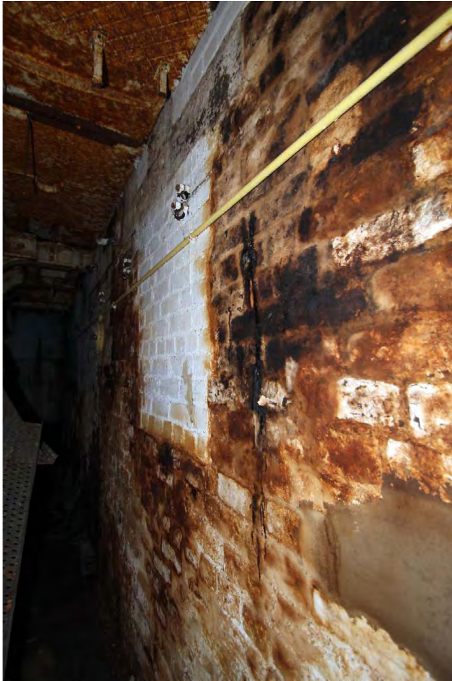
Plate 25. Engine House (Building 8), south wall, showing gearwheel housing, viewed from north-west.
