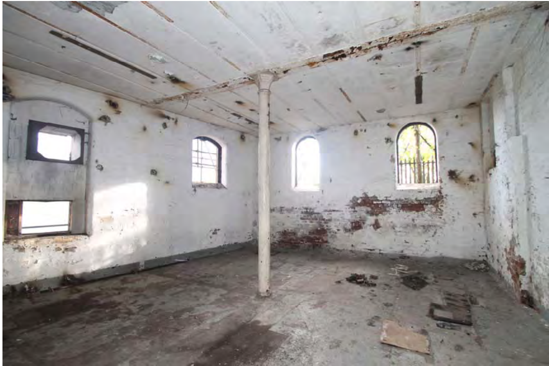
Plate 20. Boiler House upper floor (Building 9), viewed from south-west.
