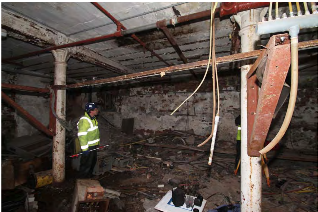
Plate 17. Boiler House ground floor (Building 9), viewed from north-west.
