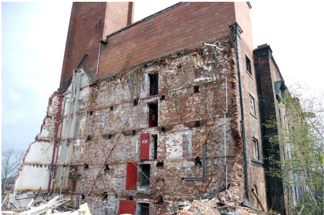
Plate 80. Warehouse Northern Bay (Building 1A), following demolition, viewed from south-east.
