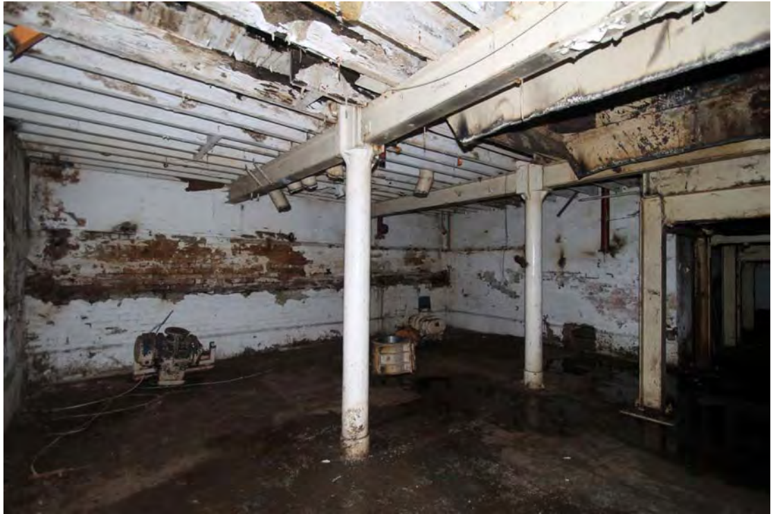
Plate 55. Building 10 (New Warehouse), ground floor, western part, viewed from south-east.
