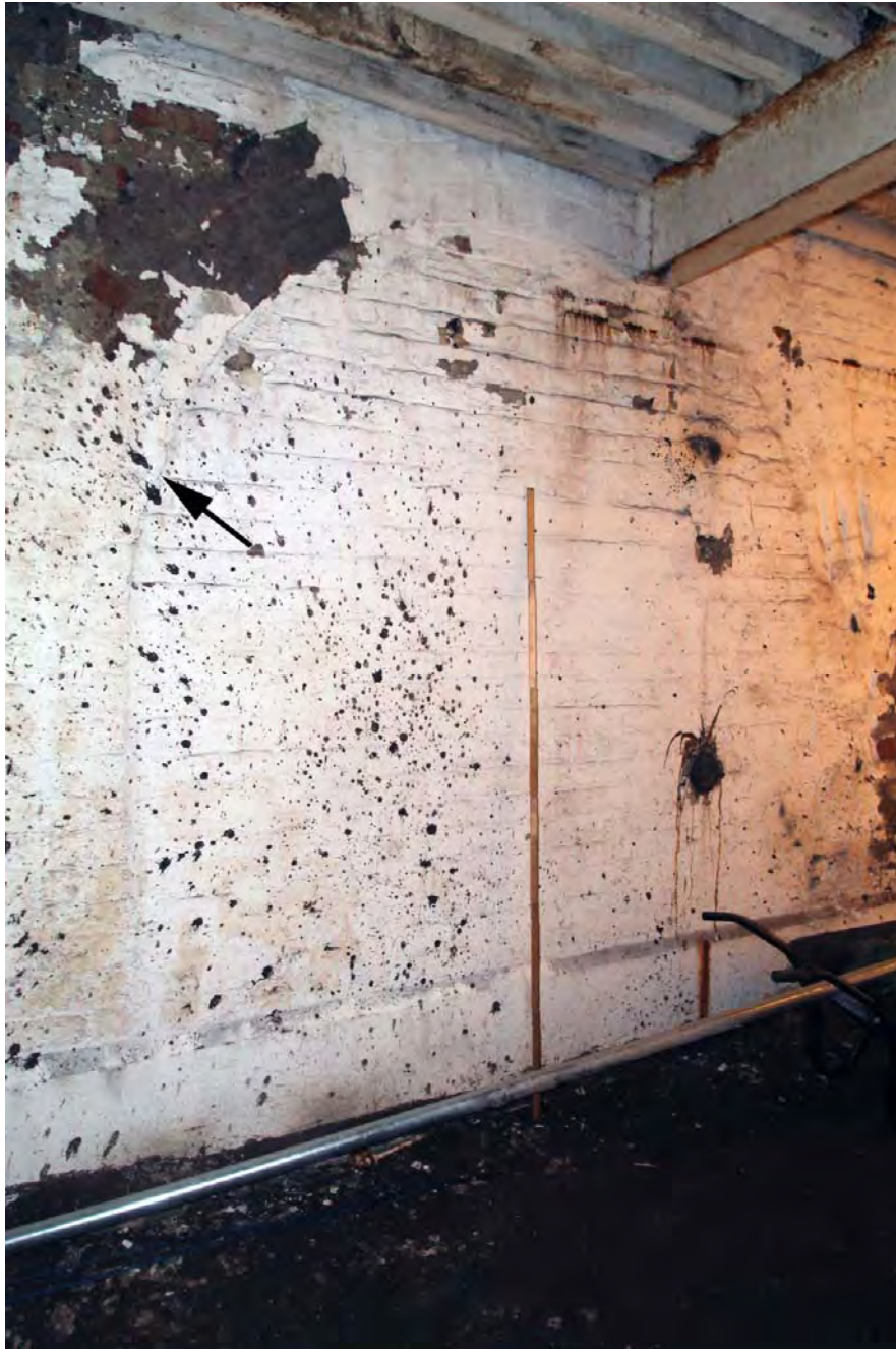
Plate 23. Original external Boiler House doorway, viewed in east wall of Building 10.
