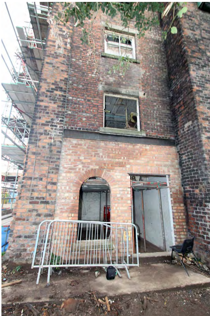
Plate 15. Building 2, viewed from east, after demolition of Building 1.
