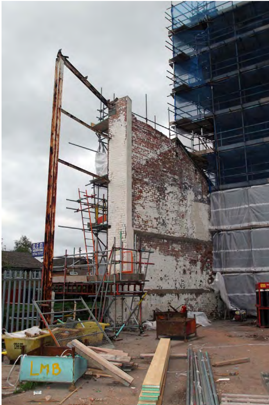
Plate 6. North internal elevation of Building 13, viewed from south-west.
