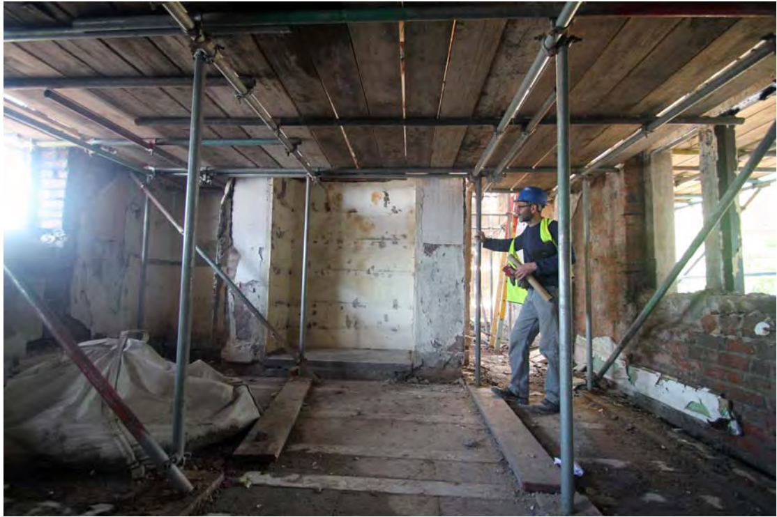
Plate 85. Mansion House, ground floor, Later Kitchen (Room G8), viewed from south.
