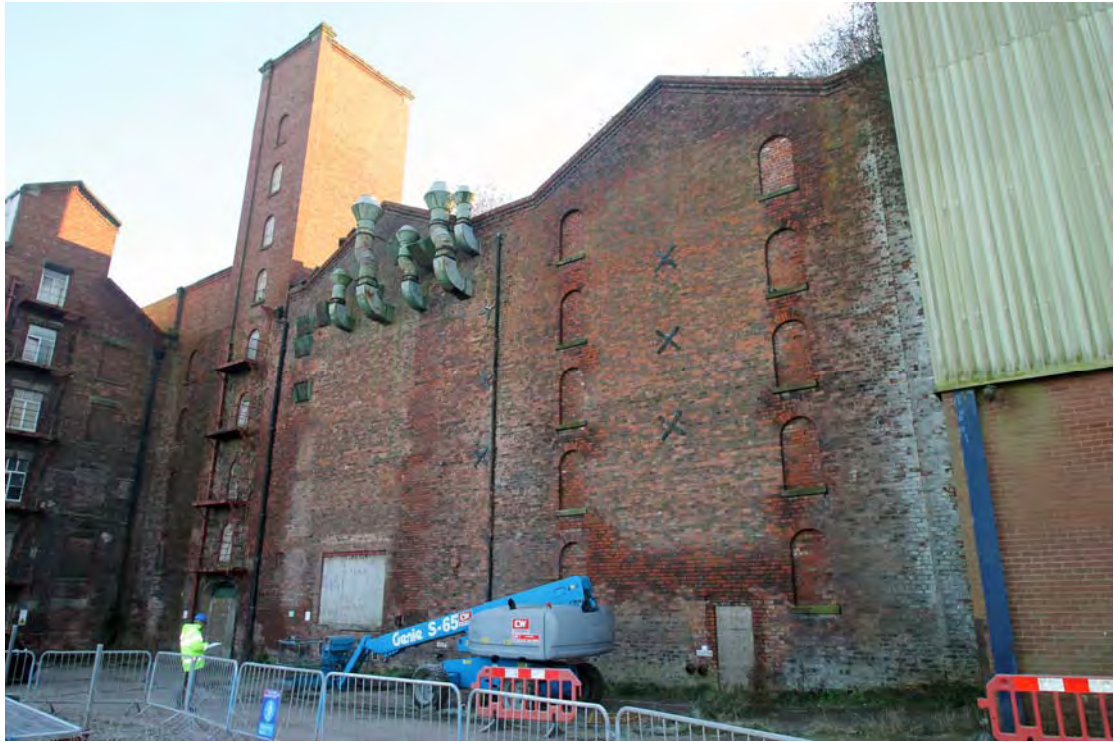
Plate 69. Warehouse Northern and Central Bay (Buildings 1A & 1B), viewed from south-west.
