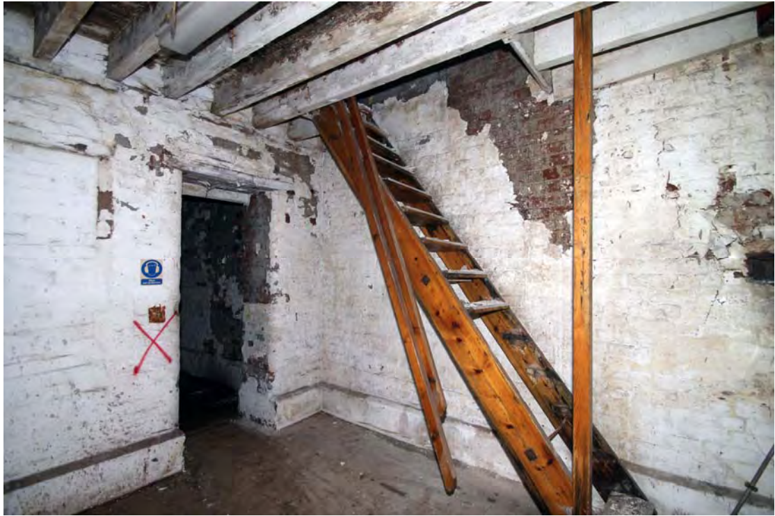
Plate 39. Stair Tower (Building 7), ground level, viewed from south-west.
