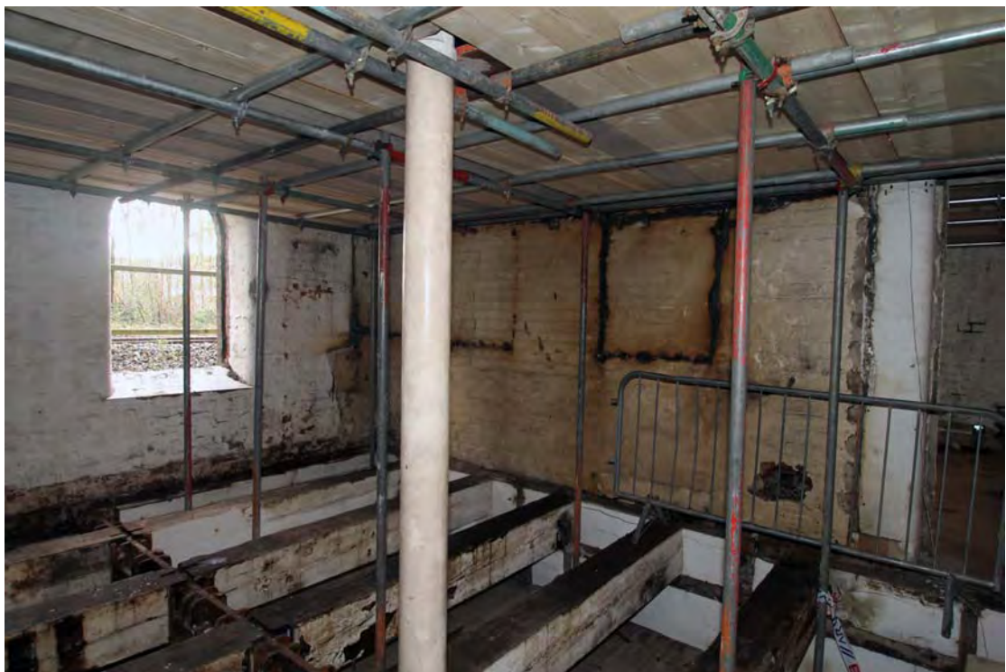
Plate 34. Original mill (Building 6), first floor, south-east corner, viewed from north-west.
