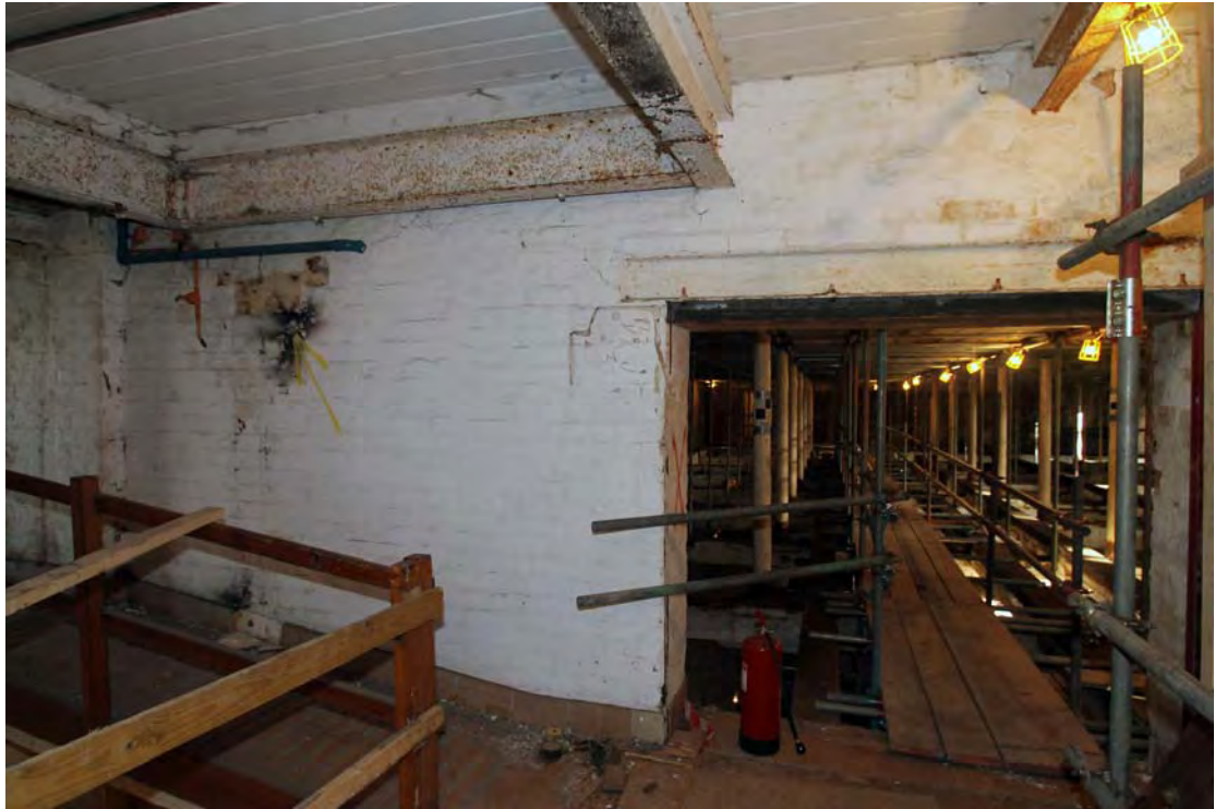
Plate 66. Building 4, first floor level, view from south, looking into Building 6.
