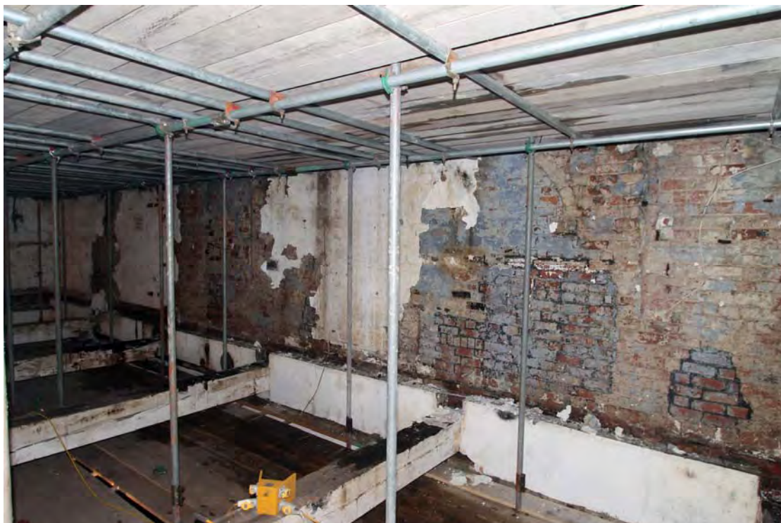
Plate 36. Original mill (Building 6), first floor, west wall, viewed from north-east, showing blocked windows.
