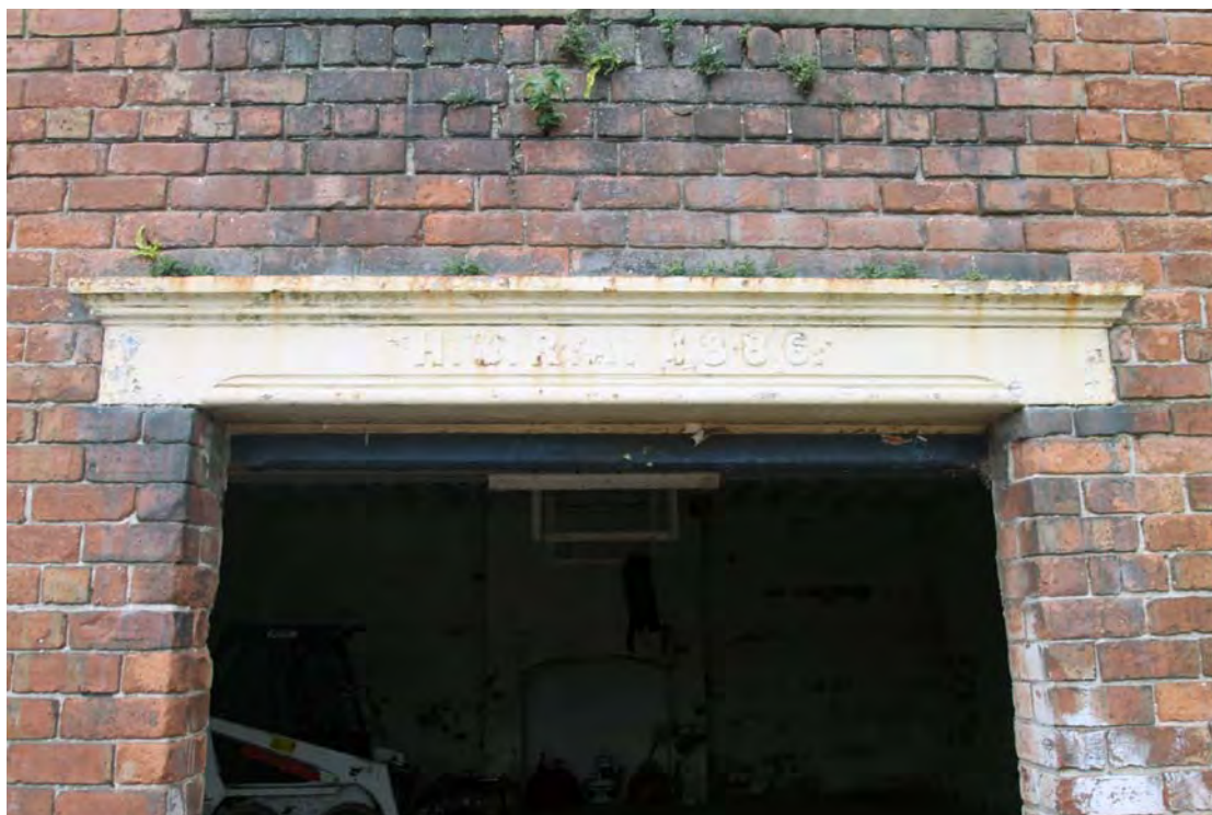
Plate 4. Building 19, south elevation, cast-iron lintel, viewed from south.
