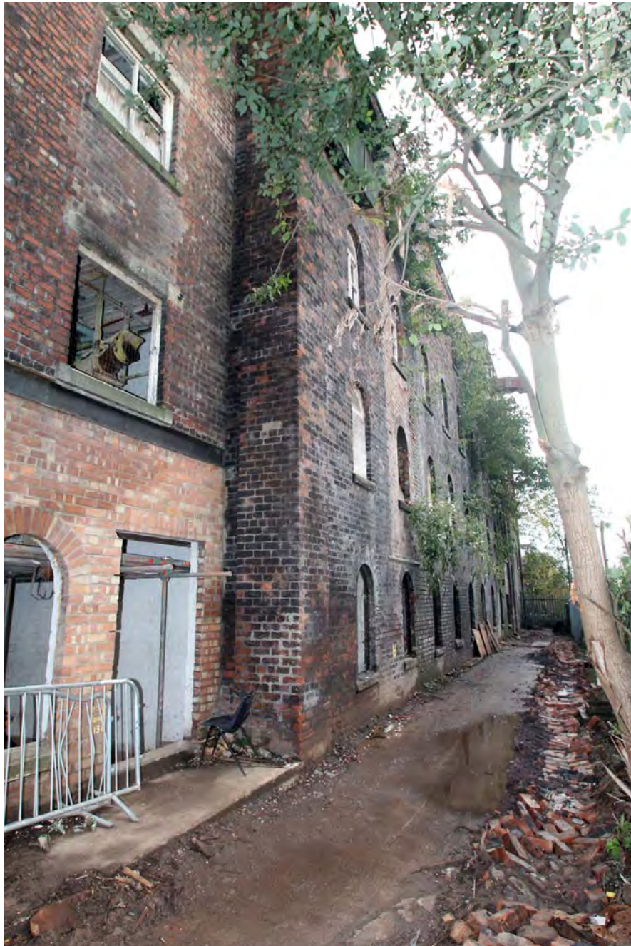
Plate 14. Building 6 (right), building 2 (left), viewed from south-east.
