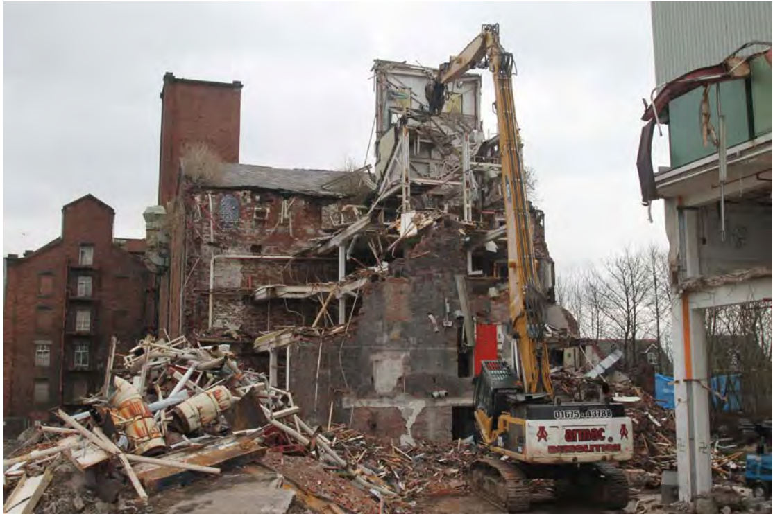
Plate 71. Warehouse Southern Bay (Building 1C) under demolition, viewed from south.
