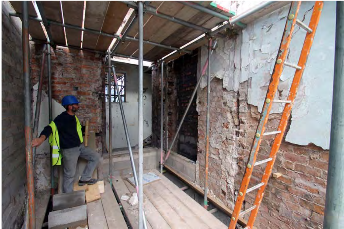
Plate 89. Mansion House, first floor, room F1, viewed from south.
