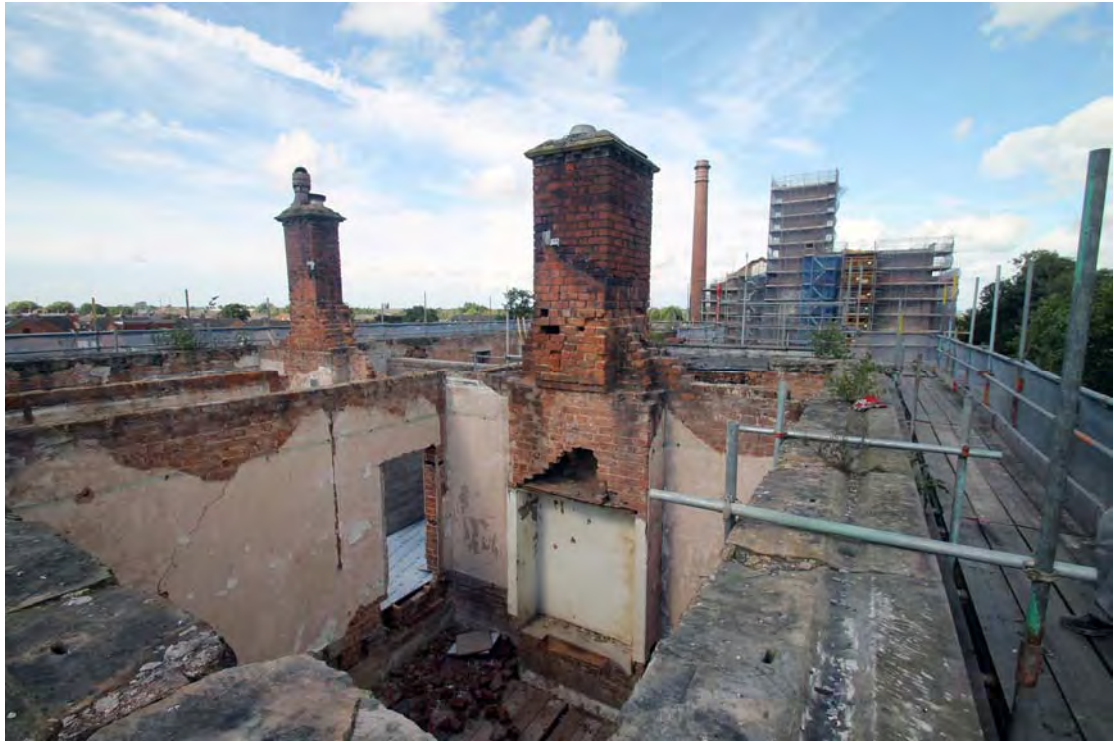
Plate 97. Mansion House, first floor, view over room F2, viewed from south-east.
