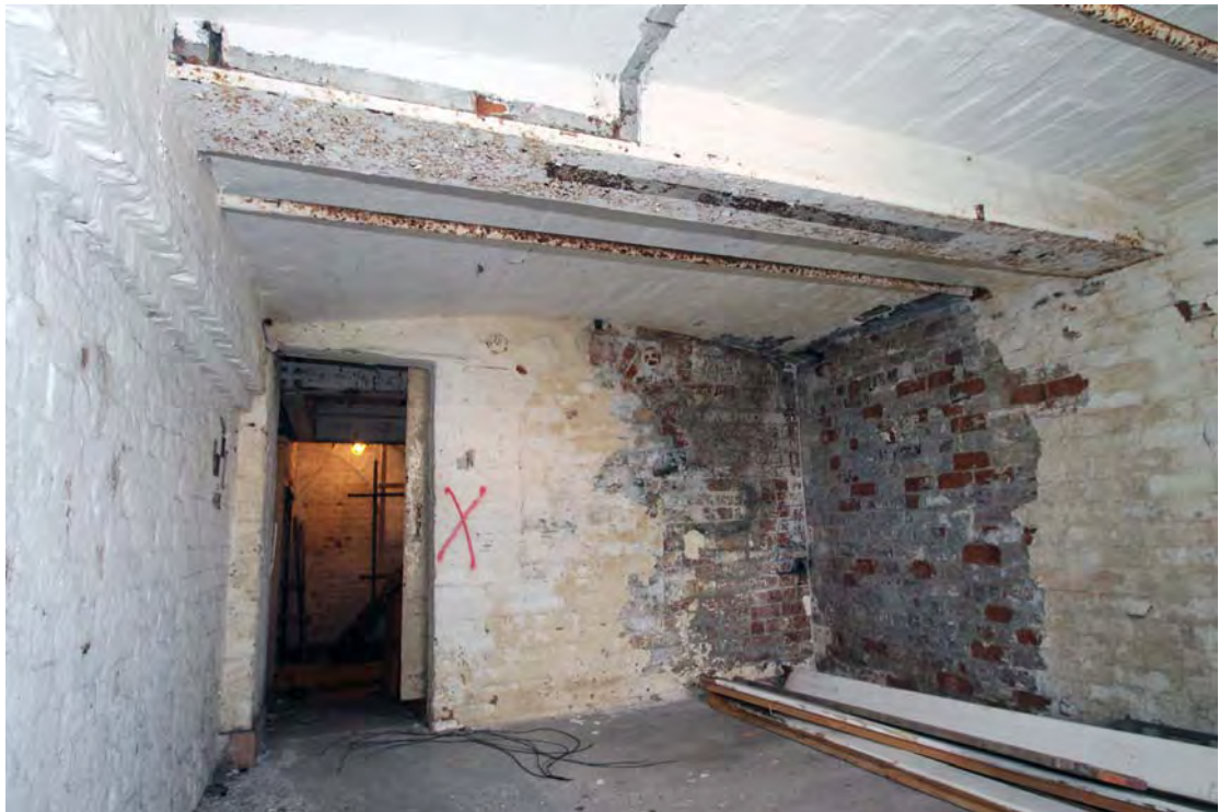
Plate 63. Building 5, first floor level, view from west.
