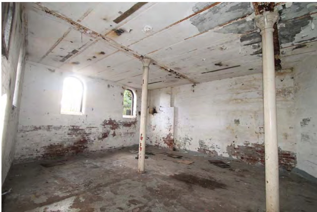
Plate 21. Boiler House upper floor (Building 9), viewed from north-west.
