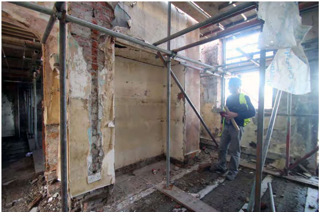
Plate 86. Mansion House, ground floor, Room G9, viewed from north-east.
