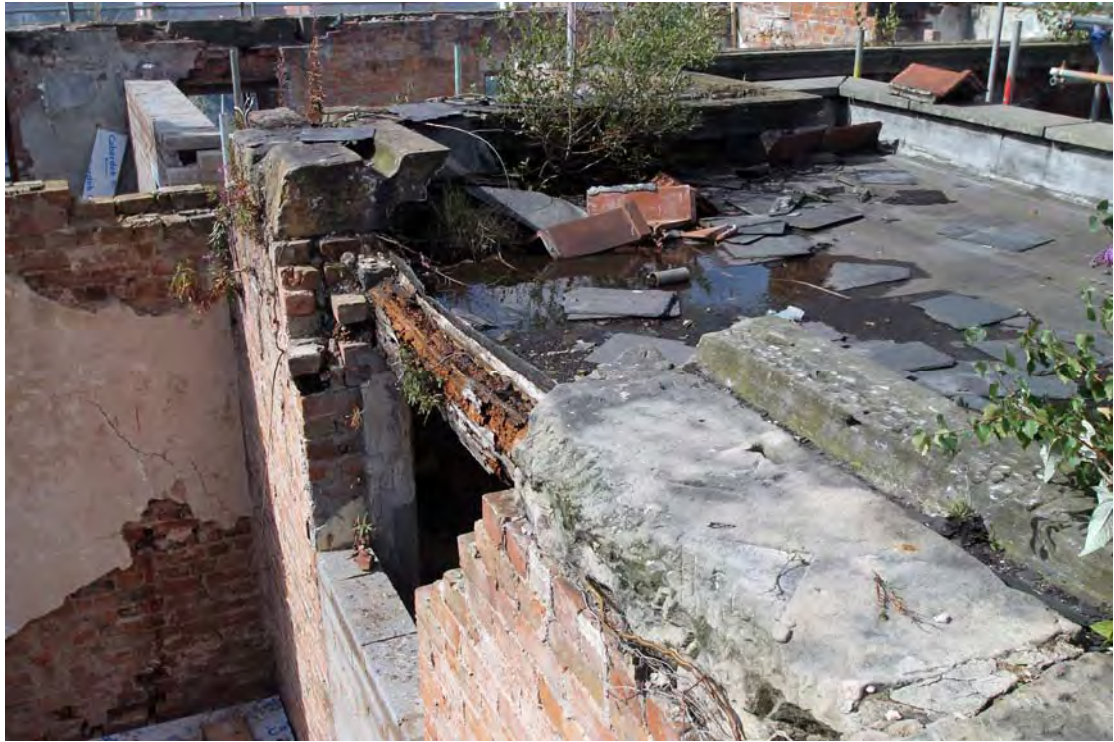
Plate 101. Mansion House, first floor, view over room F7, viewed from south-east.
