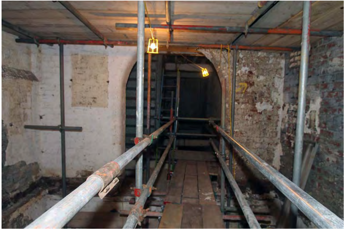
Plate 41. Stair Tower (Building 7), first floor, viewed from north.
