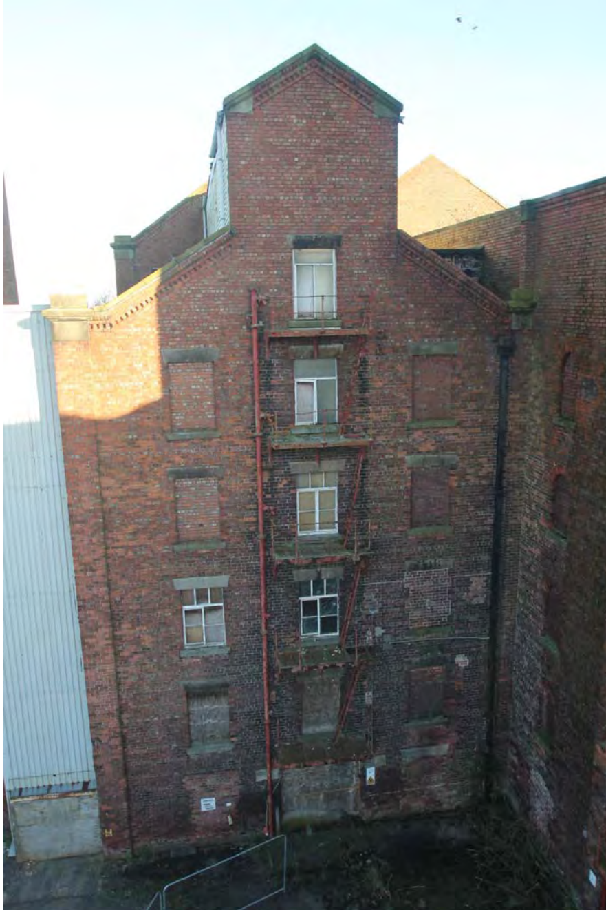
Plate 54. Building C, south elevation, viewed from cherry picker.
