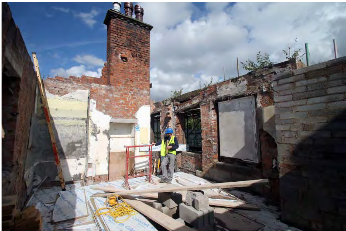
Plate 94. Mansion House, first floor, room F8, viewed from south.
