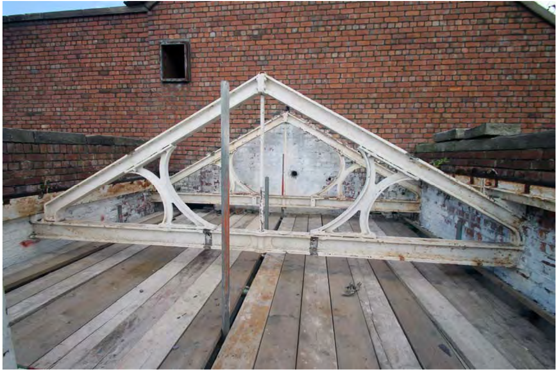
Plate 51. Building 17, roof level, showing cast-iron roof trusses, viewed from south.
