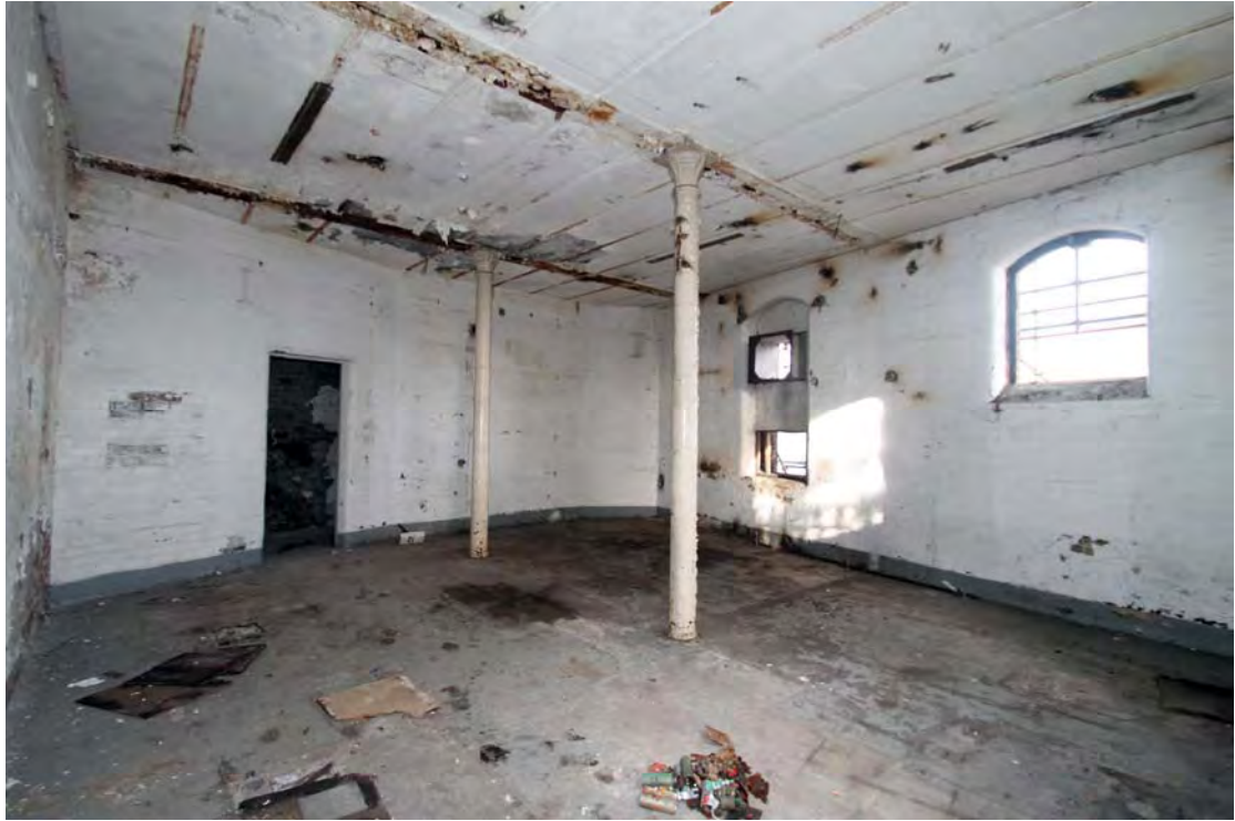
Plate 22. Boiler House upper floor (Building 9), viewed from south-east.
