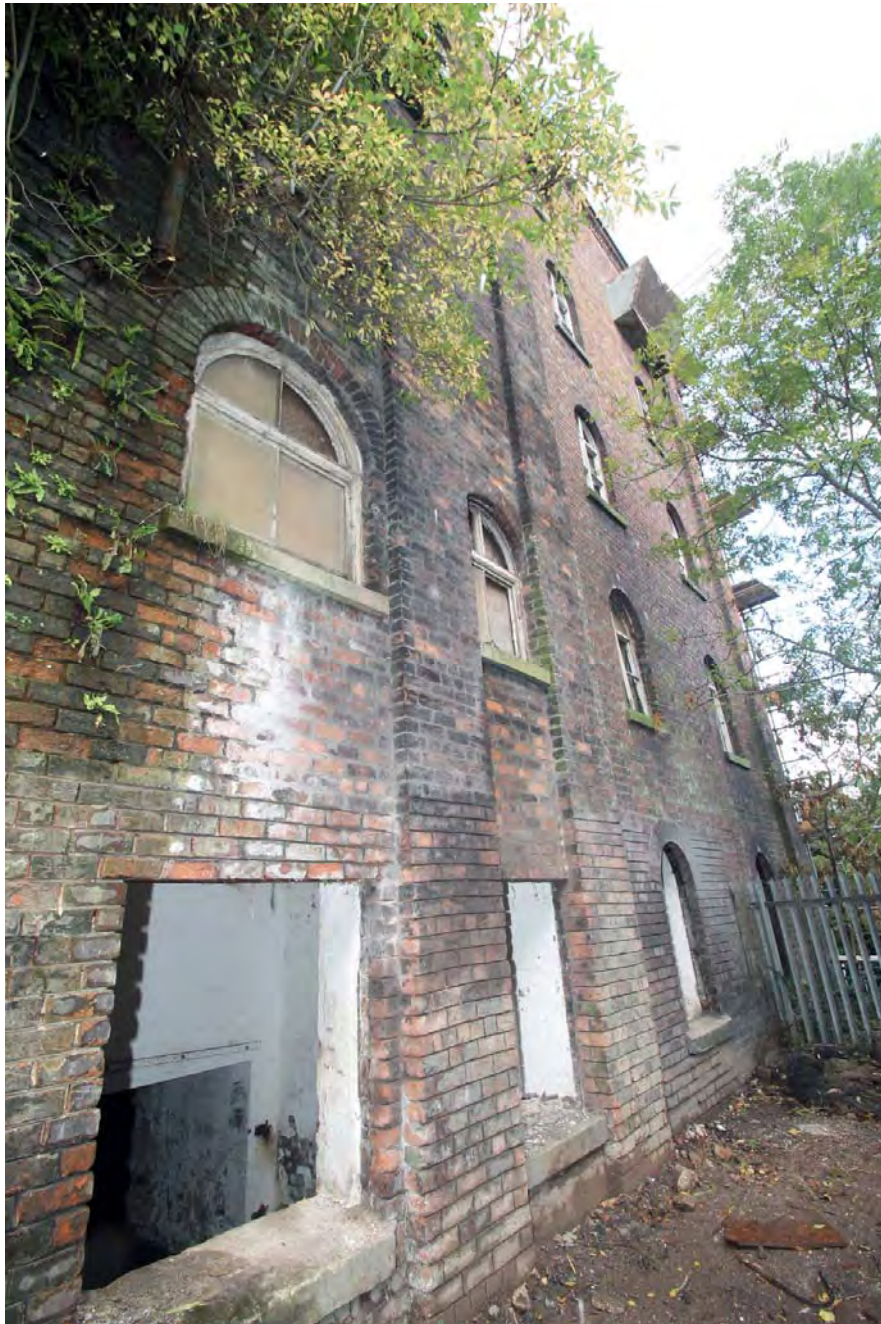
Plate 13. Partially blocked windows of Building 8 (Beam Engine House), viewed from south-east.
